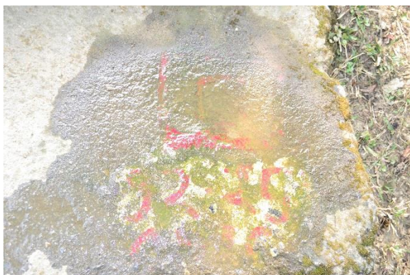
CWC. HFL point near Golaghat pump house (ch 82.87)
