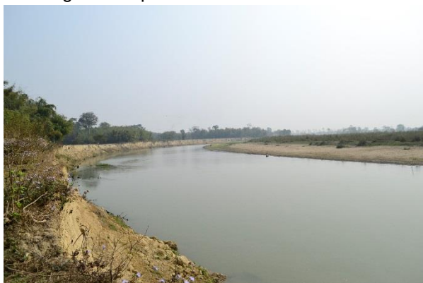
Bathali Kuha No.1 village Critical area
