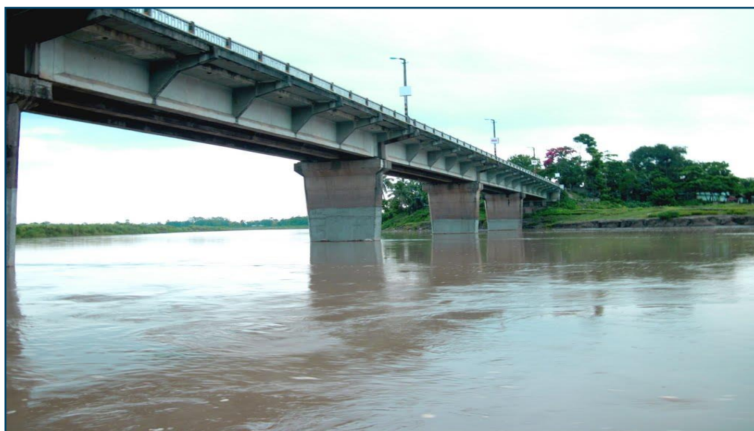
Figure 23 Rajabari Rail Bridge (Ch 51.57 km)
