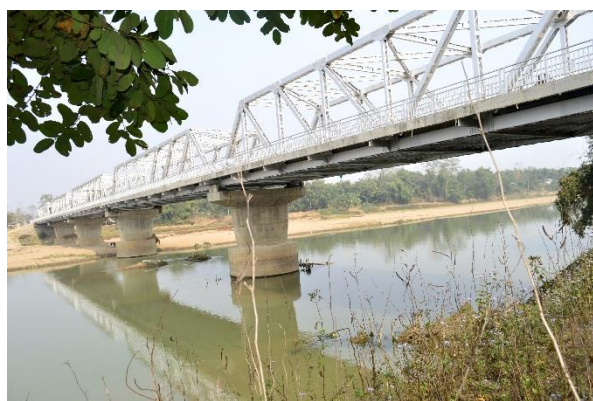
Dhansari Bridge no-2 (Ch. 79.83)
