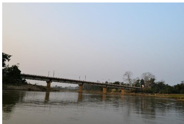
Golaghat Bridge (Ch 82)
