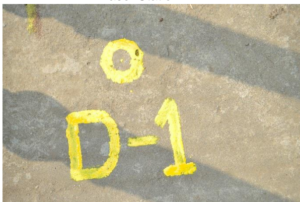
Banch Mark transfer point
