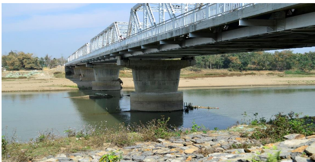
Figure 32 Example of protected bank in Dhansiri River near Still Bridge
