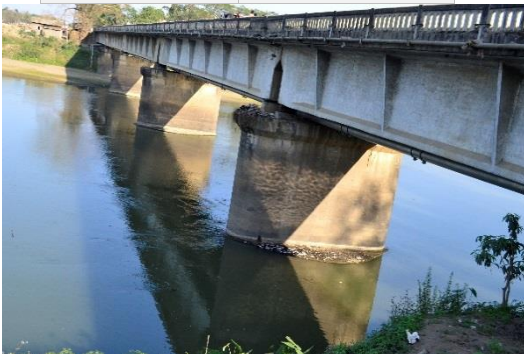
Figure 20 Numaligarh RCC Bridge (ch. 31.16)
