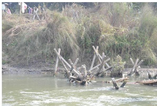
Porcupines nera to Golaghat Bridge (Ch 33.04)
