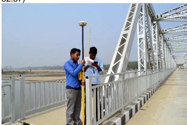
Marking the BM near Dhansari Bridge no-2 (Ch. 79.83)
