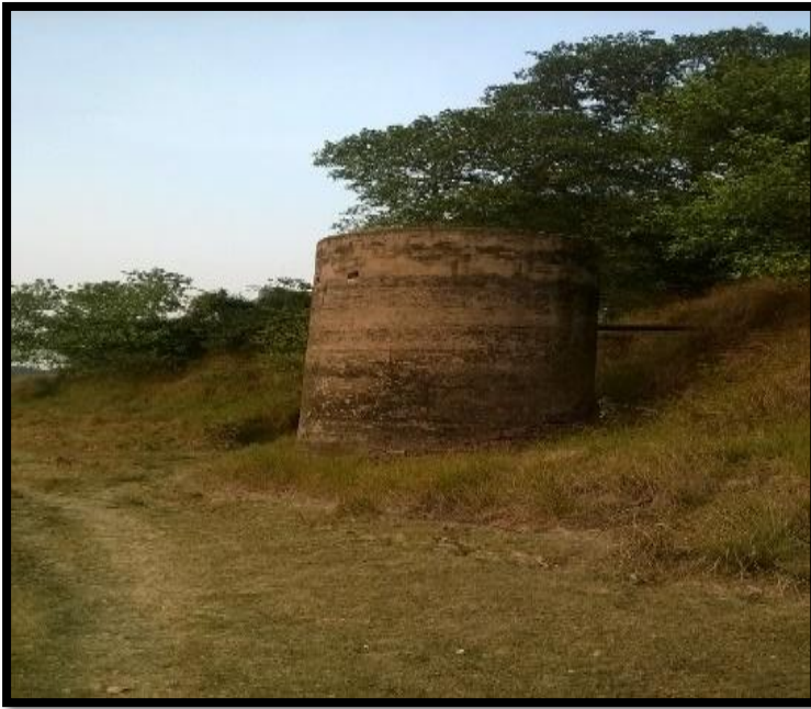
Well at Ch. 82.15 km
