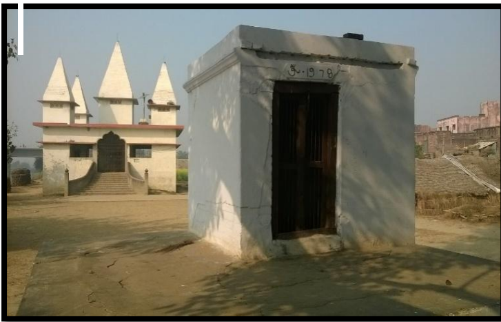
Shiv Temple at Ch 71.10 km
