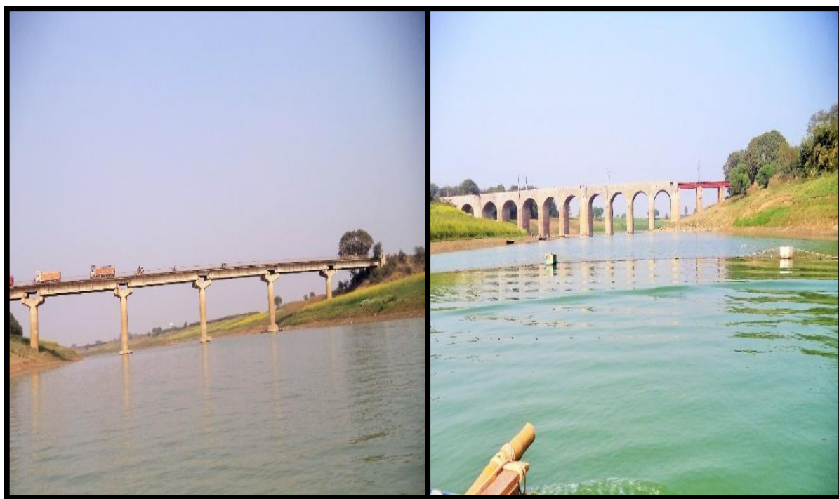
Chausa Bridge at Ch 2.35 km & Chausa Rail Bridge at Ch 3.48 km
