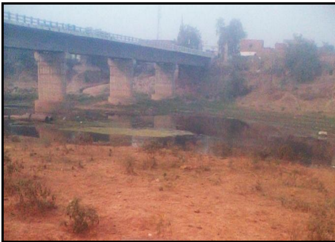
Kakarait Bridge at Ch. 85.98 km
