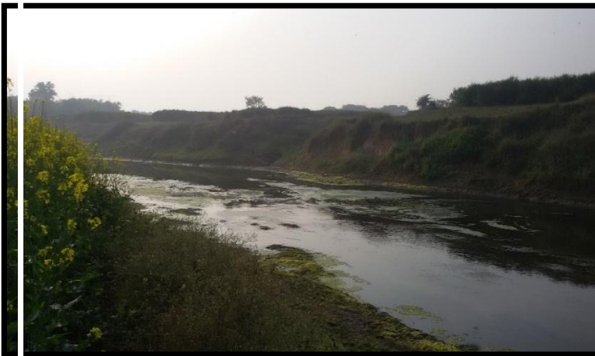
Shallow depth at Ch 43.0 km
