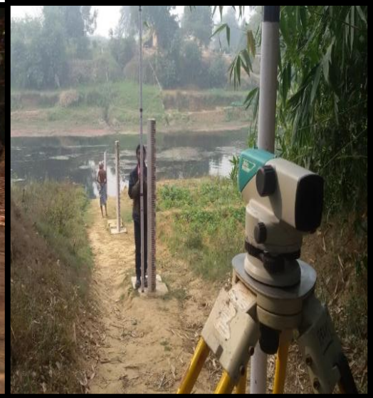
Levelling Between BM & TBM
