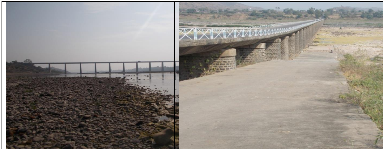
Figure 2.26 – View of Akteshwar and Gora Bridge
