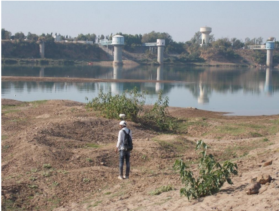
Figure 2.16 – Water Intake pump house of NTPC
