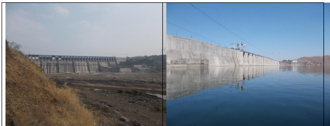
Figure 2.2 – Downstream and Up-stream view of Sardar Sarovar Dam
