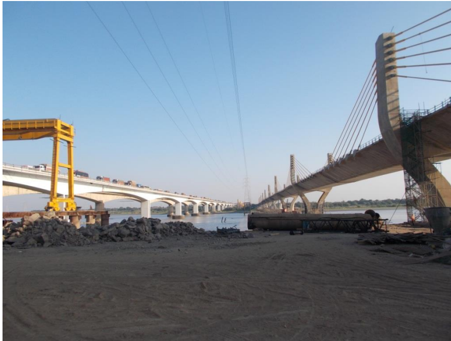
Figure 2.12 – Bridges at Jadeshwar
