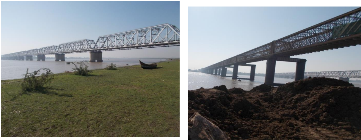
Figure 2.11 – Railway and Road Bridge at Bharuch
