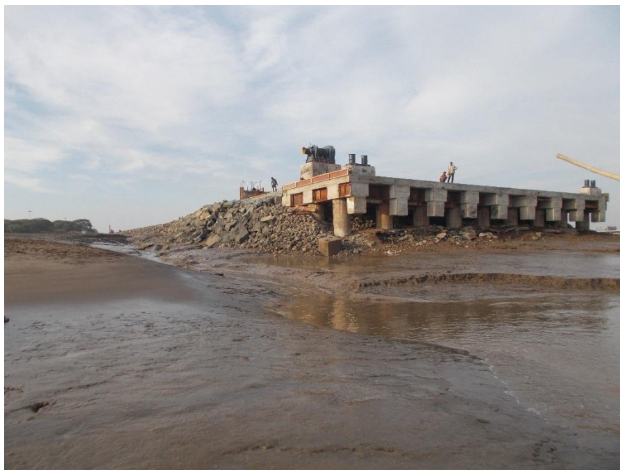
Figure 2.6– View of under- construction Godrej Jetty
