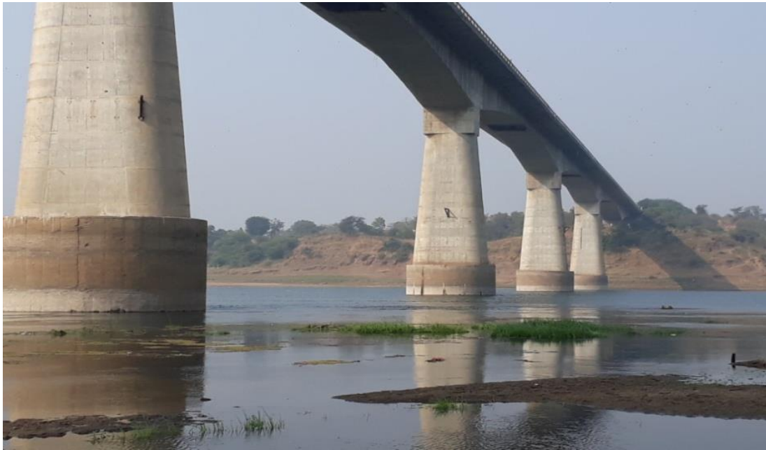
Figure 2.21 – Poicha Bridge near Chandod
