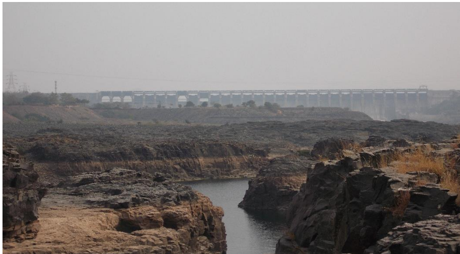
Figure 2.28 – Rocky portion at downstream of Sardar Sarovar Dam
