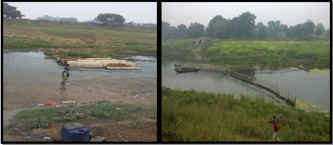
RCC pipe at Ch.18.00 & Bamboo barrier at Ch. 20.50 km
