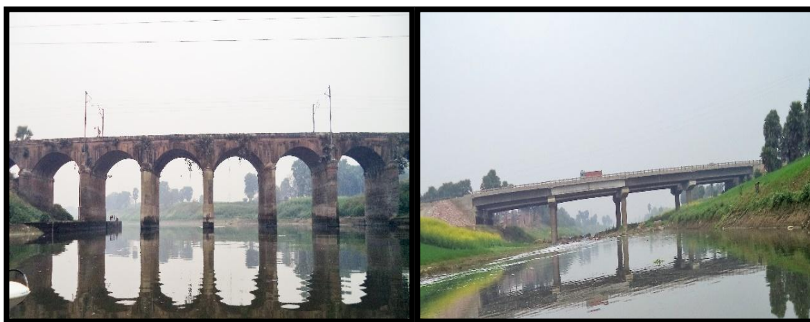
Fatuha Rail Bridge at Ch 1.17 km & Naryan Bridge at Ch 5.32 km
