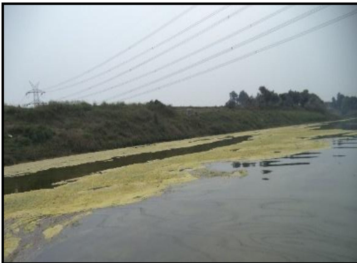
HT Line at Ch 27.10 km
