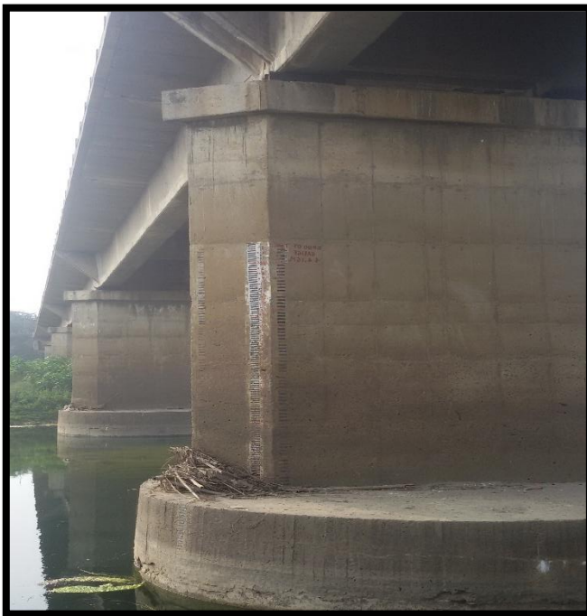
Bench Mark at Gaurichak Punpun Bridge
