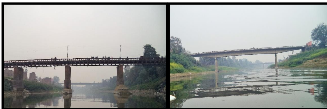
Loha Bridge at Ch 0.57 km & New Bridge at Ch 0.87 km
