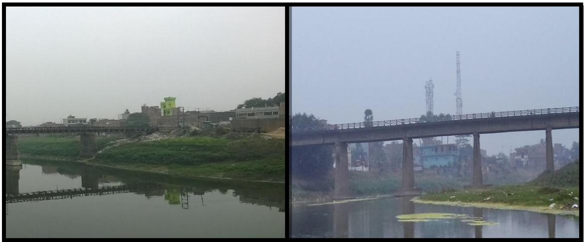
Houses at Ch 0.56 km & Ch 21.8 km
