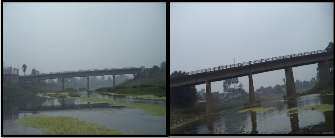
Fatehpur Bridge at Ch 18.12 km& Gourichak Bridge at Ch 21.8 km
