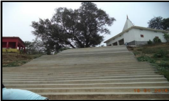
Pitch protected at Ch. 27.30 km
