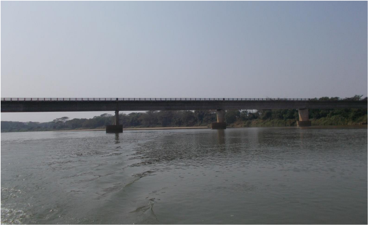
Figure 31: Kalapada bridge at CH: 30.3km
