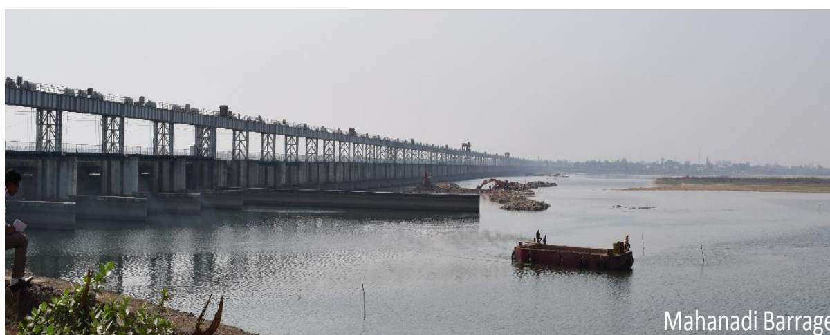
Figure 21: Jobra Barrage (CH: 100km) across Mahanadi River
