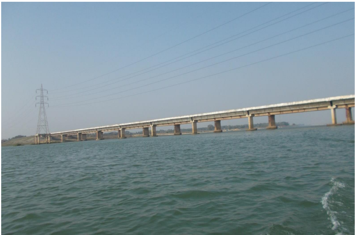
Figure 34: Marshaghai NH bridge at CH: 20.8km
