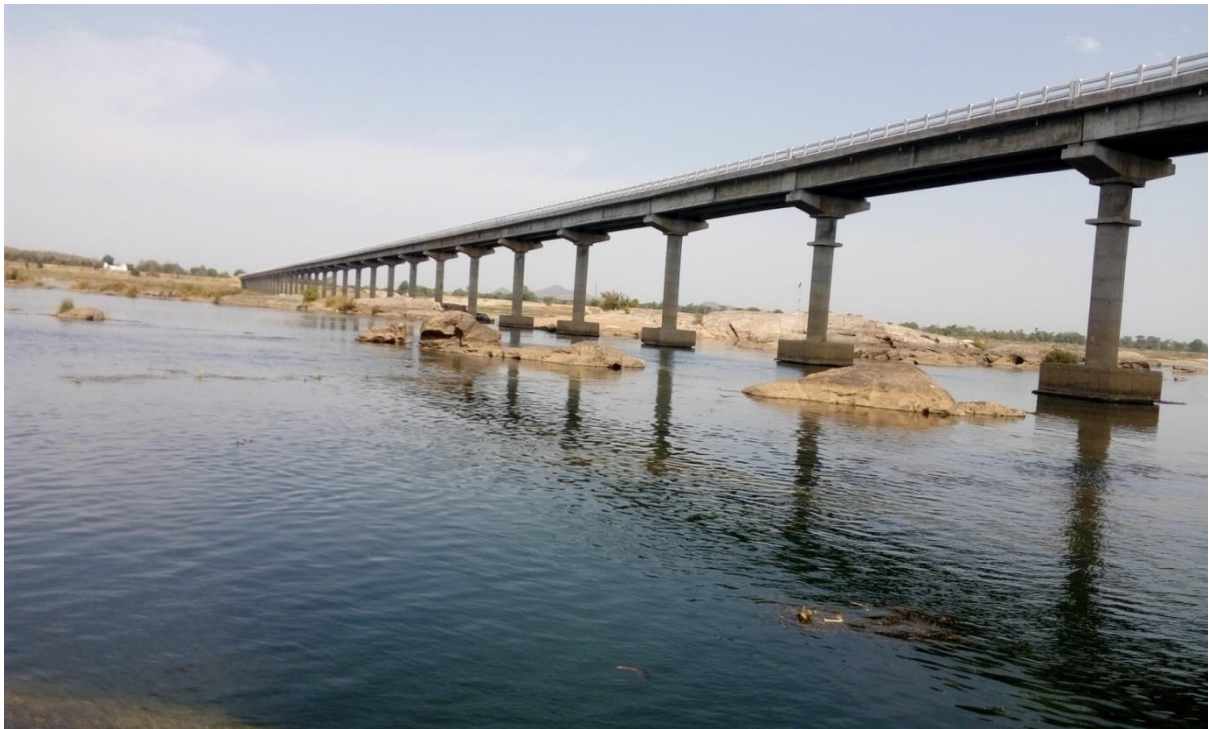
Figure 25: Binka bridge at CH: 381km
