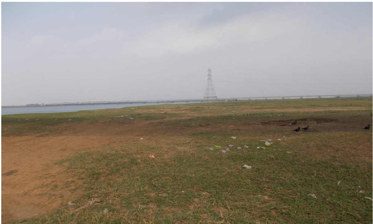
Figure 16: Bhutamundeï Rail Bridge (CH:16.5km) across Mahanadi River
