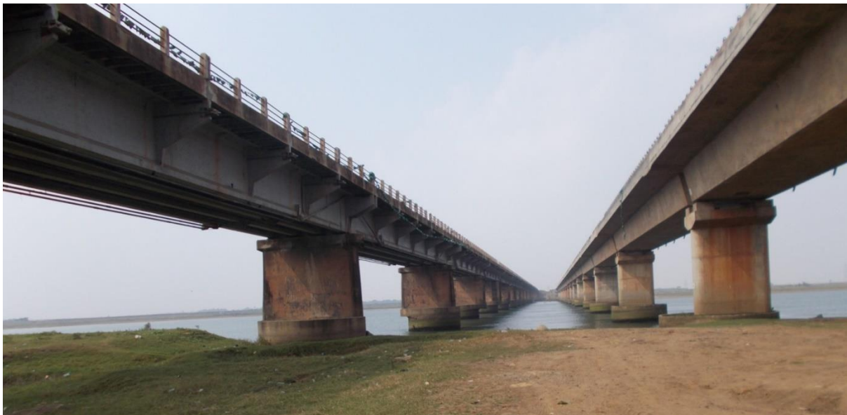
Figure 14: Bhutamundei Bridge (CH:17.4km) across Mahanadi River
