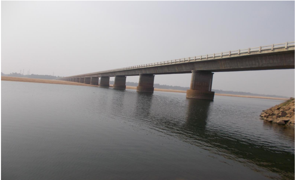
Figure 17: Kessann Nagar Bridge(CH: 79.2km) across Mahanadi River
