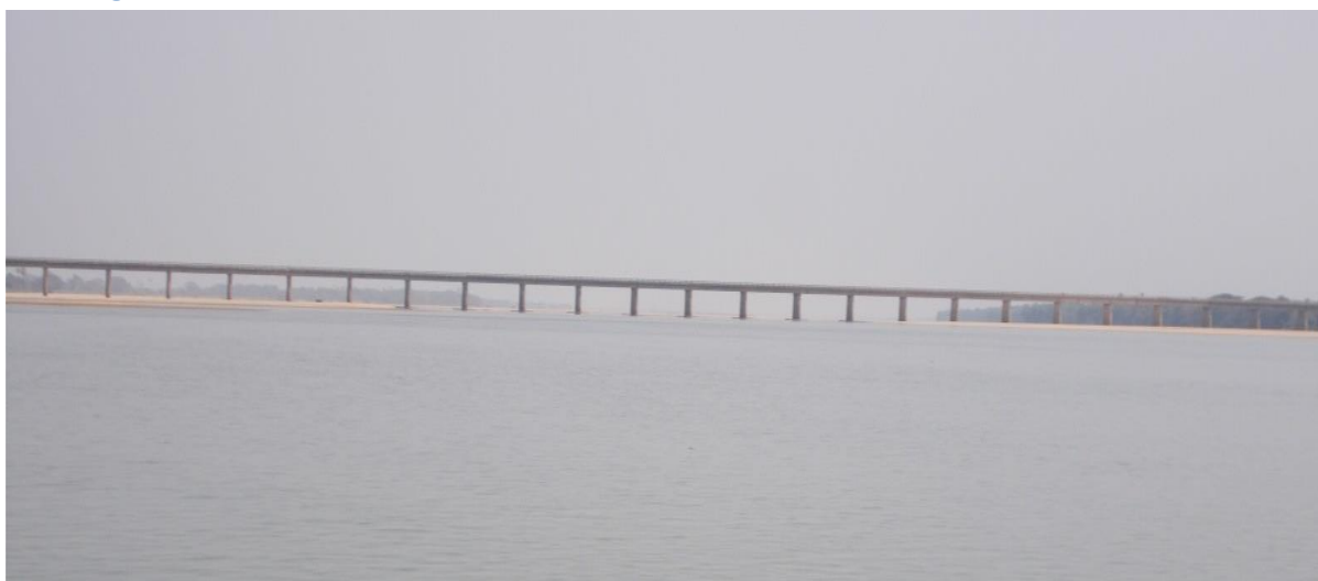
Figure 29: Sisua bridge at CH: 76.25km
