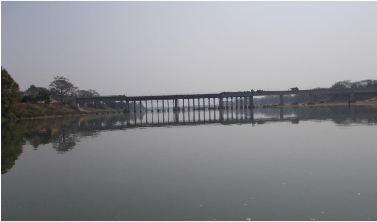
Figure 33: Basapur bridge at CH: 40km
