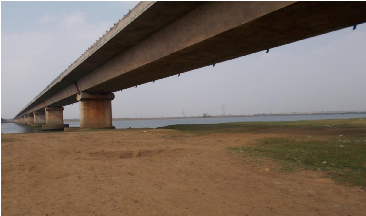
Figure 15: Bhutamundeï NH Bridge (CH:17.6km) across Mahanadi River
