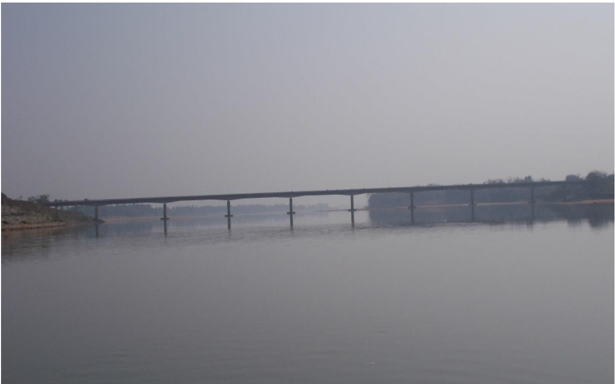
Figure 32: Ashureswar bridge at CH: 54.5km
