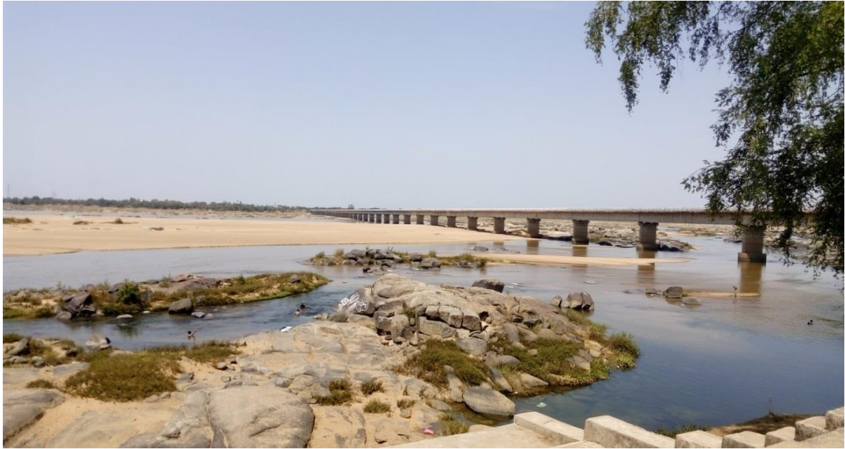
Figure 24: Sonepur bridge at CH: 357km
