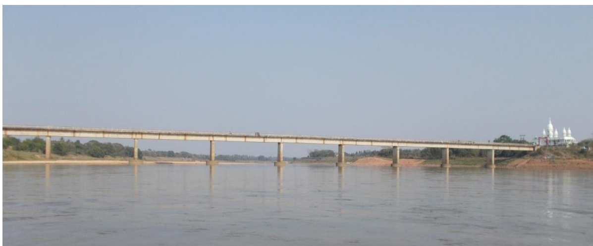
Figure 30: Barpada bridge at CH: 63km
