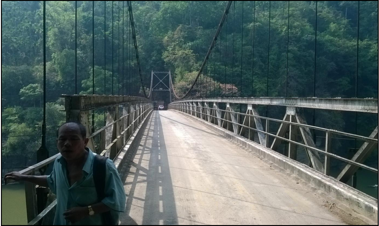
Figure 6 Steel Bridge (Chainage- 0.681 km)
