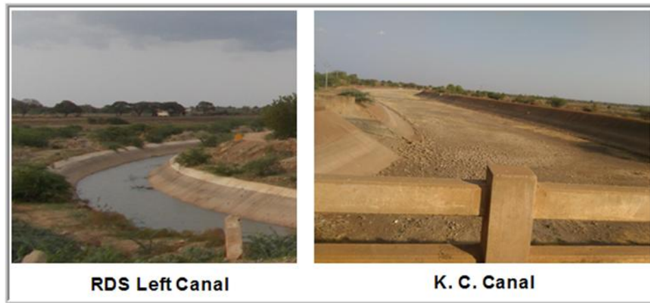
Figure 46 - Irrigational Canals (133.8 & 59.8 km chainage)
