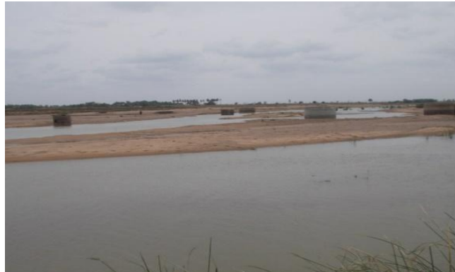
Figure 27 - Pump Wells View
