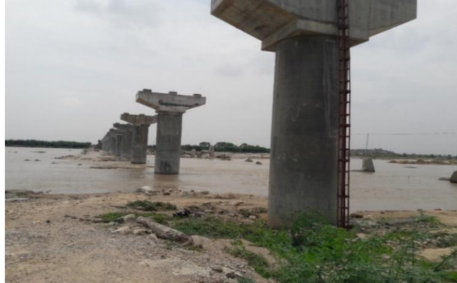
Figure 21 - Under Construction Bridge at Nagaladdine (ch. 90.96km)
