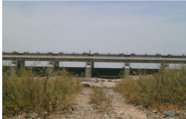
Figure 15 - Sunkesula Barrage downstream view (ch. 60.27km)
