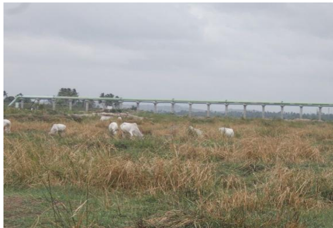
Figure 37 - BTPS Pipeline near Hebbal (ch. 228.08km)
