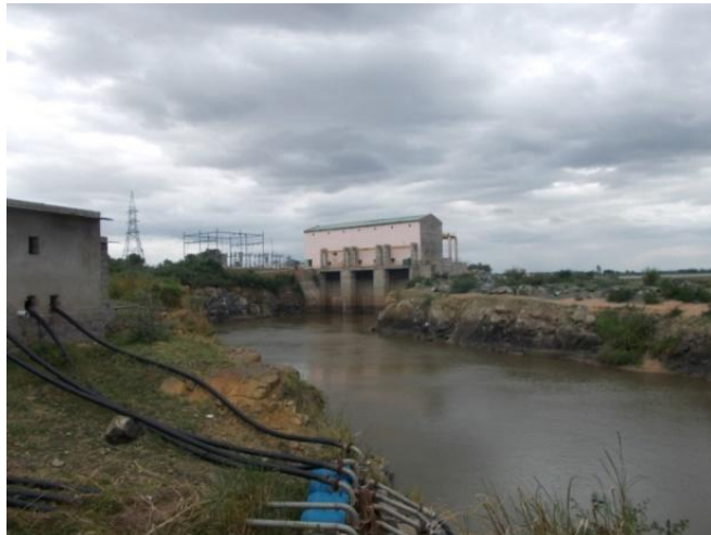
Figure 33 - Check Dam near Ulenoor (ch. 211.08km)
