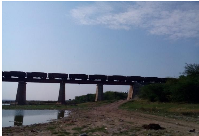
Figure 12 - View of Railway Bridge Kurnool (ch. 33.93km)
