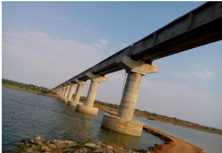
Figure 9 - View of Bridge at Alampur from Left Bank (ch. 17.17km)
