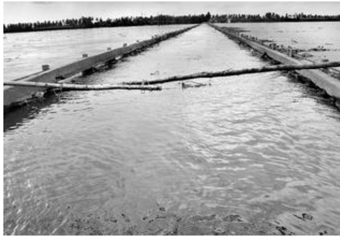
Figure 36 - Kampli Bridge submerged (News paper Source:- Hindu 4 Sep 2011)
