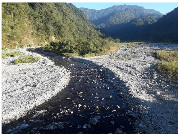
View of from Parashuram Kund Bridge Ch 86.00
