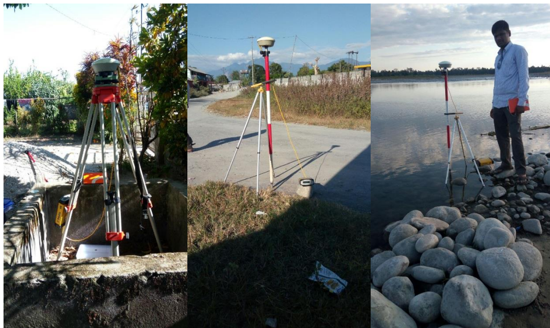
Figure 20 Topographic survey using RTK along Lohit River
