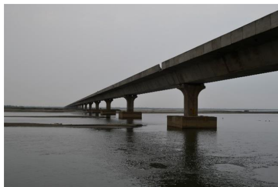
Alubari Bridge across Lohit River Ch. 47.0 km
