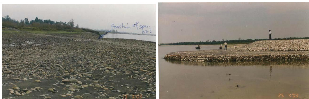
Figure 14 Spur in Lohit river before and during construction near Suparna (Source: North Eastern Council (NEC) Evaluation of NEC funded projects in Arunachal Pradesh report)
