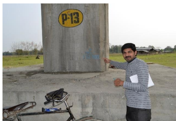
Showing HFL level at Lohit River Bridge at Dhola Ch. 5.36
