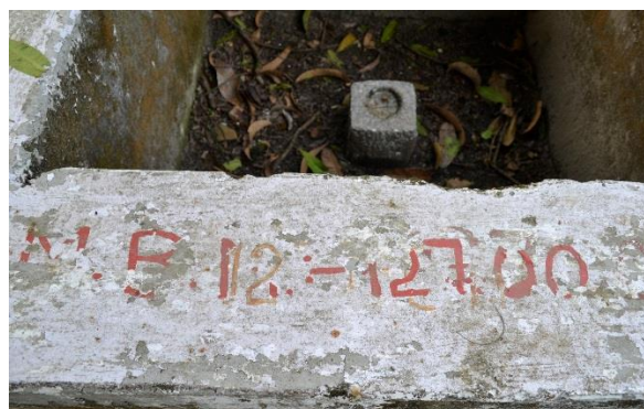
Bench mark at CWC office, Dhola(Ch. -6 km approximately)
