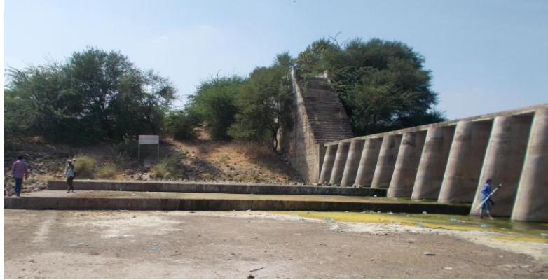
Figure 25 - Saradgi Barrage (138.85 km chainage)
