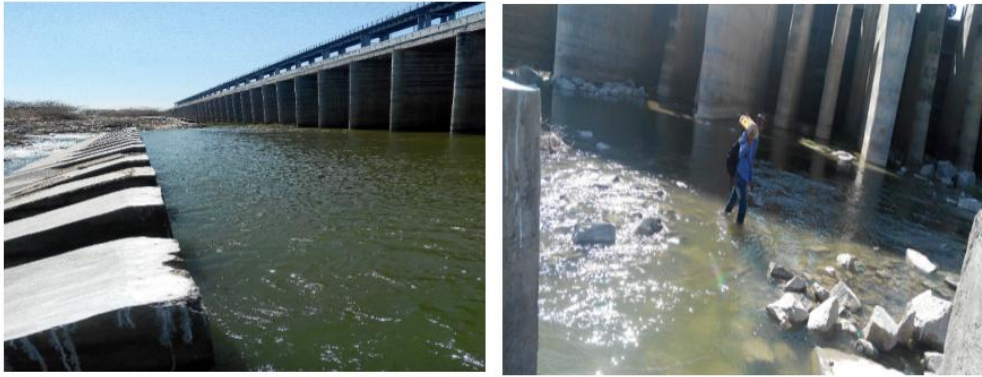
Figure 19 - Sonthi Barrage (75.22 km chainage)
