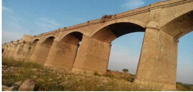
Figure 18 - Yadgir Bridge (50.08 km chainage)
