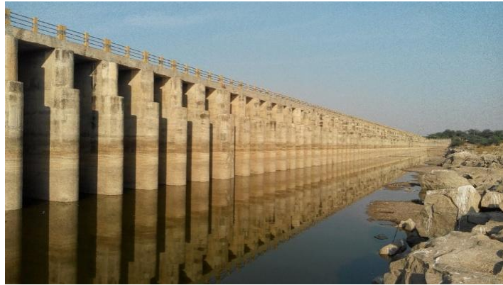
Figure 8 - Joldhadgi Gudur Barrage (10.76 km chainage)
