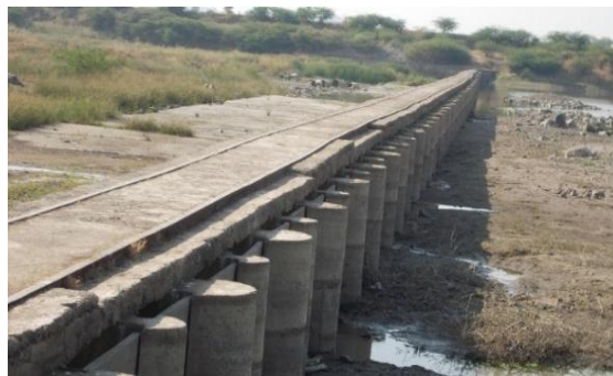
Figure 12 - Koulur Barrage (42.78 km chainage)
