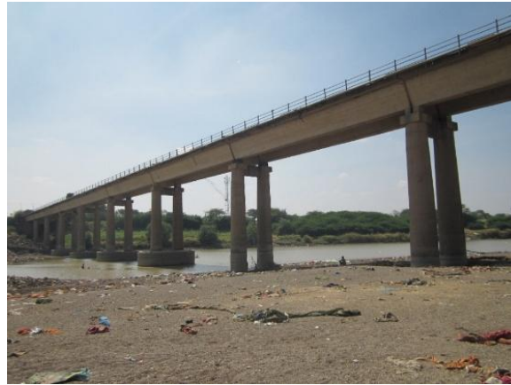
Figure 26 - Raddewadgi Bridge (123.42 km chainage)
