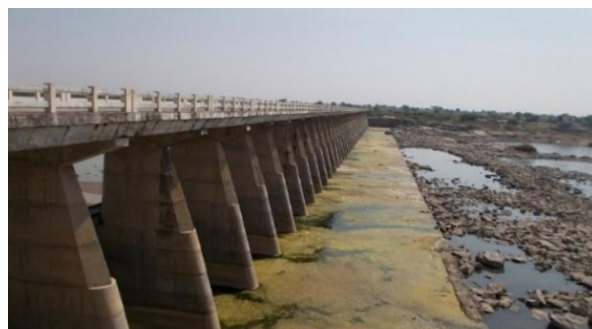
Figure 13 - Anur Barrage (25.23 km chainage)
