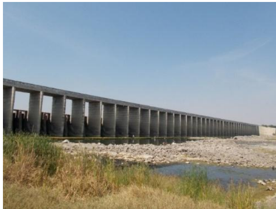
Figure 17 - Yadgir Barrage (51.79 km chainage)
