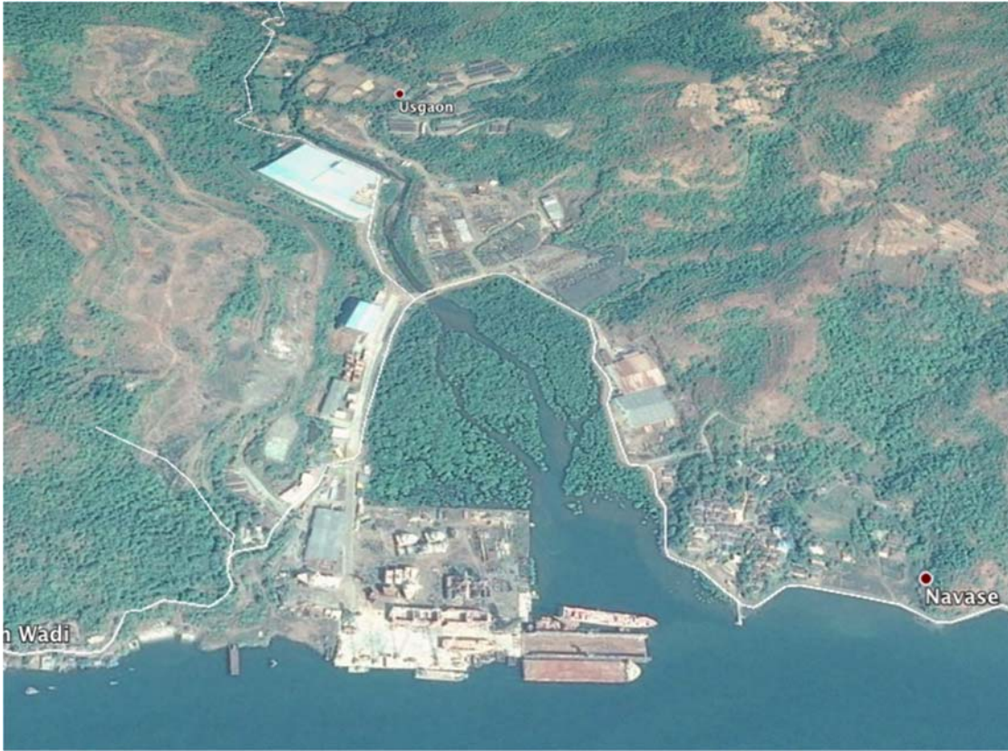
Figure 4-6 Bharati Shipyard at Usgaon
