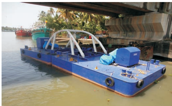
New Anchor Pontoons Deployed on 29.09.2011
