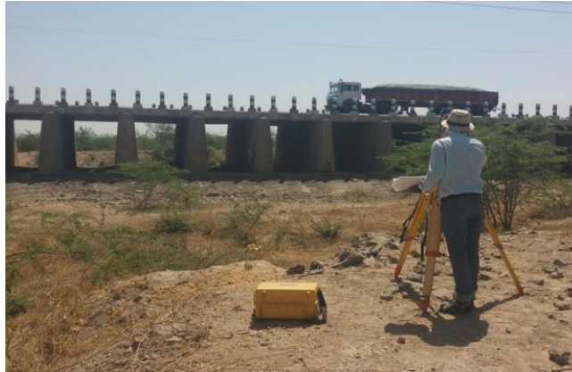
Figure 32 - Stretch 6 Balotra Road Bridge (NH-28) (166.308 km chainage)
