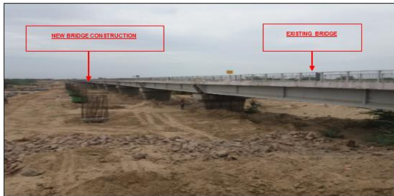
Figure 9 - Gandhav Road Bridge (NH-15) (6.850 km chainage)
