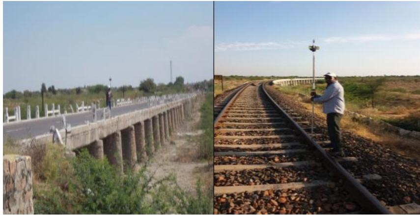
Figure 54 - Stretch 11 Pichiyak Road (334.042 km) and Bhawi Railway Bridge (331.575 km)
