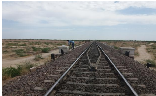
Figure 47 - Stretch 9 Luni Railway Bridge (253.522 km chainage)
