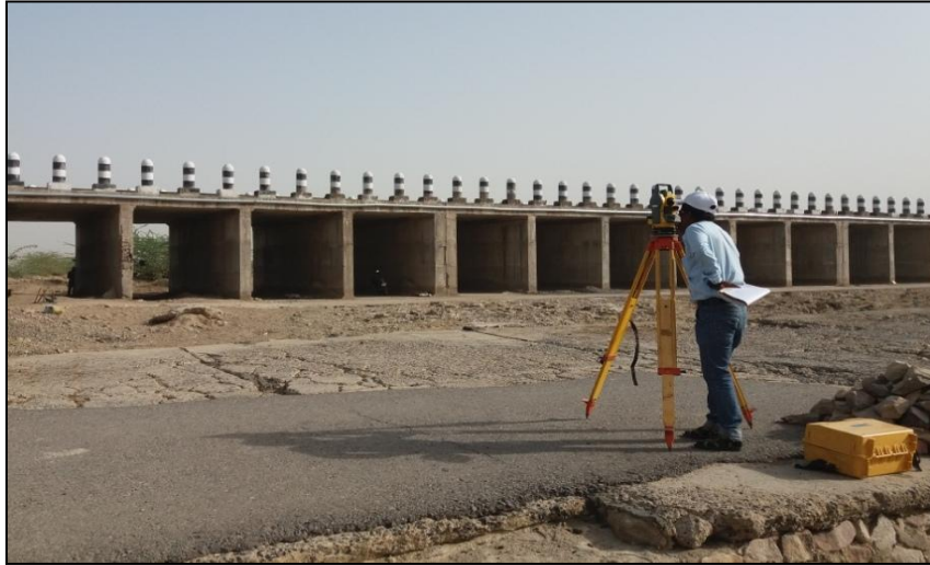
Figure 23 - Stretch 4 Gadesara Road Bridge (SH-28) (84.926 km chainage)
