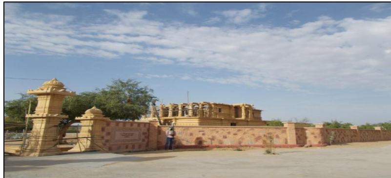
Figure 34 - Stretch 6 Temple at Tilwara (148.163 km chainage)
