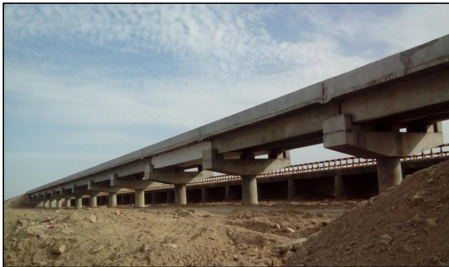
Figure 46 - Stretch 9 Kankani Road Bridge (Upper NH-65) (262.824 km chainage)
