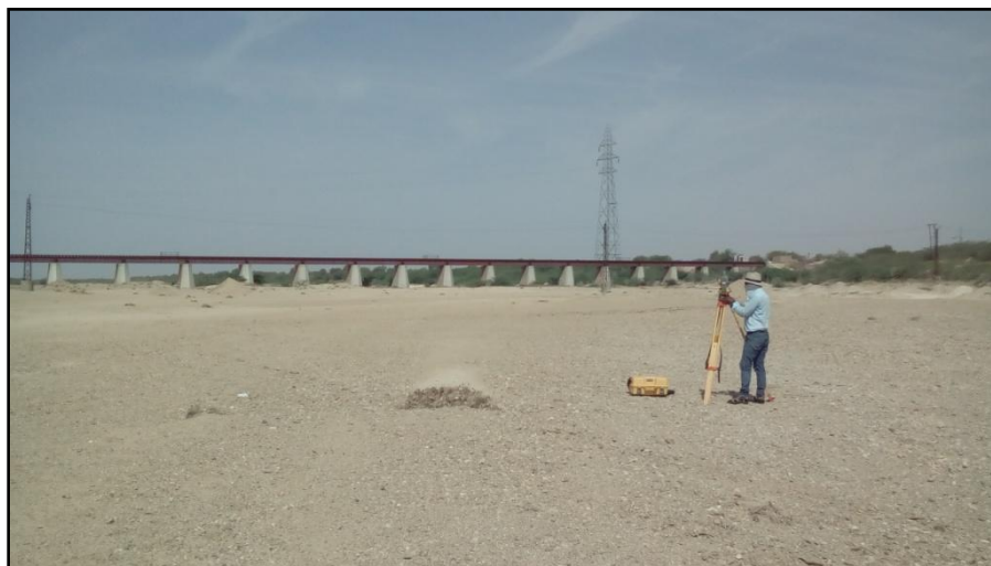
Figure 38 - Stretch 7 Samdari Railway Bridge (197.689 km chainage)
