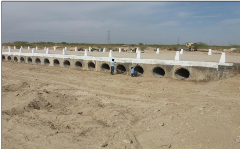
Figure 50 - Guda Bishnoiyan Sanko Road Bridge (273.058 km chainage)
