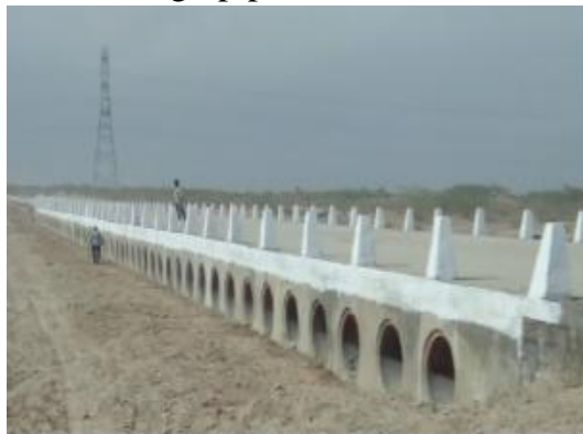
Guda Bishnoiyan Sanko Road Bridge
