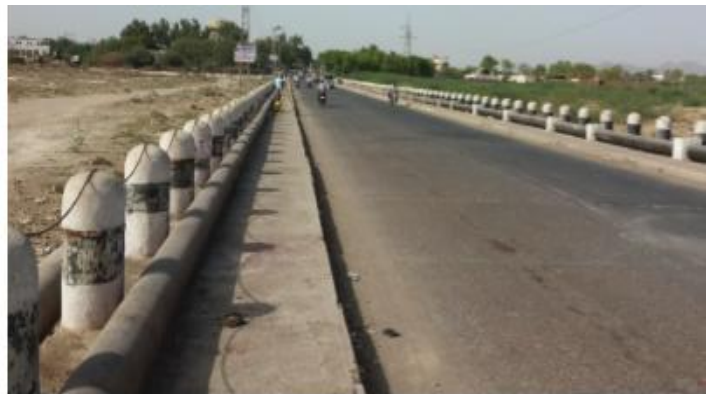
Balotra Sanko Road Bridge
