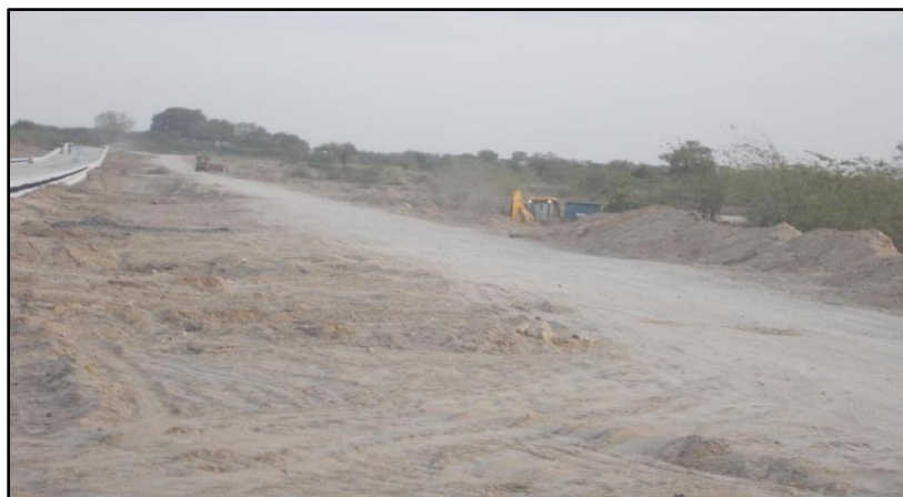
Figure 39 - Stretch 7 JCB operating in Sand Quarry near Jetharni village (192.0 km chainage)
