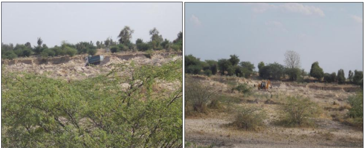
Figure 51 - Excavation Activity near Goliya (294.8 km) and Guda Bishnoiyan village (274.0 km)
