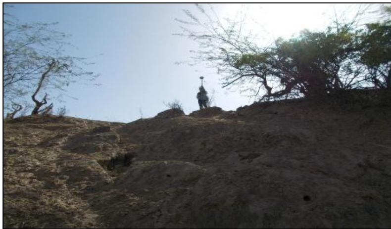
Figure 29 - Stretch 5 Loose mud cliffs on the river bank
