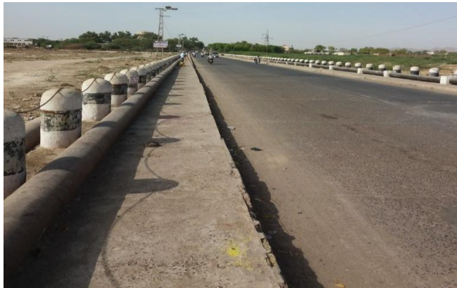
Figure 33 - Stretch 6 Balotra Sanko Road Bridge (NH-112) (163.550 km chainage)
