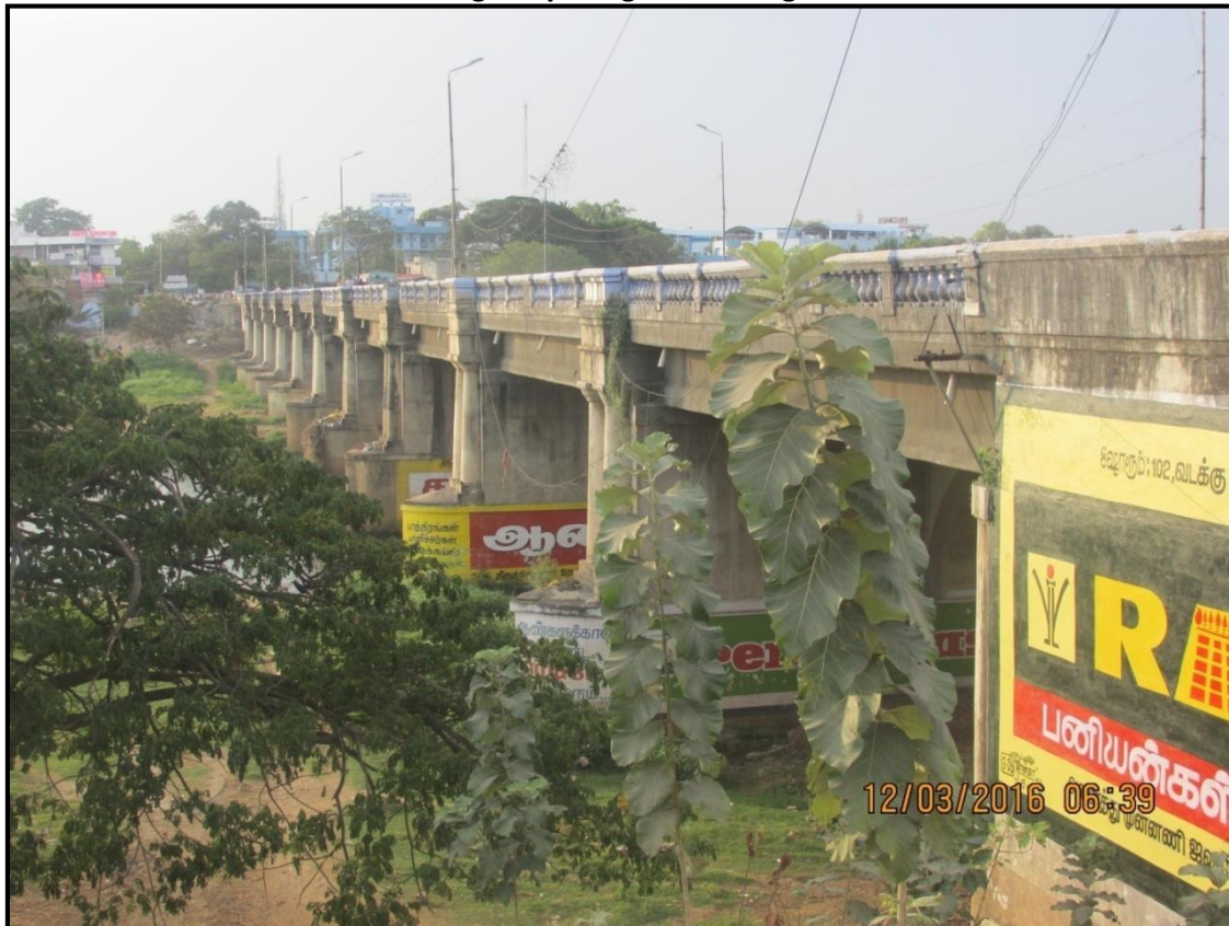
22: Kokarkullam Bridge/ Sulochna Mudliar Bridge at chainage 64 km
