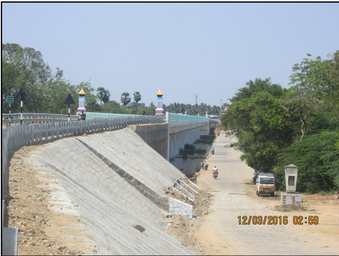
8: New Constructed Eral Bridge at Chainage 13 km
