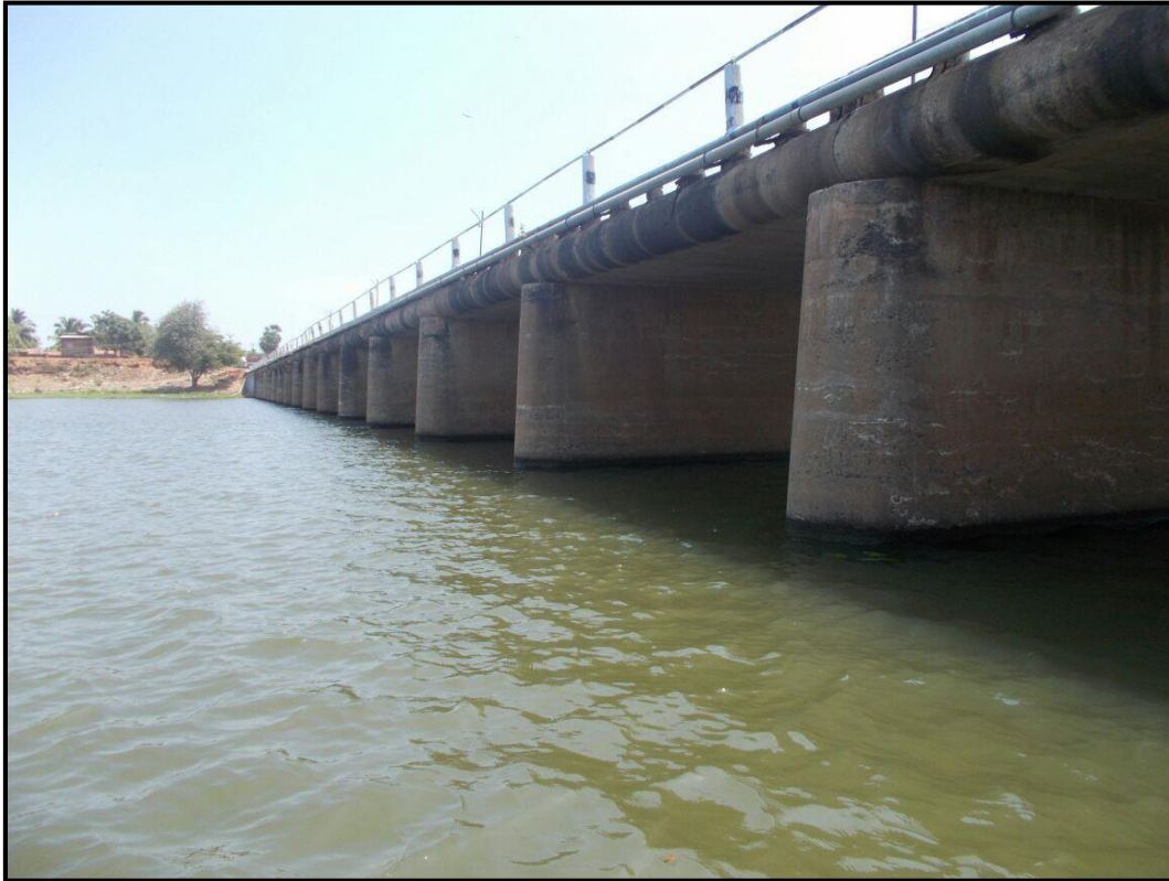
5: Authoor old Road Bridge (Chainage 7 km)
