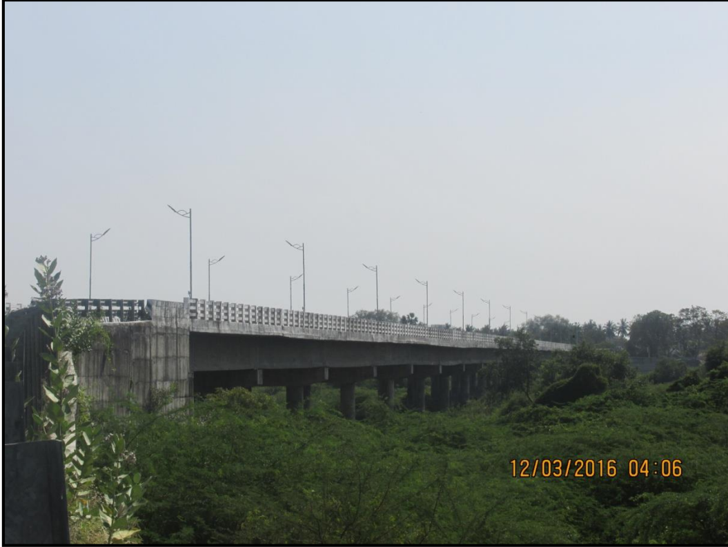
11: Srivaiguntam New Road Bridge at chainage 25.6 km
