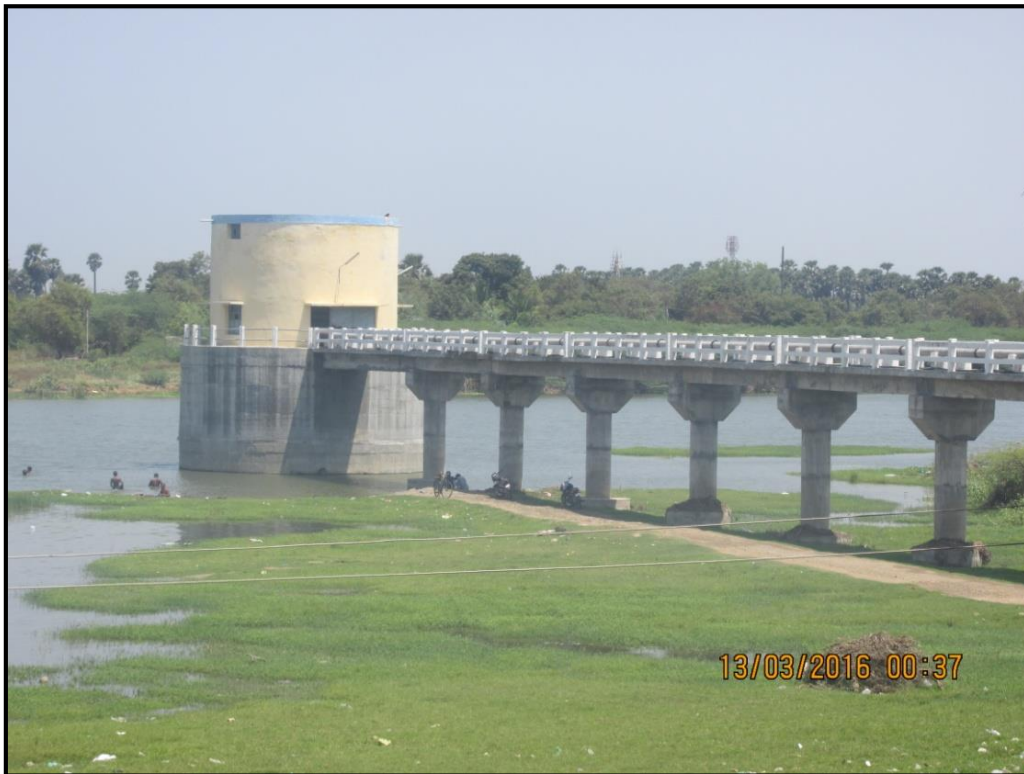
6: Water Intake at chainage 7.1 km
