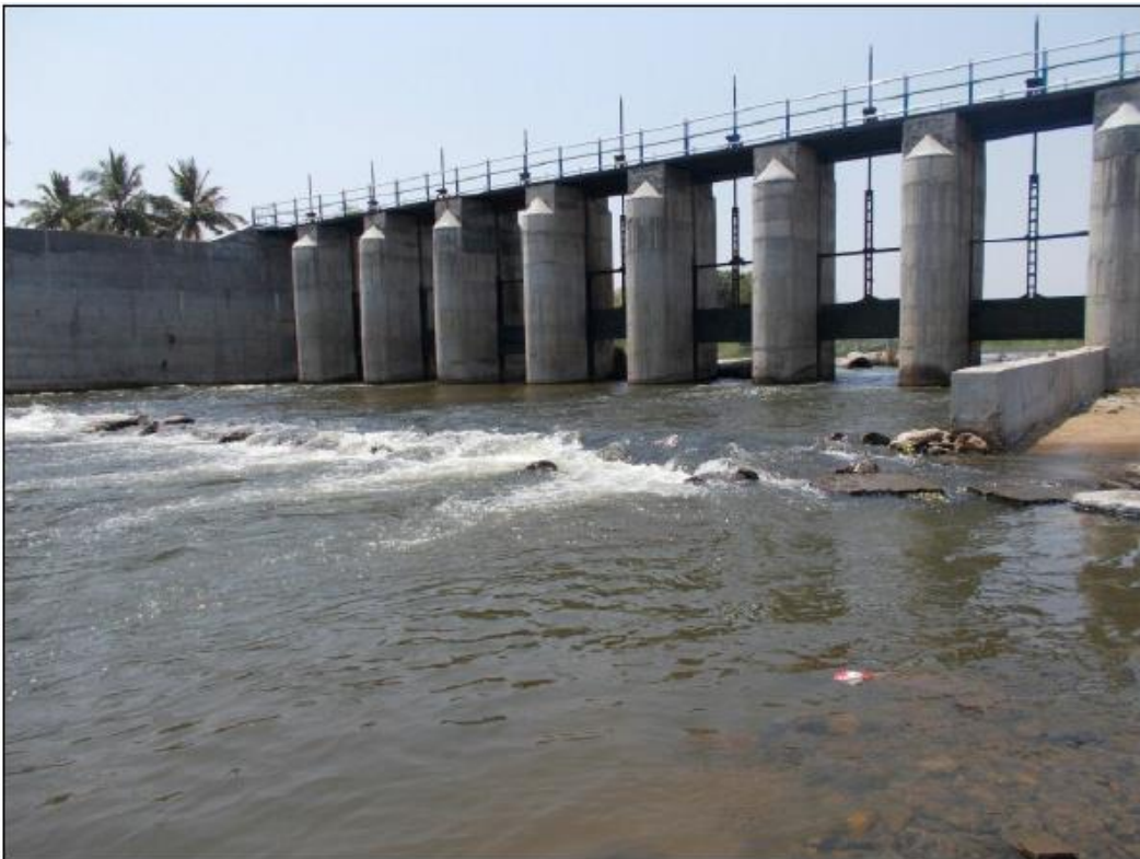
16: Pakapattai weir at chainage 40.6 km
