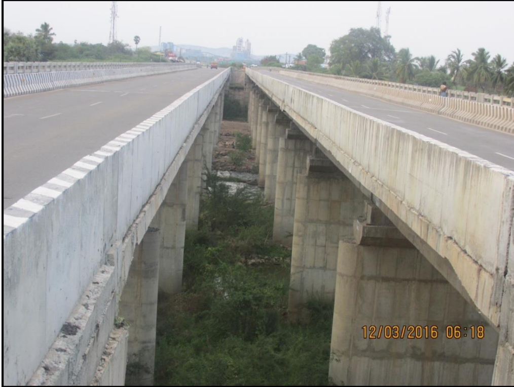
21: NH-7 Highway Bridge at chainage 59.7 km
