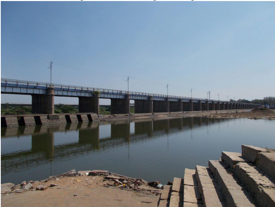
12: Srivaiguntam old Road Bridge at chainage 25.7 km
