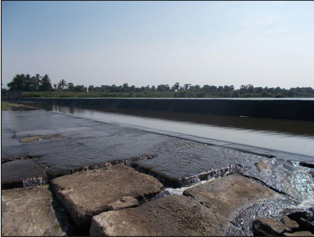
7: Latchumipuram Check Dam at Chainage 9.4 km
