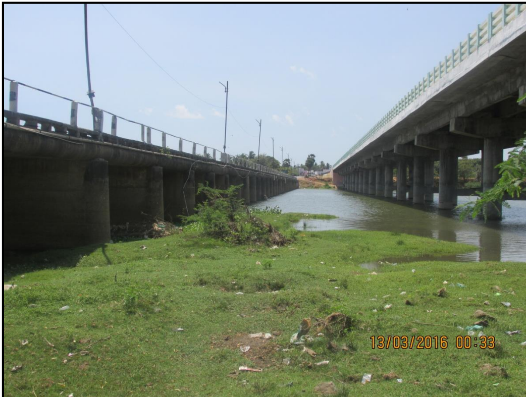
4: Authoor New Road Bridge (Chainage 6.9 km)
