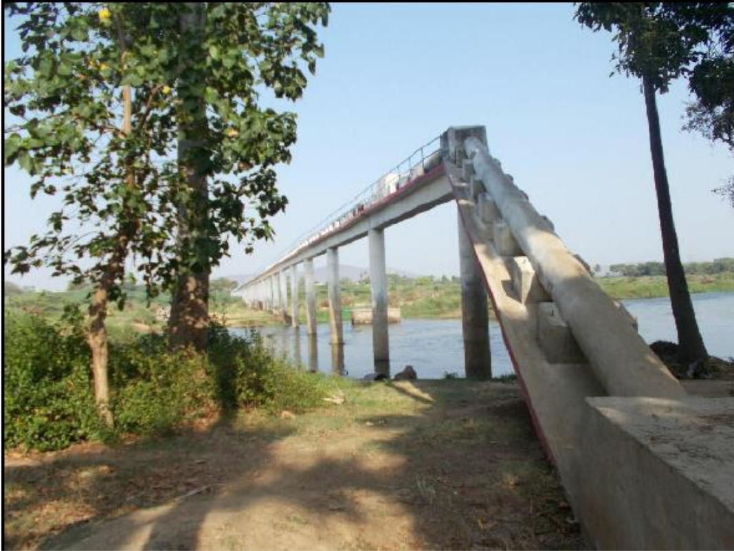
19: Water pipeline bridge at chainage 42.4 km
