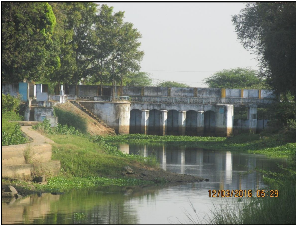
20: KALIYUVAR Regulator at Chainage 48.3 km
