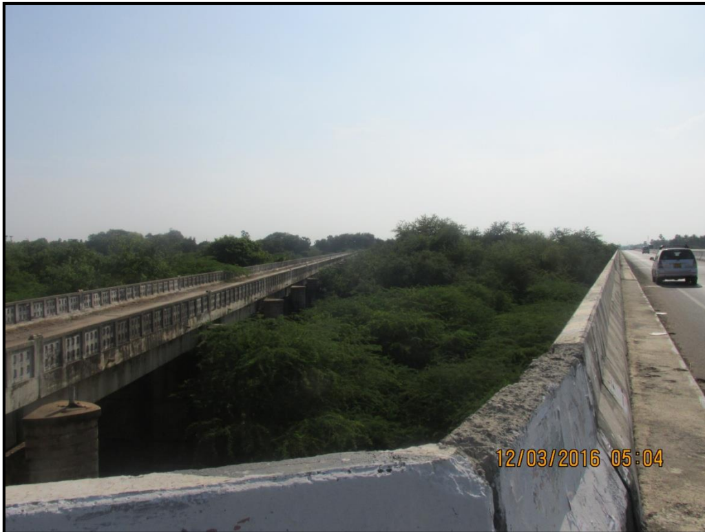
18: Murappanadu New Road Bridge & Footbridge at 41.3 km
