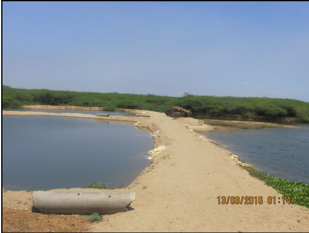
3: Earthen Bund (Sand Barrier) made by local across the river at Chainage 3.8 km to store fresh water
