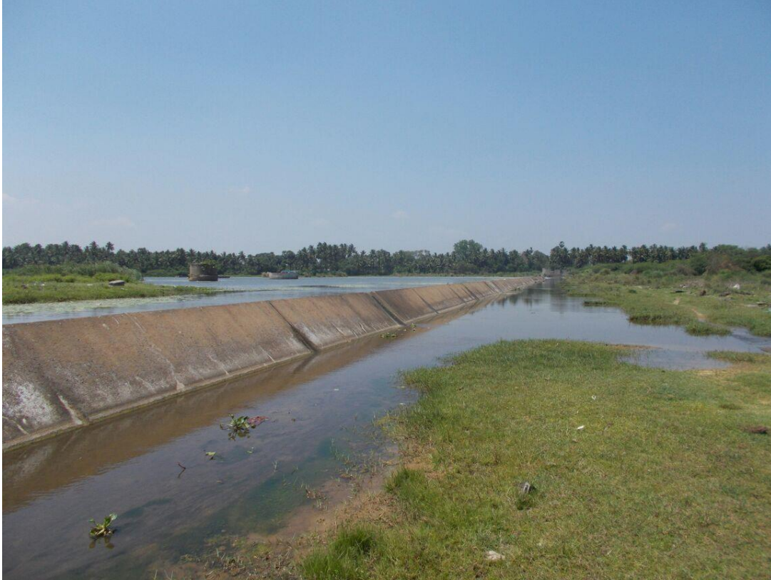
9 : View of Kurangani Dam at chainage 16 km
