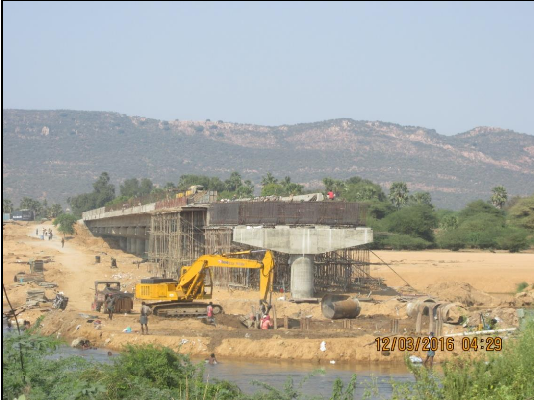
15: Road Bridge under Construction at Chainage 33.2 km
