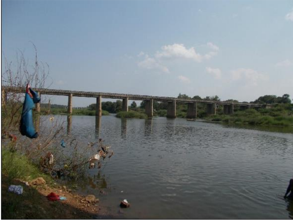
17: Old Murappanadu Bridge at chainage 41.1 km
