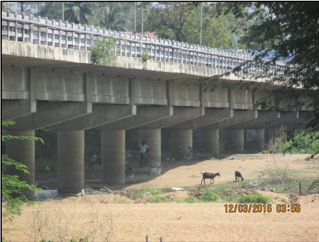
10: Alwarthopu Road Bridge at chainage 21.4 km
