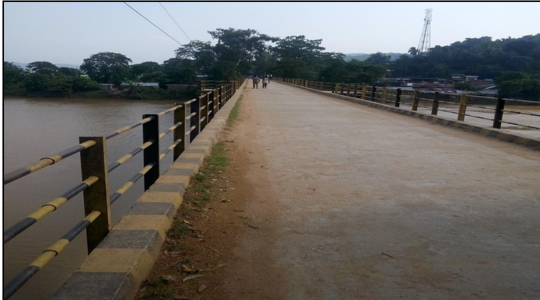
Figure 11 –Kalang RCC Bridge (Chainage- 14.944 km)
