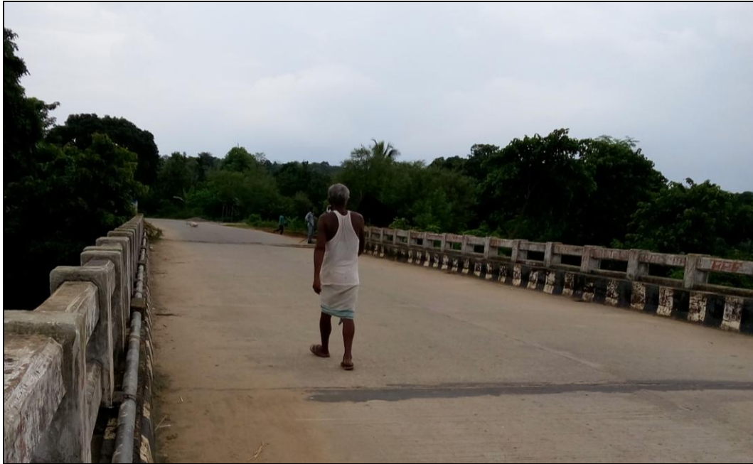
Figure 16 RCC Bridge (Chainage- 49.893 km)
