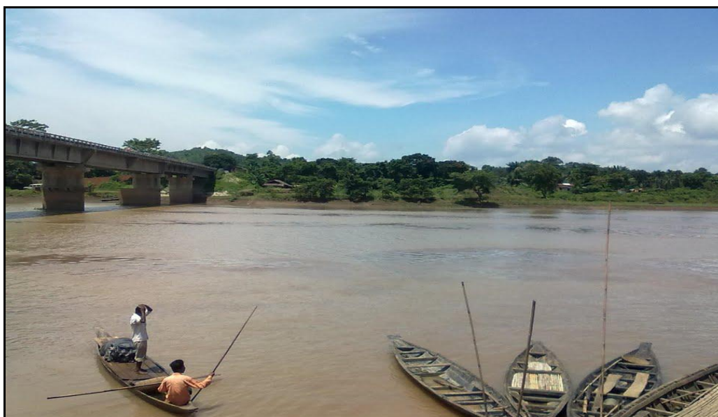
Figure 8 Digaru Ghat (Chainage-4.600 km)
