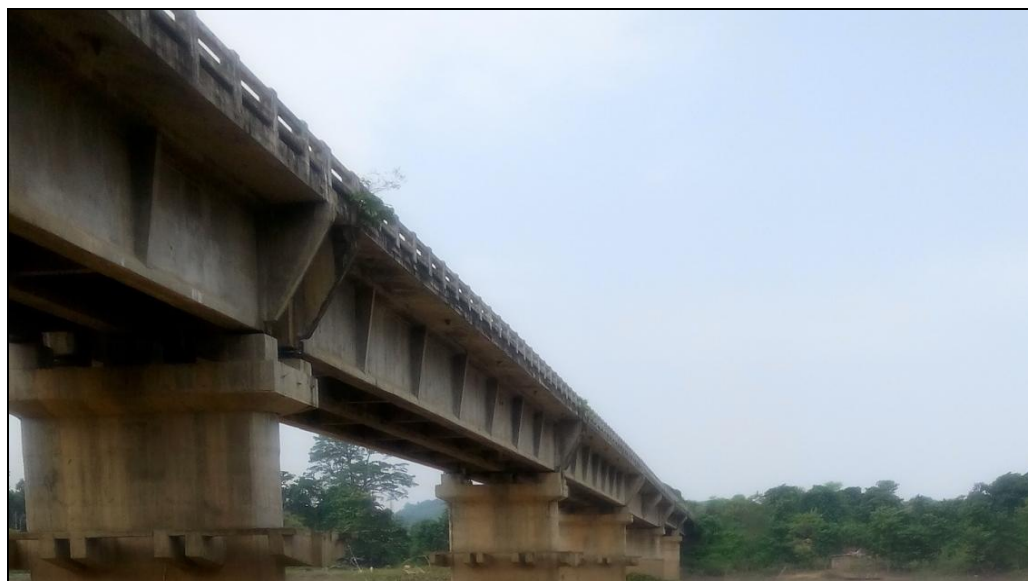
Figure 9 Gobordhon RCC bridge (Chainage-5.658 km)
