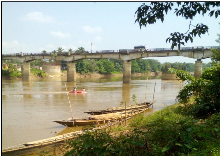
Figure 33 Site Picture of the Gobordhon RCC Bridge
