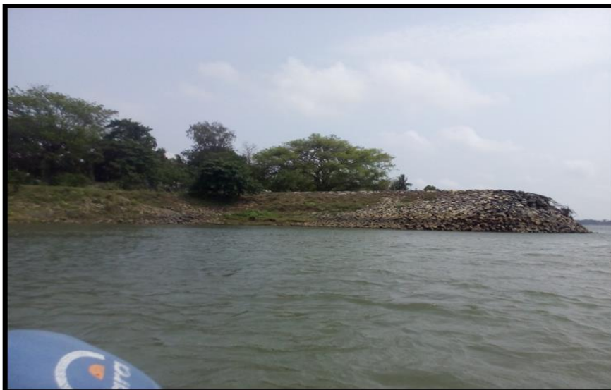
Bund at Chainage 29.0
