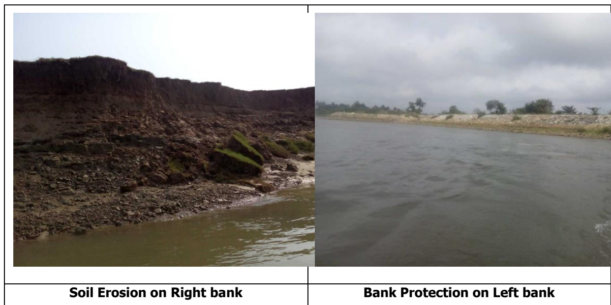
Figure 7: Photographs of Sub-stretch 2
