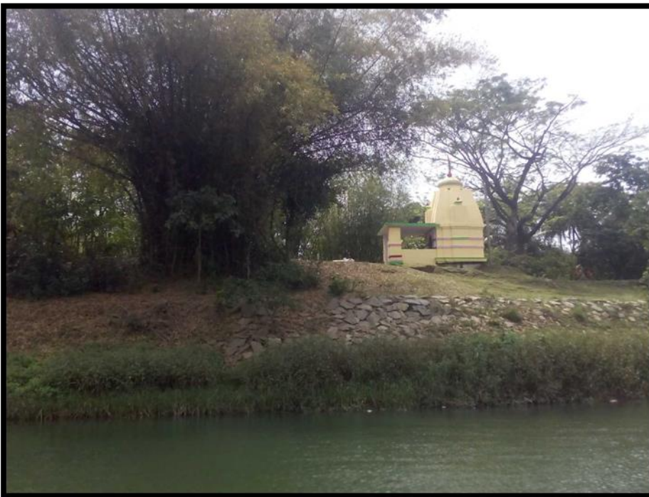
Temple at Chainage 29.5
