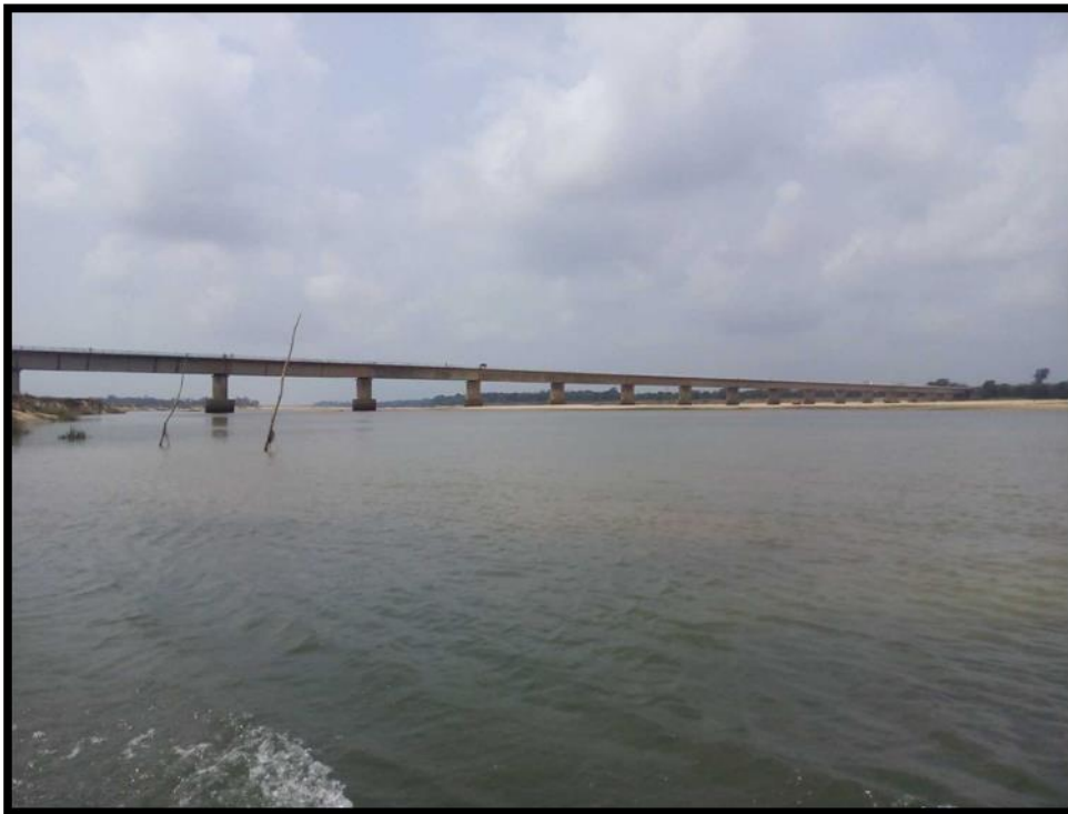
Bridge at Balipal Chainage 29.0
