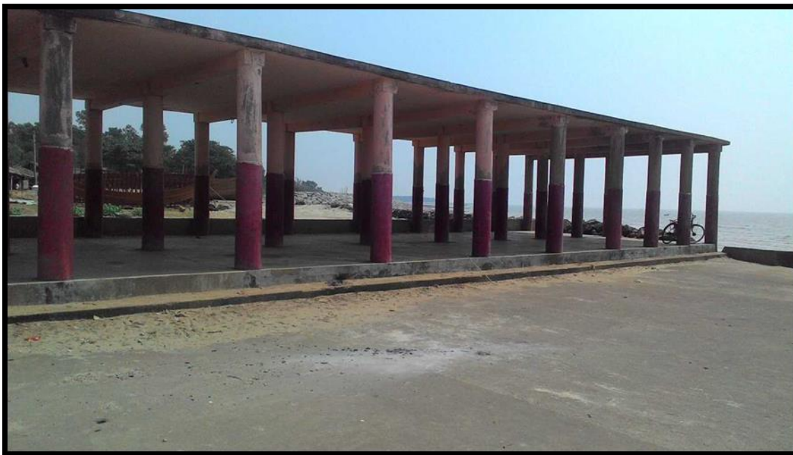
Chandrabali Jetty Area at Chainage 1.5
