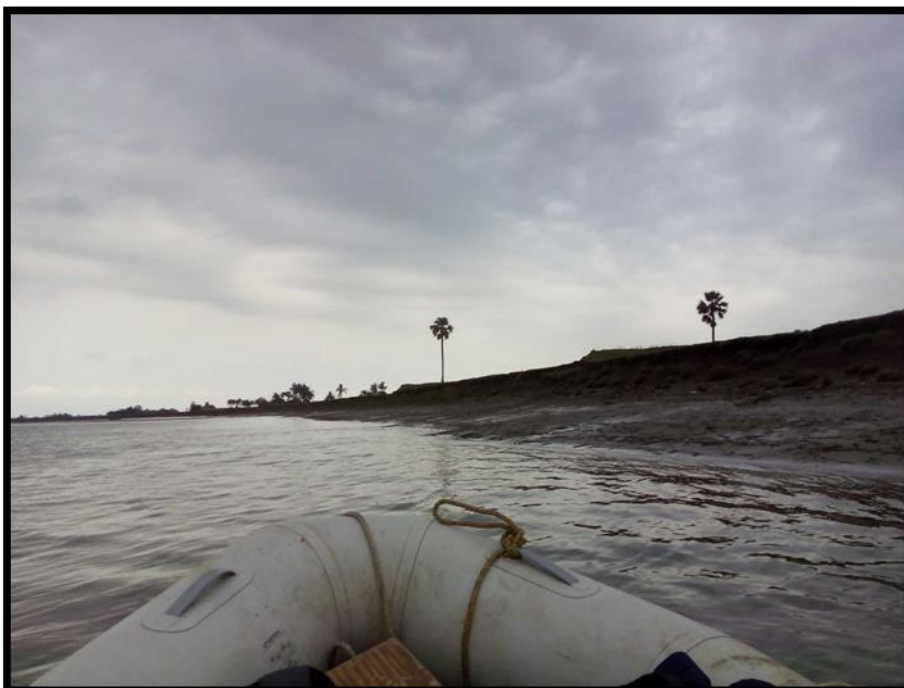
Soil Erosion at chainge 8.0
