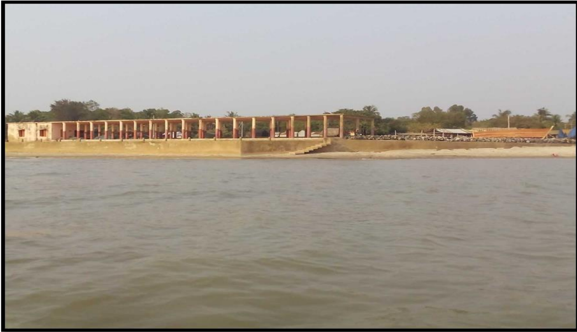
Chandrabali Jetty Area at Chainage 1.5
