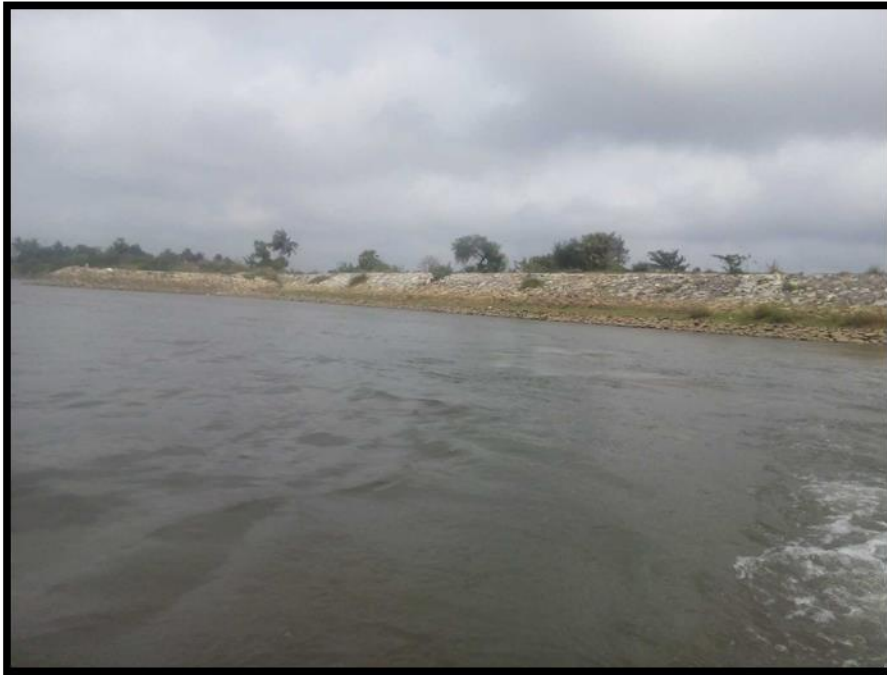
Bank Protection at Chainage 24.0
