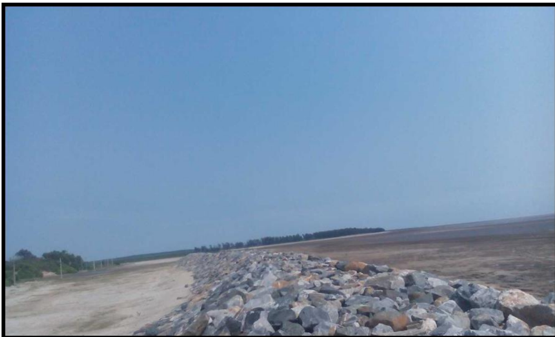
Bank Protection at Chainage 1.4
