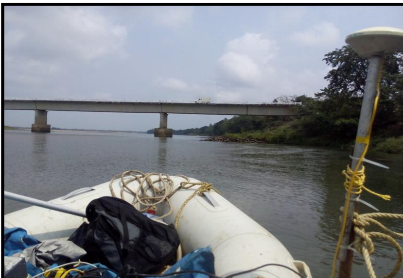
Bridge at Balipal Chainage 29.0
