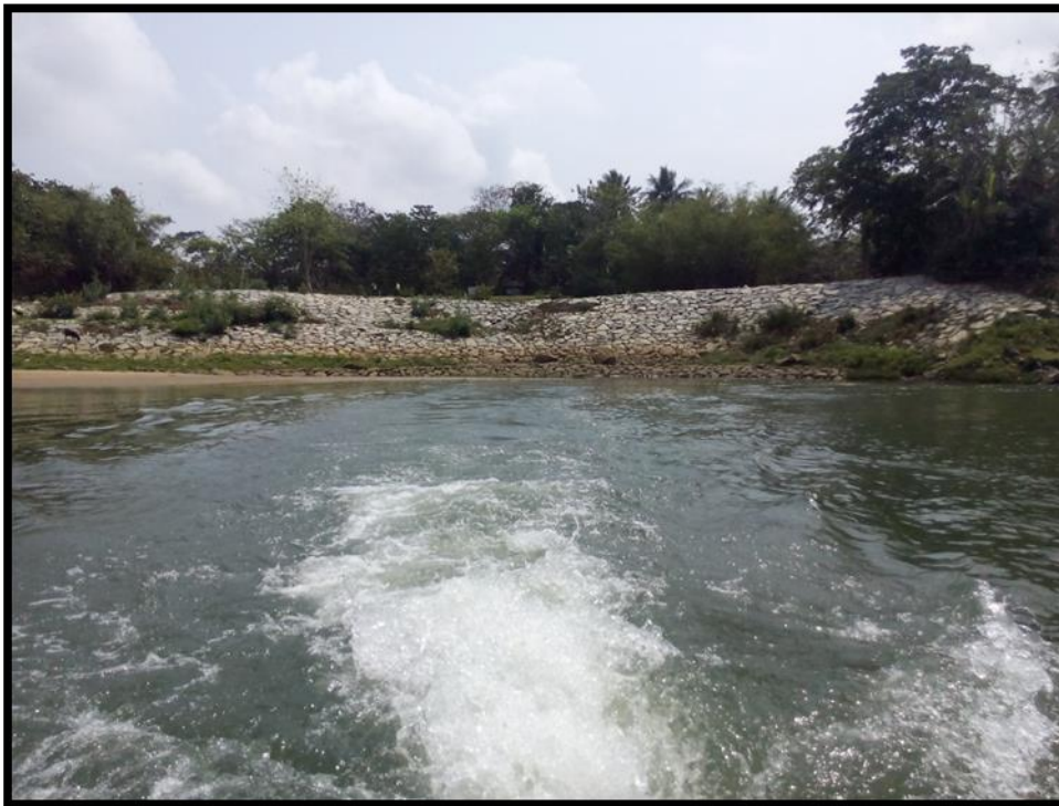
Bank Protection at Chainage 28.3
