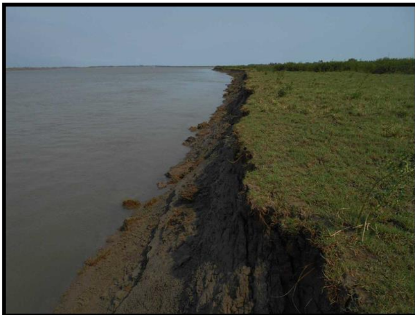
Soil Erosion at chainge 5.5
