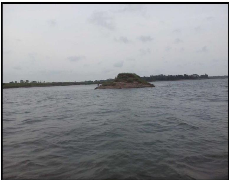
Island at Chainage 20.5
