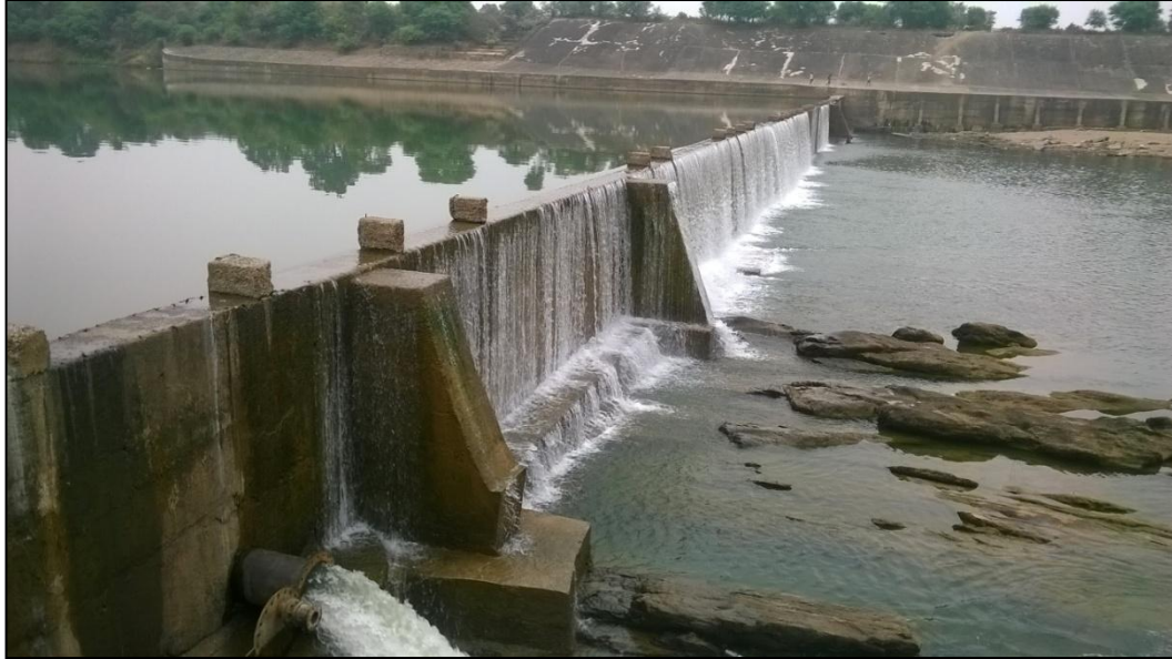
Figure 11- Check Dam at Kalpatanga village (Chainage-10.642 km)
