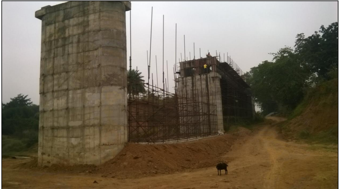
Figure 13-Under-Construction RCC Bridge (Chainage-16.724 km)
