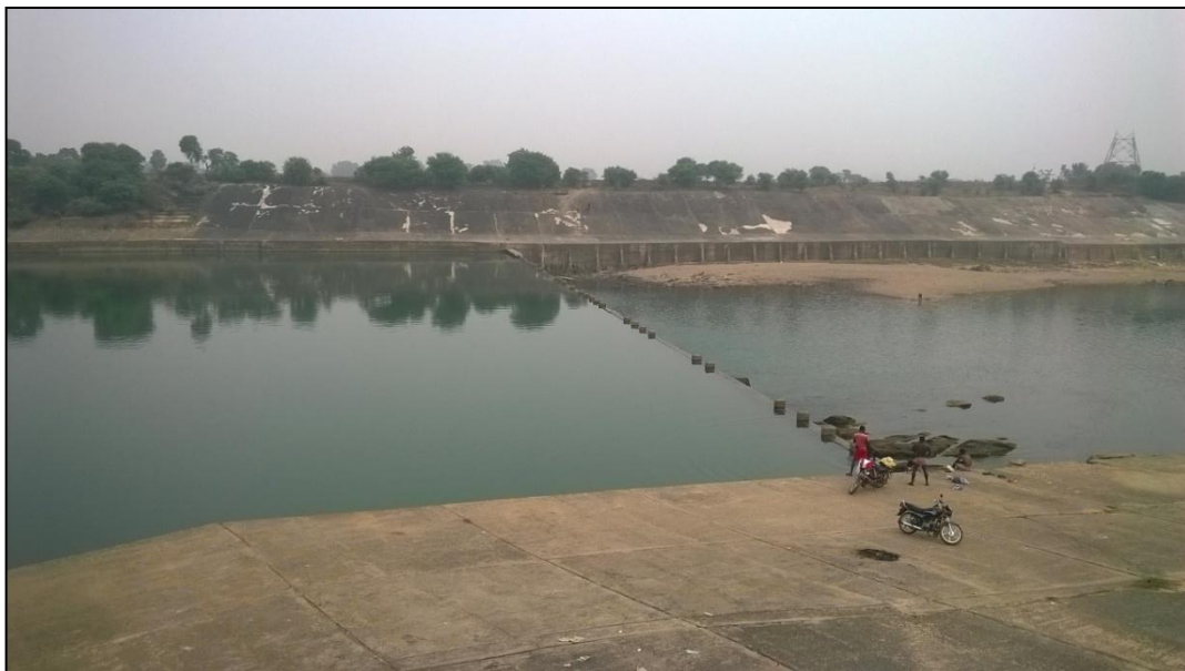
Figure 12-Check Dam at Dudra village (Chainage-15.623 km)
