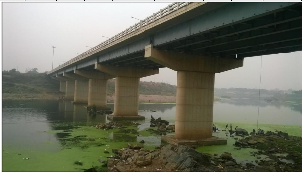
Figure 6- Adityapur Toll Bridge (4.615 km)
