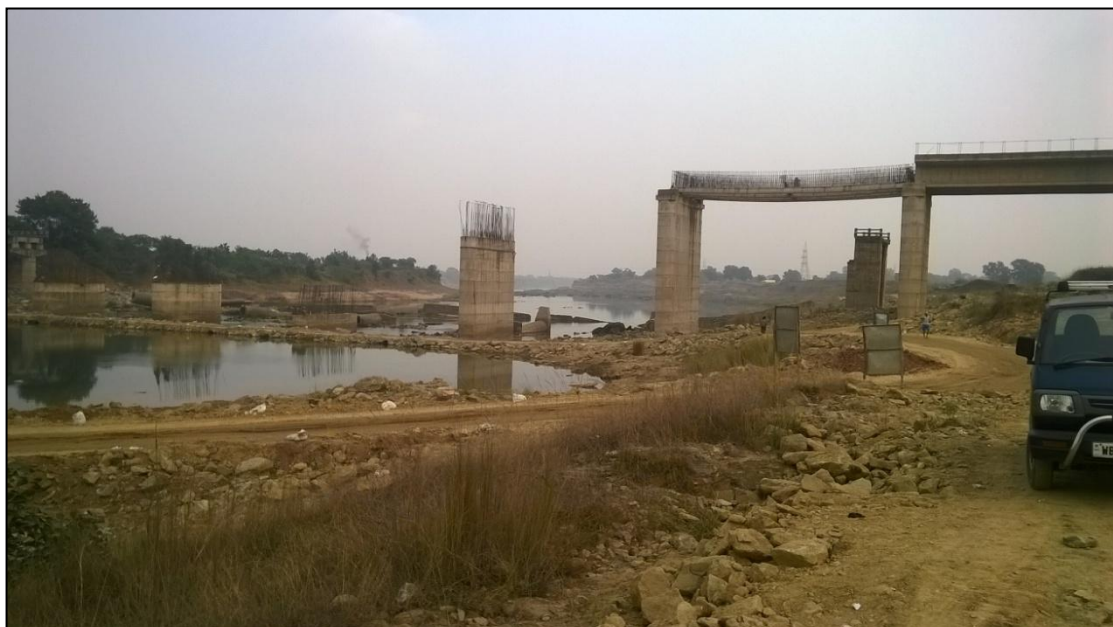
Figure 14-Under-Construction RCC Bridge (Chainage-22.104 km)
