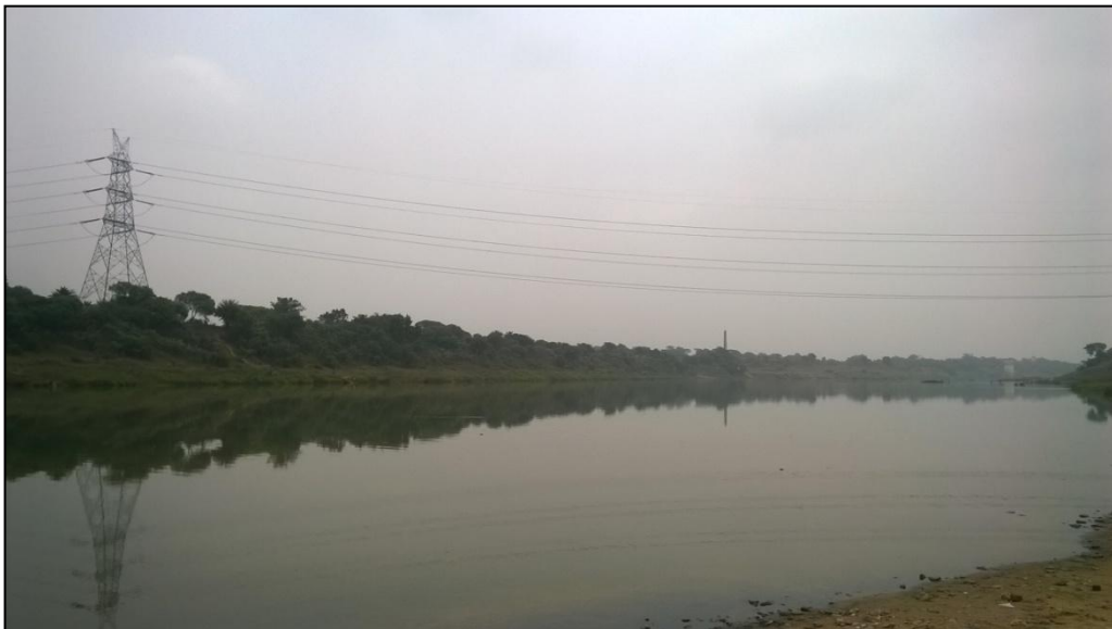
Figure 9- High Tension Line (Chainage-3.498 km)
