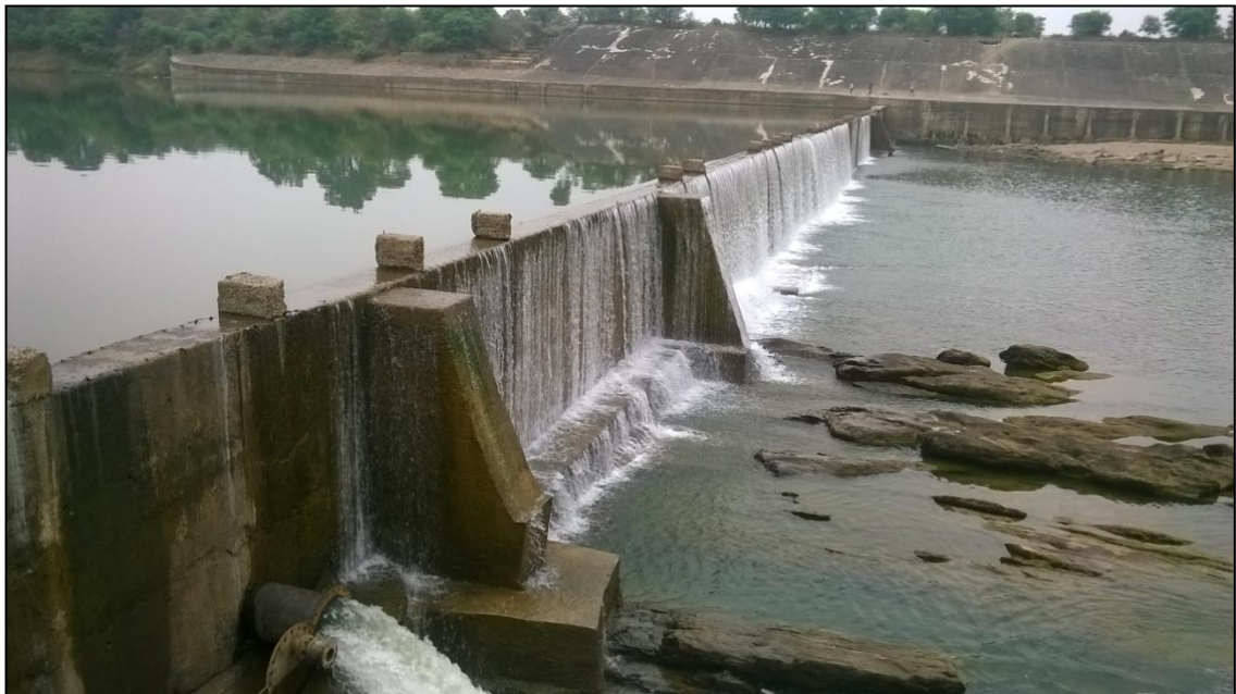
Figure 29-Check Dam near at Chainage 10.642 km
