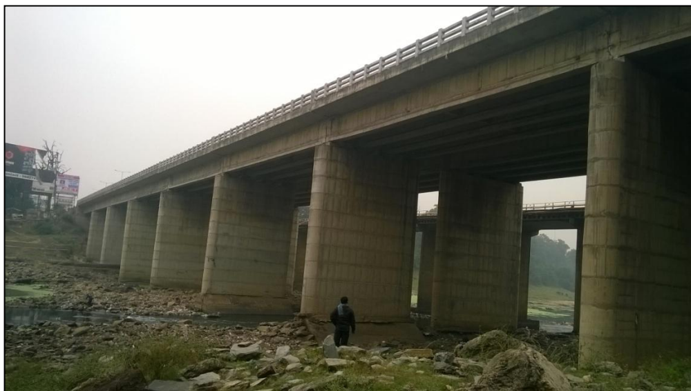
Figure 7- Adiyapur RCC Colony Bridge (Chainage-8.610 km and 8.636 km)
