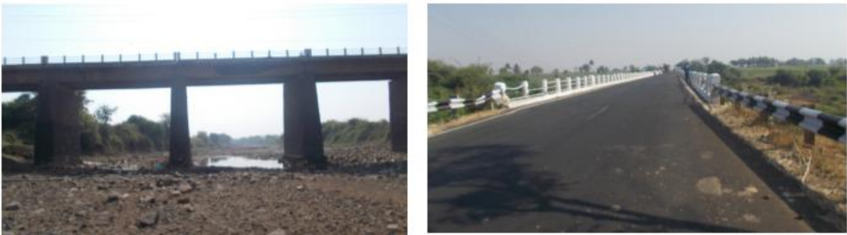
Figure 18 - Chinchakhandi Bridge (91.06 km chainage)
