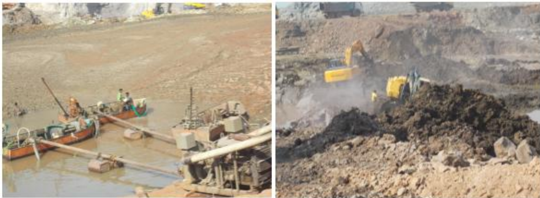
Figure 10 - Under construction Barrage at Herkal Village (16.85 km chainage)
