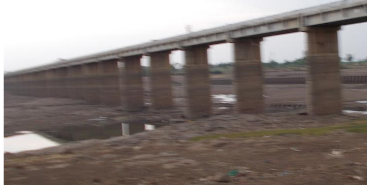
Figure 13 - Yadahalli Bridge (38.7 km chianage)
