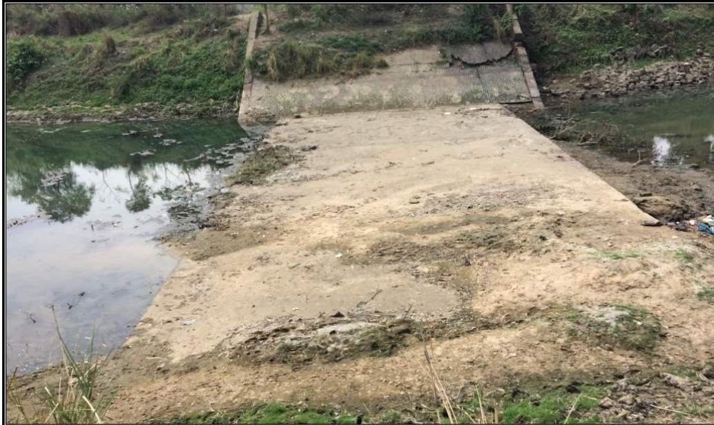
CHAINAGE 62.89 Km UNDERPASS CANAL ISUFABAD
