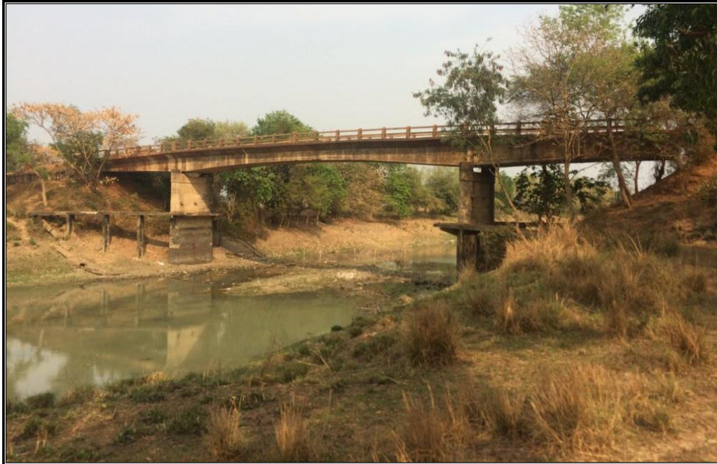
CHAINAGE 51.369 Km BRIDGE URA-DALIMGARYA
