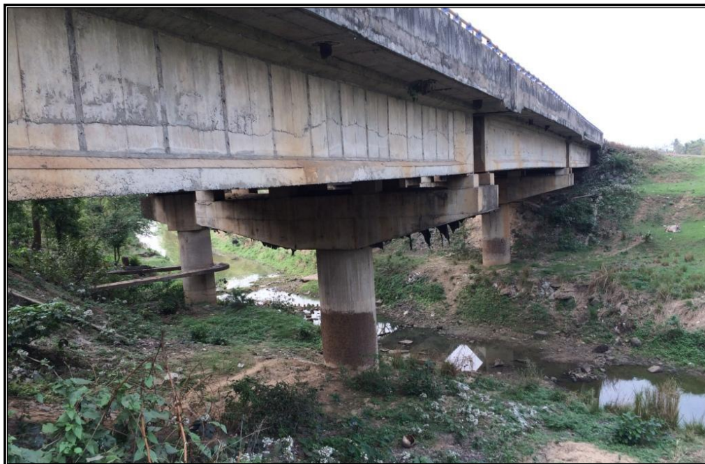
CHAINAGE 89.735 Km BRIDGE NH KANAI DANGA
