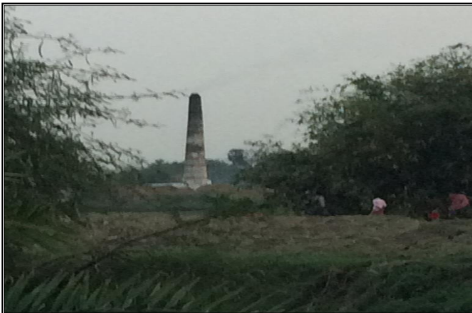
CHAINAGE 80.984 Km BRICK KILN TOTPARA
