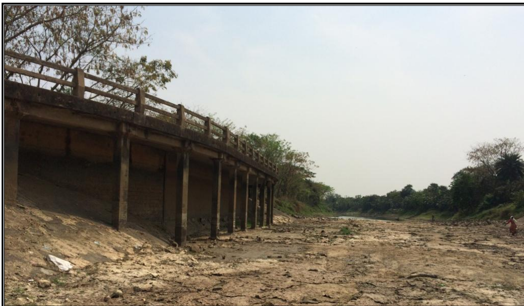
CHAINAGE 64.87 Km UNDERPASS CANAL UDAYPALLI
