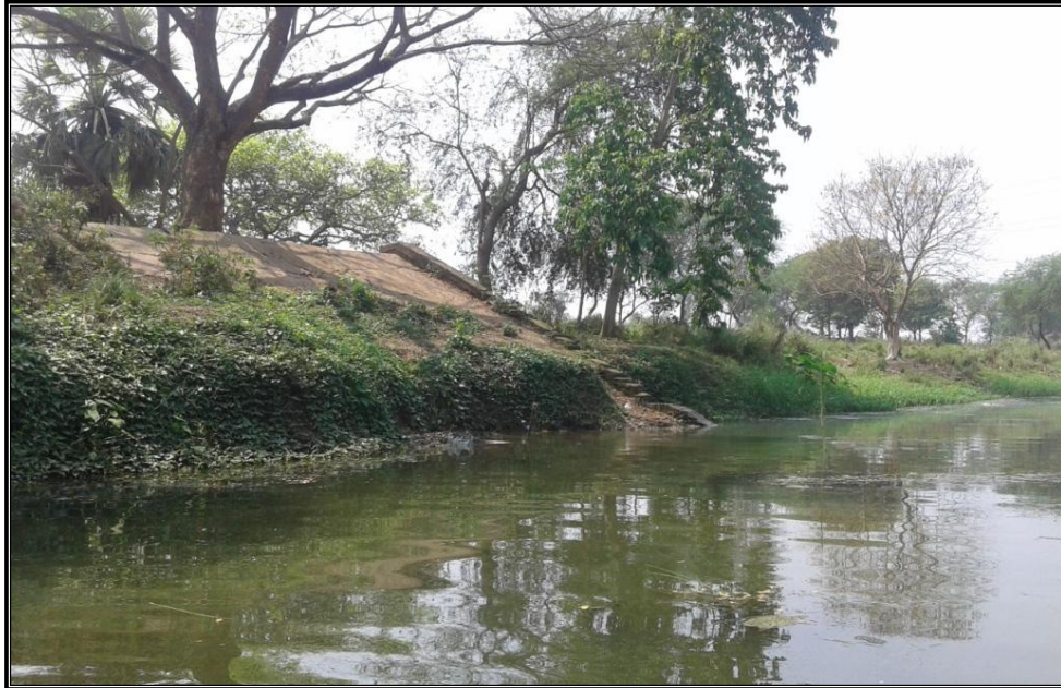
CHAINAGE 131.9 Km CULVERT KHALSI
