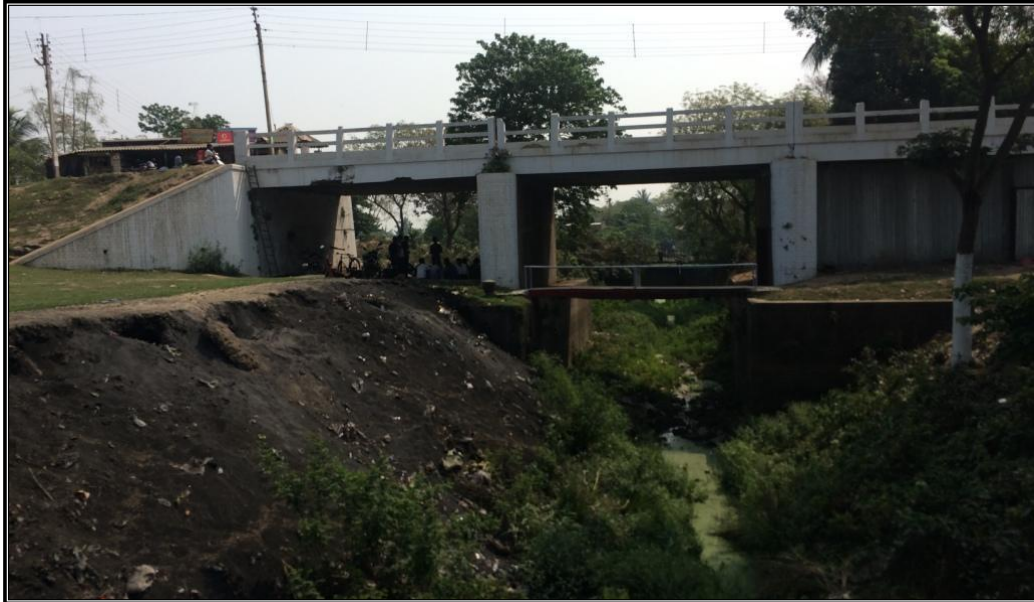
CHAINAGE 69.697 Km LOCK GATE SADHARGHAT BURDWAN
