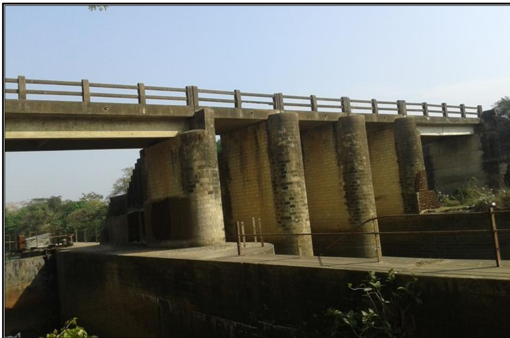
CHAINAGE 108.264 Km BRIDGE BOINCHI(BATIKA)
