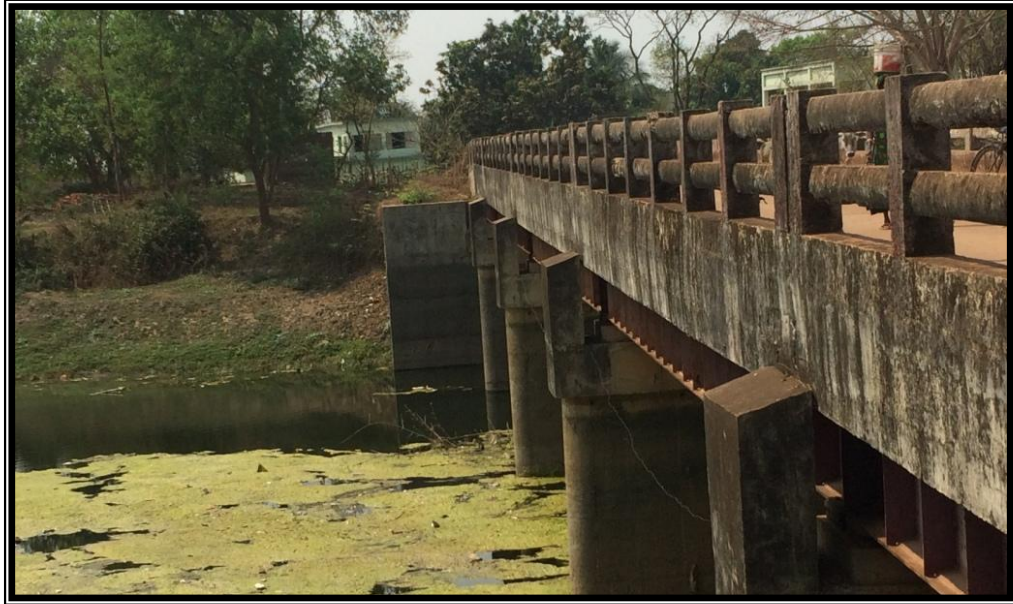
CHAINAGE 22.214 Km BRIDGE SHALDANGA
