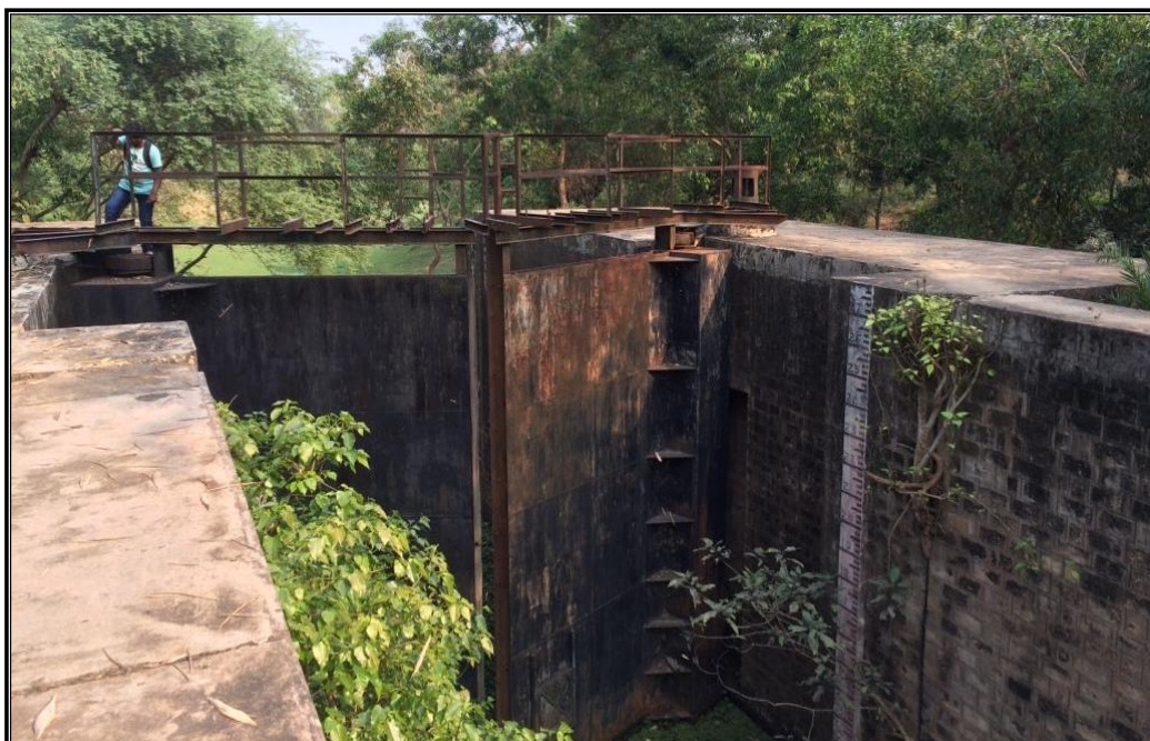
CHAINAGE 88.025 Km LOCK GATE MAHESPUR
