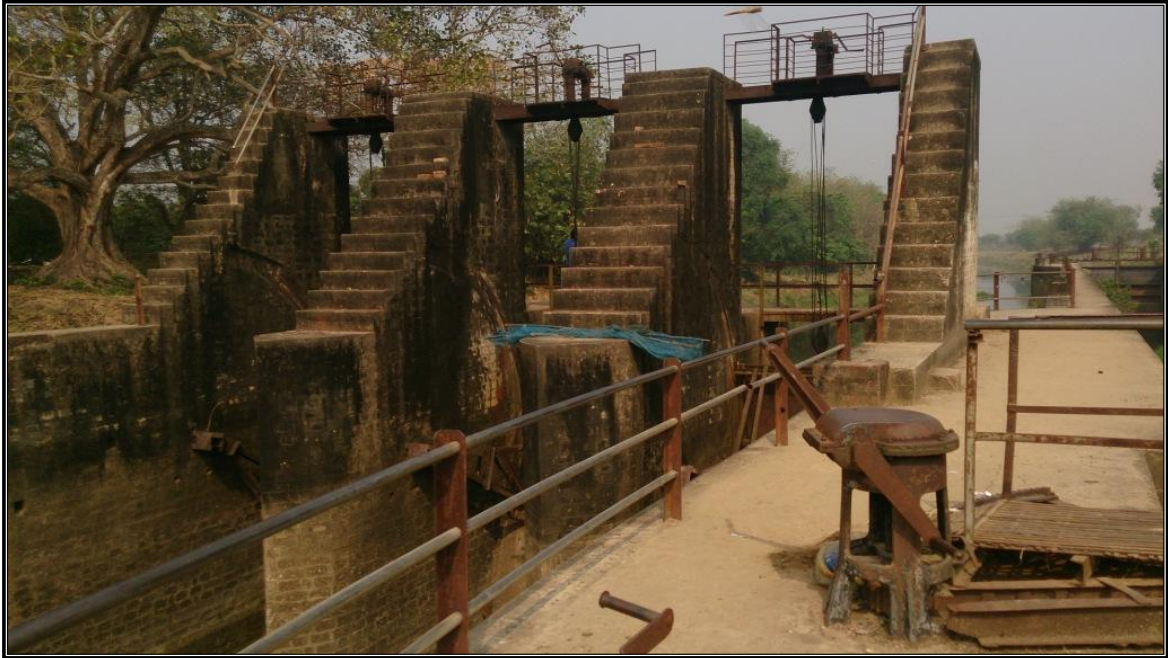
CHAINAGE 126.21 Km LOCK GATE HOERA
