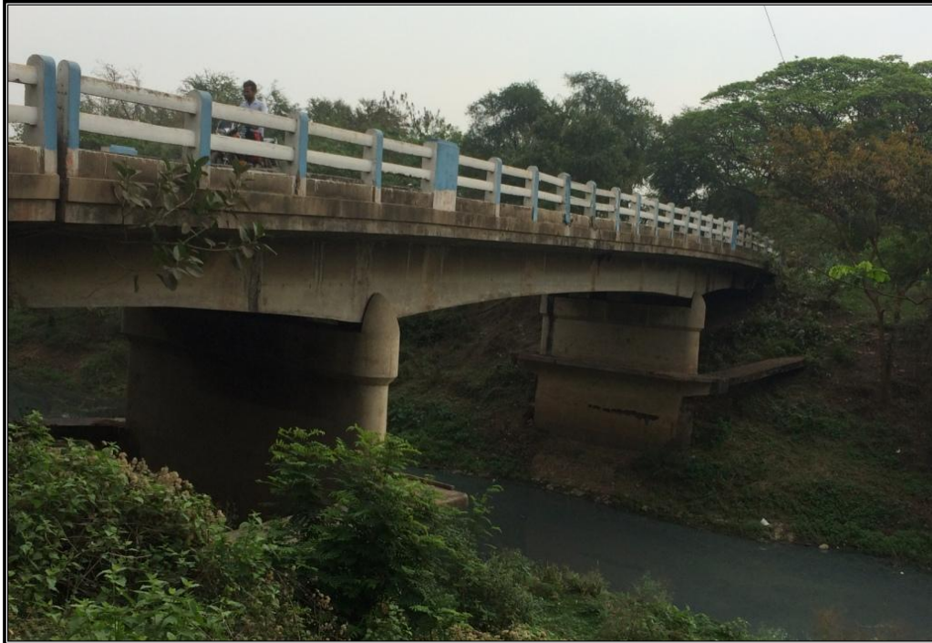
CHAINAGE 98.347 Km BRIDGE BAGILA (GODHIPUR)
