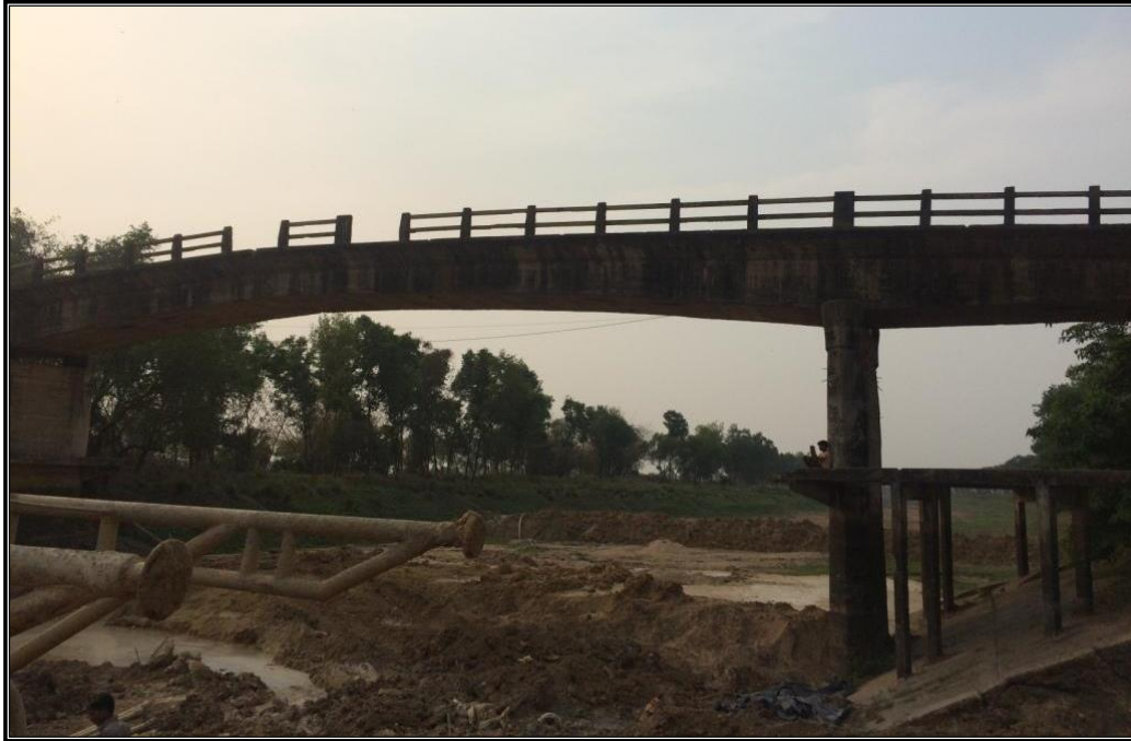
CHAINAGE 45.808 Km BRIDGE KHETURA_1
