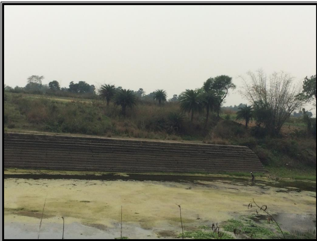
CHAINAGE 10.576 Km CONCRETE LADDER RAJBANDH
