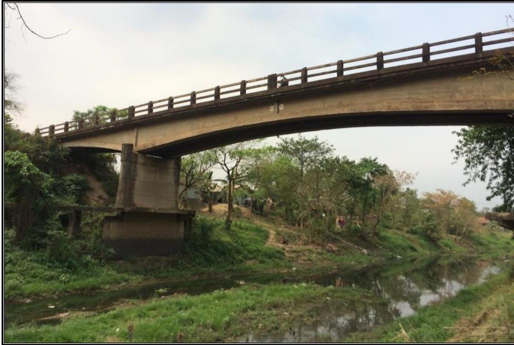
CHAINAGE 99.898 Km BRIDGE BAGILA
