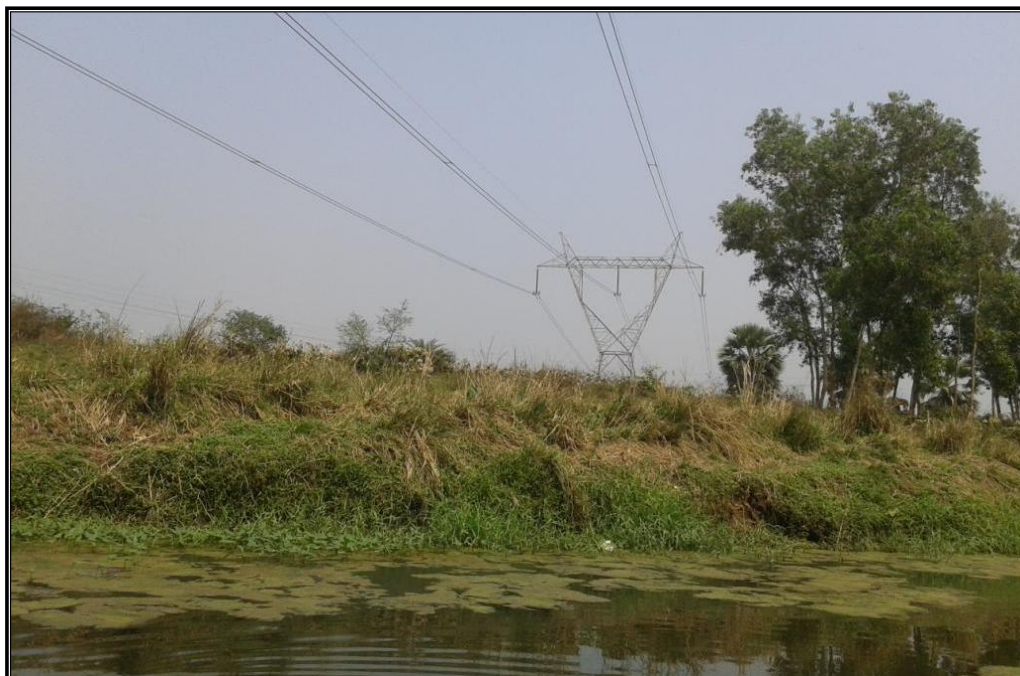
CHAINAGE 131.58 Km HIGH TENSION ELECTRIC LINE KHALSI
