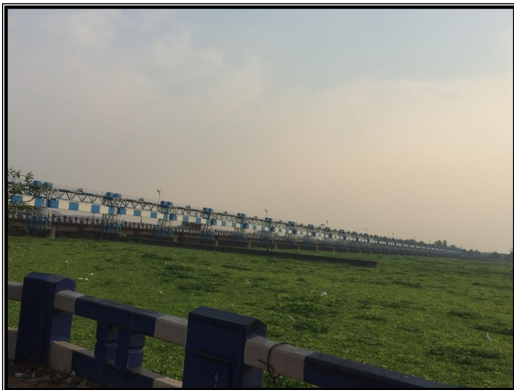
CHAINAGE 0.175 Km LOCK GATE SUKUMARNAGAR
