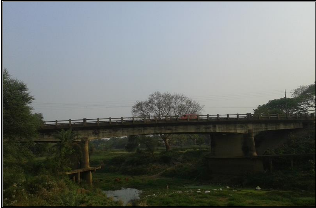
CHAINAGE 119.295 Km BRIDGE PANDUA CHANDANI MARKET
