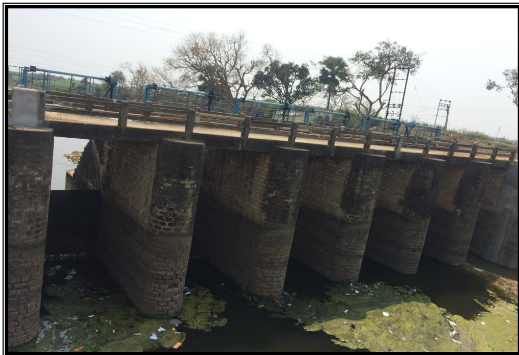
CHAINAGE 16.59 Km LOCK GATE CUM BRIDGE PRAYAGPUR
