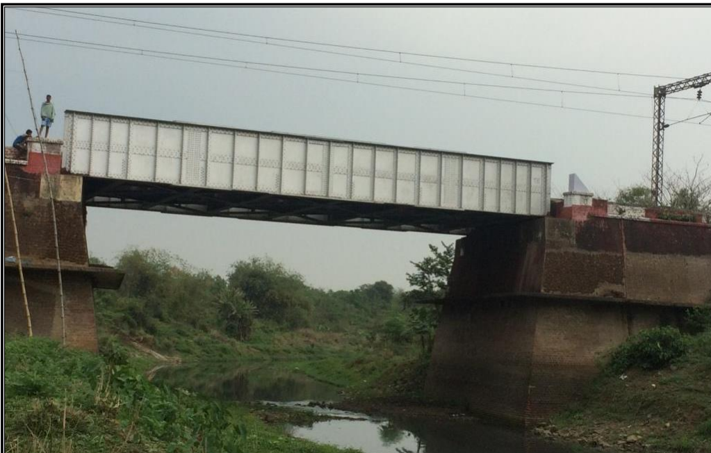
CHAINAGE 98.854 Km RAILWAY BRIDGE BAGILA(NUDIPUR)
