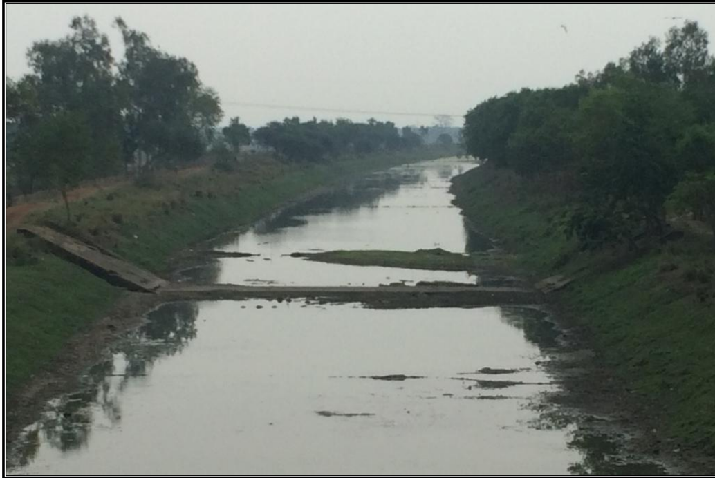
CHAINAGE 41.458 Km UNDERPASS CANAL SUJAPUR
