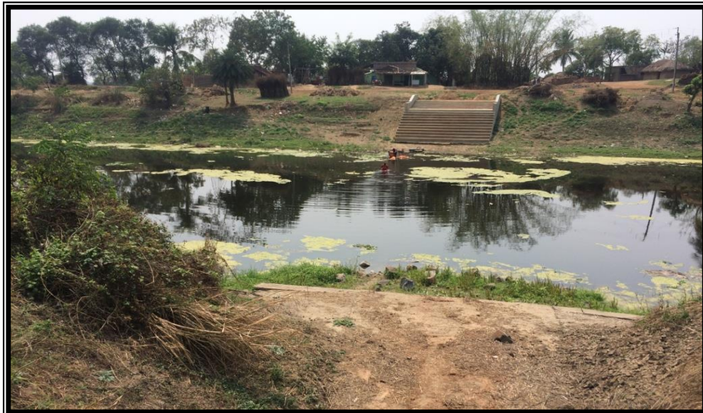
CHAINAGE 14.351 Km CONCRETE LADDER SHOKNA
