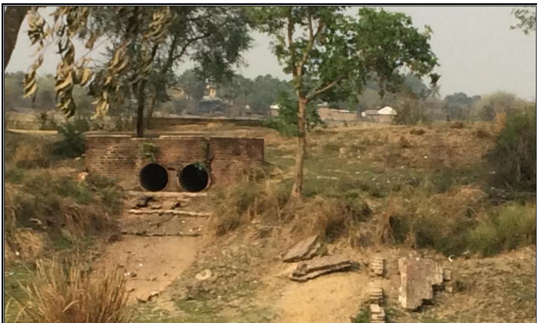
CHAINAGE 49.925 Km CULVERT SHARUL
