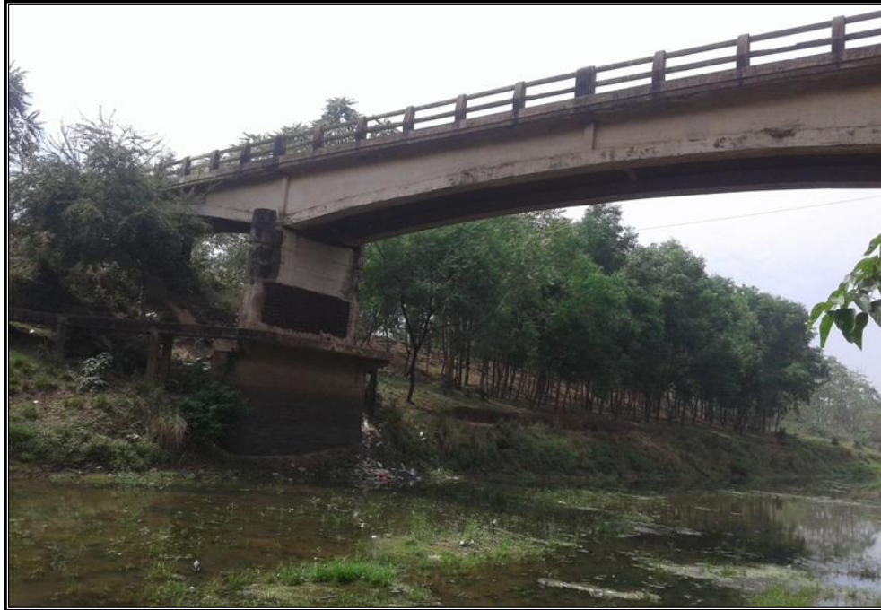
CHAINAGE 112.05 Km BRIDGE CHAU BERA
