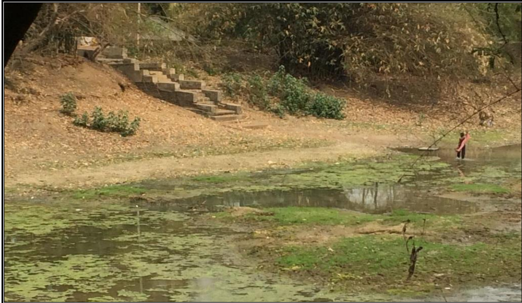
CHAINAGE 55.924 Km CONCRETE LADDER SASANGA
