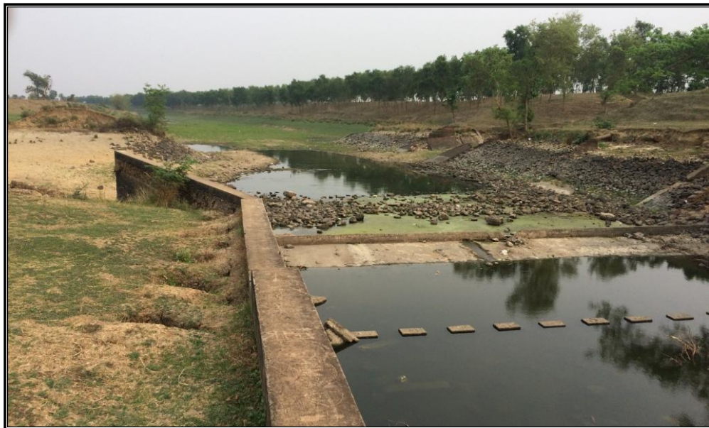
CHAINAGE 43.192 Km LOCK GATE RAMPUR_2
