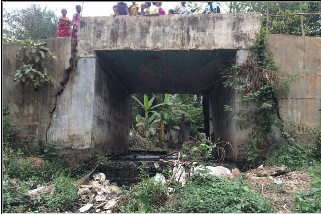
CHAINAGE 94.959 Km CULVERT KHANRO SARANI (JOLASAGAR)
