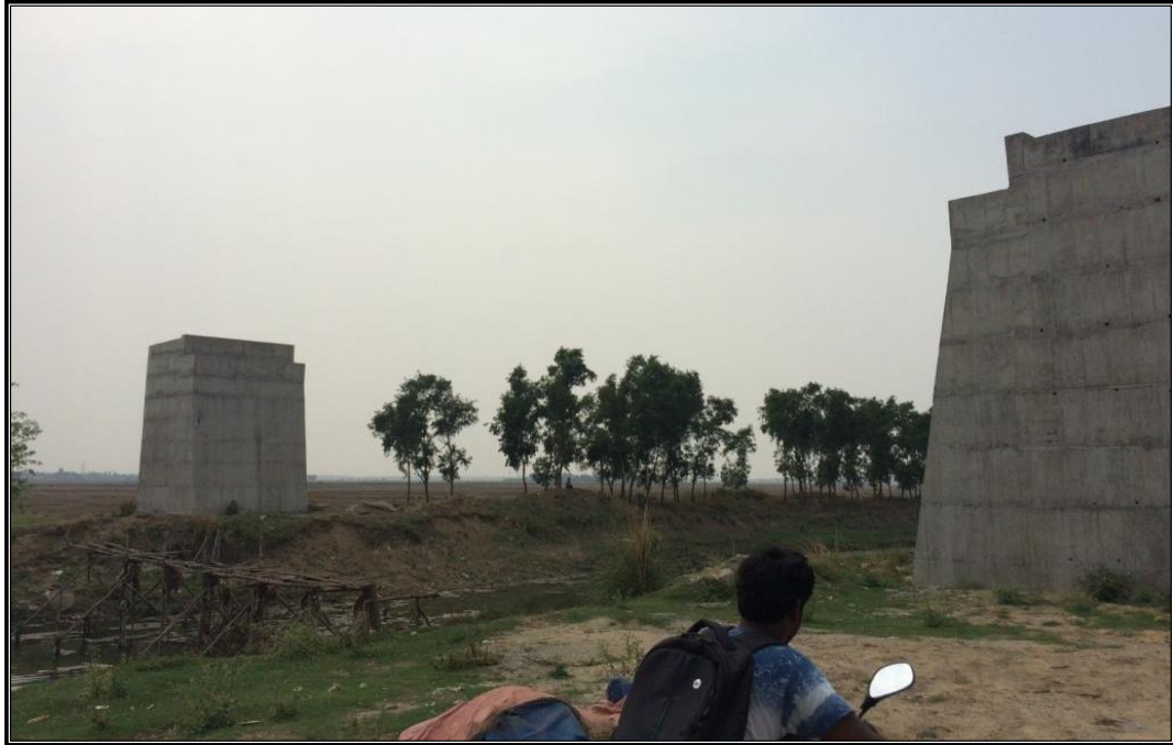
CHAINAGE 58.018 Km RAILWAY BRIDGE UNDER CONSTRUCTION NABABAHT
