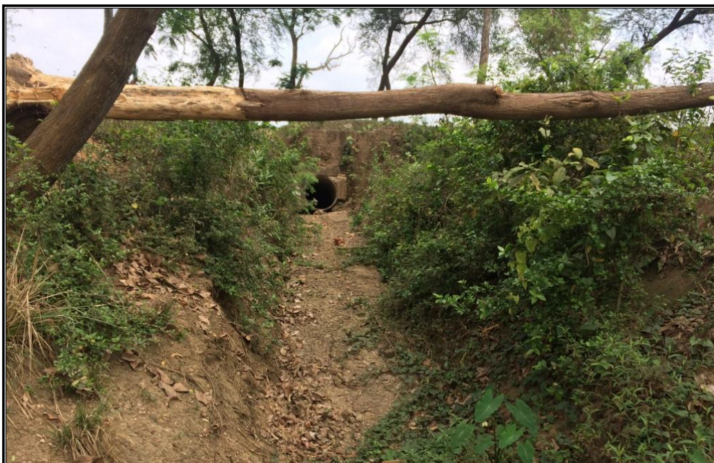
CHAINAGE 100.368 Km CULVERT BAGILA
