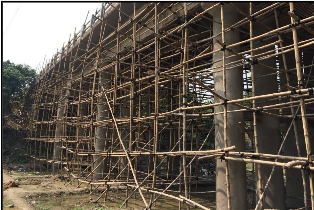
CHAINAGE 69.446 Km BRIDGE SADHARGHAT BURDWAN
