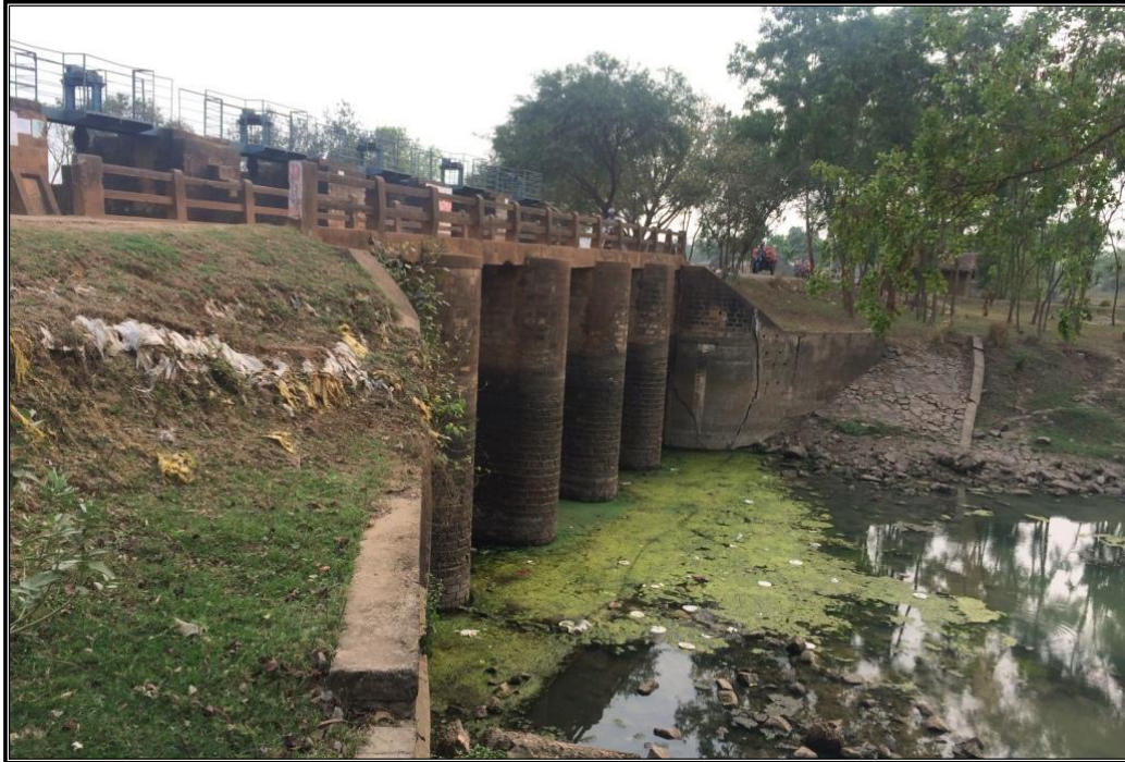
CHAINAGE 47.721 Km LOCK GATE CUM BRIDGE DARBARPUR_3
