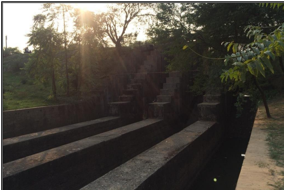
CHAINAGE 86.242 Km LOCK GATE PALLA COLONY
