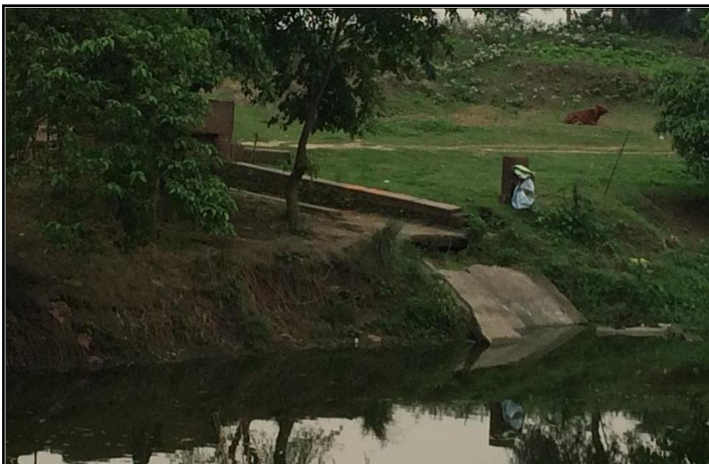
CHAINAGE 96.46 Km CULVERT KHANRO SARANI
