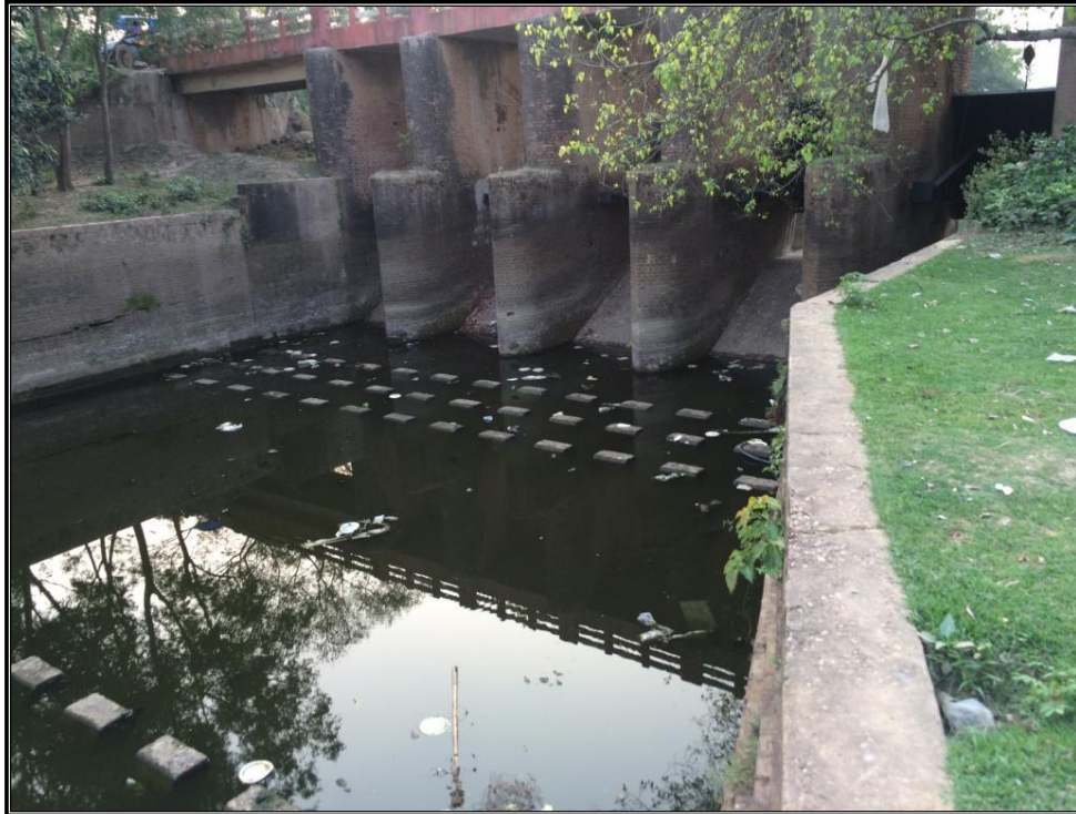
CHAINAGE 81.963 Km LOCK GATE DAKSHIN GOPALPUR (ROOPNATH PALLI)
