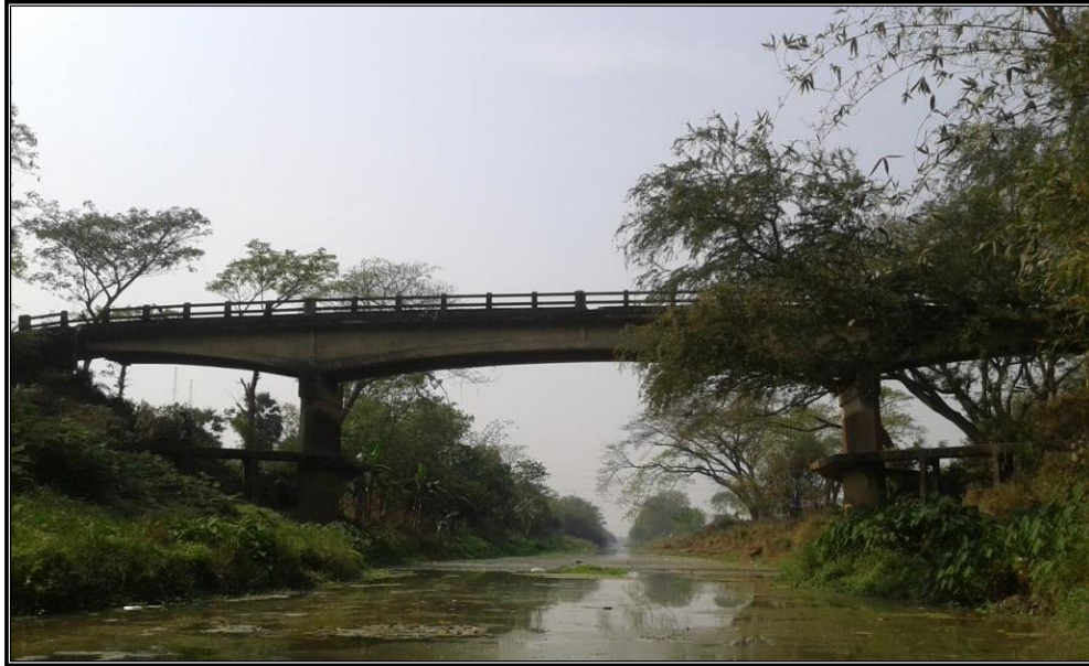
CHAINAGE 131.156 Km BRIDGE KHALSI
