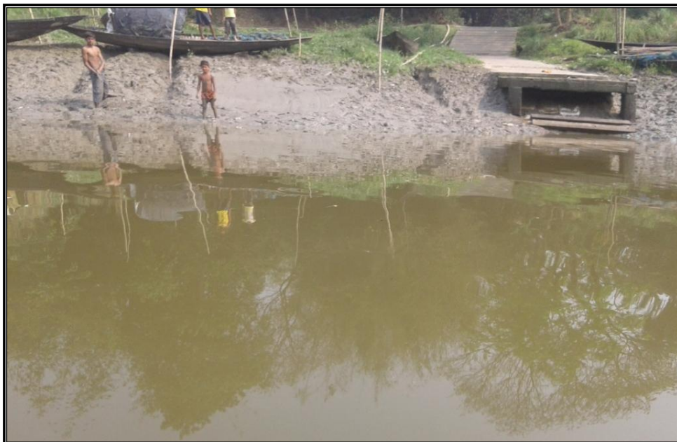
CHAINAGE 134.4 Km CONCRETE STRUCTURE NITYANANDPUR
