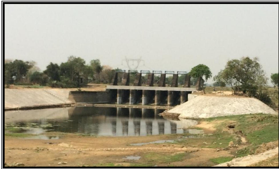
CHAINAGE 26.824 Km LOCK GATE KRISHNARAMPUR
