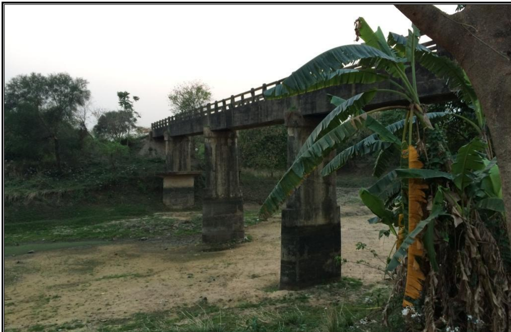
CHAINAGE 79.08 Km BRIDGE BELNA
