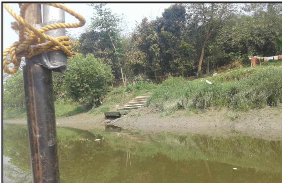
CHAINAGE 133.9 Km CONCRETE STRUCTURE NITHYANANDPUR
