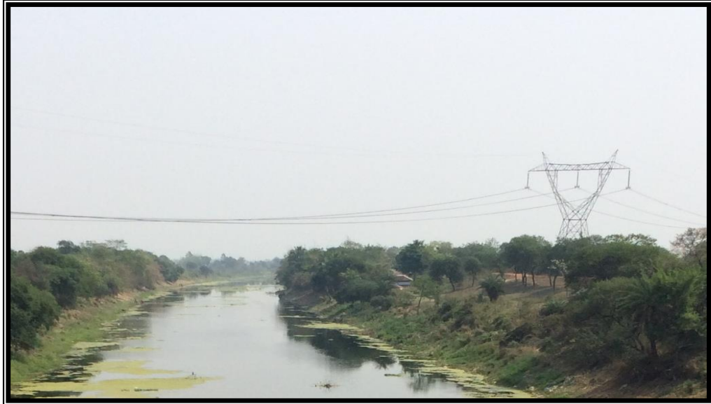
CHAINAGE 13.507 Km HIGH TENSION LINE SHOKNA
