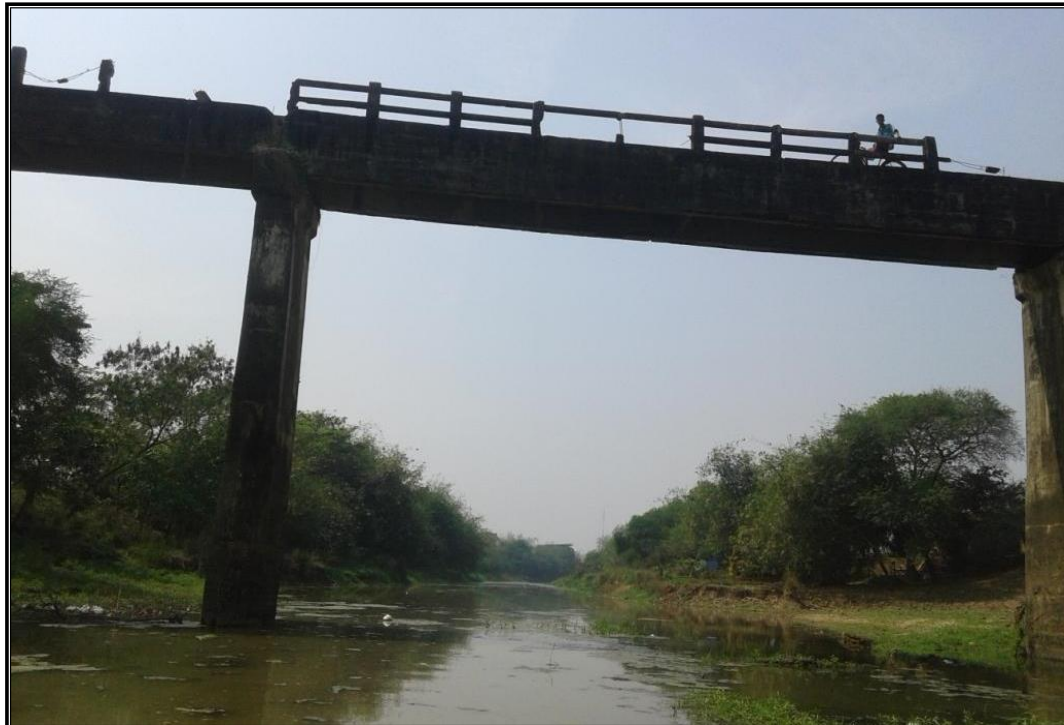
CHAINAGE 129.92 Km BRIDGE DIGSUI
