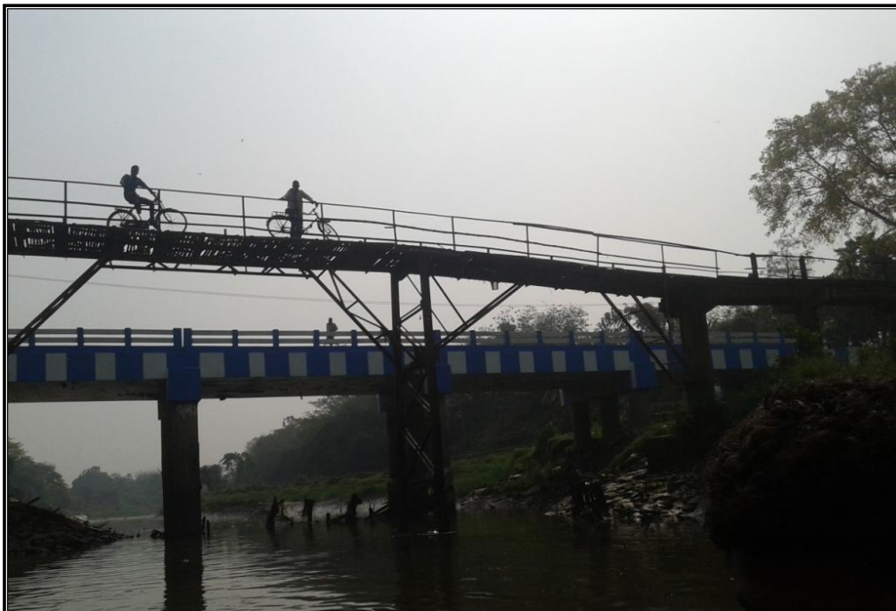
CHAINAGE 133.02 Km METAL BRIDGE AND CONCRETE BRIDGE DAKSHIN GOPALPUR
