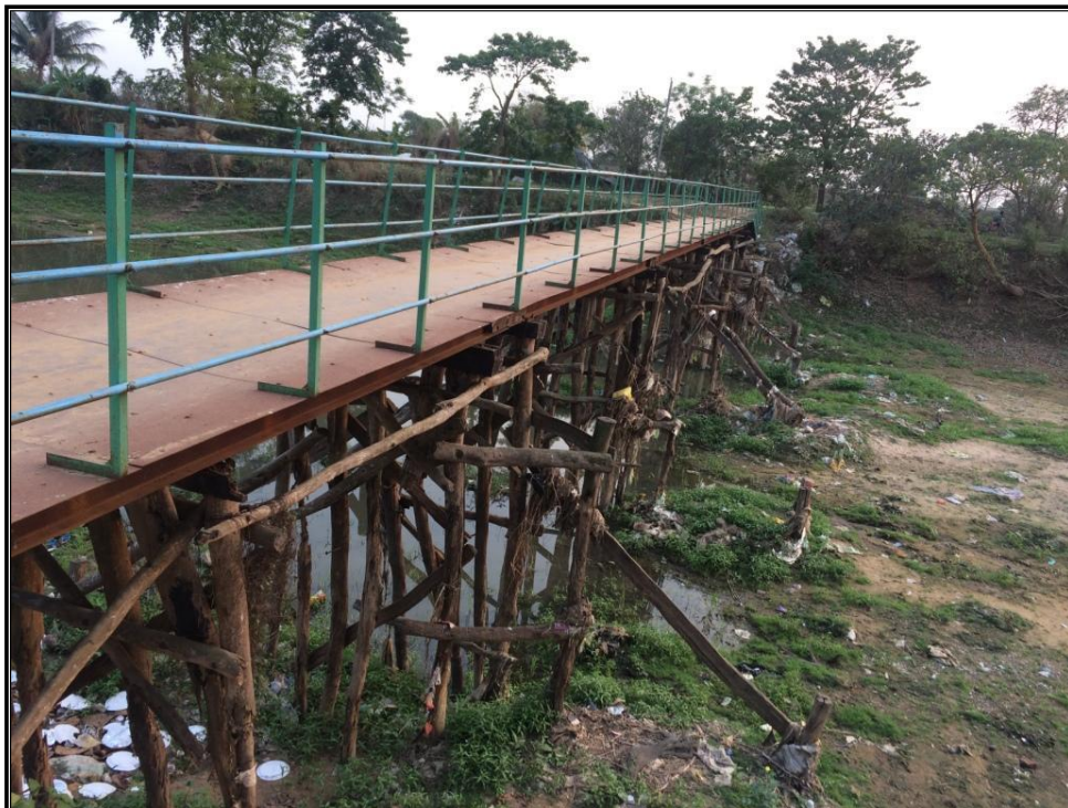
CHAINAGE 82.259 Km WOODEN BRIDGE DAKSHIN GOPALPUR
