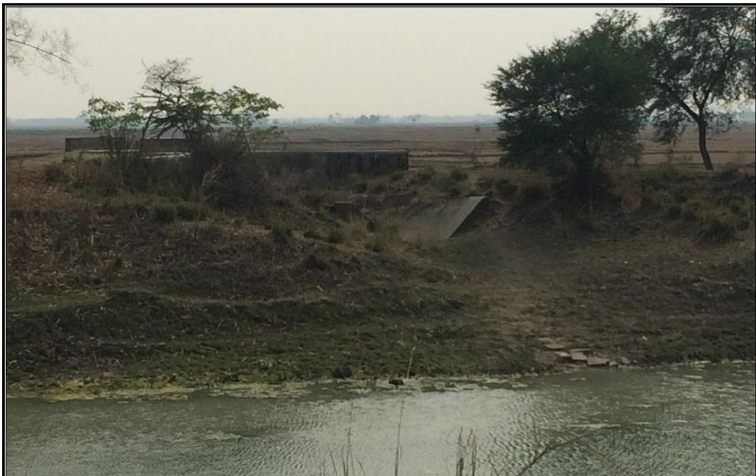
CHAINAGE 53.49 Km CULVERT MOHANPUR
