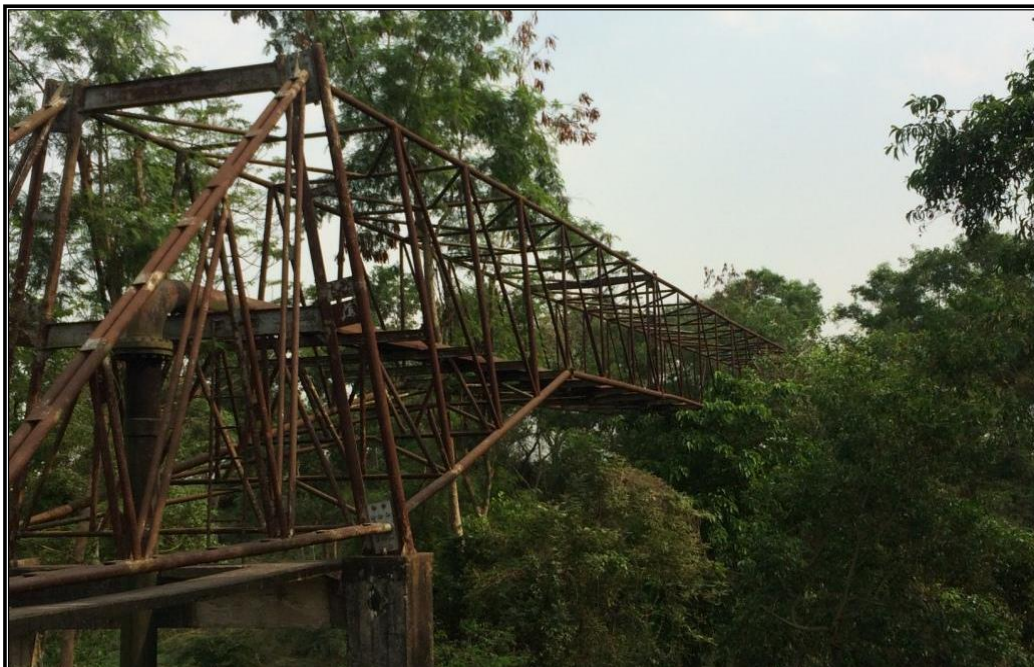
CHAINAGE 88.66 Km GAS PIPE LINE CROSSING OVER CHANCHAI_1
