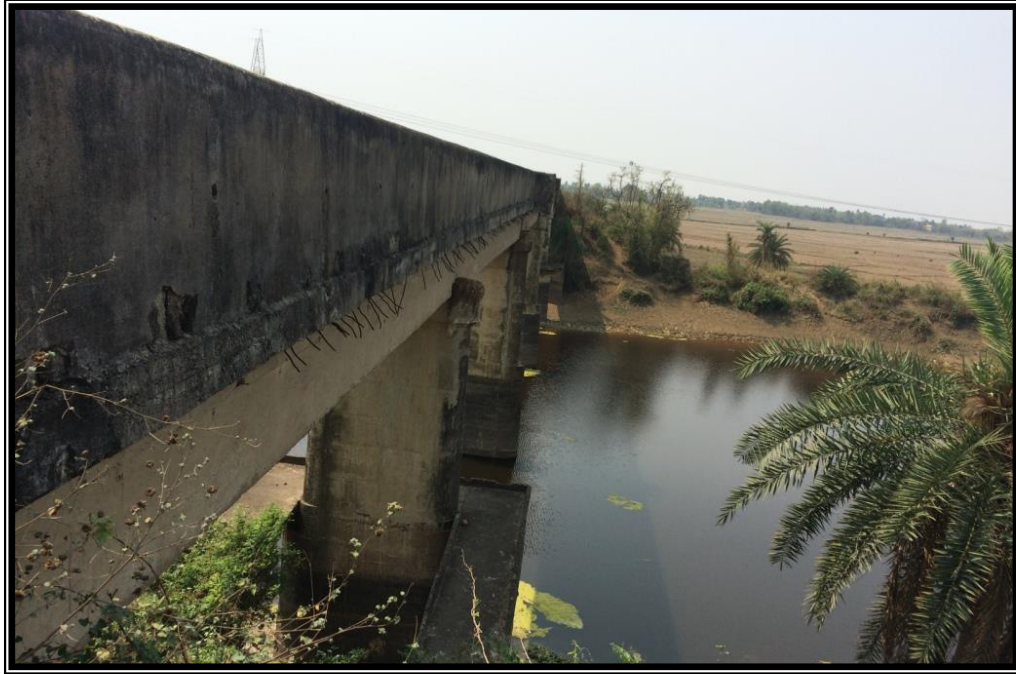
CHAINAGE 19.95 Km BRIDGE BHARATPUR
