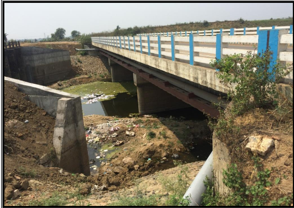
CHAINAGE 16.546 Km BRIDGE PRAYAGPUR
