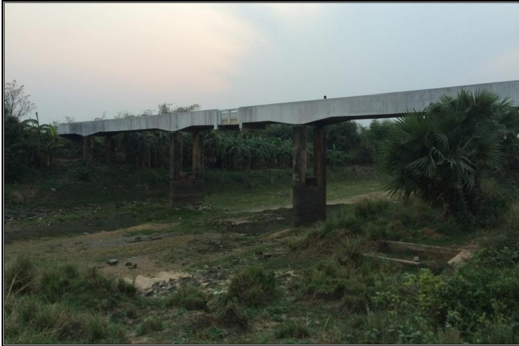
CHAINAGE 78.089 Km BRIDGE AMIRPUR
