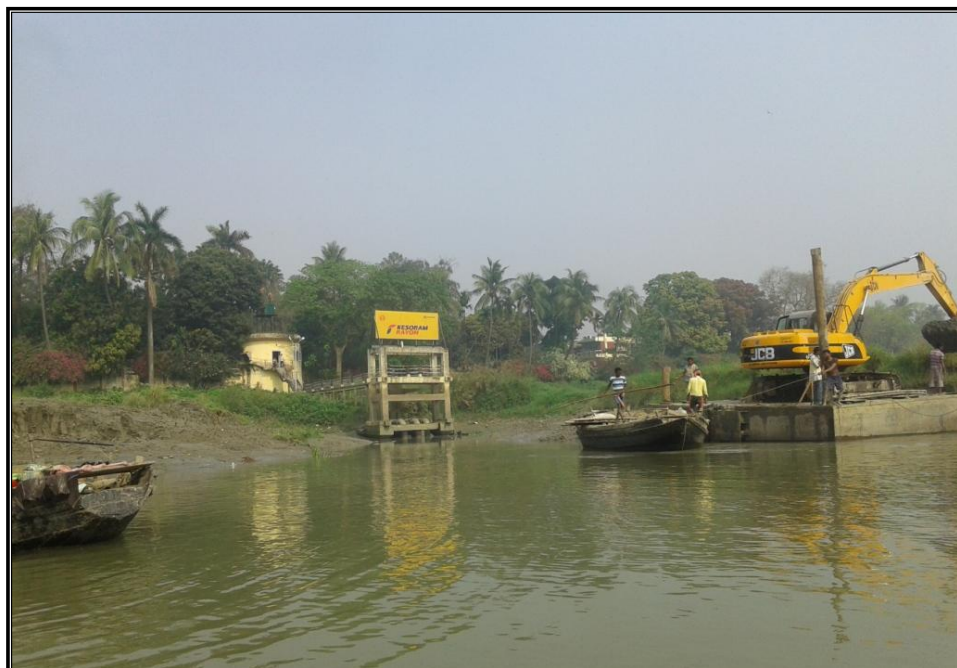
CHAINAGE 136.4 Km NAYA SARAYA
