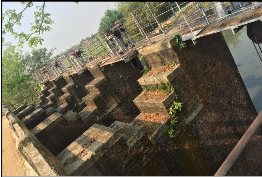
CHAINAGE 76.764 Km LOCK GATE CHAITPUR_1
