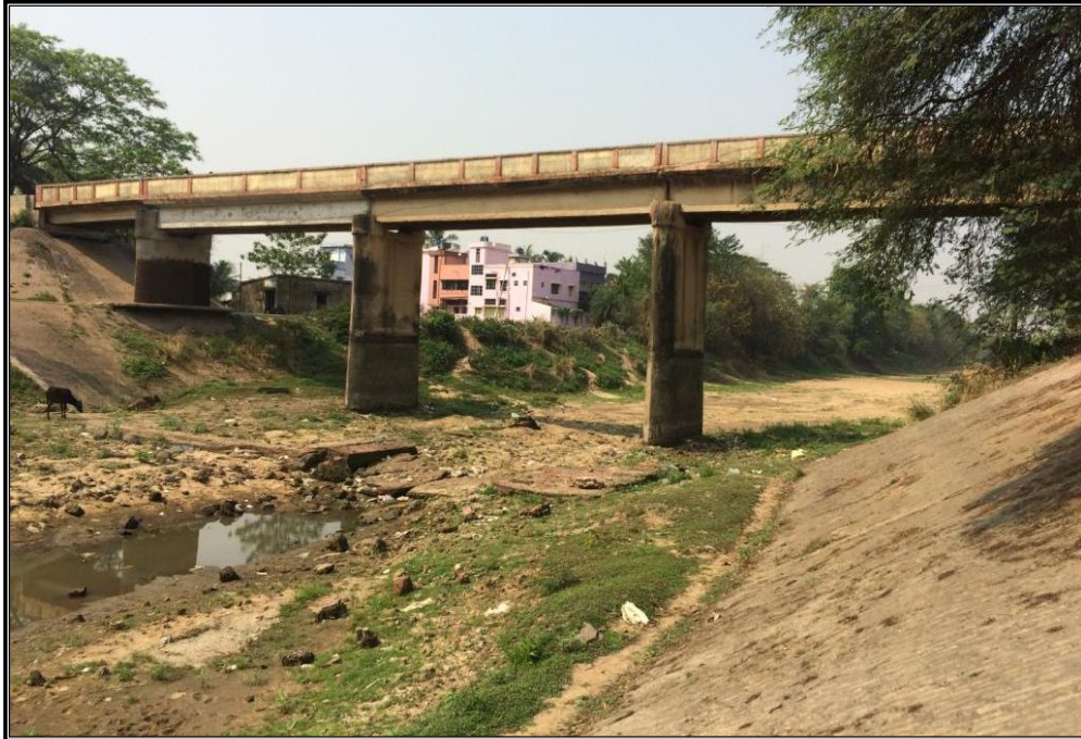
CHAINAGE 73.026 Km BRIDGE PALLA
