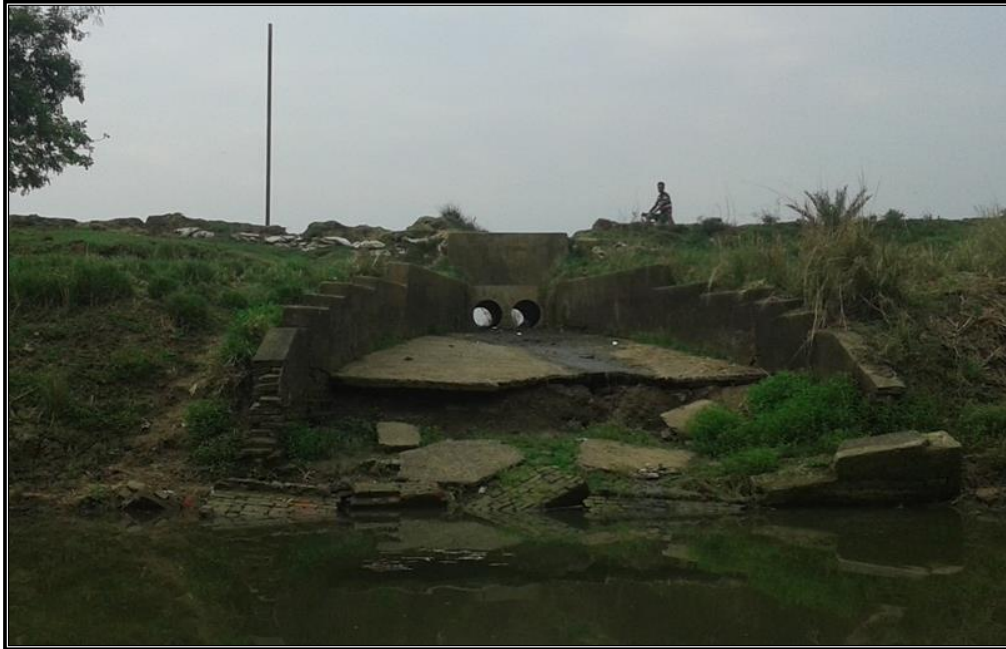
CHAINAGE 114.773 Km CULVERT TINNA
