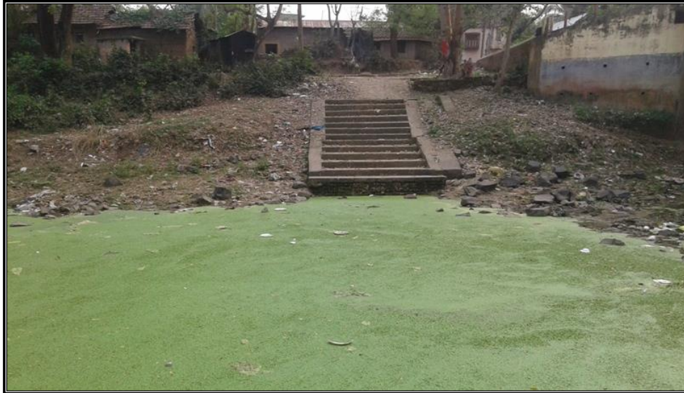
CHAINAGE 118.44 Km CONCRETE LADDER PANDUA
