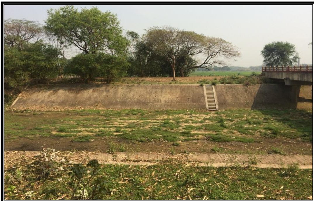
CHAINAGE 74.548 Km CONCRETE PAVEMENT AT DVC PAMRA
