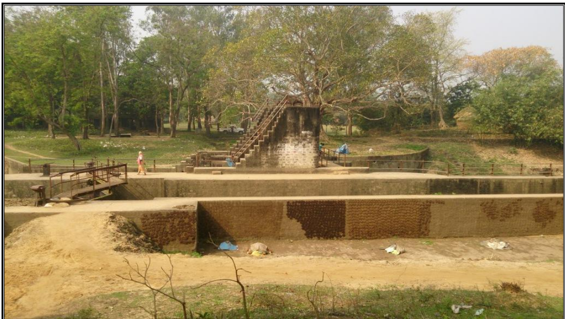
CHAINAGE 126.21 Km LOCK GATE HOERA_1
