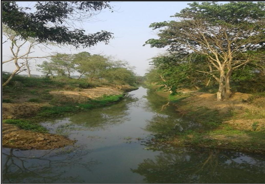
CHAINAGE 105.942 Km SMALL CANAL KOCHMALI
