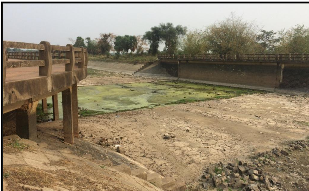
CHAINAGE 44.7 Km UNDERPASS CANAL HARIPUR
