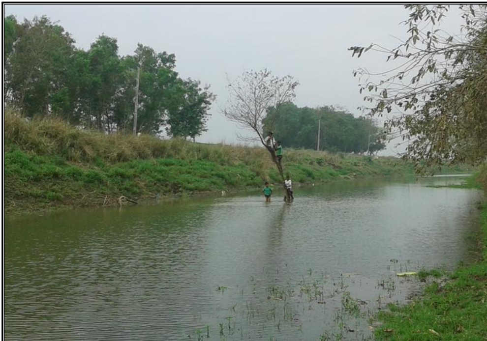
CHAINAGE 14.845 Km TINNA
