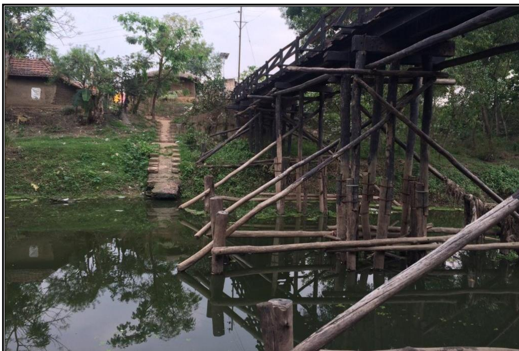
CHAINAGE 96.907 Km CONCRETE LADDER AND WOODEN BRIDGE DILALPUR
