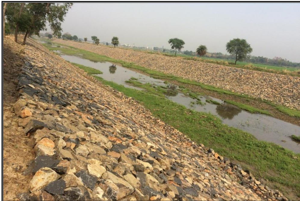
CHAINAGE 75.82 Km TO 75.376 Km STONE PITCHING AT DVC CANAL CHAITPUR
