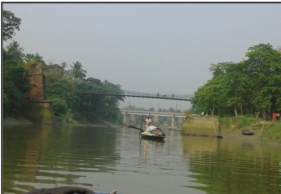
CHAINAGE 135.4 Km KATLA HANGING BRIDGE SERPUR
