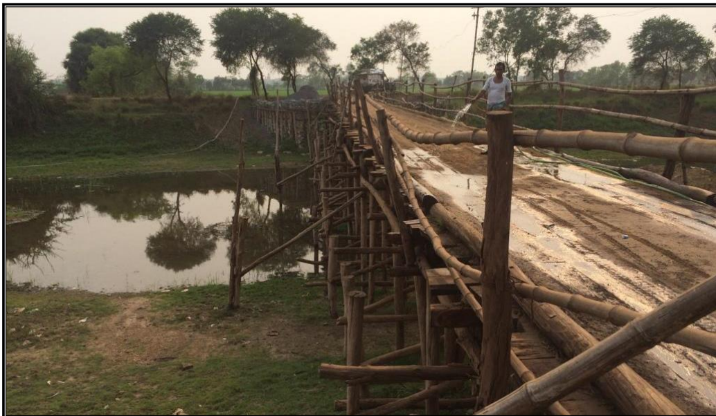
CHAINAGE 45.953 Km WOODEN BRIDGE KHETURA
