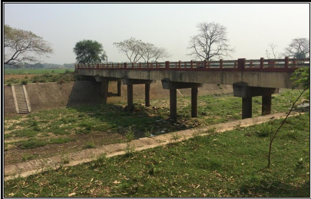
CHAINAGE 74.595 Km BRIDGE PAMRA
