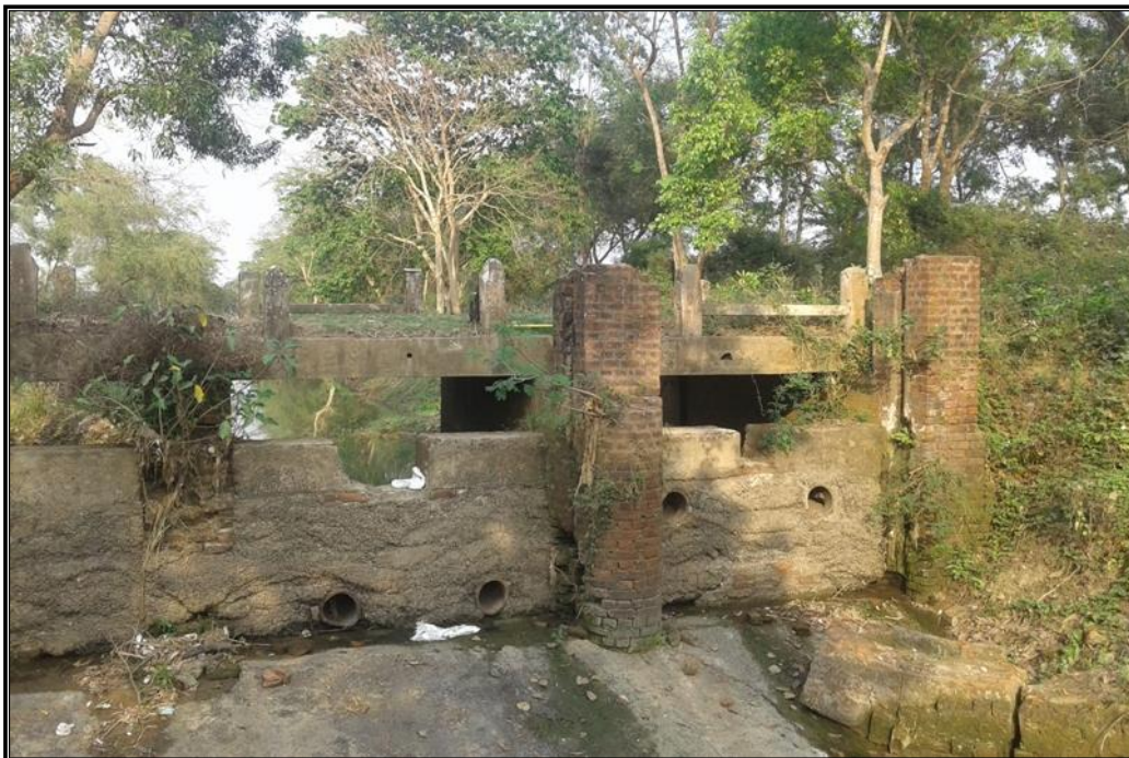
CHAINAGE 105.942 Km CULVERT KOCHMALI
