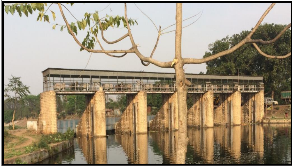
CHAINAGE 0.175 Km LOCK GATE SUKUMARNAGAR
