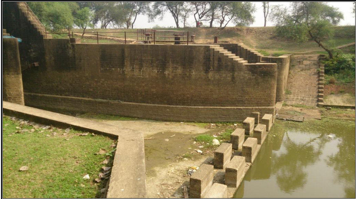
CHAINAGE 126.21 Km LOCK GATE HOERA_2
