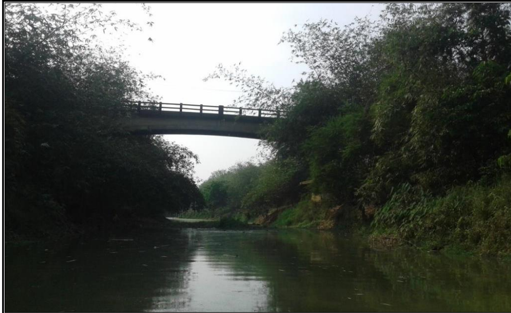
CHAINAGE 127.70 Km BRIDGE CHANPARAI
