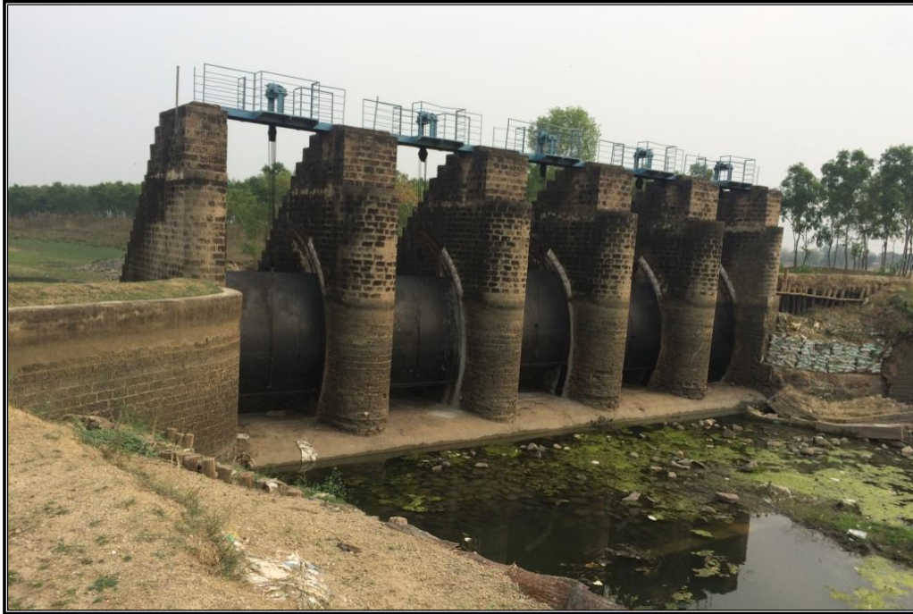
CHAINAGE 43.192 Km LOCK GATE RAMPUR
