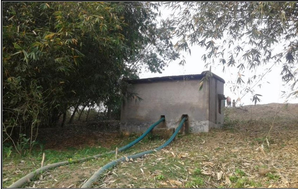
CHAINAGE 104.557 Km PUMP HOUSE DEBIPUR
