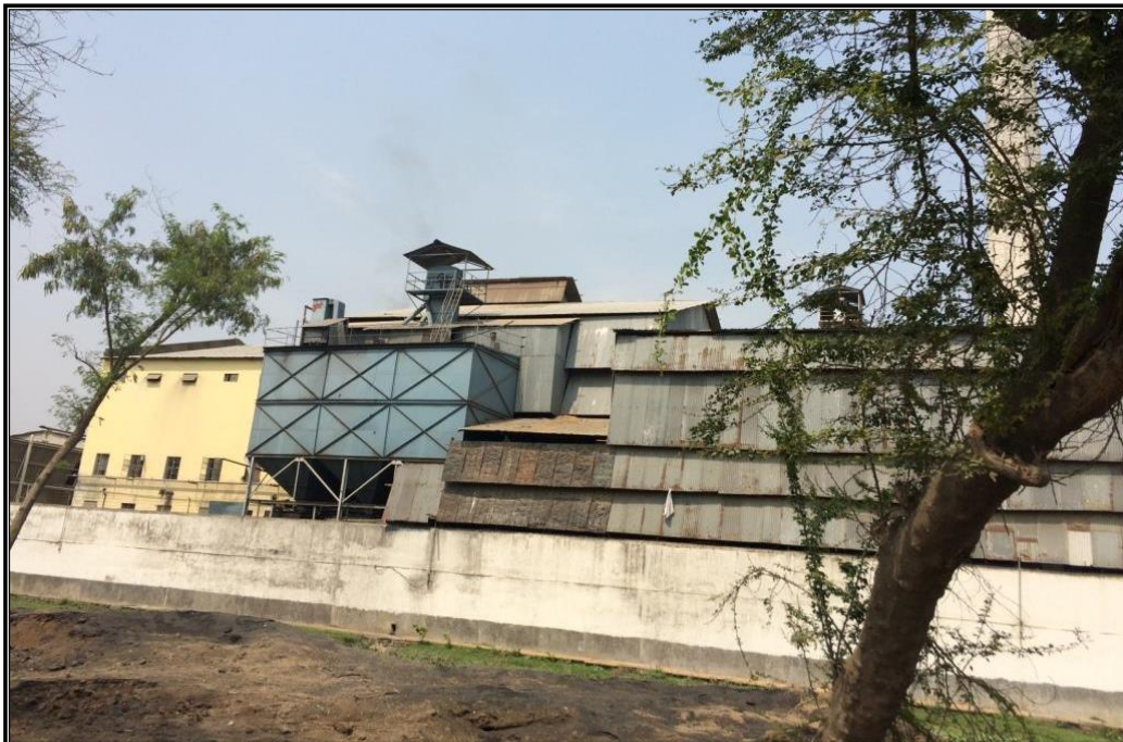
CHAINAGE 61.149 Km RICE MILL KASIMPUR
