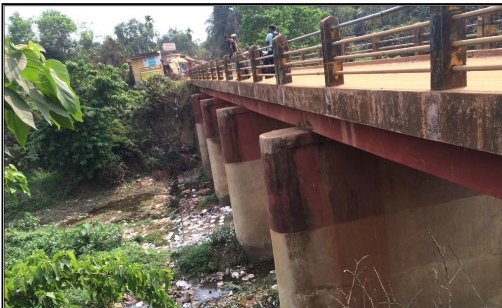
CHAINAGE 92.603 Km BRIDGE MAHESH DANGA
