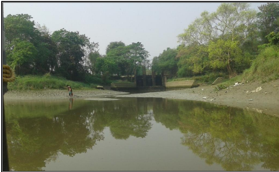
CHAINAGE 132.14 Km LOCK GATE GOPALPUR
