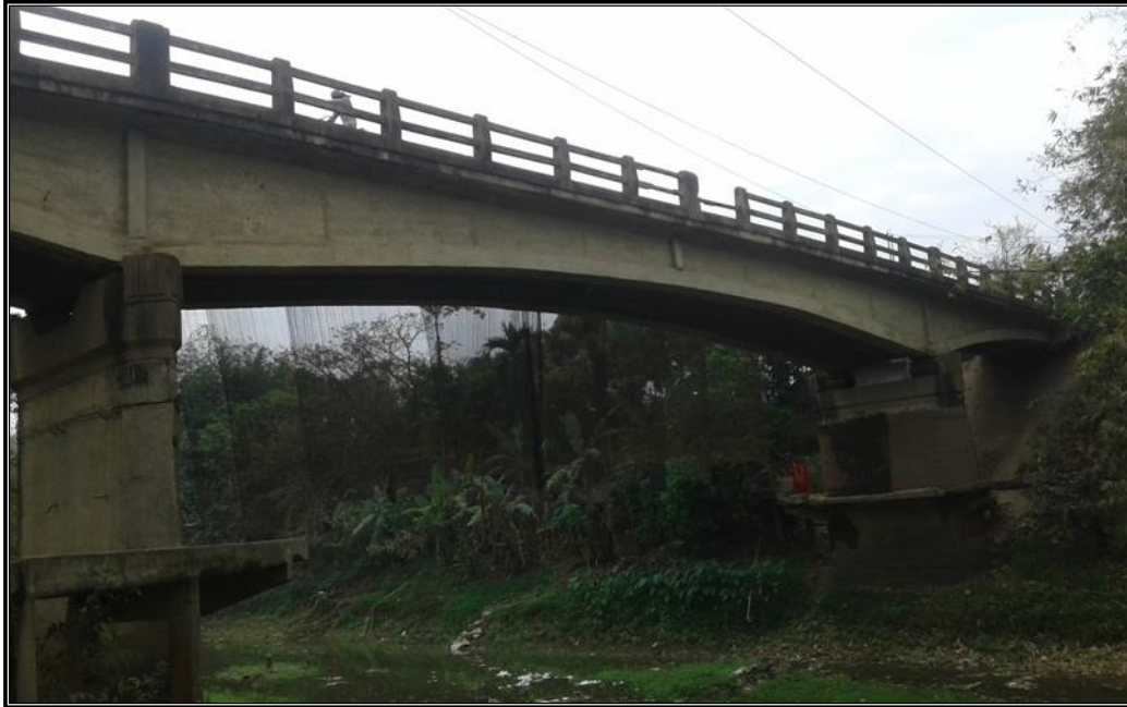
CHAINAGE 115.677 Km BRIDGE TINNA
