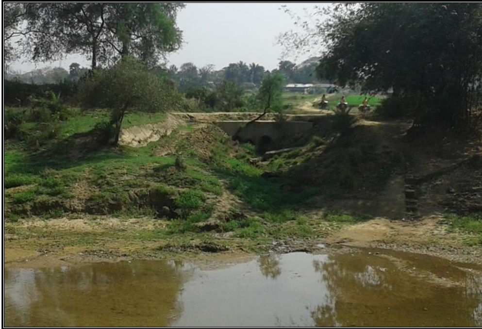
CHAINAGE 110.013 Km CULVERT BOINCHI GRAM
