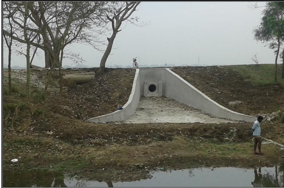
CHAINAGE 113.615 Km CULVERT SIMLAGARH
