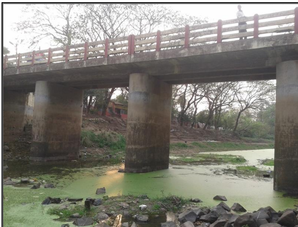
CHAINAGE 118.42 Km BRIDGE PANDUA(BHAJANPUR)
