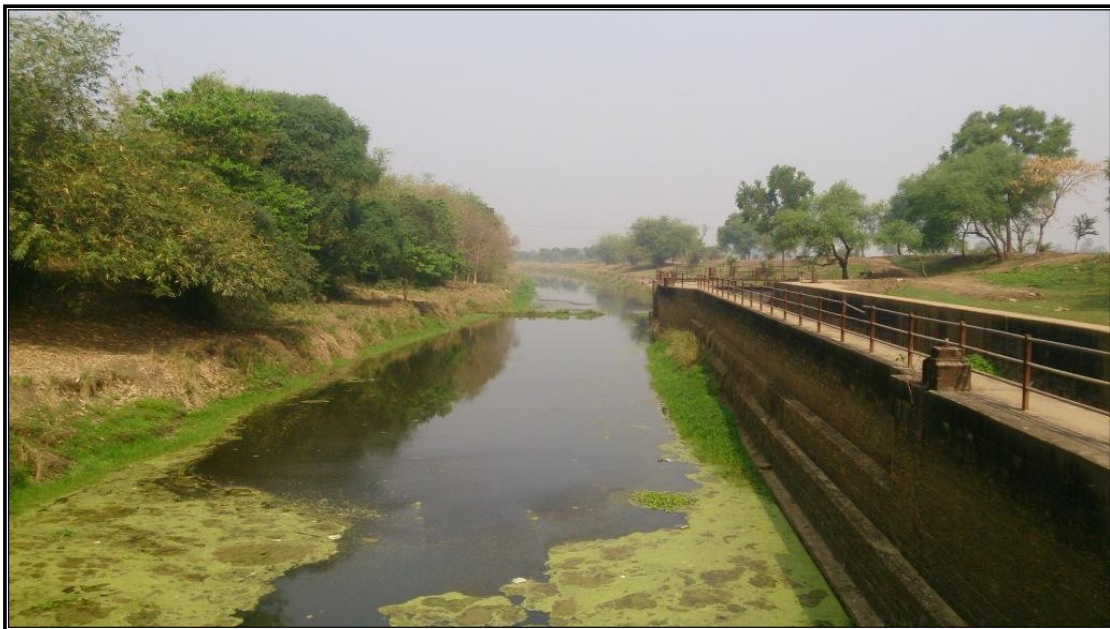
CHAINAGE 126.21 Km LOCK GATE HOERA_3
