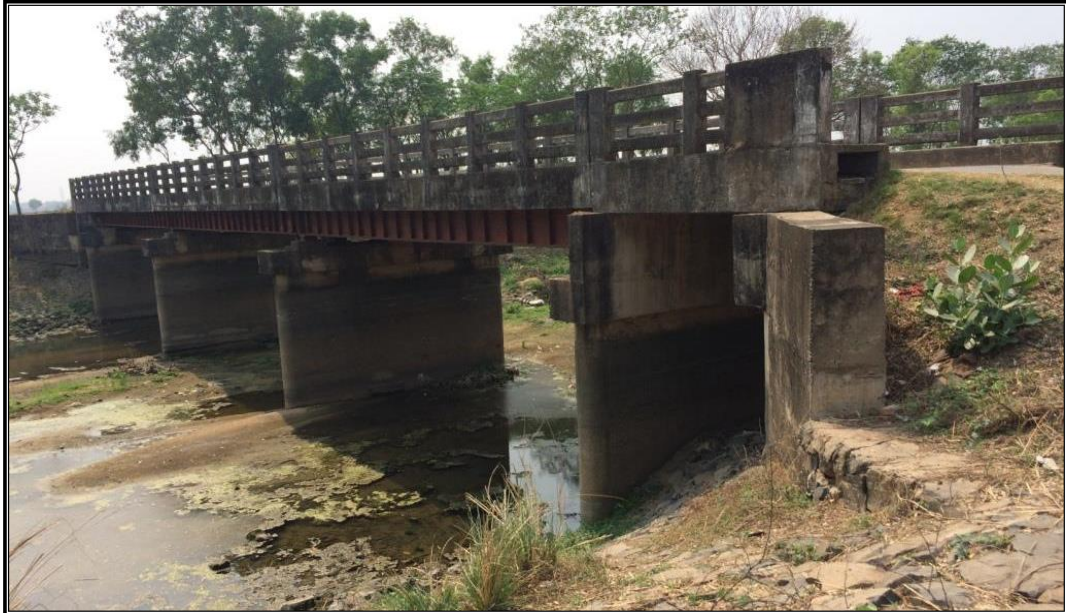
CHAINAGE 58.713 Km BRIDGE NALA
