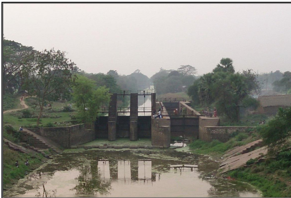
CHAINAGE 119.177 Km LOCK GATE PANDUA
