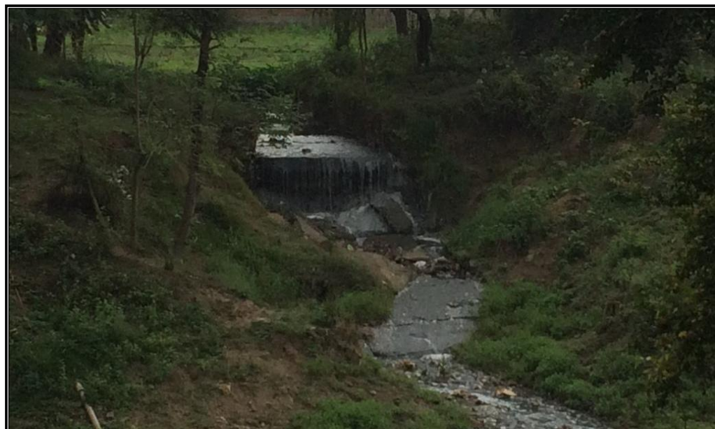
CHAINAGE 98.246 Km DRAINAGE BAGILA (GODHIPUR)
