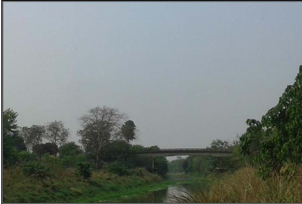
CHAINAGE 123.00 Km BRIDGE TANBA
