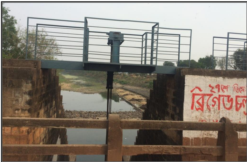
CHAINAGE 47.721 Km LOCK GATE CUM BRIDGE DARBARPUR_2
