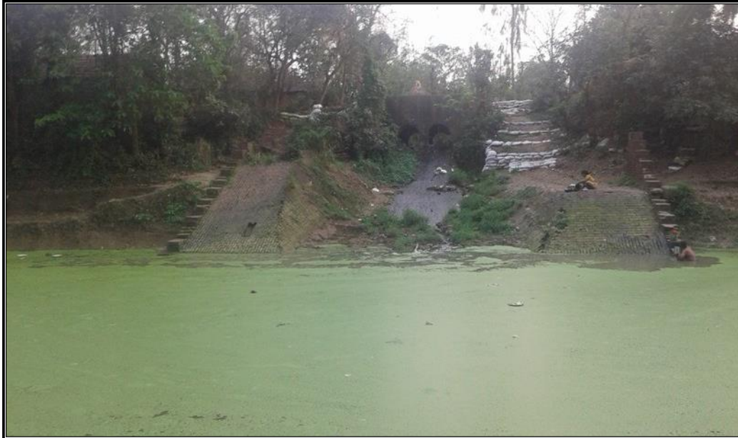
CHAINAGE 117.785 Km CULVERT MAHADEBPUR
