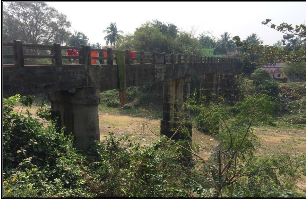
CHAINAGE 71.51 Km BRIDGE BECHARHAT
