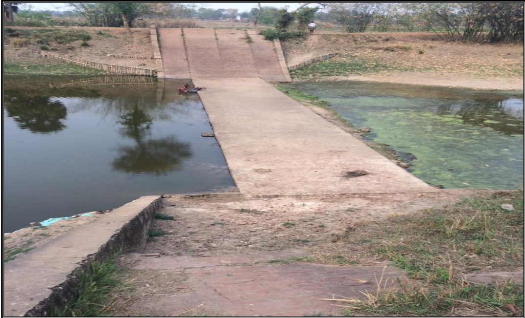
CHAINAGE 49.208 Km UNDERPASS CANAL DALPUR
