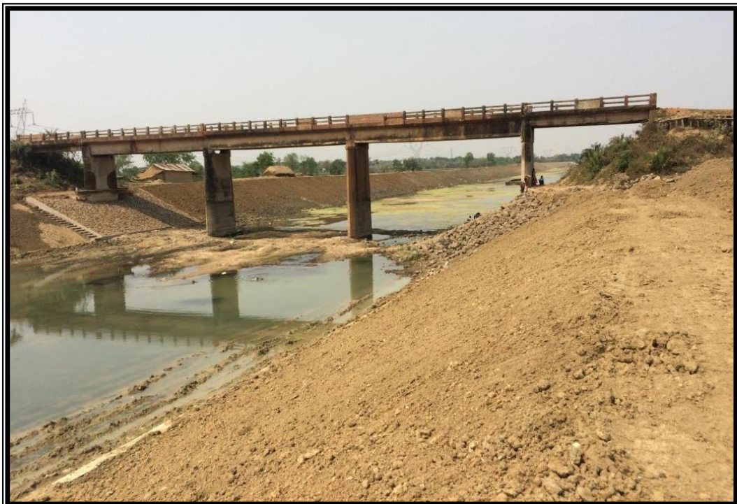
CHAINAGE 28.483 Km BRIDGE PARDAH
