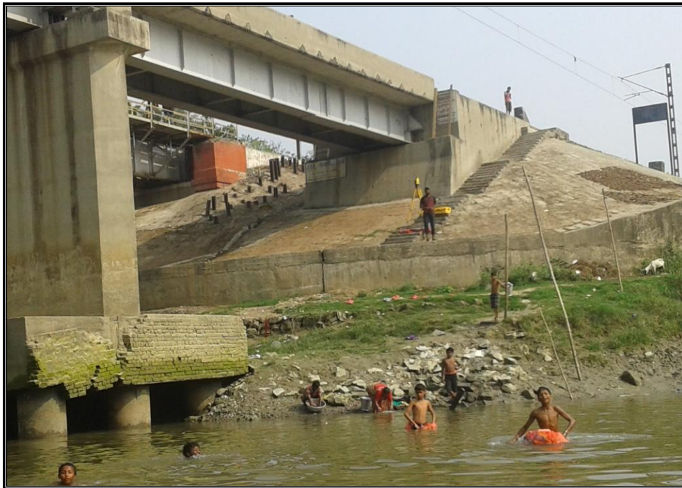
CHAINAGE 135.2 Km RAILWAY BRIDGE KUNTIGHAT_1
