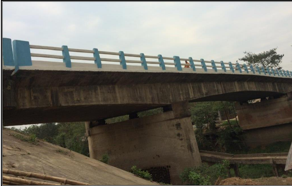
CHAINAGE 95.035 Km BRIDGE KHANRO SARANI(JOLASAGAR)
