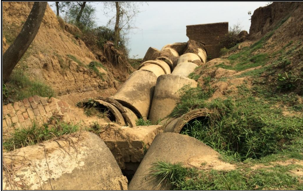
CHAINAGE 101.379 Km CULVERT BAGILA
