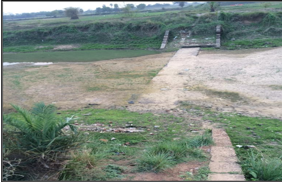
CHAINAGE 80.826 Km UNDER PASSING CANAL TOTPARA
