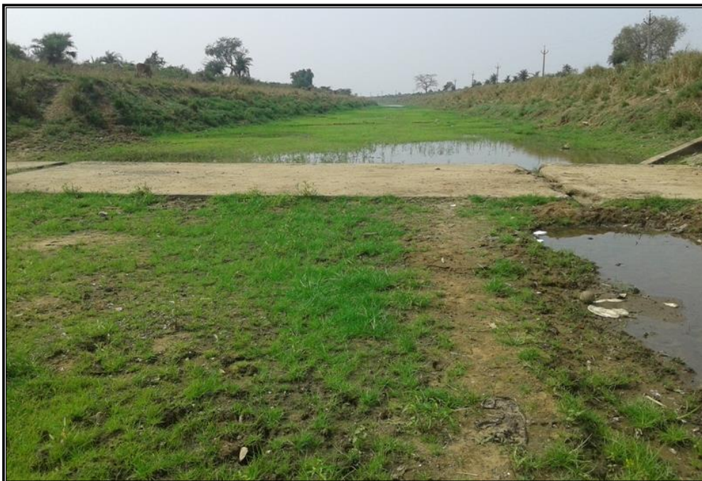
CHAINAGE 122.326 Km UNDERPASS CANAL NIALA
