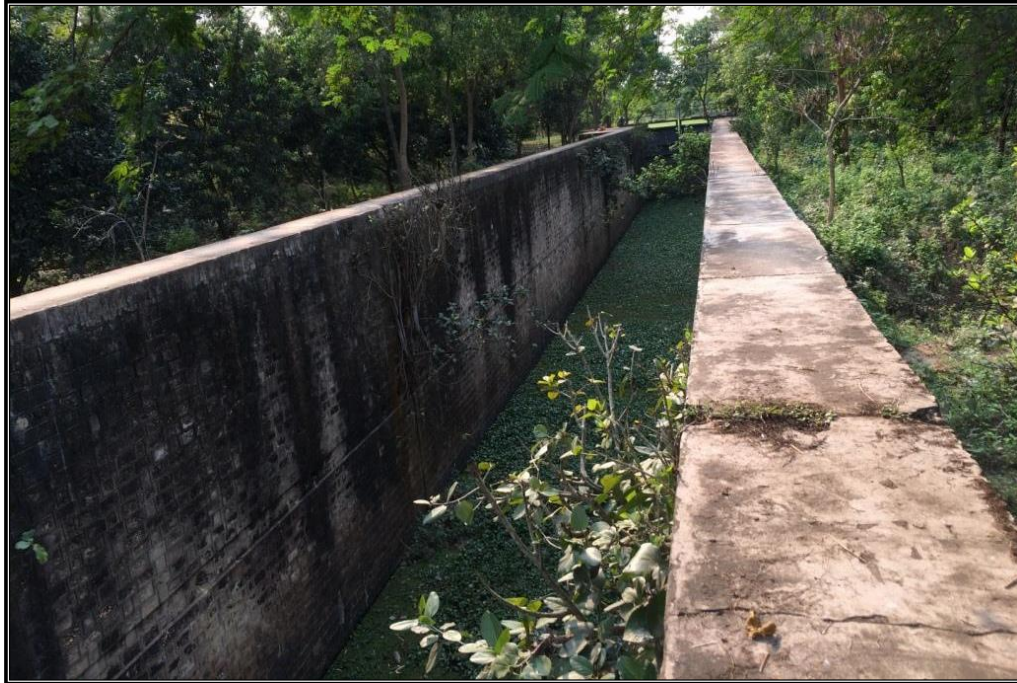
CHAINAGE 88.025 Km LOCK GATE MAHESPUR_1
