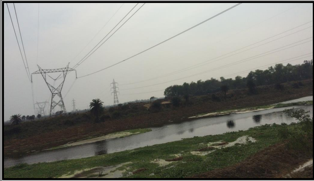
CHAINAGE 6.573 Km HIGH TENSION LINE BANSKOPA
