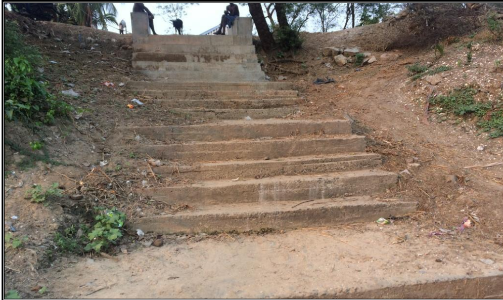
CHAINAGE 84.373 Km CONCRETE LADDER PALLA
