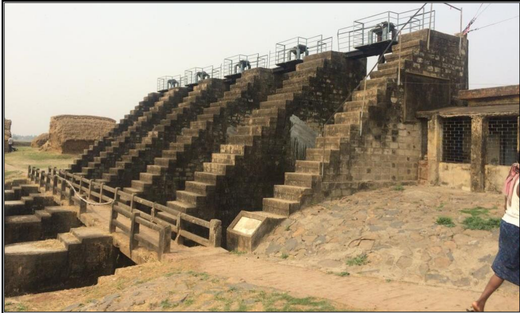
CHAINAGE 39.953 Km LOCK GATE PURSA
