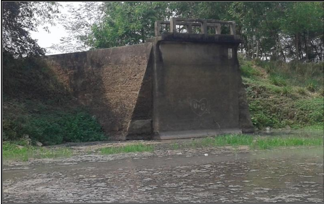
CHAINAGE 125.419 Km UNDERPASS CANAL MADHUSUDANPUR
