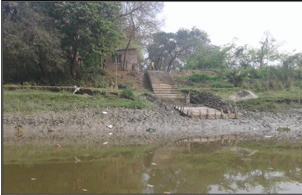
CHAINAGE 133.3 Km CONCRETE LADDER DAKSHIN GOPALPUR
