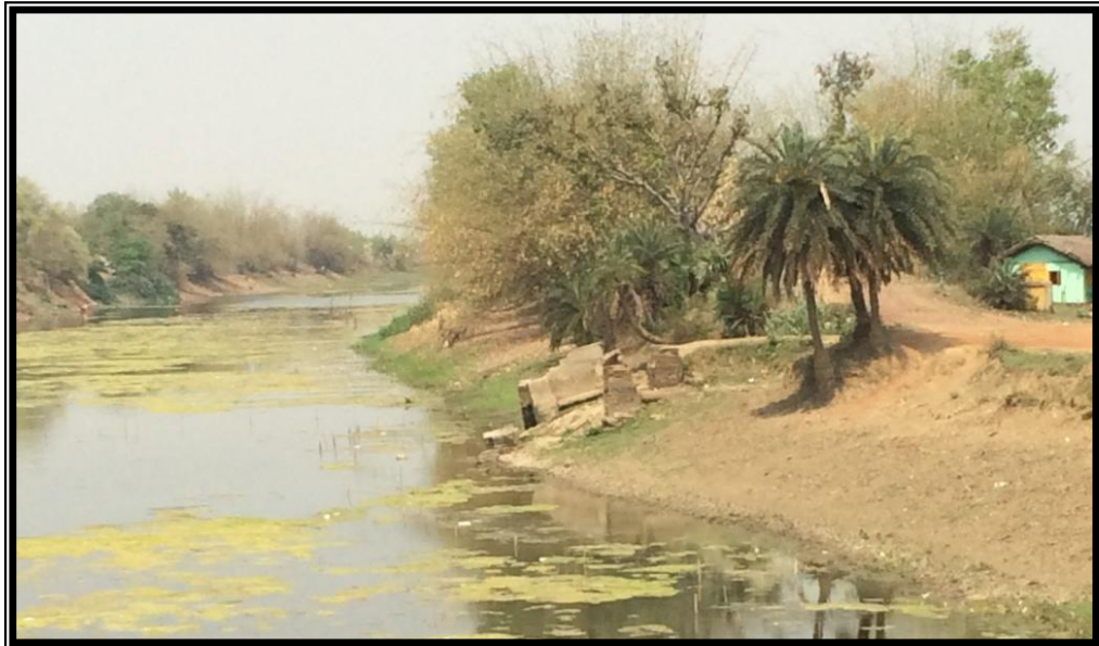
CHAINAGE 22.057 Km CULVERT SHALDANGA
