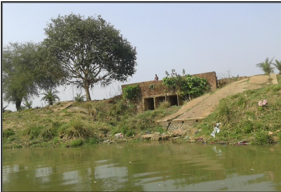
CHAINAGE 128.80 Km CULVERT TARAGOON
