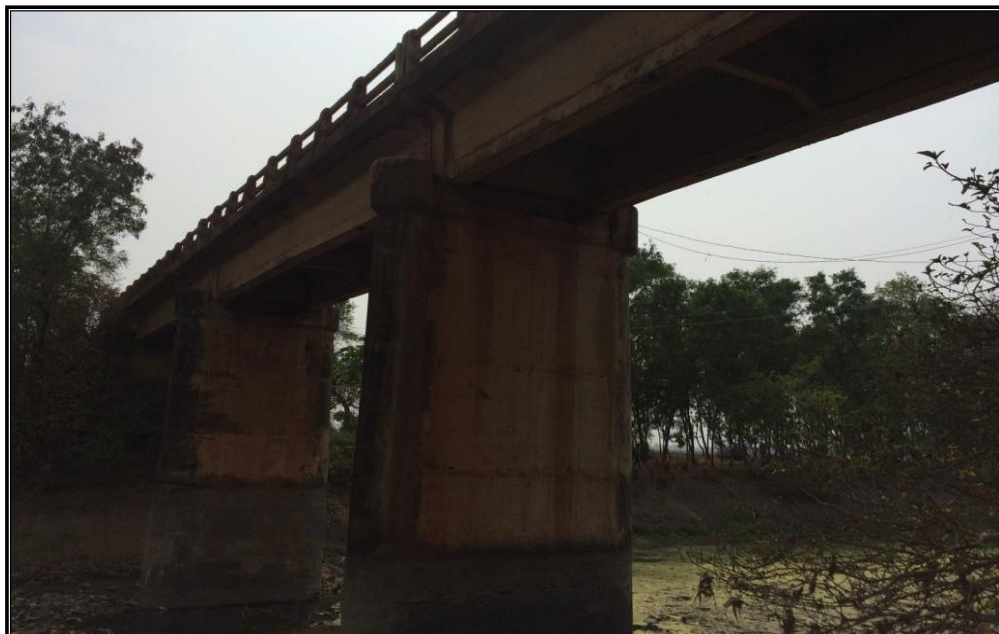
CHAINAGE 56.559 Km BRIDGE SASANGA
