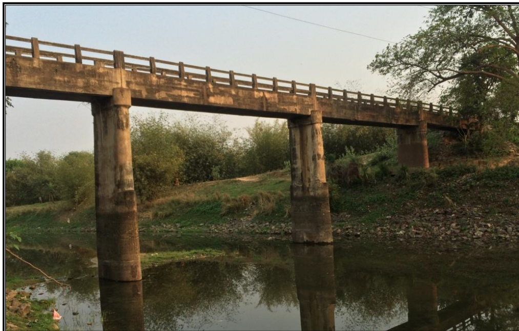
CHAINAGE 84.491 Km BRIDGE PASCHIM PALLA
