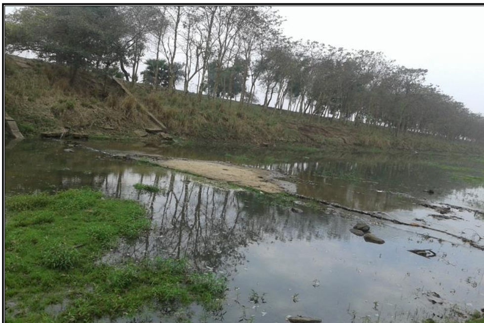
CHAINAGE 113.929 Km UNDERPASS CANAL SIMLAGARH
