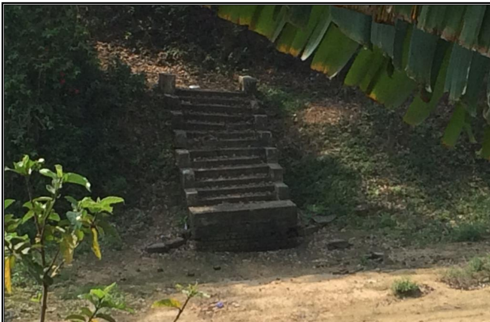
CHAINAGE 72.074 Km CONCRETE LADDER SIBATLA
