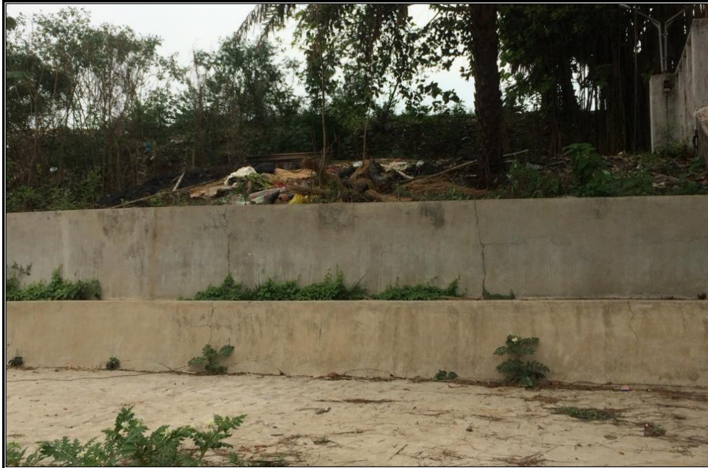
CHAINAGE 98.227 Km CEMETRY BAGILA (NUDIPUR)
