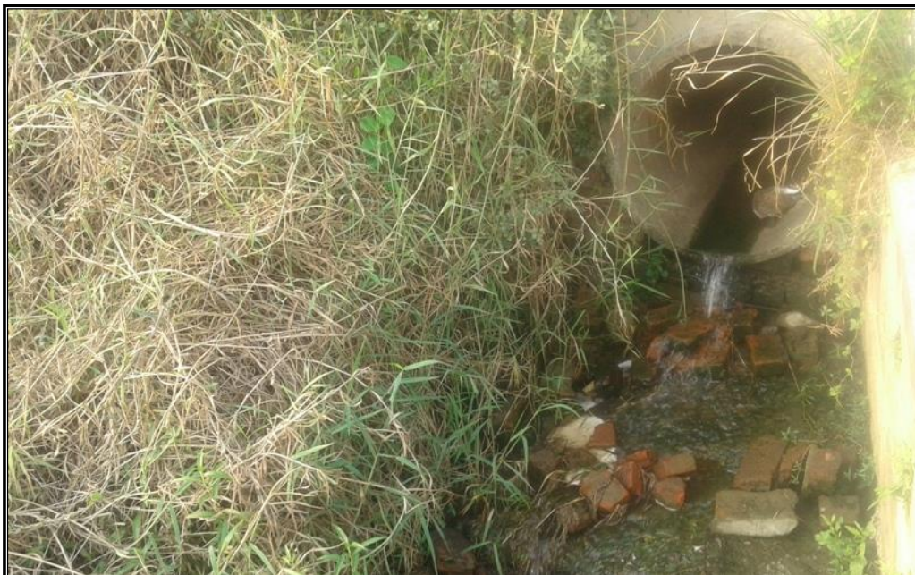
CHAINAGE 105.436 Km CULVERT KOCHIMALI
