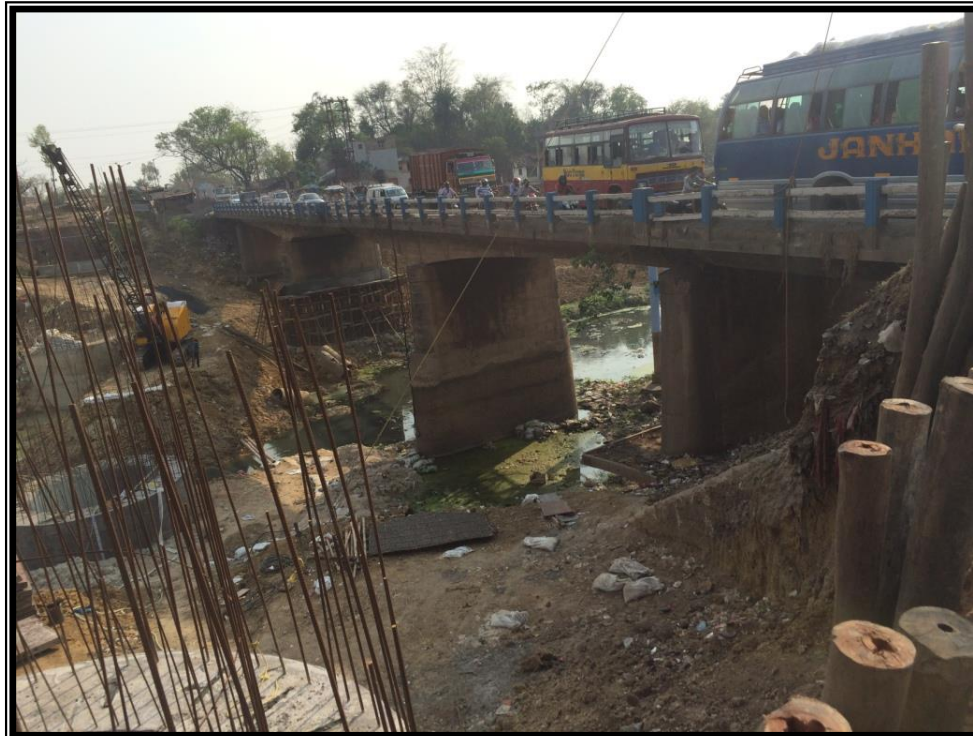
CHAINAGE 2.0 Km BRIDGE NETAJI SUBHASH PALLY
