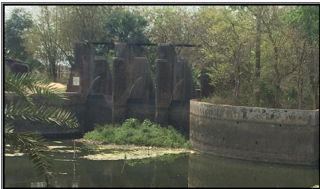
CHAINAGE 22.654 Km LOCK GATE TO DAMODAR RIVER RANDIHA
