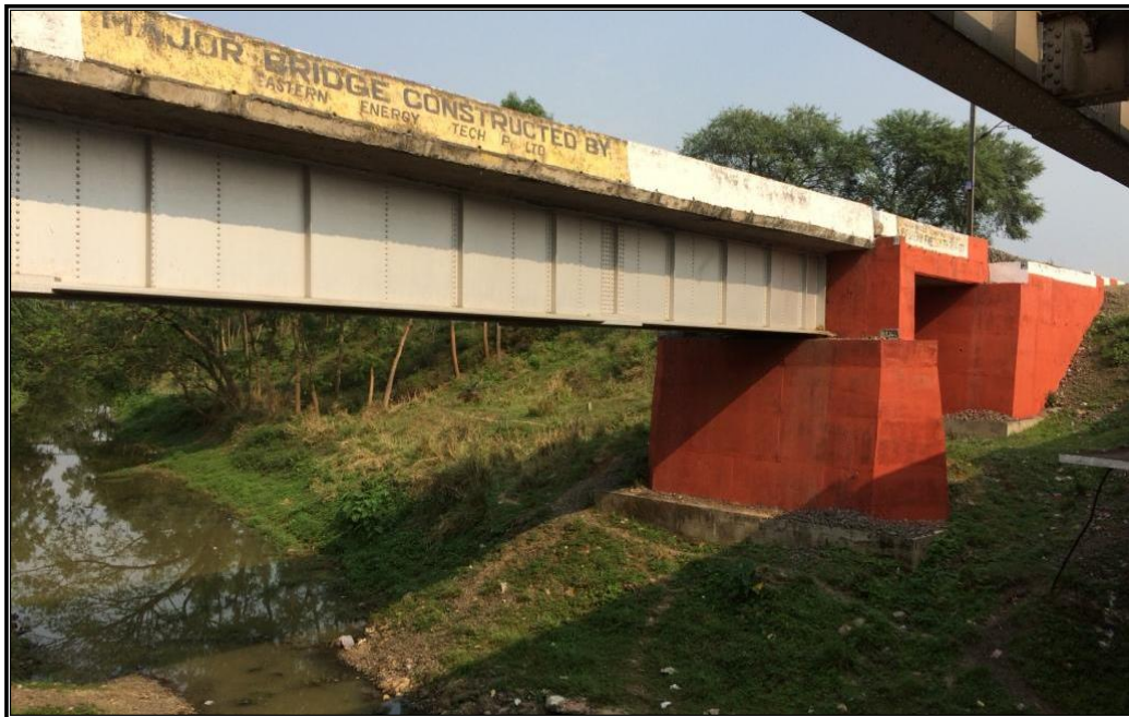
CHAINAGE 88.47 Km RAILWAY BRIDGE CHACHAI
