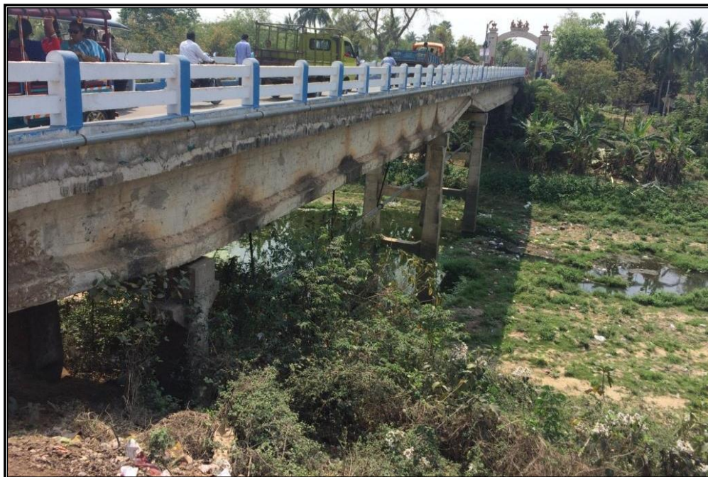
CHAINAGE 65.96 Km BRIDGE KANCHAN NAGAR
