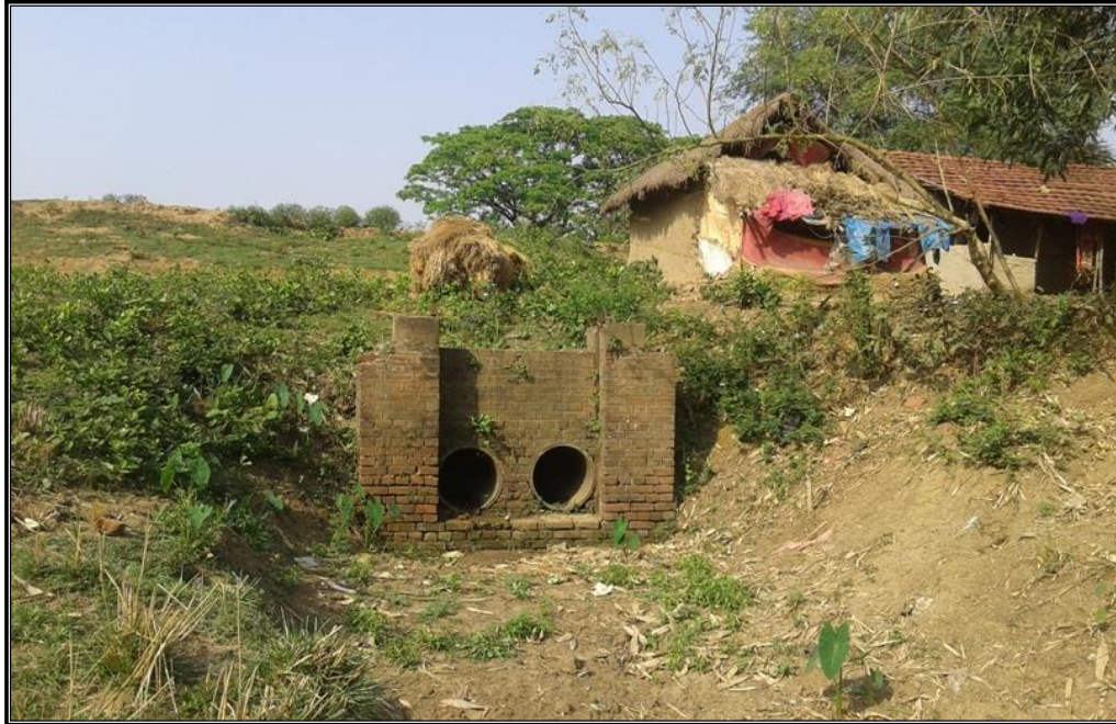
CHAINAGE 108.188 Km CULVERT MALLIKPUR
