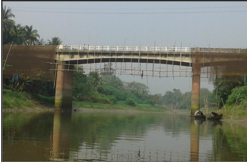
CHAINAGE 134.9 Km BRIDGE KUNTIGHAT
