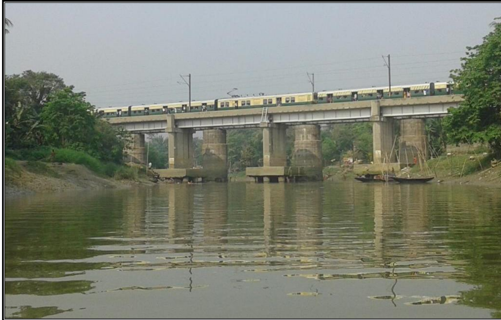
CHAINAGE 135.2 Km RAILWAY BRIDGE KUNTIGHAT
