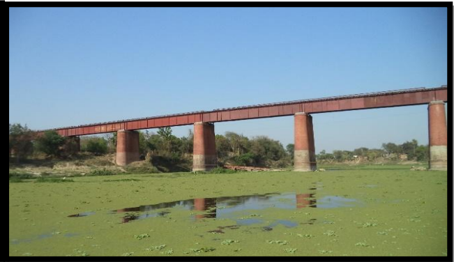
Chakpanchhaita Rail Bridge at Ch 95.69 km
