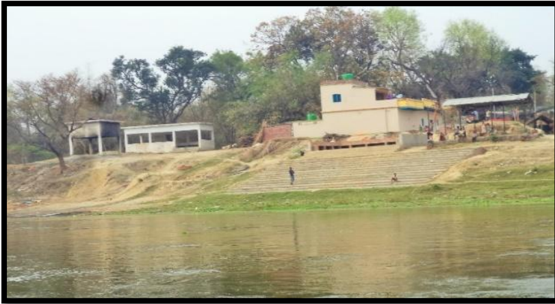
Ghat on River Bank at Ch 171.60 km
