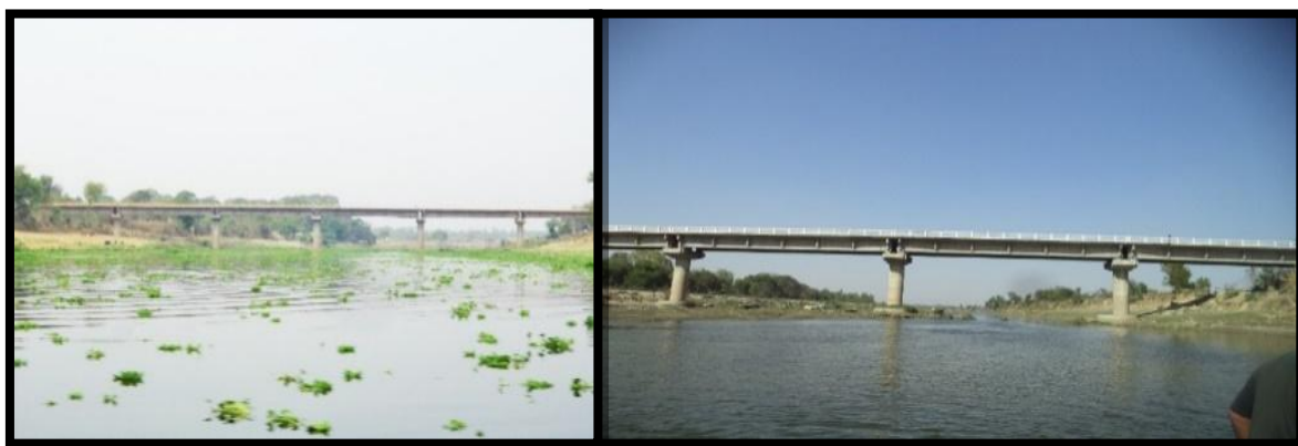
Semri Bridge at Ch 427.41 km Naipura Bridge at Ch 437.67 km
