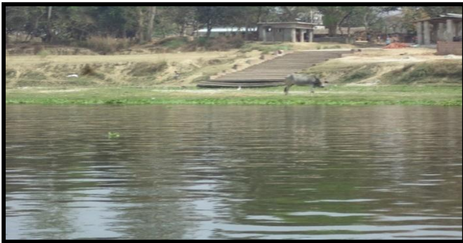
Ghat at Ch 274.59 km
