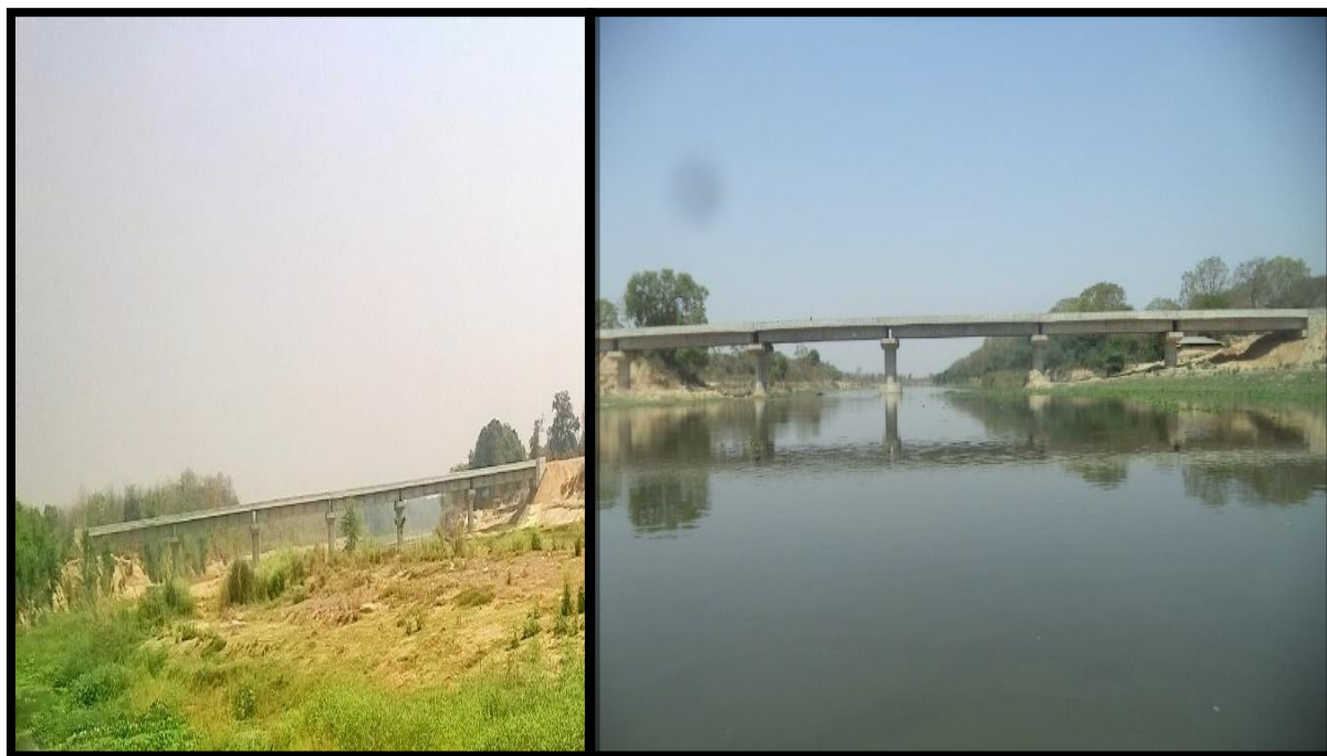
Sathin U/C Bridge at Ch 327.45 km
