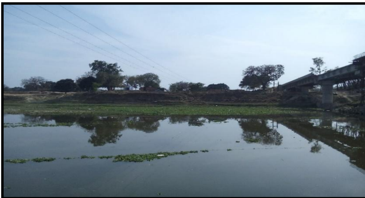
Electric Line at Ch 255.199km
