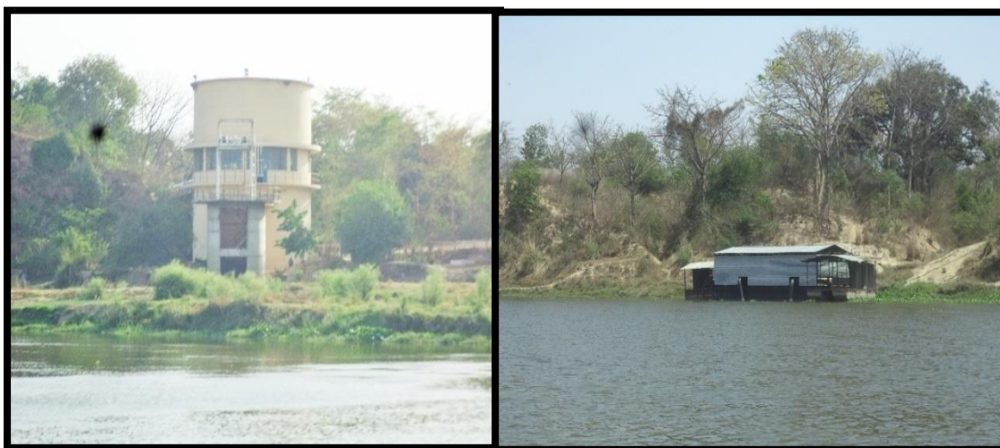
Water Tank at Ch 327.160 km & Water Pump at Ch 341.507 km
