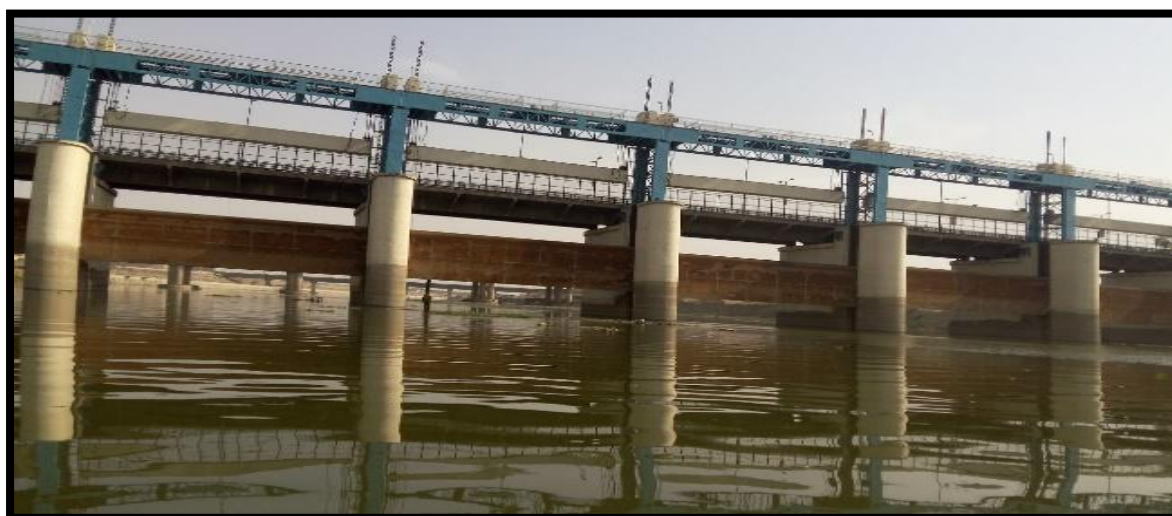
Gomti Barrage at Ch.507.870 km
