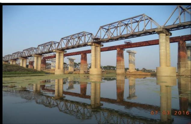
Rajwari Rail Bridge Ch. 3.73 km
