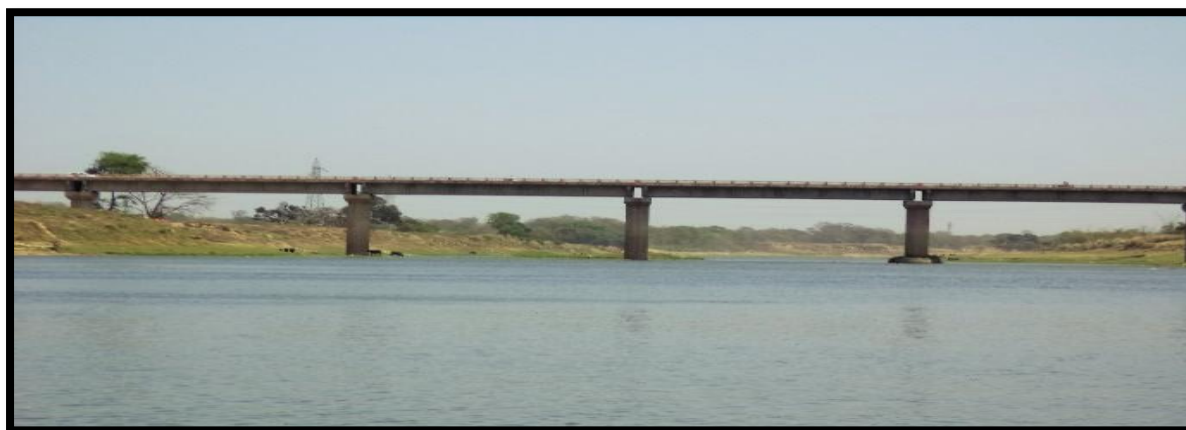
Saidpur Bridge at Ch 231.46 km
