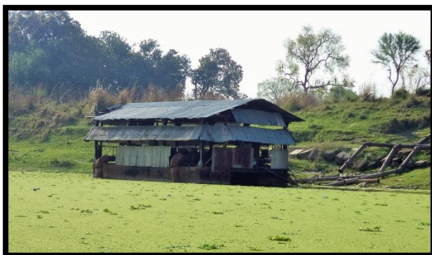
Irrigation Pump at Ch 29.67 km
