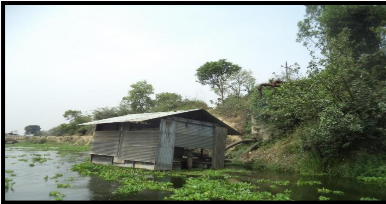
Water Pump at Ch 416.4 km
