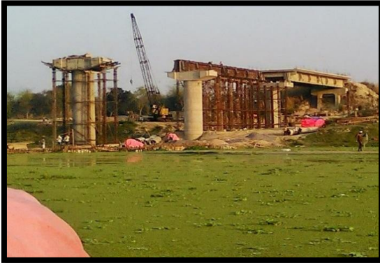
Jafrabad U/C Bridge at Ch 91.335 km
