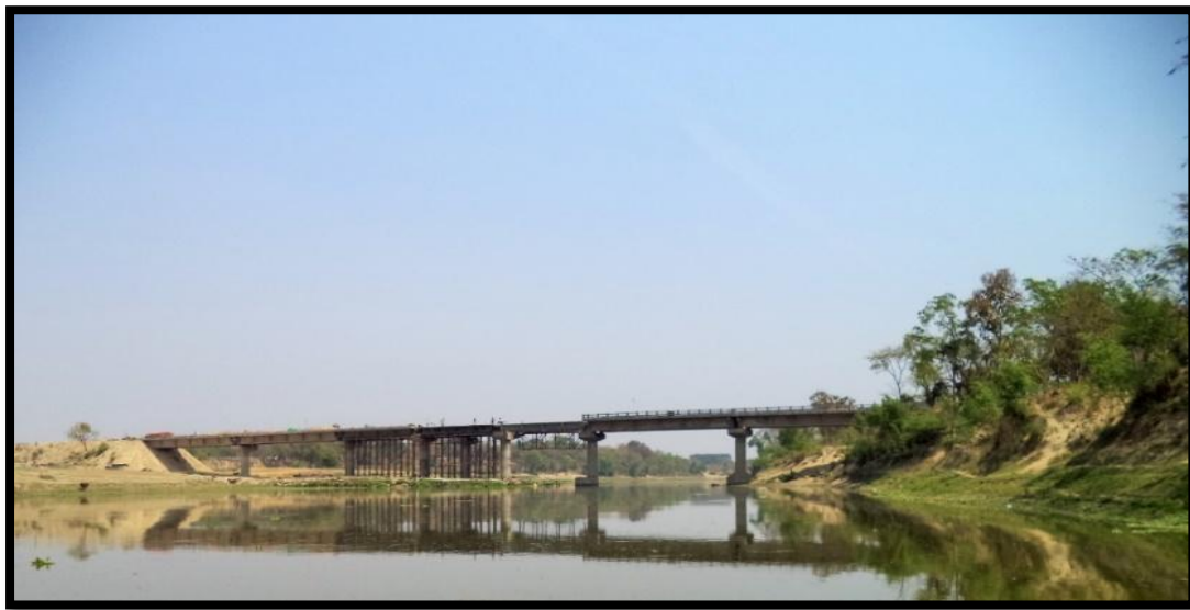
Papad Ghat Under Construction Bridge Ch 206.65 km
