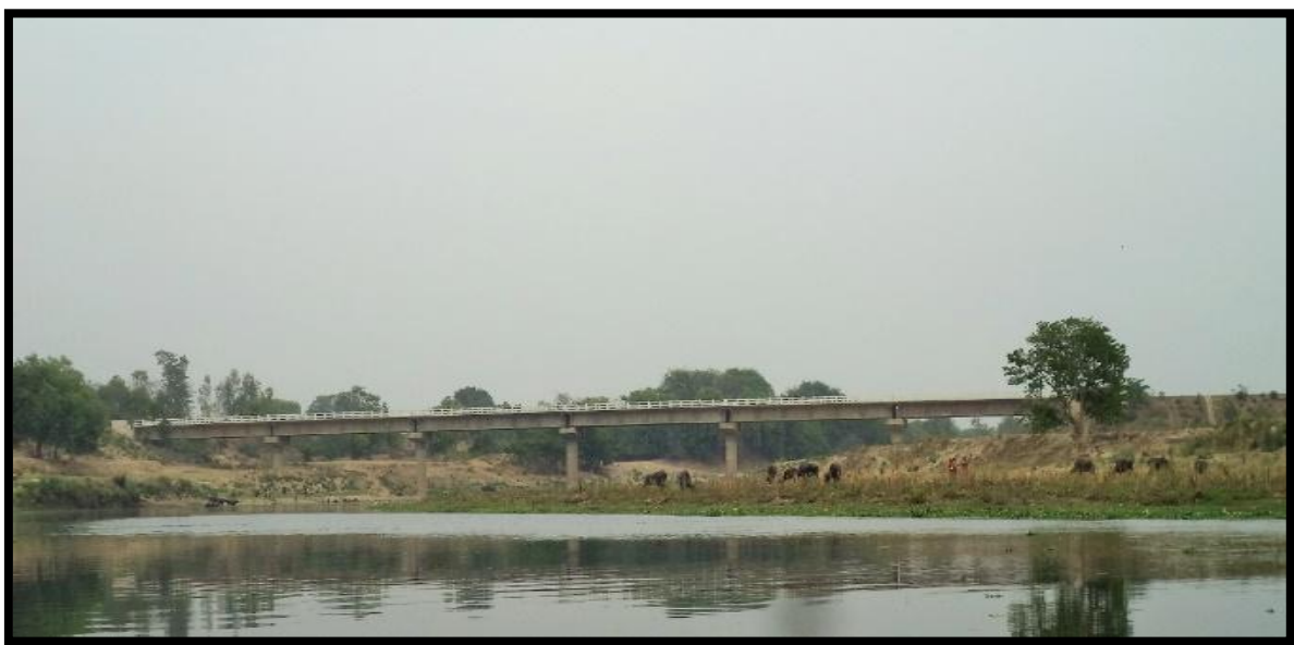
Fatehpur Bridge at Ch 471.97 km
