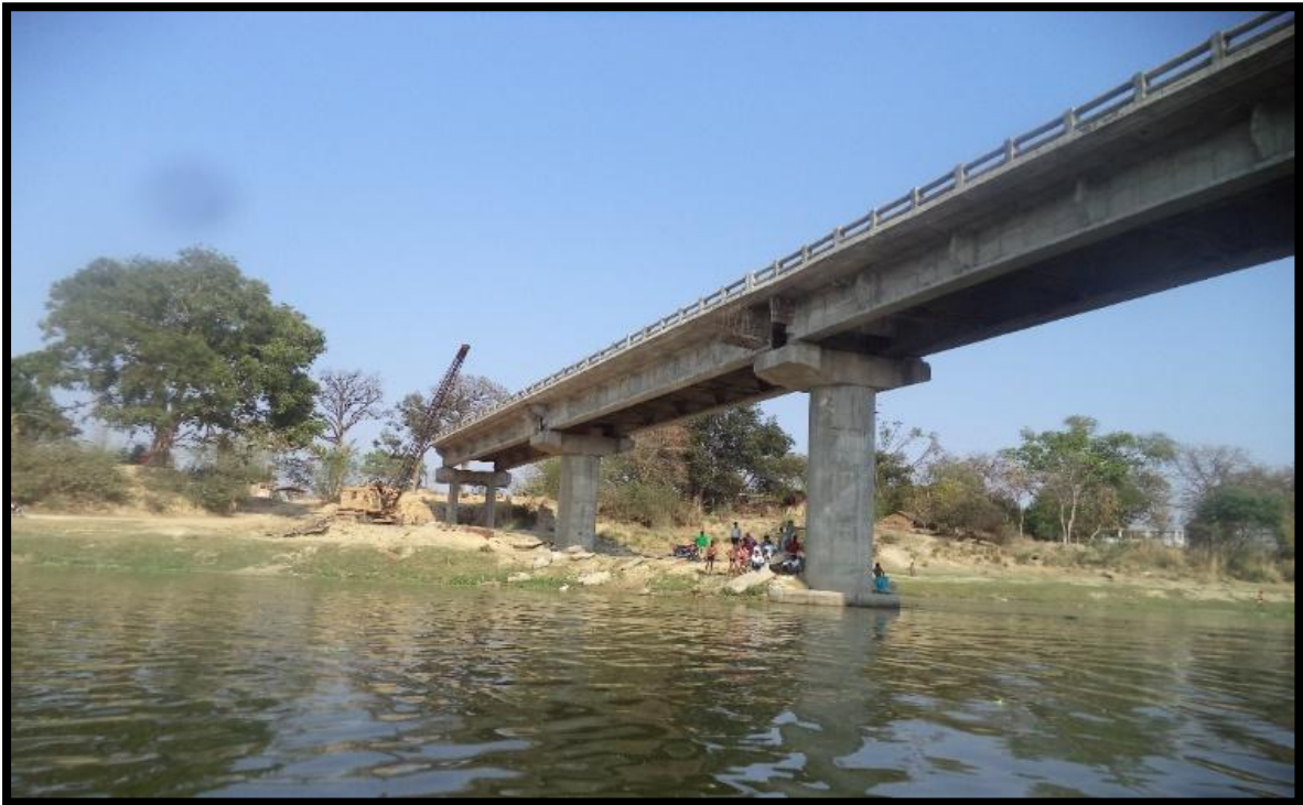
Imiliya U/C Bridge at Ch 148.35 km
