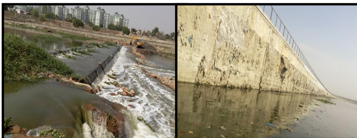
Anicuts at Ch 506.087 km
