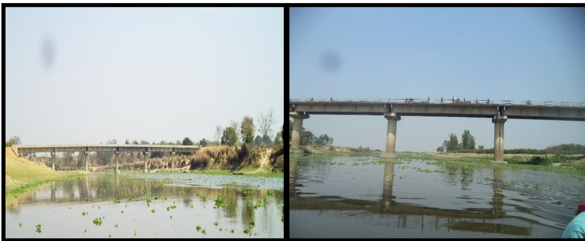
Mithnepur Bridge at Ch 284.32 km Isauli Bridge at Ch 293.94 km
