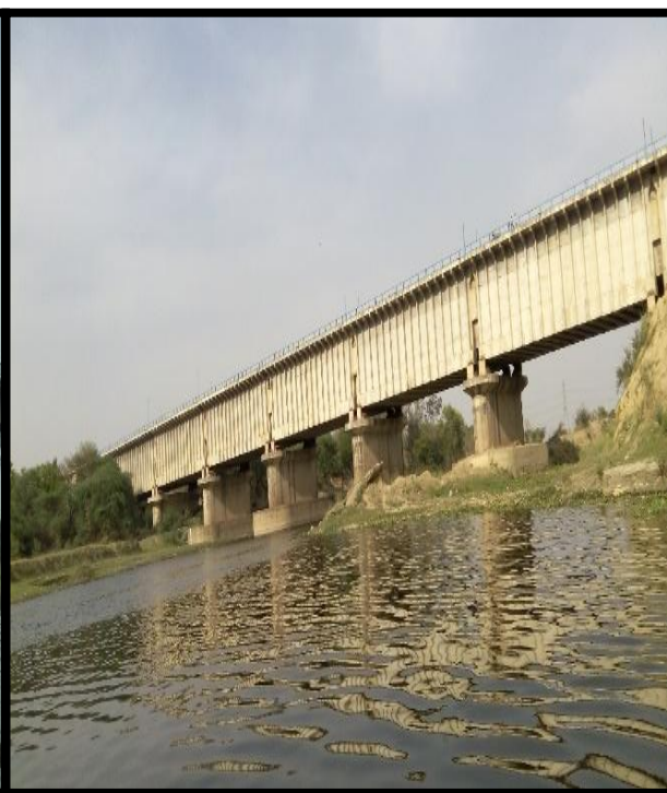
Indra Canal at Ch 491.160 km
