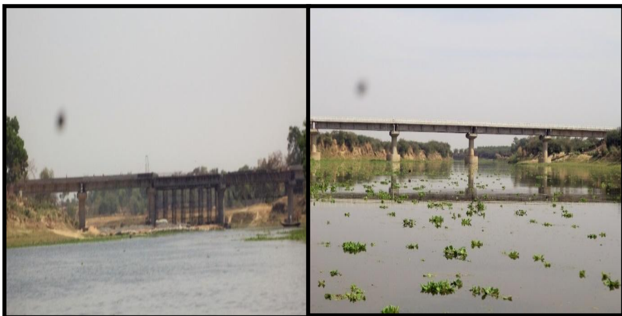
Kalkhura U/C Bridge at Ch 255.230 km
