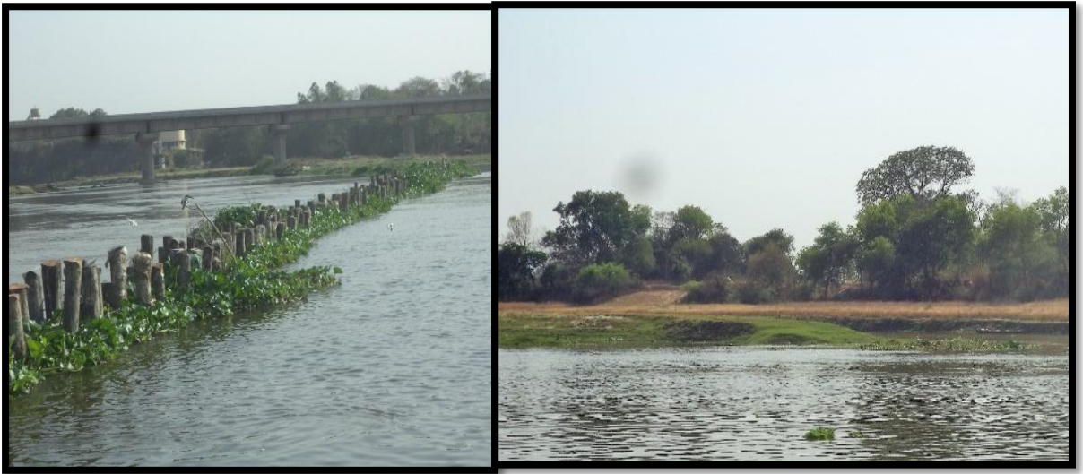
327.115 km to 327.542 km & Island at Ch 333.900 km
