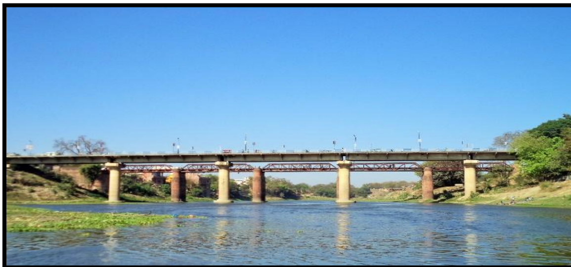
Sultanpur Bridge at Ch 239.08 km
