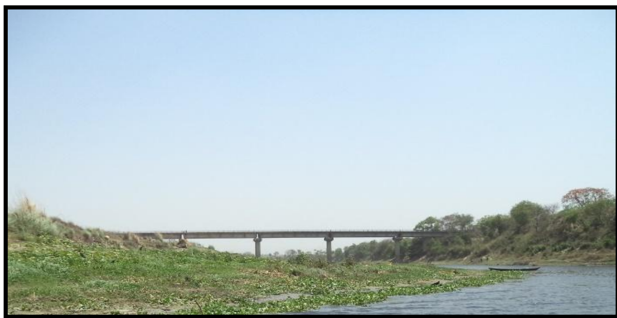
Ibraheembad Bridge at Ch 455.02 km
