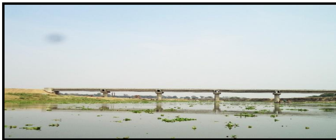
Thauri Bridge at Ch 314.266 km
