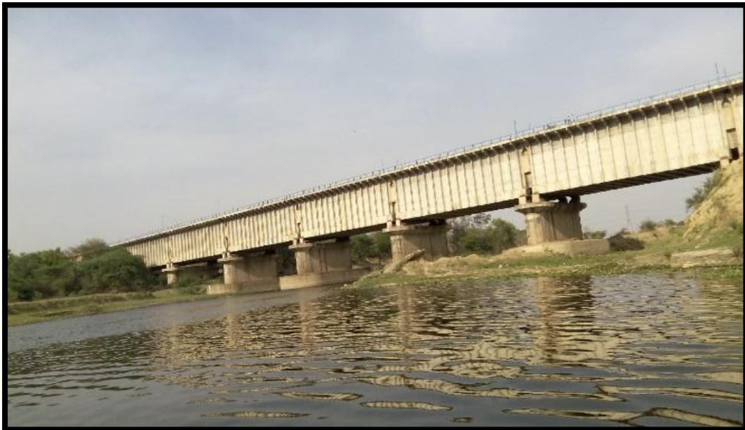
Indra Canal at Ch 491.160 km
