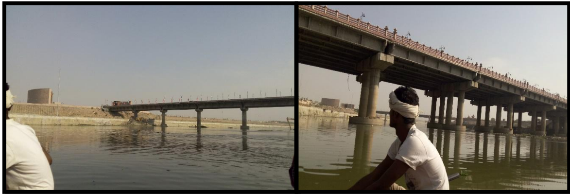
Lucknow Bypass Bridge at Ch 507.310 km
