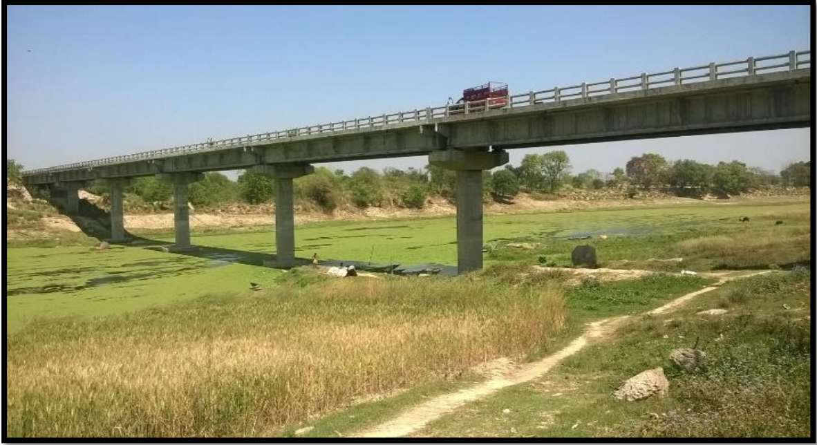
Pilkichha Bridge at Ch 139.23 km
