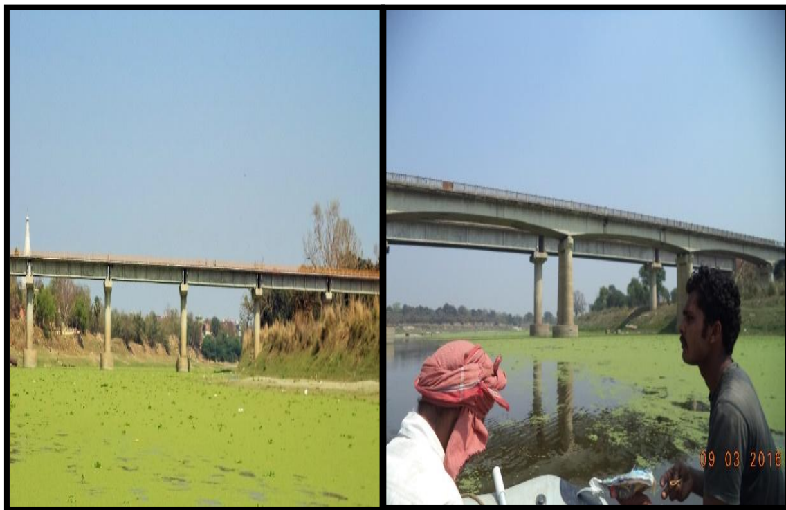
Banshakti Barrage at Ch. 29.08 km Balua Bridge at Ch. 39.03 & 39.05 km
