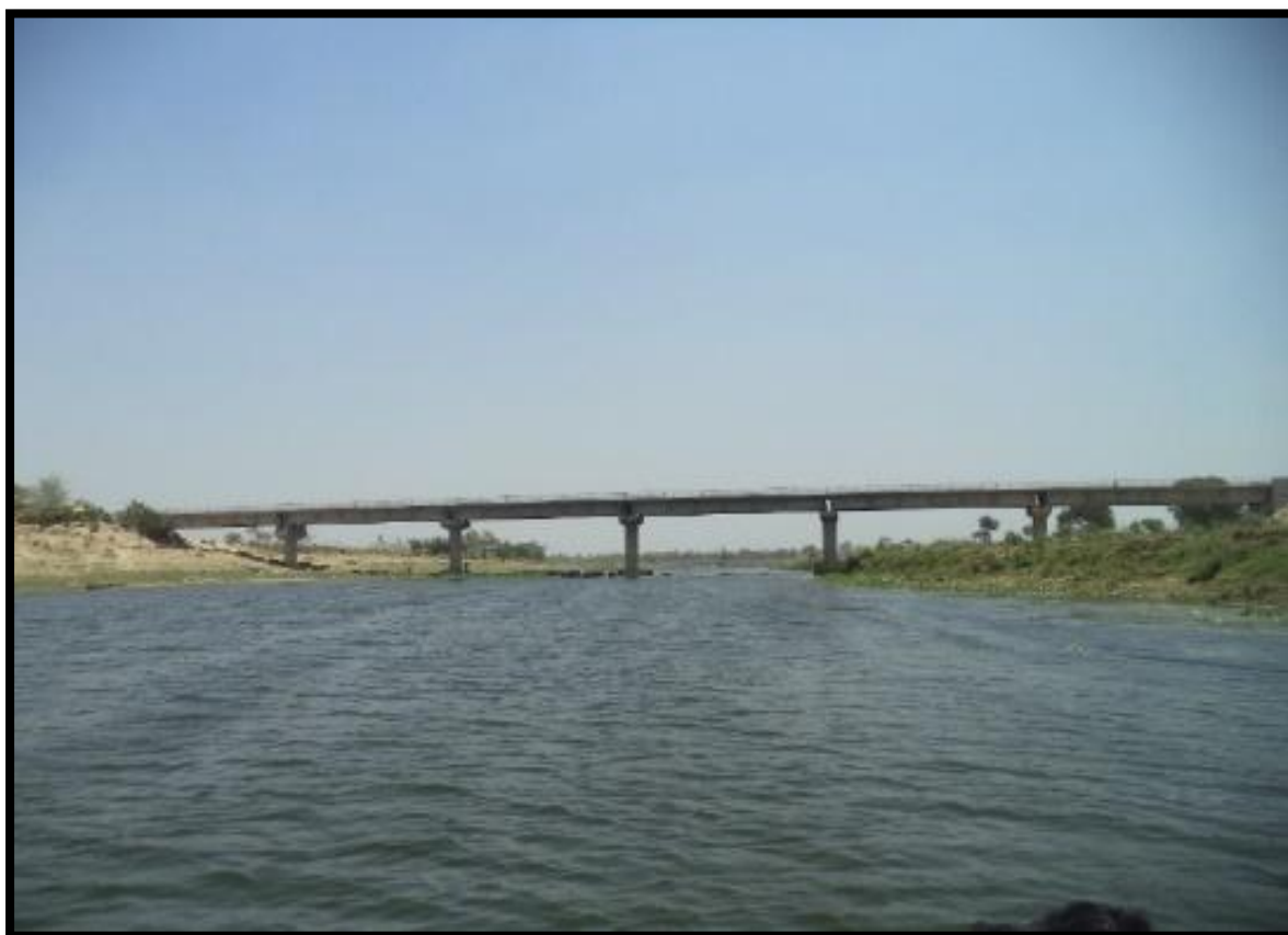
Dandupur Bridge at Ch 399.24 km
