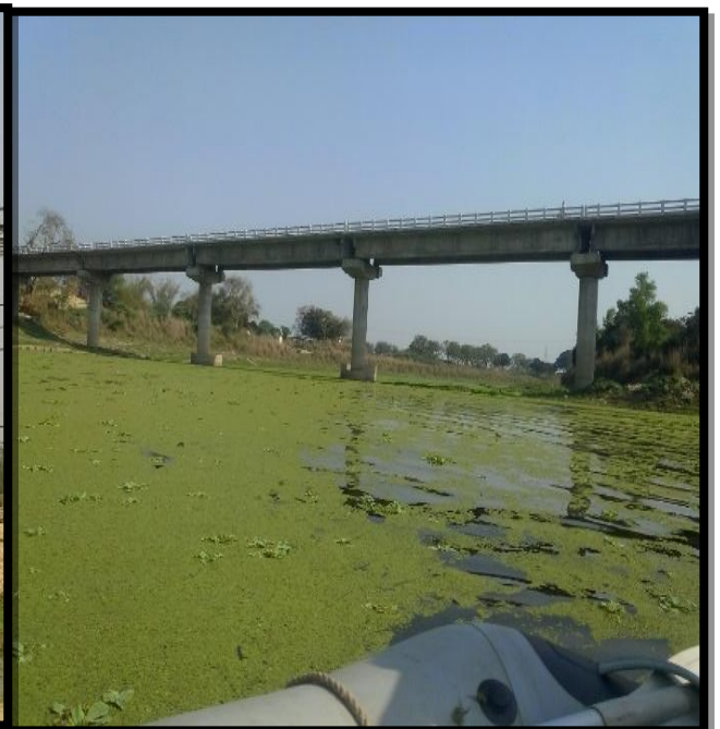
ECO Belao Bridge Ch 74.4 km
