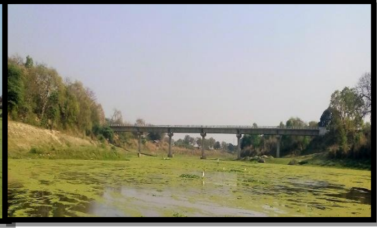
Jafrabad Bridge at Ch 85.36 km
