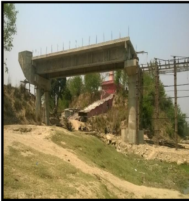
Pierce U/C Bridge at Ch 66.50 km
