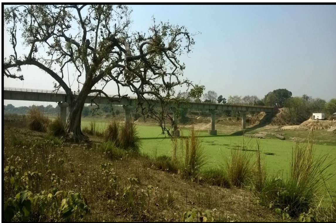
Chuncha Bridge Ch 109.83 km
