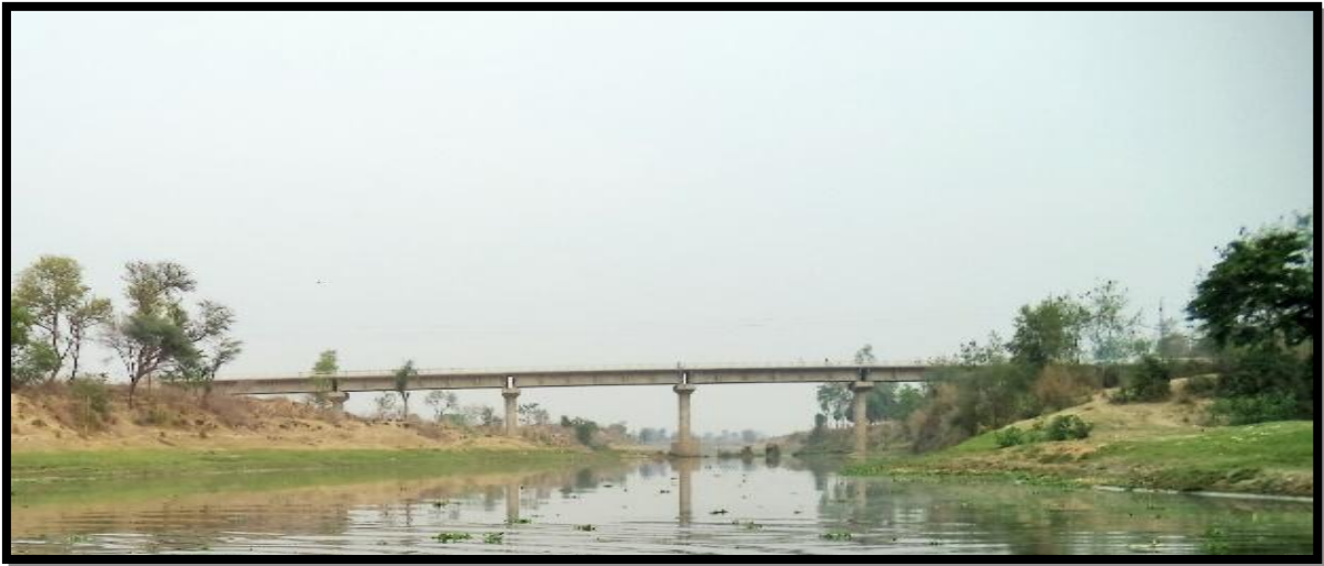
Chamartaliya Bridge at Ch 469.780 k
