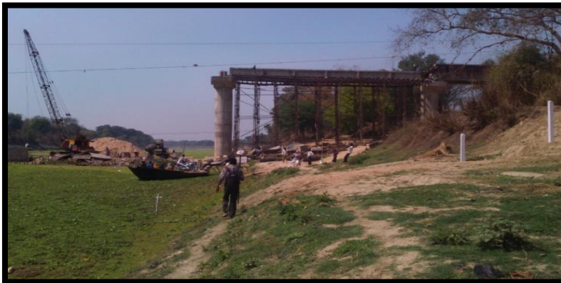
Pasewan Ferry Ghat at Ch 55.80 km
