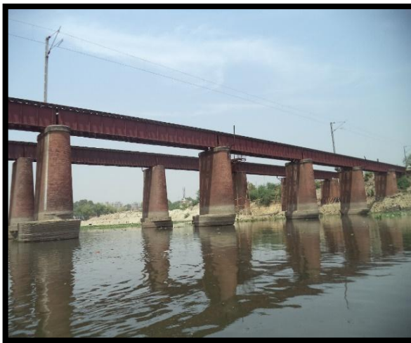
Dalgunj Rail Bridge at Ch 513.500 km
