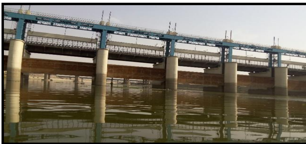
Gomti Barrage at Ch.507.87 Km
