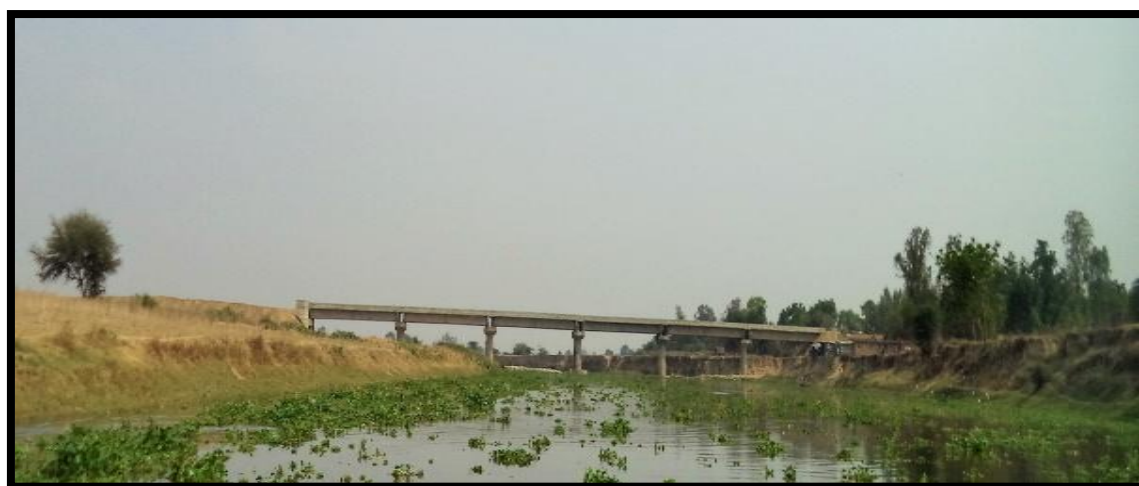
Gajarpur u/c Bridge at Ch 306.625 km
