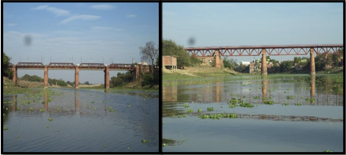
Sultanpur Old Bridge at Ch 239.11 km
