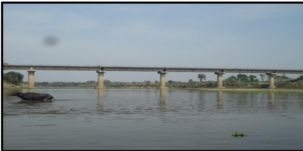
Brasin Bridge at Ch 239.11 km
