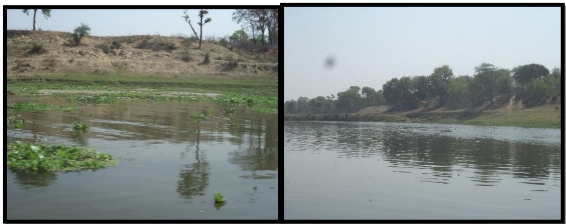
Shallow Depth at Ch 350.500 km
