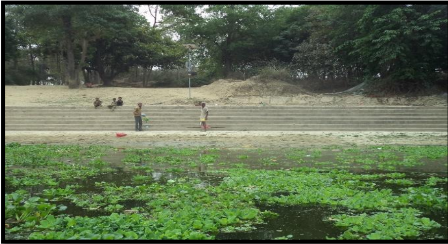
Stairs at Ch 418.06 km
