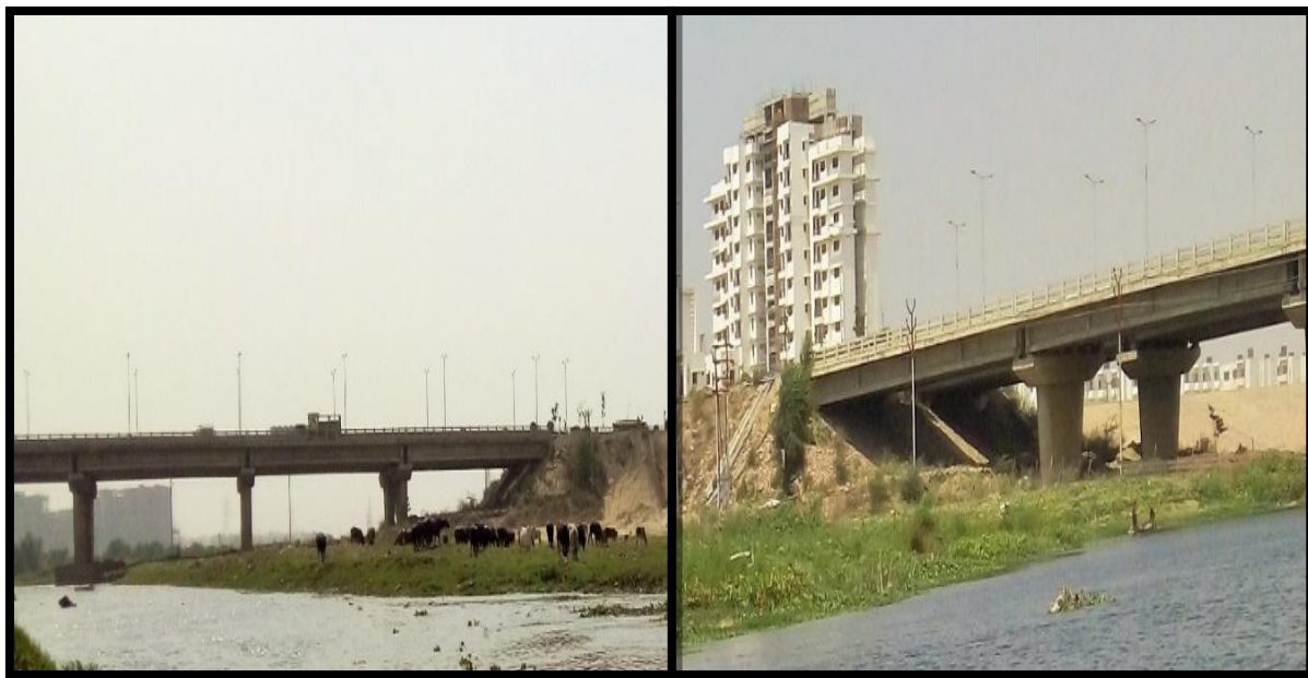
Ardonamau Bridge at Ch 499.00 km & Ch 499.020 km
