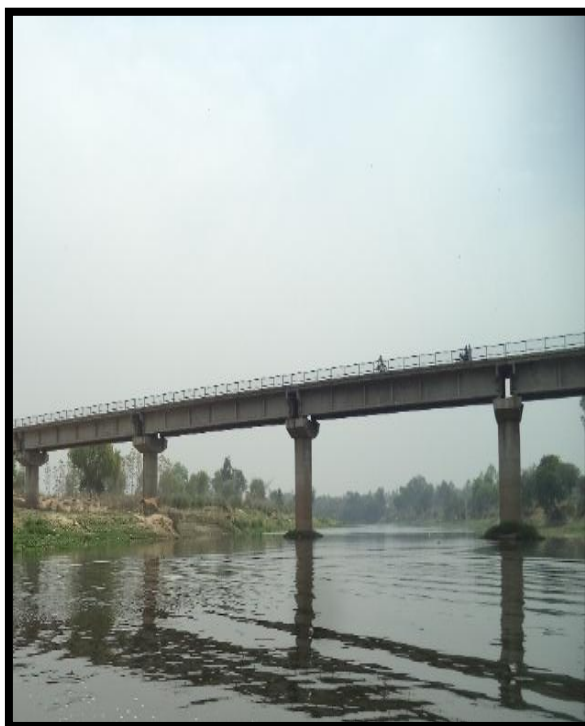
Nizampur Bridge at Ch 482.02 km
