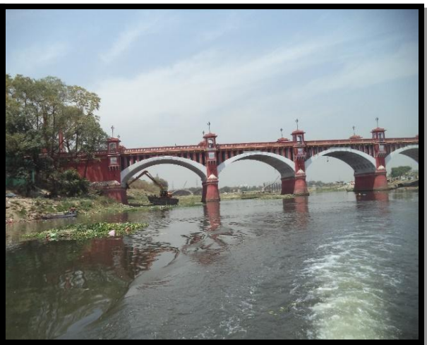
Loha Pool at Ch 514.240 km
