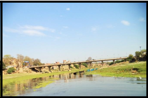
Lokbandhu Bridge at Ch 98.51 km
