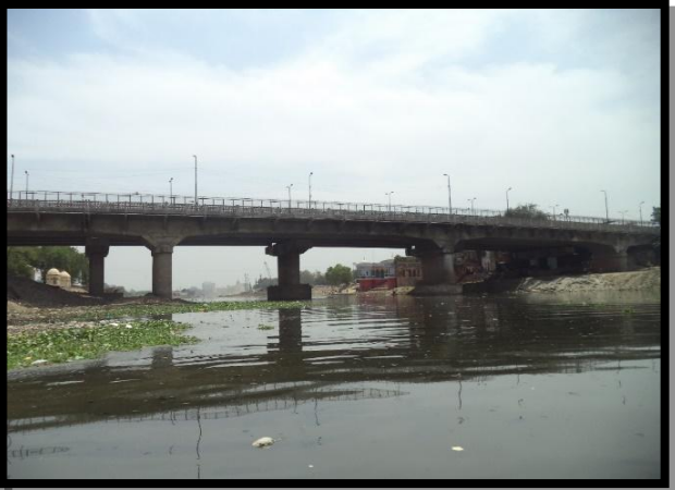
Acharya Nagendra Dev Bridge Ch 513.25 km
