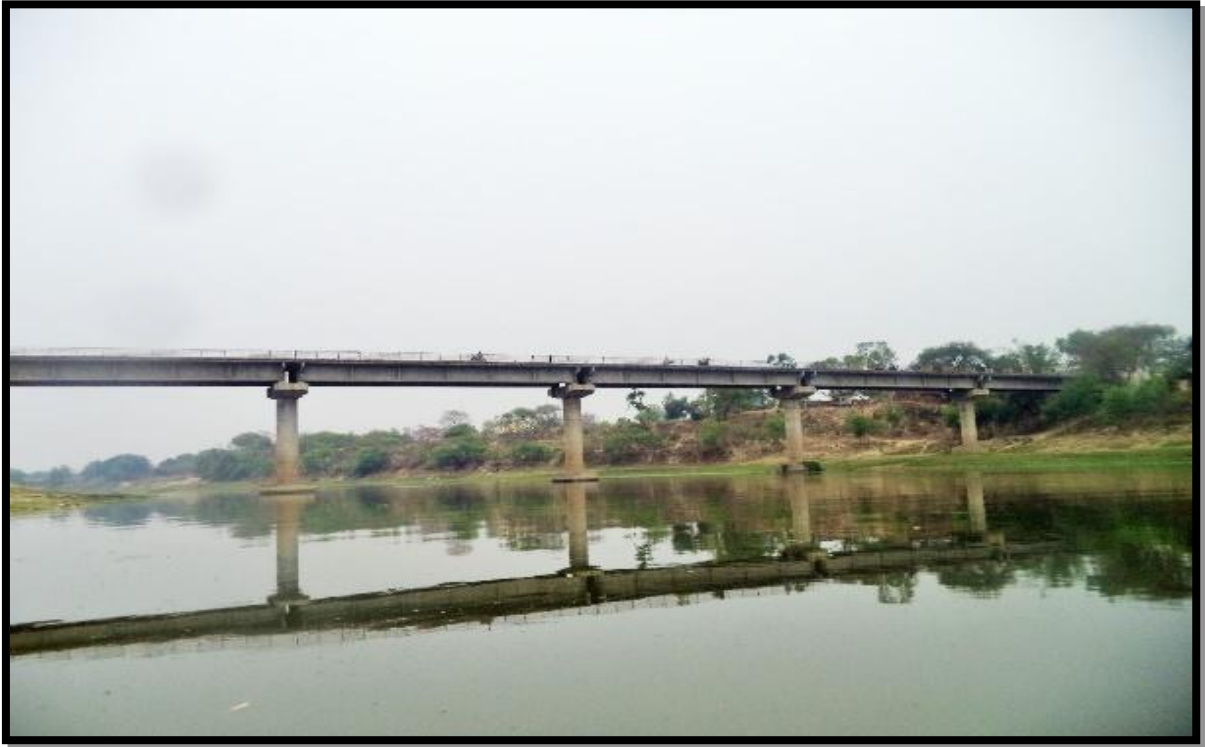
Tripathi Setu Bridge at Ch 158 km
