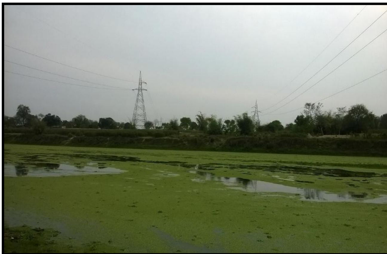
HT Lines at Ch 104.327 km & Ch 104.393 km
