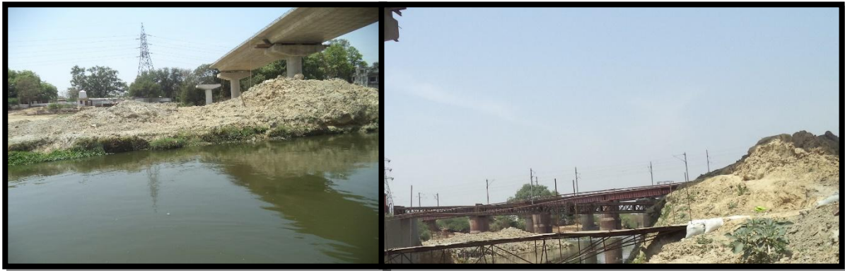
U/C Bridge at Ch 505.180 km
