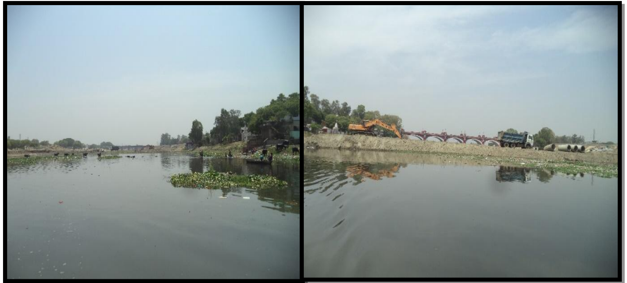
Shallow Depth at Ch 513.50 km to 514.00 km Sewage Line Construction at Ch 514.00
