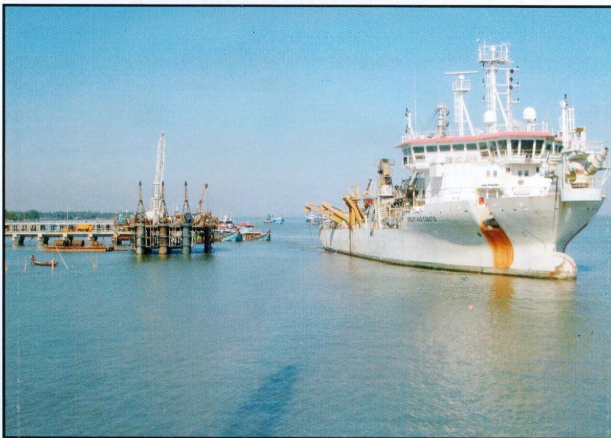
Dredging and Construction of IWT Jetty at Sittwe in progress
