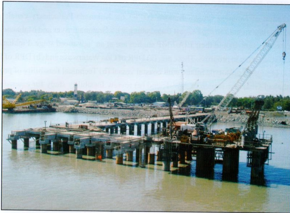
Construction of Port & backup facilities at Sittwe in progress
