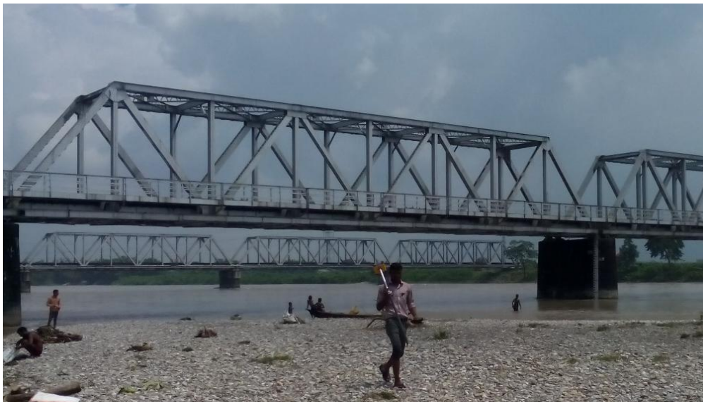
Figure 17 Pakriguri Rail Bridge (Chainage- 54.807km and 54.961 km)
