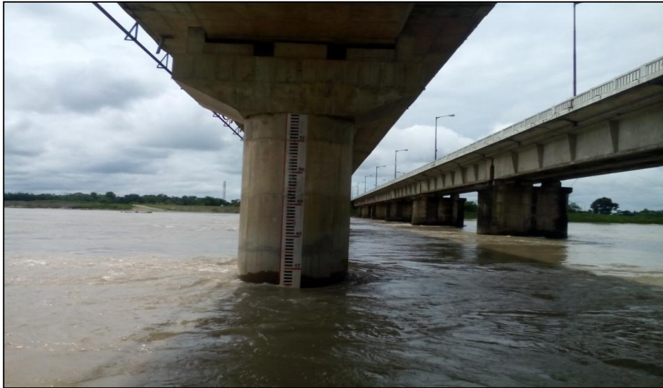
Figure 16 Pakriguri RCC Bridge (Chainage-56.660 km and 56.680 km)
