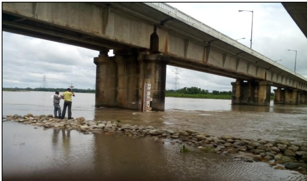
Figure 8 RCC Bridge (Chainage-16.701 km)
