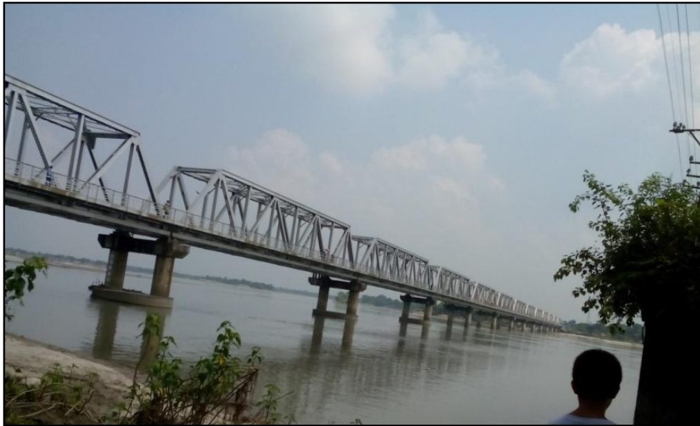
Figure 7 Rail Bridge (Chainage- 11.894 km)
