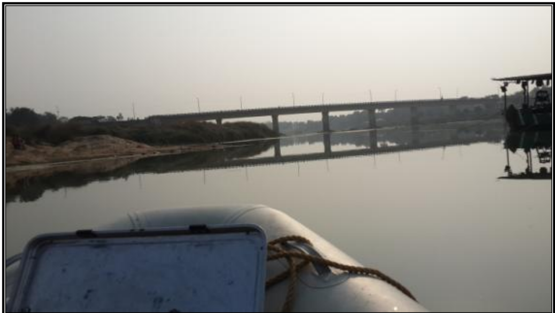
MAJOR RAILWAY BRIDGE CHAINAGE AT 55.0 KM
