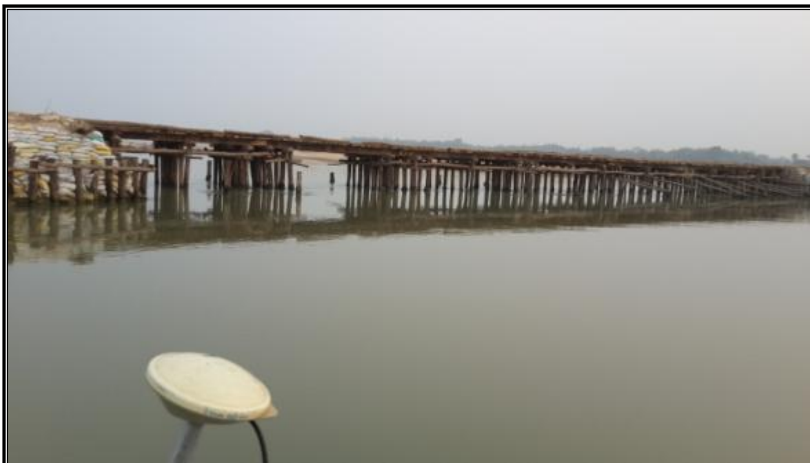
MANIK HATI WOODEN BRIDGE CHAINAGE AT 124.0 KM
