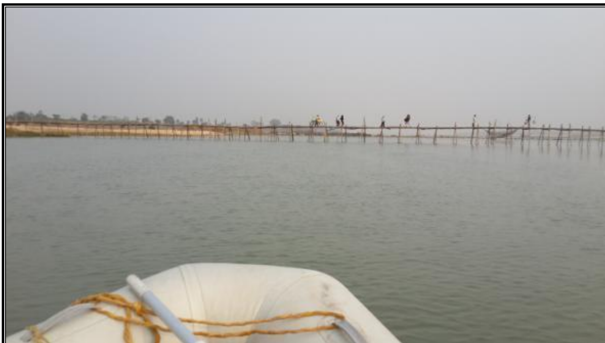
BAMBOO BRIDGE CHAINAGE AT 96.0 KM
