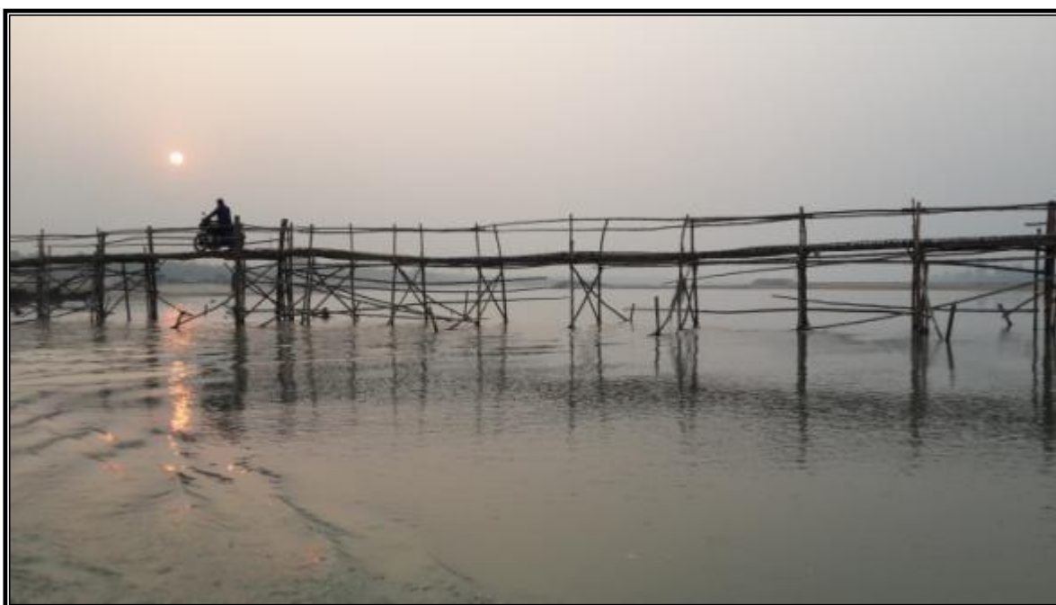
BAMBOO BRIDGE CHAINAGE AT 58.0 KM
