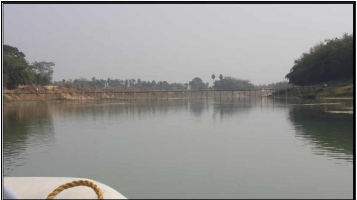
KANSONA BAMBOO BRIDGE CHAINAGE AT 46.0 KM
