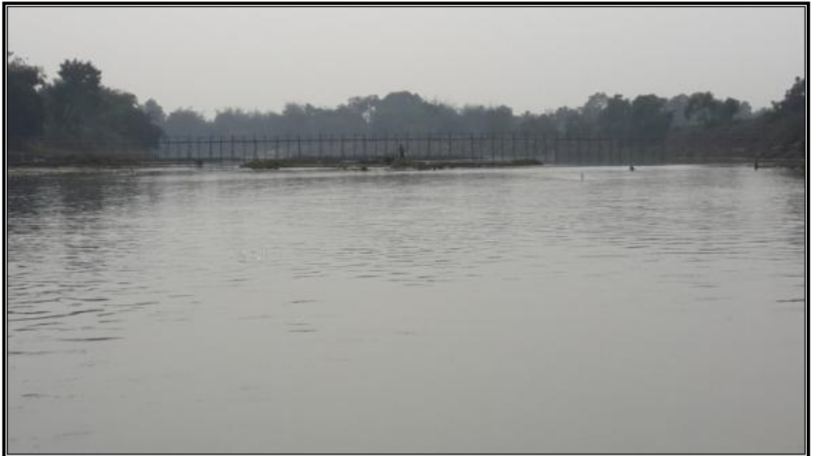
BEGUA BAMBOO BRIDGE CHAINAGE AT 44.0 KM
