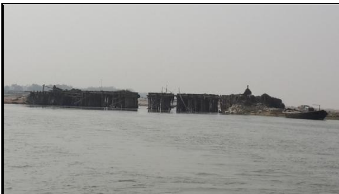
BONOGRAM BAMBOO BRIDGE CHAINAGE AT 88.0 KM
