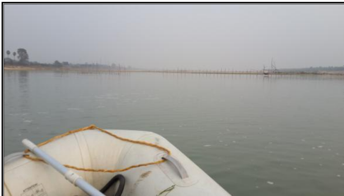
KUMRUL BAMBOO BRIDGE CHAINAGE AT 84.0 KM
