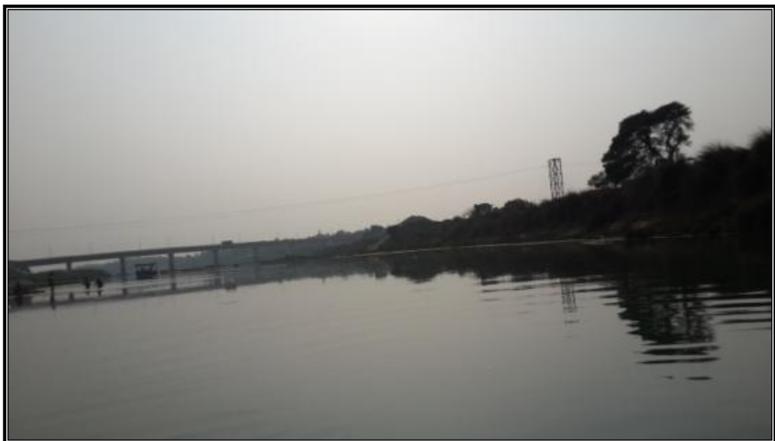
GOURANGACHAK MAJOR BRIDGE & HIGH TENSION LINE CHAINAGE AT 52.0 KM
