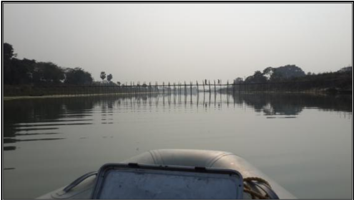
KUMARCHAK BAMBOO BRIDGE CHAINAGE AT 47.0 KM
