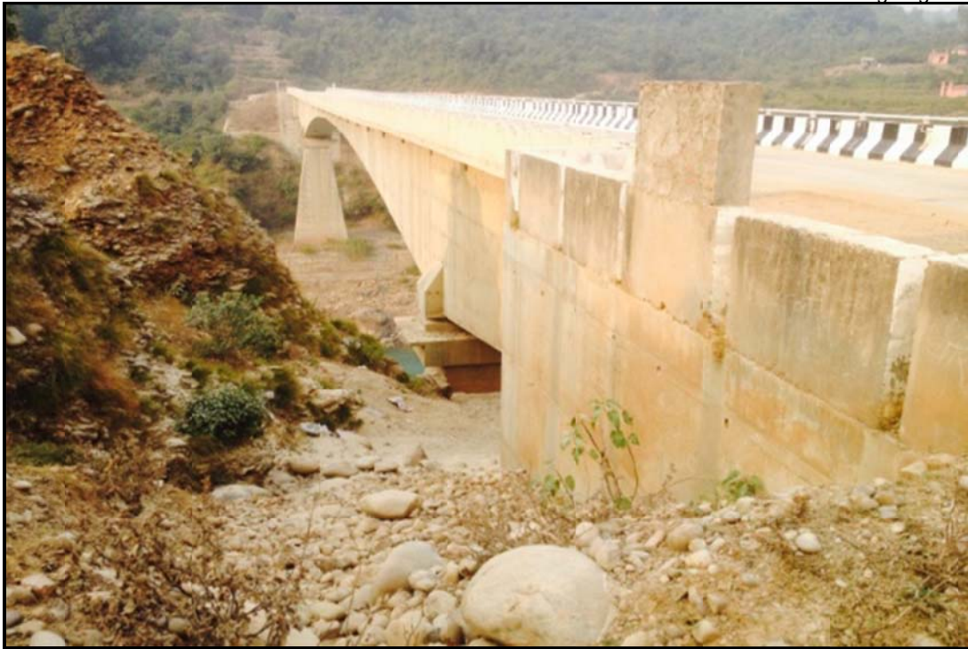
Figure 12 – Ch.16.00 Km Village Road Bridge Crossing River
