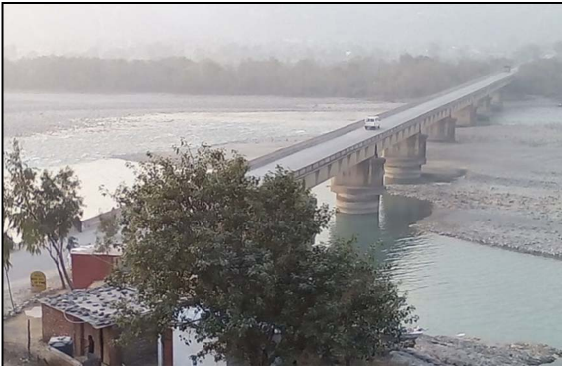
Figure 23 – Ch.-34.22 Km Bridge on Chenab River in Reasi District
