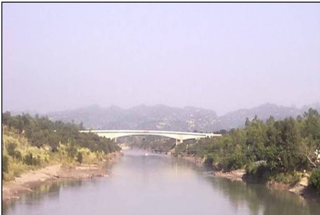
Figure 9 – Ch.4.165 Km Akhnoor by Pass Bridge
