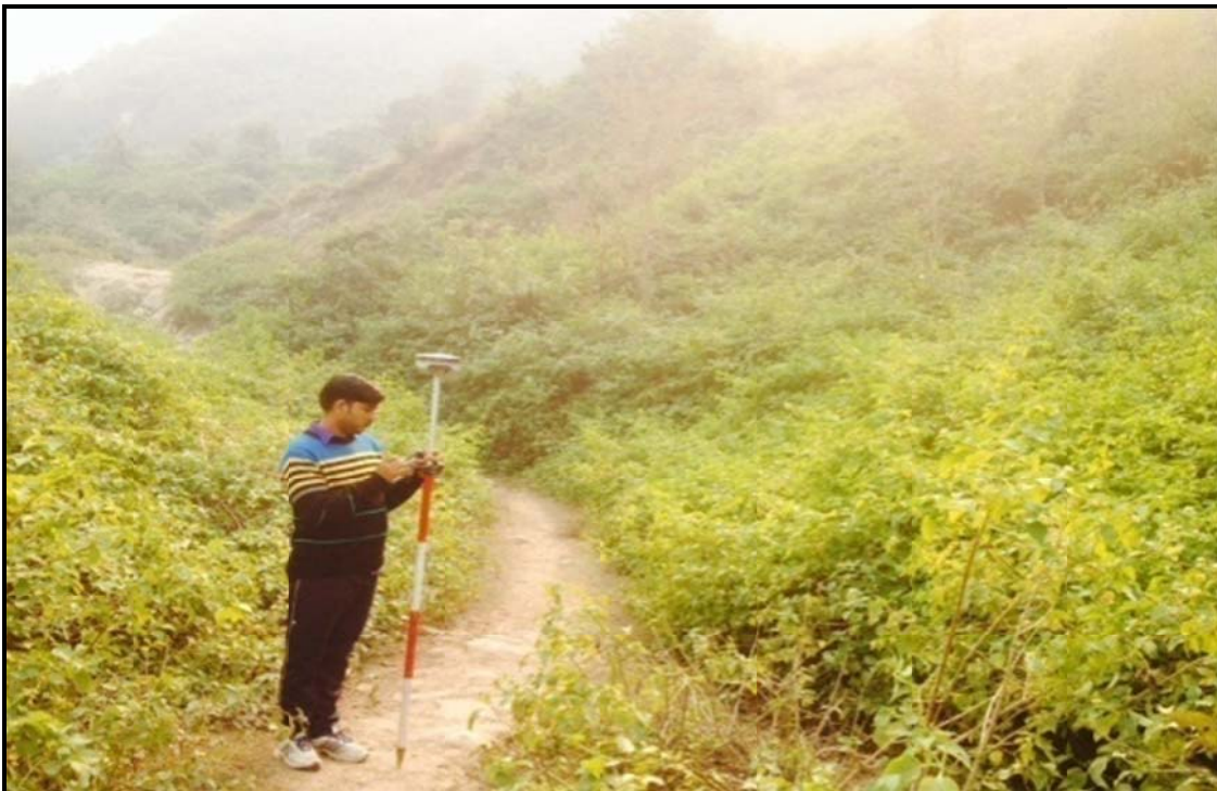
Figure 17 – Ch.-24.00 Km Topographic Survey on Progress
