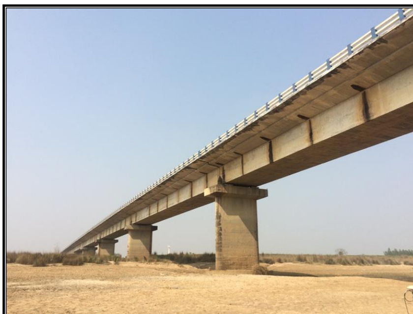
NOTUNHAT MAJOR ROADWAYS BRIDGE CHAINAGE 48.90
