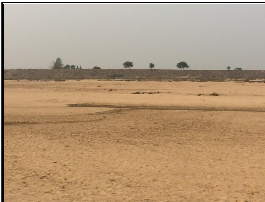
JASHRA EMBANKMENT WALL CHAINAGE 32KP
