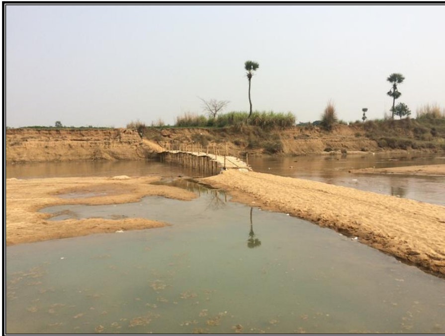
JAHANABAD WOODEN BRIDGE CHAINAGE 38
