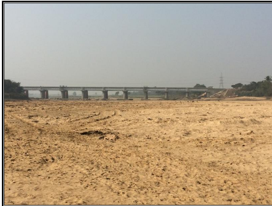
CHARKHI MAJOR ROADWAYS BRIDGE CHAINAGE 75.5
