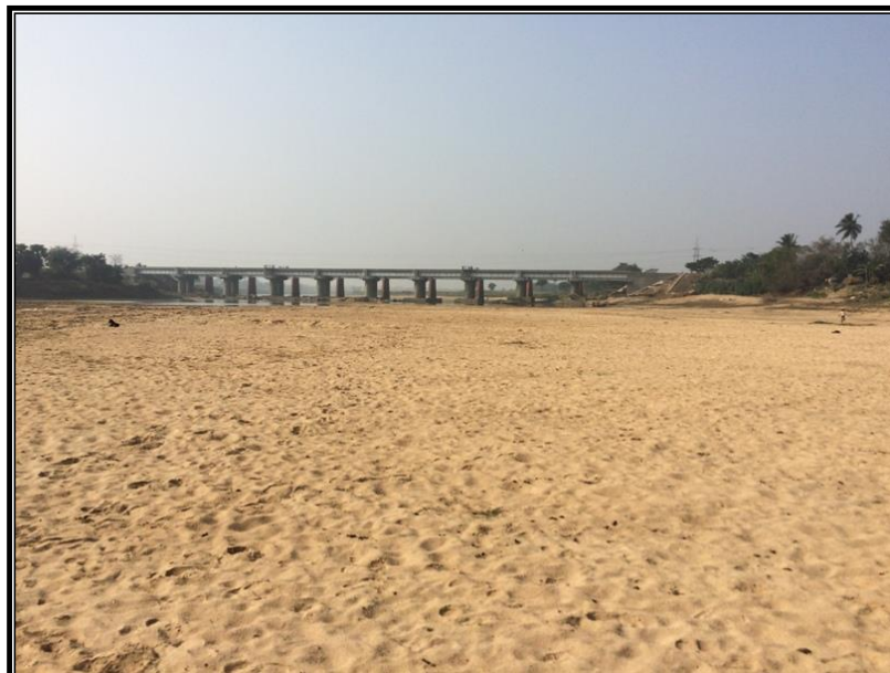
RAILWAY BRIDGE 83KP (2)
