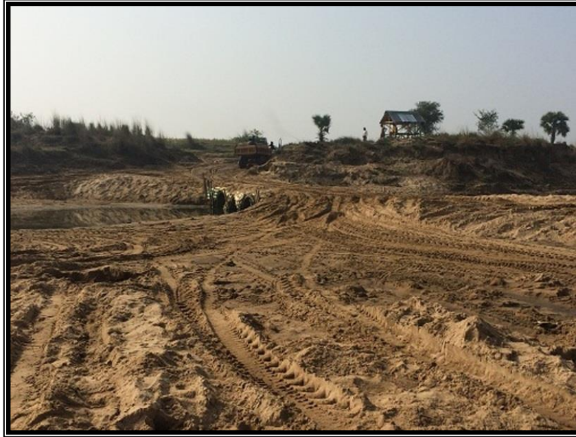
SAND MINING CHAINAGE 84KP
