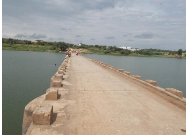
Figure 192 - Jayakwadi Road Bridge (ch968.095km)
