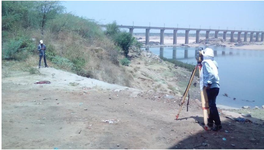
Figure 15 - Bhadrachalam Road Bridge -NH-30 (ch.0.00km)
