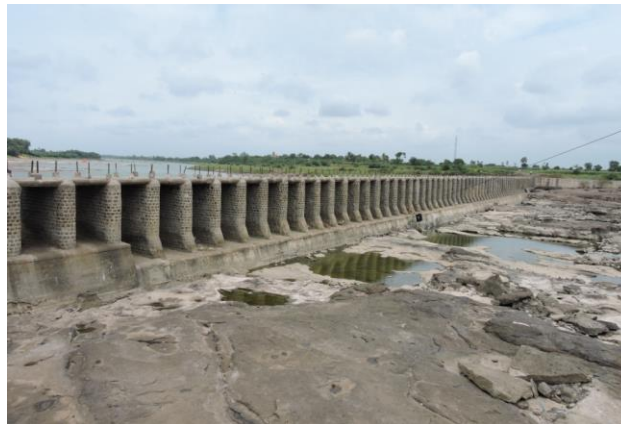
Figure 229 - Check Dam near Mahegaon Deshmukh village (ch. 1115.338km)
