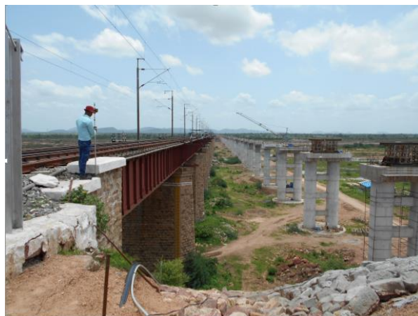
Figure 53 - Manchiryal Railway Bridge (ch.301.231km)
