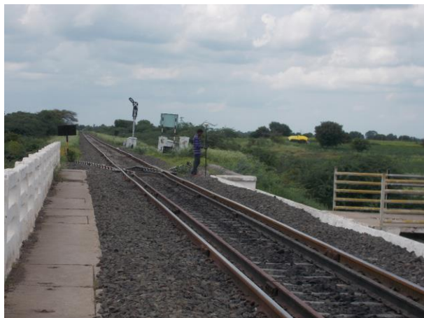
Figure 134 - Gangakhed Railway Bridge (ch.715.107km)
