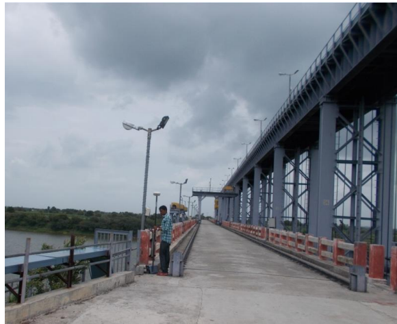
Figure 129 - Digras Barrage (ch. 671.142km)
