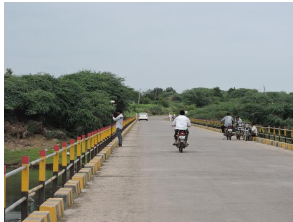
Figure 226 - Kumbhari Road Bridge (ch. 1111.293km)
