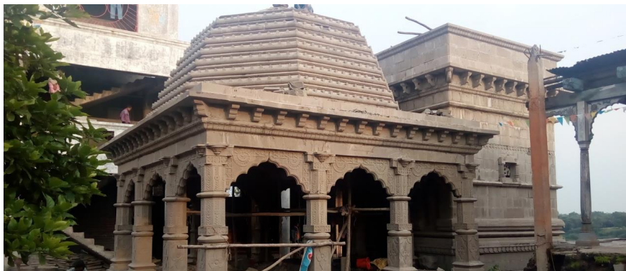
Figure 181 - Sant Dyneshwar Mauli Jalambhumi (ch. 946.736km)
