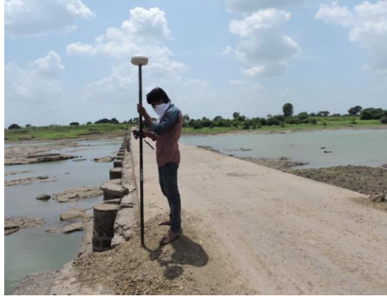
Figure 205 - Check Dam near Domegram village (ch. 1041.42km)
