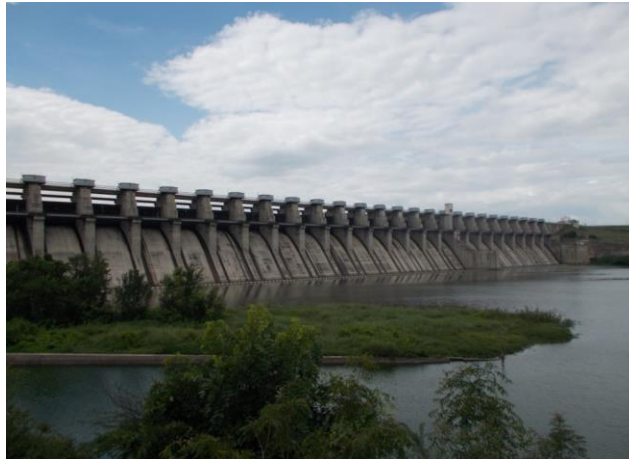
Figure 193 - Jayakwadi Dam (ch. 968.499km)
