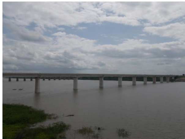
Figure 87 - Basra Railway line Bridge (ch.515.833km)
