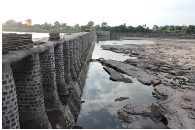
Figure 213 - Check Dam near Naur village (ch. 1064.729km)
