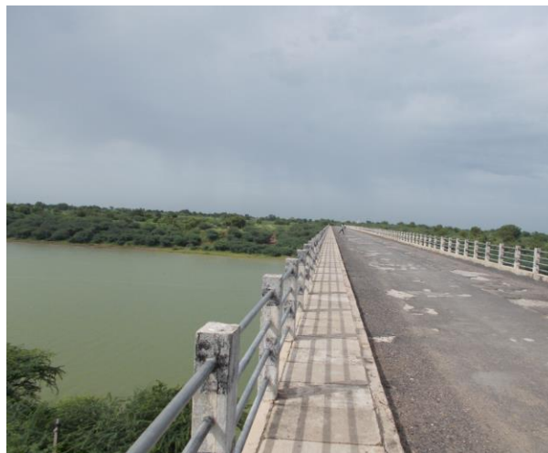
Figure 124 - Penur Road Bridge (ch. 647.194km)
