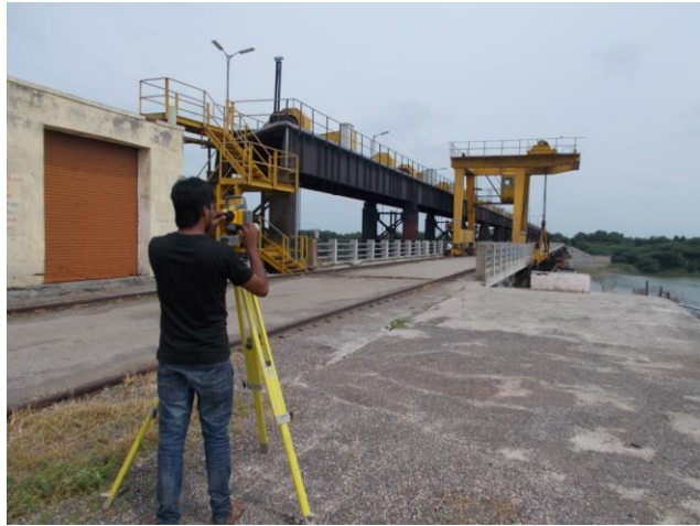
Figure 169 - Mangrul High-Level Barrage (ch. 873.218km)
