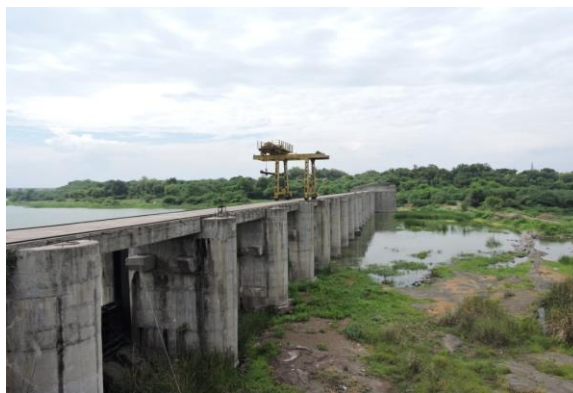
Figure 189 - Chanakwadi Barrage (ch. 964.641km)
