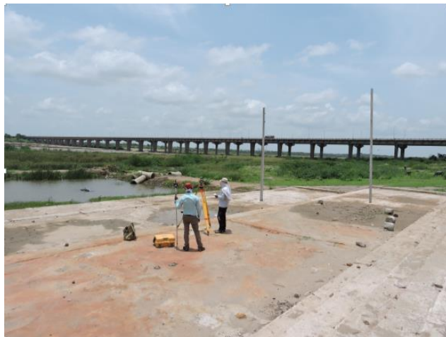
Figure 49 - Mancherial Road Bridge (ch.290.04km)
