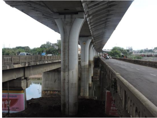
Figure 256 - Mumbai-Agra Highway Bridge and Fly over (ch. 1201.622km)
