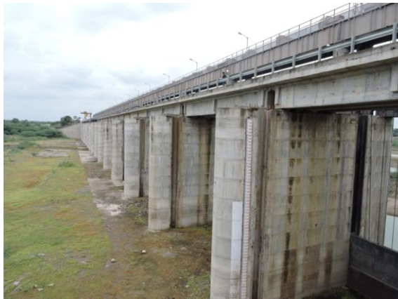
Figure 183 - Apegaon High-level Barrage (ch. 947.174km)
