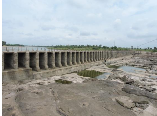
Figure 225 - Check Dam near Hingani village (ch. 1107.705km)
