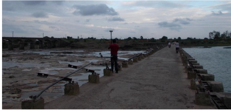
Figure 215 - Check Dam near Naur village (Puntamba Kolhapur Type Bandhara) (ch. 1077.218km)
