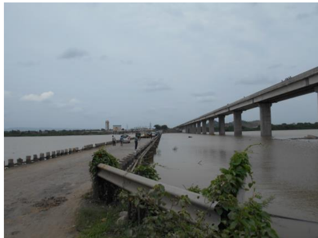
Figure 57 - Rayapatnam Road Bridge (Old – ch.338.333km & New – ch.338.389km)
