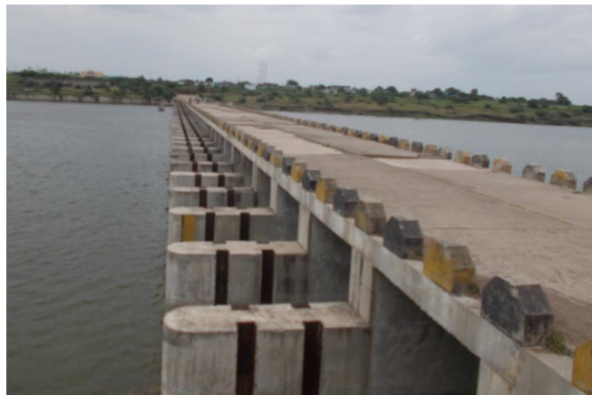
Figure 110 - Eidgah-Wajegaon Road Bridge (ch. 611.544 km)
