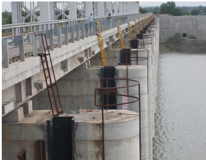
Figure 100 - Baligon Barrage (ch. 568.339km)
