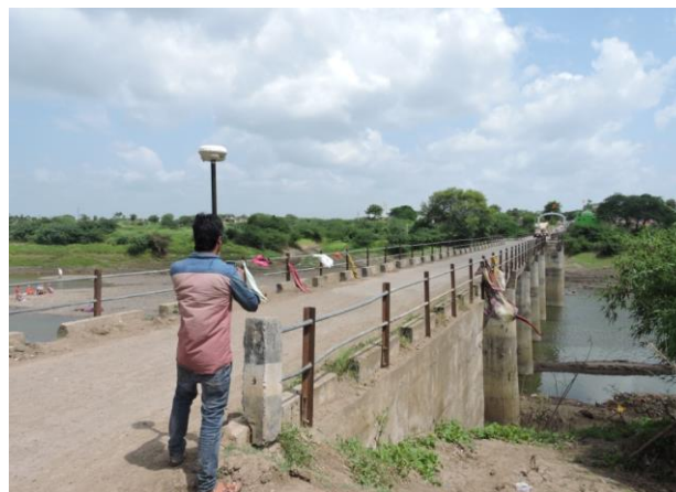
Figure 210 - Wanjargaon Road Bridge (ch. 1059.5km)
