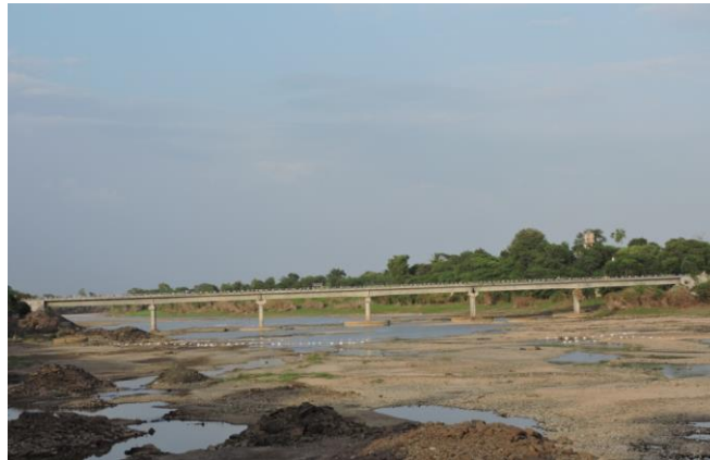
Figure 212 - Naur Road Bridge (ch. 1064.338km)
