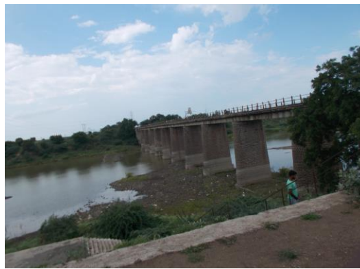
Figure 140 - Parbhani-Gangakhed State Highway Road Bridge (ch.723.031km)
