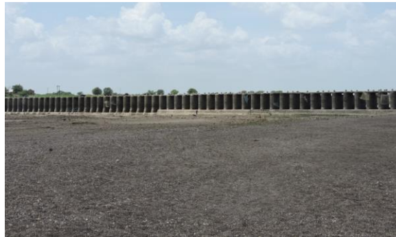
Figure 206 - Check Dam near Humrapur village (ch.1046.832km)
