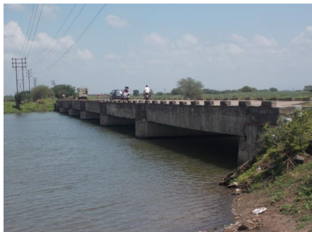
Figure 241 - Karanjgaon Road Bridge (ch. 1157.081km)
