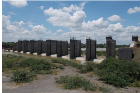
Figure 154 - Tarugavan High-Level Barrage (ch. 782.892km)
