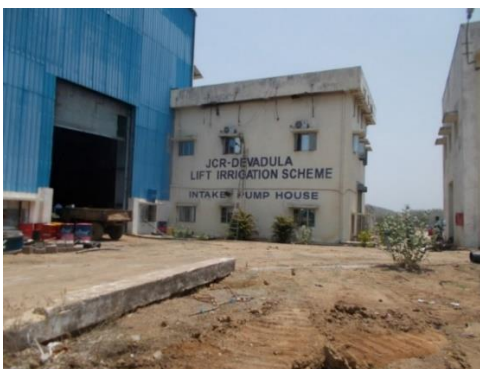
Figure 34 - JCR- Devadula Lift Irrigation Scheme (ch.148.29km)
