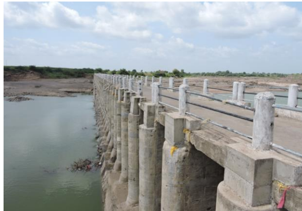
Figure 209 - Check Dam near Bhalgaon (ch.1059.332km)
