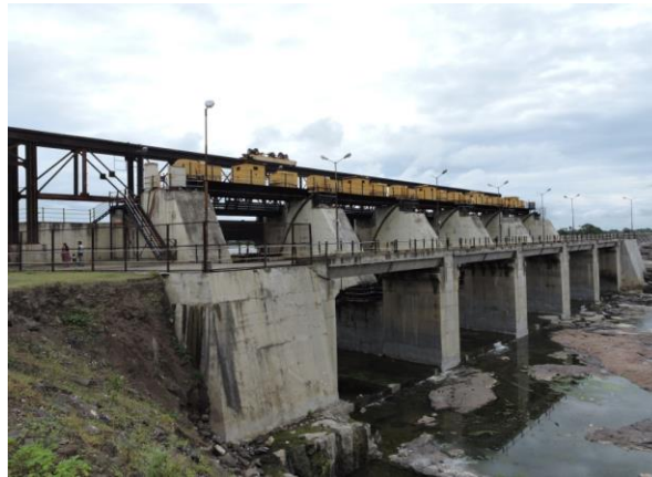
Figure 240 - Nandhur Madhyameshwar Dam (ch. 1149.288km)
