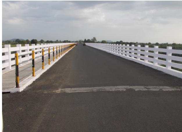
Figure 109 - Parbhani Nanded Bypass Road-(NH-204 (ch.610.448km)
