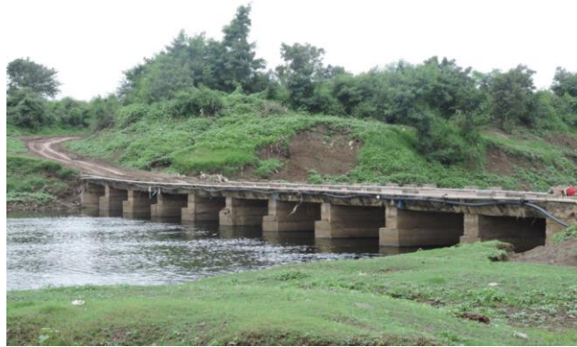
Figure 246 - Darnasangvi Road Bridge (ch. 1180.638km)
