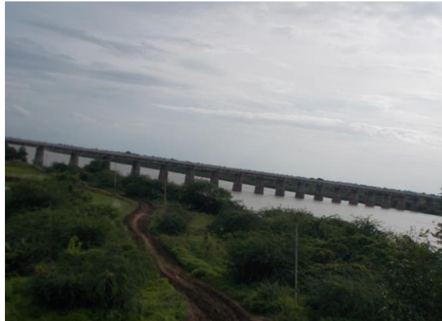
Figure 86 - Basar Road Bridge (ch.515.504km)
