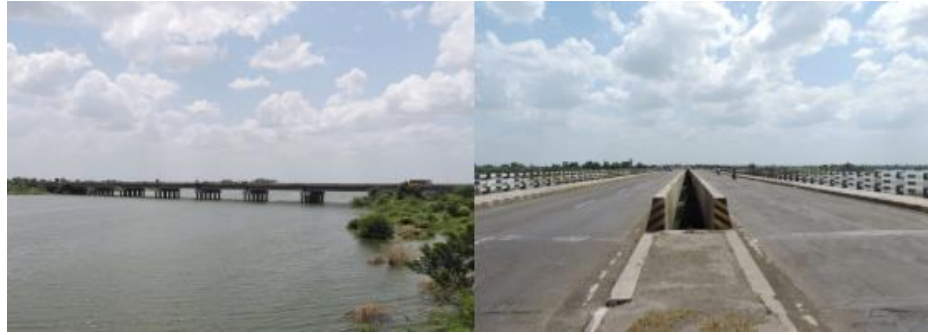
Figure 197 - Ahmednagar- Aurangabad Road Bridge (ch. 1014.12km)
