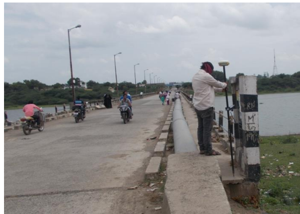
Figure 119 - Hsapur-Asarjan Road Bridge (ch. 617.471km)
