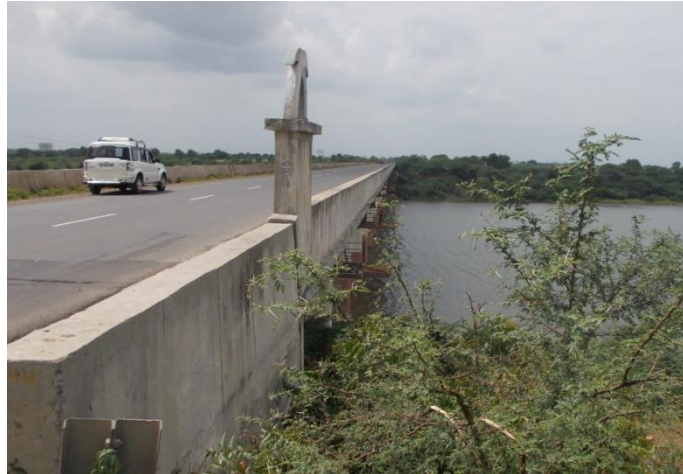
Figure 111 - Degloor- Naka Road (ch.611.878km)
