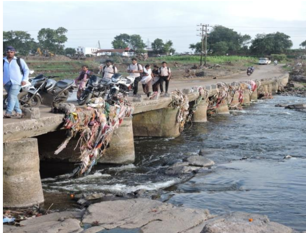
Figure 248 - Odha Road Bridge (ch. 1188.294km)
