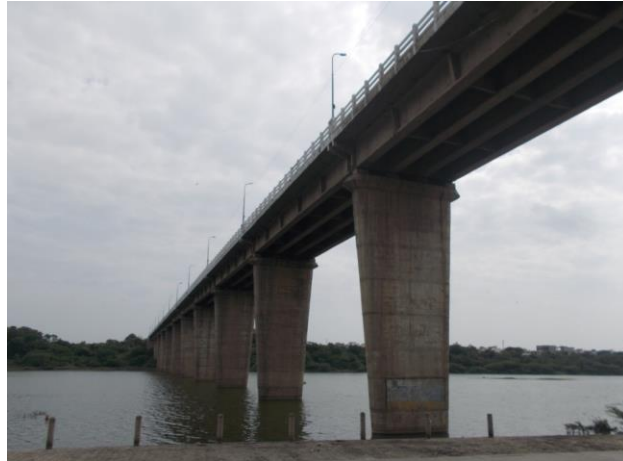
Figure 114 - Vikas Nagar-Old Mondha Road Bridge (ch. 614.641km)
