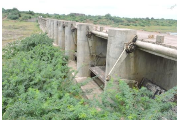
Figure 173 - Patharwala Barrage (ch. 907.618km)
