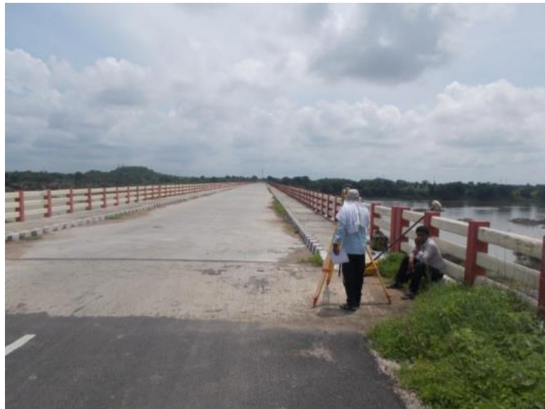
Figure 72 - Gummiryal Godavari Road Bridge (ch.434.730km)
