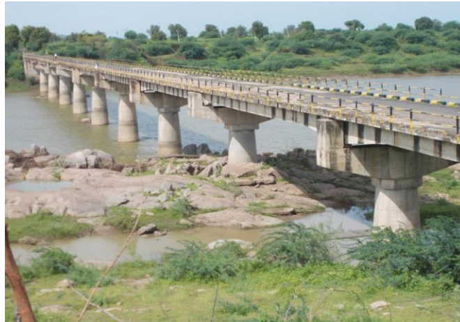
Figure 96 - Kundalwadi- Jarikot Road Bridge (ch.545.590km)
