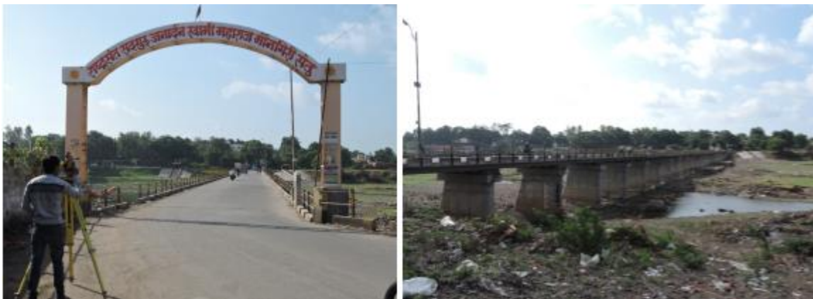
Figure 224 - Kopergaon Road Bridge (Maungiri Setu) – ch. 1100.293km
