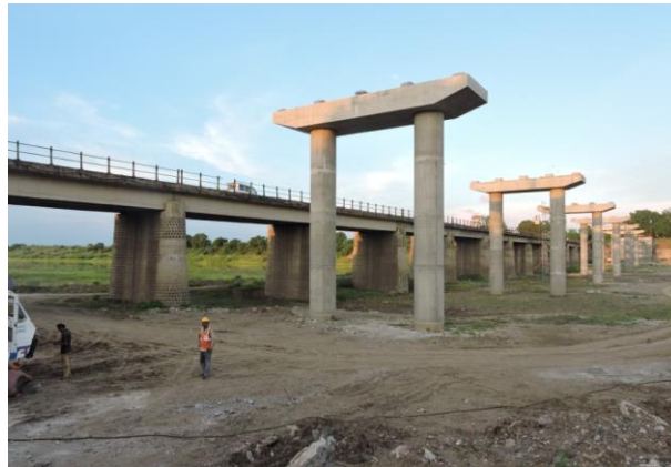
Figure 158 - Under construction Road Bridge (ch. 810.165km)
