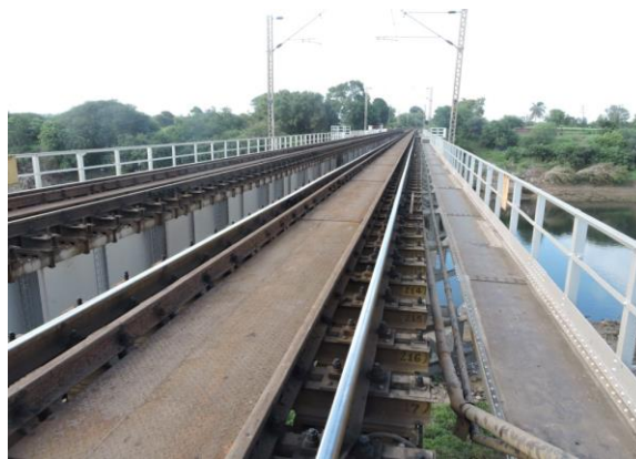
Figure 251 - Panchak Railway line Bridge (ch. 1192.181km)
