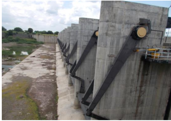
Figure 137 - Muli Barrage (ch. 720.262km)
