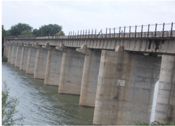
Figure 103 - Mahati- Eli Gaon River Bridge (ch. 585.545km)
