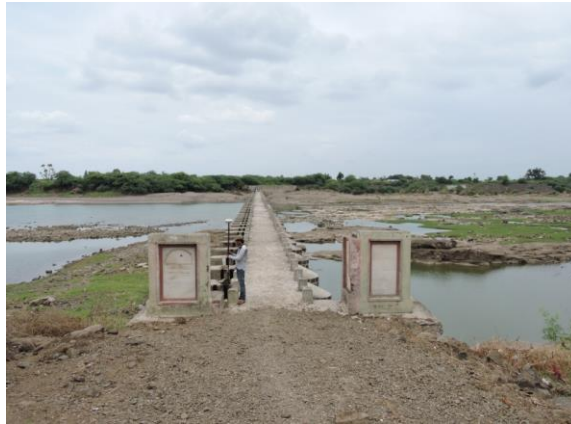
Figure 218 - Check Dam near Duch Khurd village (ch. 1084.368km)
