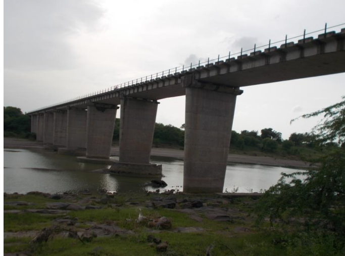
Figure 99 - Baligon Road Bridge (ch.567.519km)
