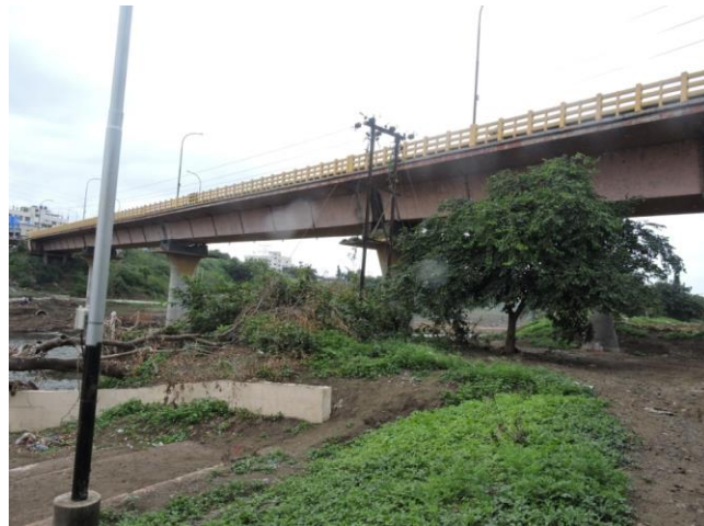
Figure 255 - Tapovan Road Bridge (ch. 1200.82km)
