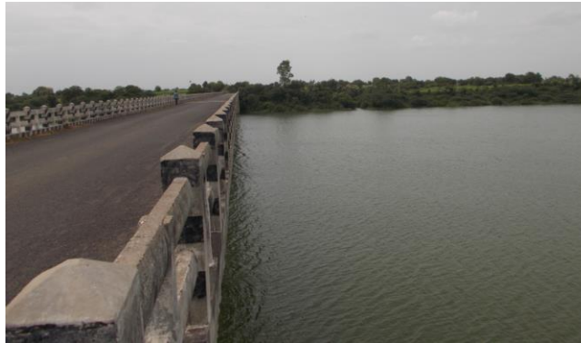
Figure 128 - Purna - Loha Road Bridge (ch. 665.762km)
