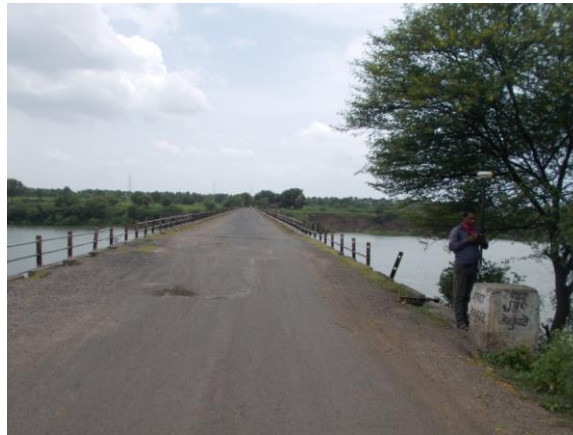
Figure 105- Amdura Road Bridge (ch. 600.951km)
