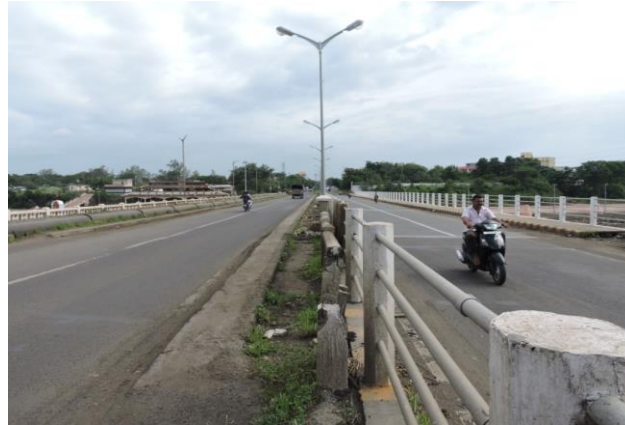
Figure 252 - Nandur Naka Road Bridge-NH-60 (ch. 1195.923km)
