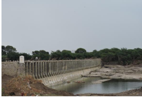
Figure 231 - Check Dam near Maygaon Devi village (ch. 1125.943km)
