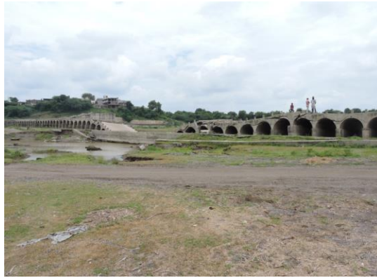
Figure 182 - Apegaon- Kurnapimpri Road Bridge (ch. 946.774km)
