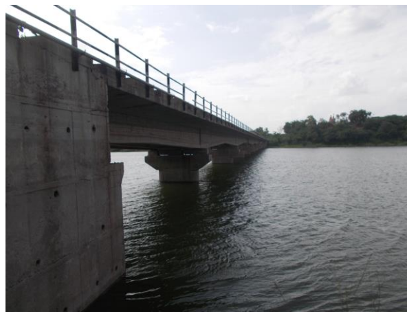
Figure 130 - Palam - Tadkalas Raod Bridge (ch. 679.68km)
