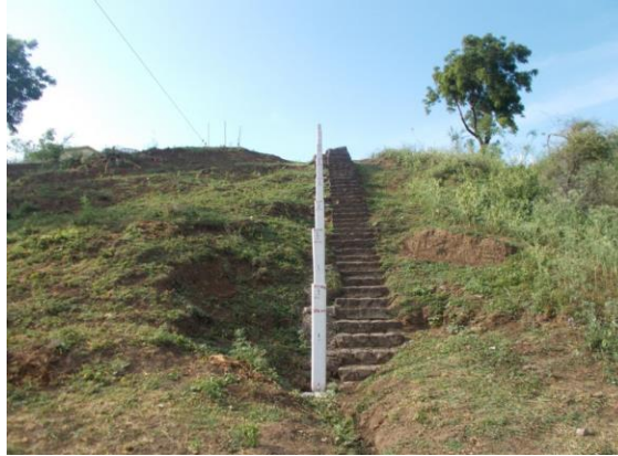
Figure 135 - CWC gauge station Gangakhed (ch.715.11km)
