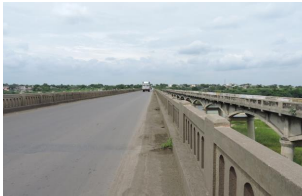
Figure 175 - Jalna Beed Road Bridge (ch. 916.64km)
