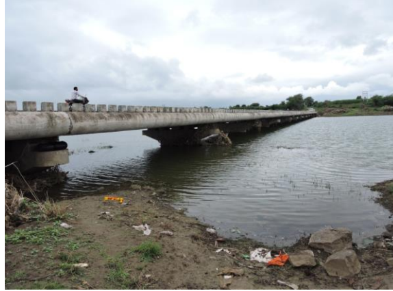
Figure 239 - Dharangaon Road Bridge (ch1146.714km)
