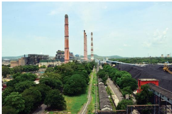
Figure 261 - NTPC Ramagundem (ch.293.200km)
