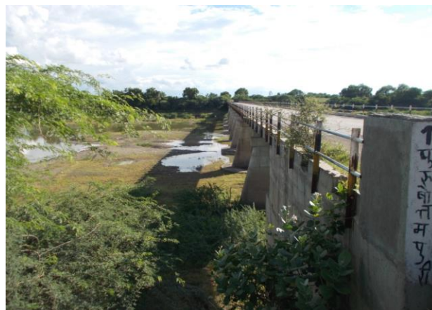
Figure 163 - Sadola-Ashti Road Bridge (ch. 834.469km)
