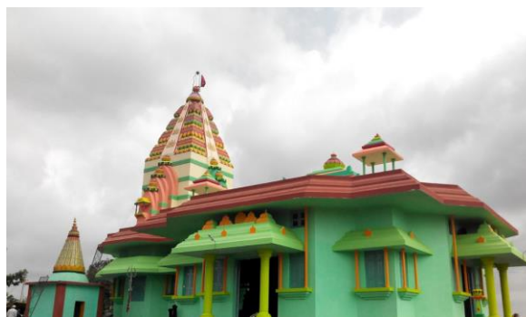
Figure 230 - Mayagaon Devi Temple (ch. 1124.601km)
