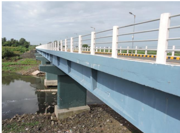
Figure 253 - Old Saikheda Road Bridge (ch. 1198km)
