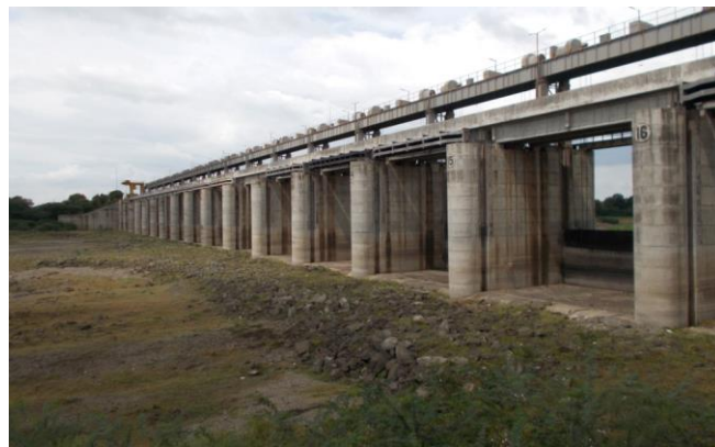
Figure 170 - Jogladevi Barrage (ch. 890.798km)
