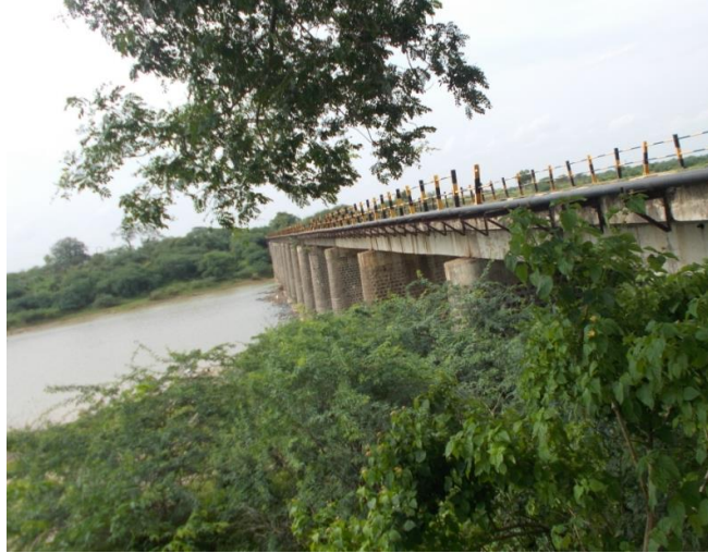
Figure 97 - Narsi-Umri Road Bridge (ch.553.55km)
