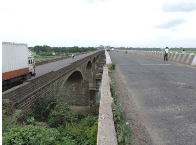
Figure 223 - Sangamner - Kopergaon Road Bridge (ch. 1099.287km)
