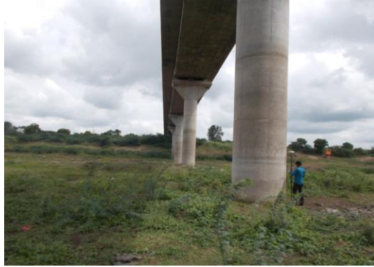
Figure 150 - Sonpeth-Pathari Road Bridge (ch. 767.025km)
