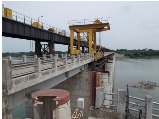
Figure 166 - Rajatakli High-Level Barrage (ch.857.147km)
