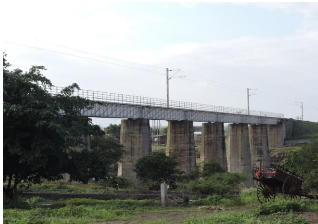
Figure 249 - Odha Railway line Bridge (ch. 1188.608km)
