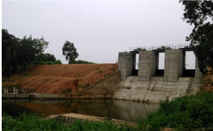
Figure 88 - Ali Sagar Lift Irrigation (ch.519.612km)
