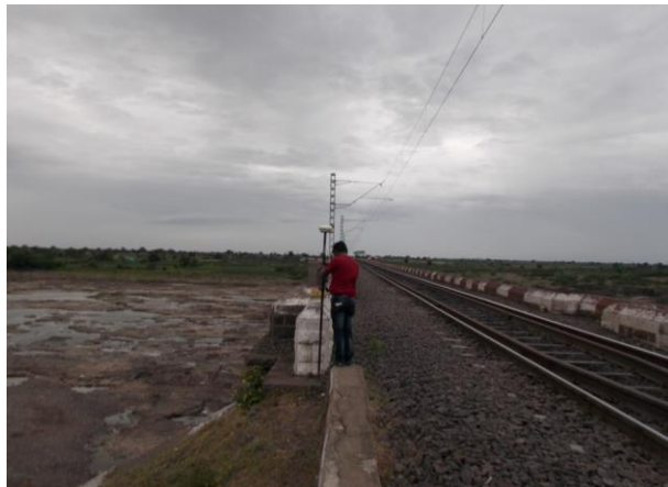
Figure 214 - Railway line Bridge near Dongaon village (ch. 1077.01km)
