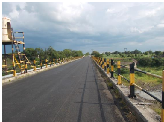
Figure 142 - Shelgaon- Shirshi Road Bride (ch.748.281km)
