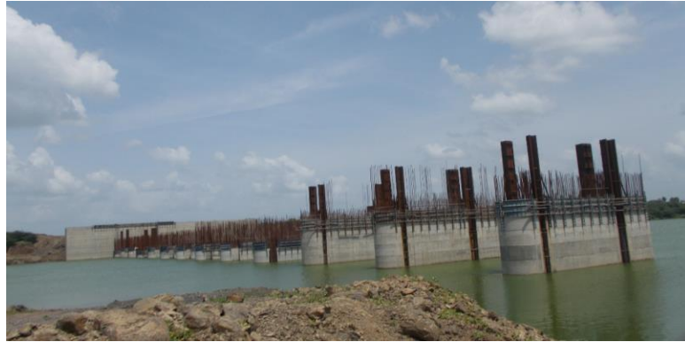
Figure 125 - Anteshwar Barrage (ch. 653.866km)
