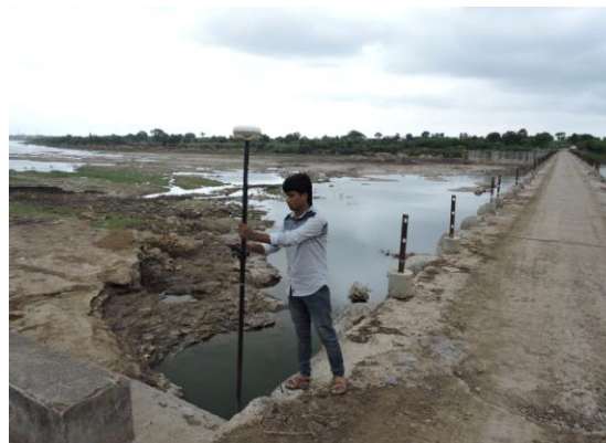
Figure 233 - Check Dam near Kanlad village (ch. 1131.56km)
