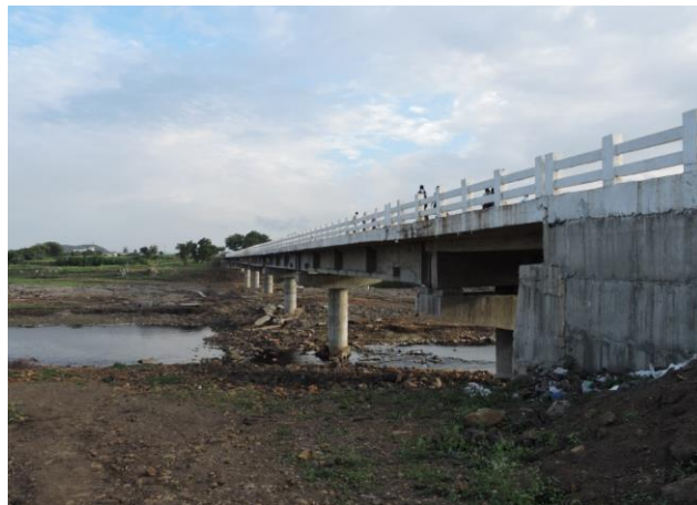
Figure 247 - Lakhalgaoon Road Bridge (ch. 1186.016km)
