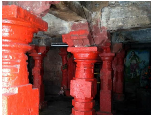
Figure 131 - Somnath Temple (ch.684.417km)
