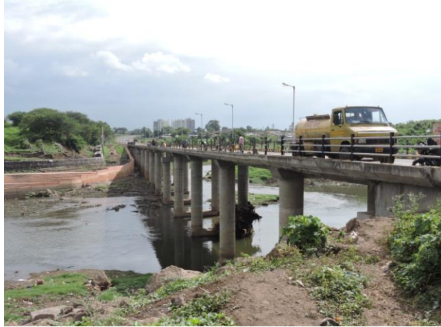
Figure 254 - Samta Nagar Road Bridge (ch. 1198.765km)
