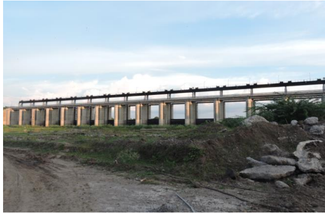
Figure 157 - Dhalegaon Barrage (ch. 810.0km)
