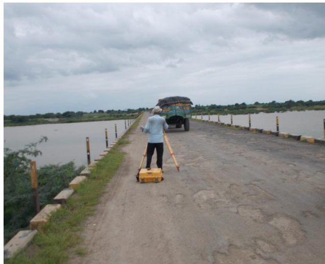
Figure 89 - Kandakurthi Road Bridge (ch.527.355km)
