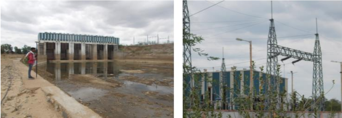
Figure 17 - Hydro Power Plant Barrage Dummugudem 24 MW (ch. 21.903km)
