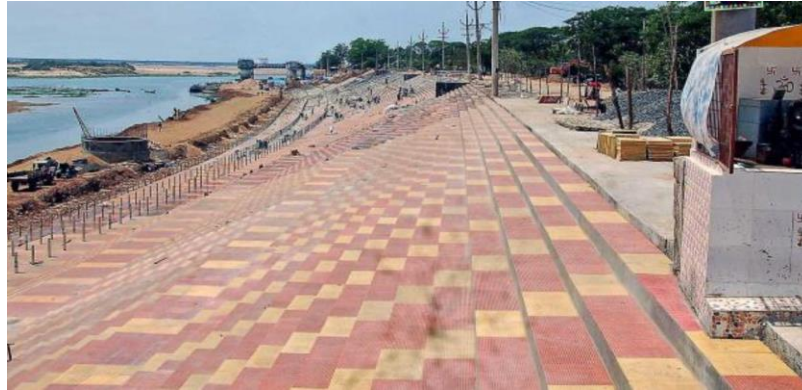
Figure 59 - Pushkar Ghat at Dharmapuri (ch.346.0km)
