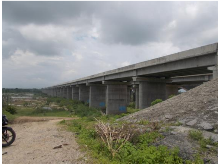
Figure 75 - Srinagar- Kanyakumari (NH-44) Road Bridge (ch.452.10km)
