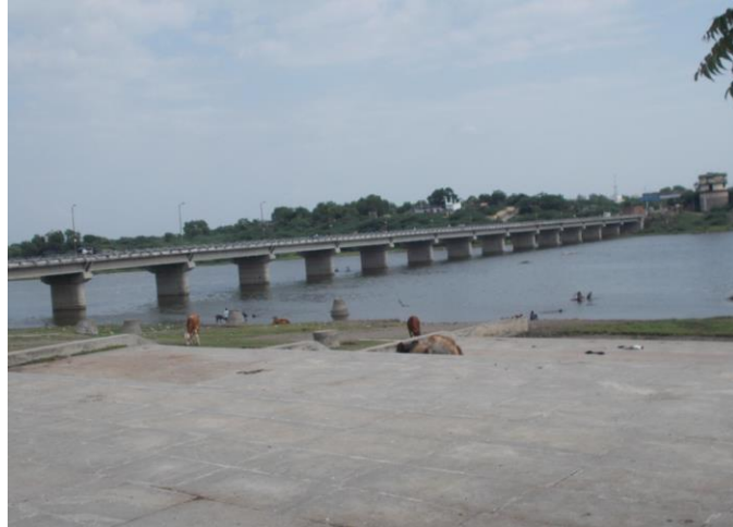
Figure 112 - Navghat Road Bridge (ch. 613.493km)
