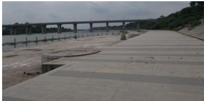
Figure 113 - Ghats near Nanded on Godavari River (ch.614.30km)
