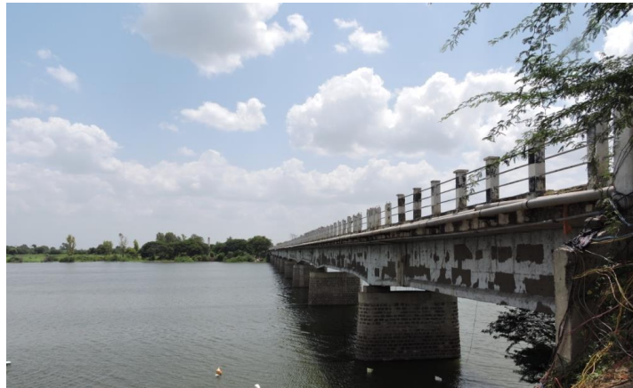
Figure 196 - Old Pravarasangam Road Bridge (ch. 1013.797km)
