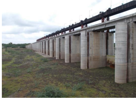
Figure 148 - Mudgal Barrage (ch.764.753km)
