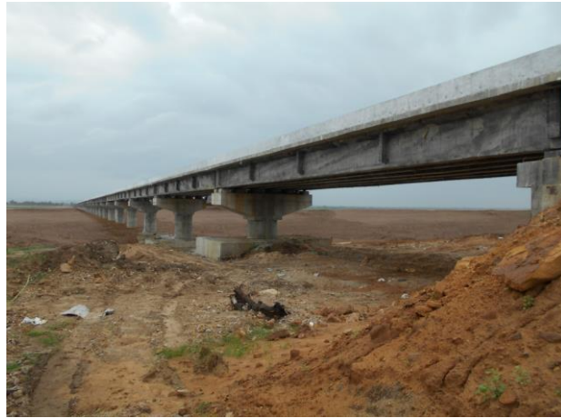
Figure 41 - Sironcha Road Bridge (ch.213.495km)
