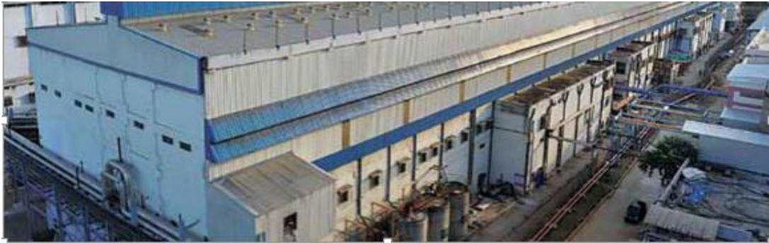
Figure 19 - ITC paper mill near Sarapaka, Bhadrachalam (ch.2.0km)
