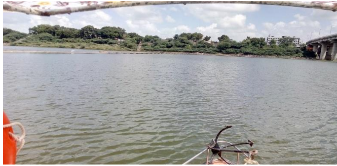
Figure 118 - Check Dam (ch.615.793km)
