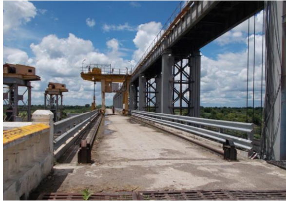
Figure 162 - Lonisawangi High-Level Barrage (ch 828.144km)
