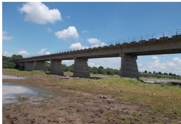
Figure 151 - Pohner Road Bridge (ch. 782.292 km)
