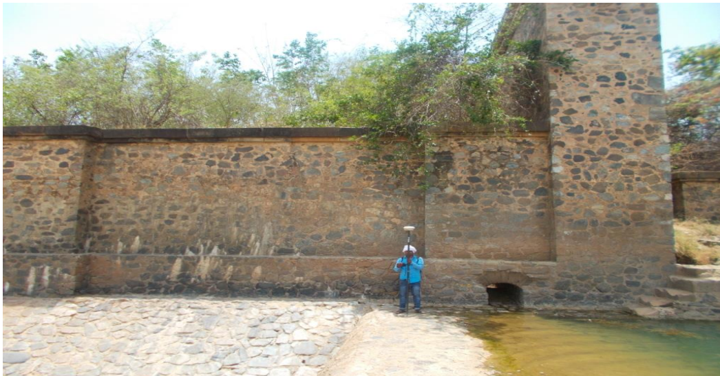
Figure 18 - Check Dam near Kasinagram (Dummagudem-ch24.043km)
