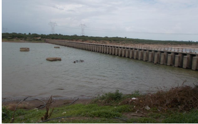
Figure 220 - Check Dam near Vari village (ch. 1090.485km)
