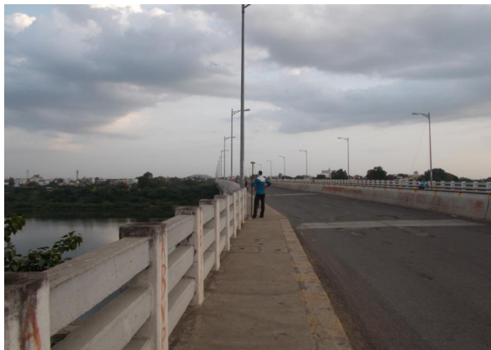
Figure 117 - Gowerdhan Ghat Road Bridge (ch. 615.639km)
