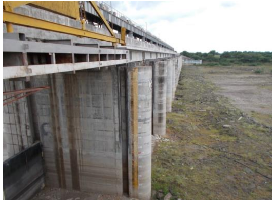
Figure 141 - Khadaka Barrage (ch.736.937km)
