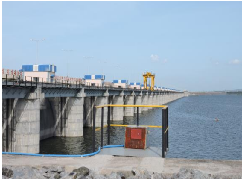
Figure 54 - Yellampally Dam (ch.310.5km)
