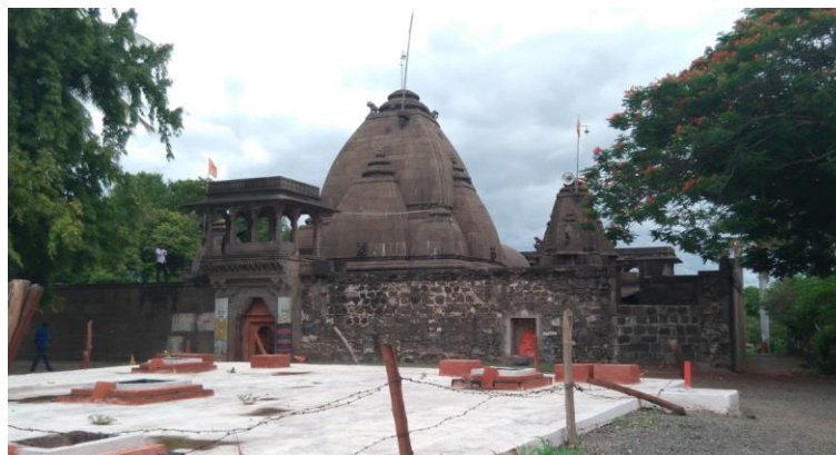
Figure 199 - Sidheshwar Temple Toka (ch.1014.846km)
