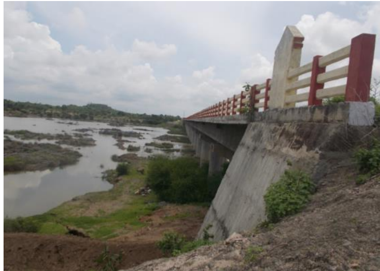
Figure 67 - Khanapur Road Bridge (ch.411.479km)
