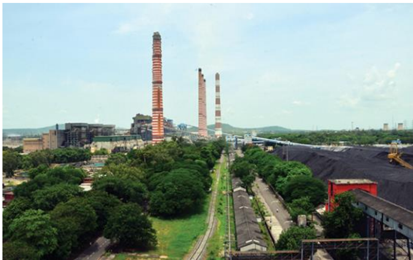
Figure 50 - NTPC Ramagundam (ch.293.20km)
