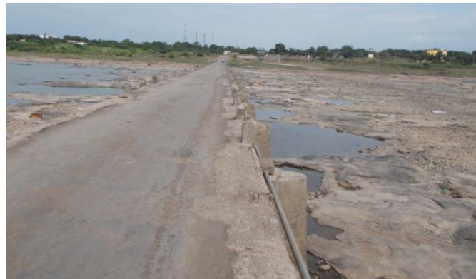
Figure 219 - Vari Road Bridge near Vari village (ch. 1086.718km)
