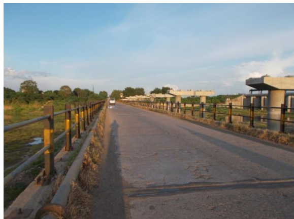
Figure 159 - Majalgaon-Pokharni Road Bridge NH-61 (ch. 810.172km)
