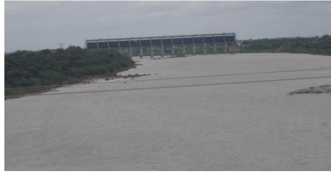
Figure 92 - Babhali Barrage (ch. 535.665km)
