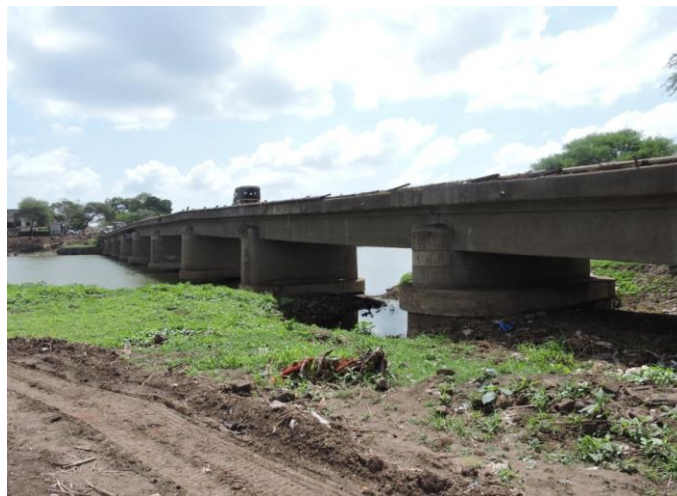
Figure 243 - Saykheda Road Bridge (ch. 1170.957km)
