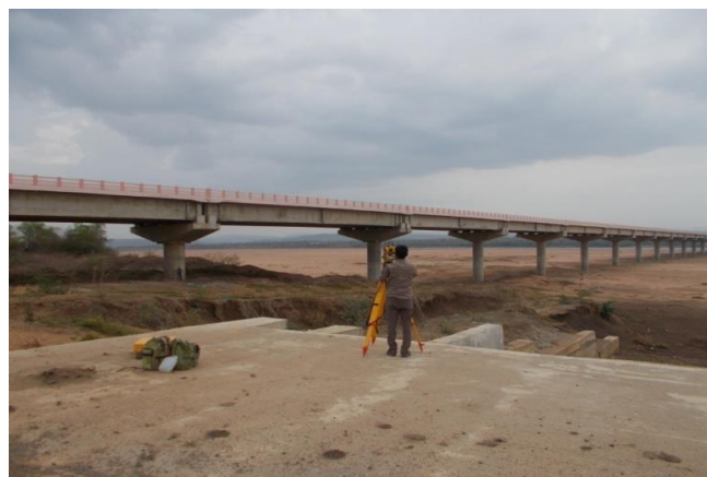
Figure 30 - Venkatapuram Road Bridge - NH-163 (Ch.112.184km)
