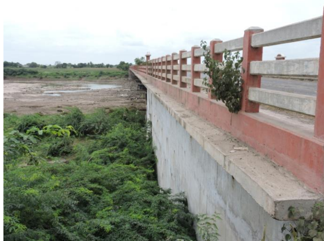
Figure 221 - Nagpur–Aurangabad–Mumbai Highway Road Bridge (ch. 1095.747km)
