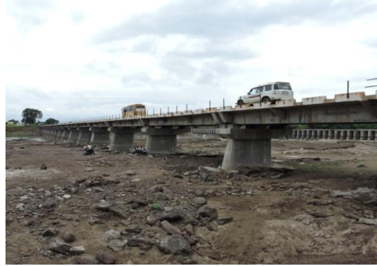
Figure 234 - Khedale Zunge Road Bridge (ch. 1137.634km)
