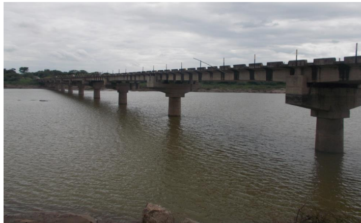
Figure 93 - Babhali Road Bridge (ch.537.968km)
