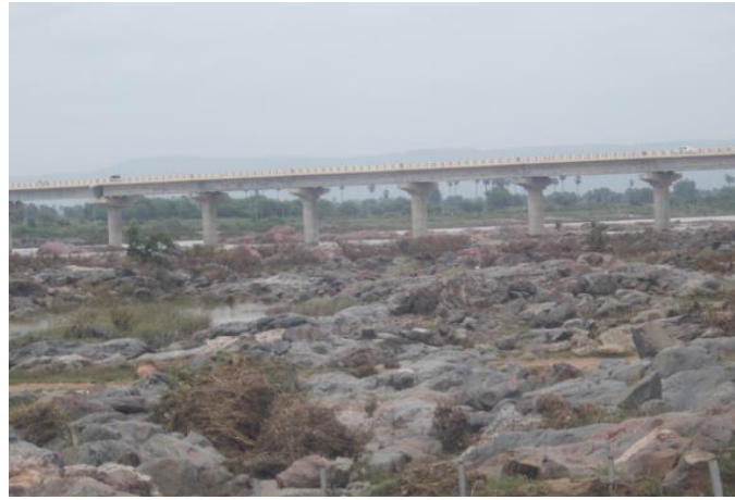
Figure 63 - Kalamadugu- Kammanur Road Bridge (ch.372.143km)
