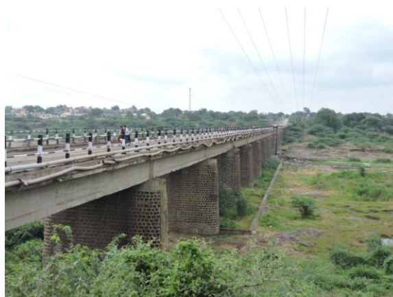
Figure 188 - Paithan – Shevgaon Road Bridge-SH- 148 (ch. 963.136km)
