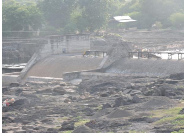
Figure 250 - Water pipeline near Odha village (ch.1188.889km)
