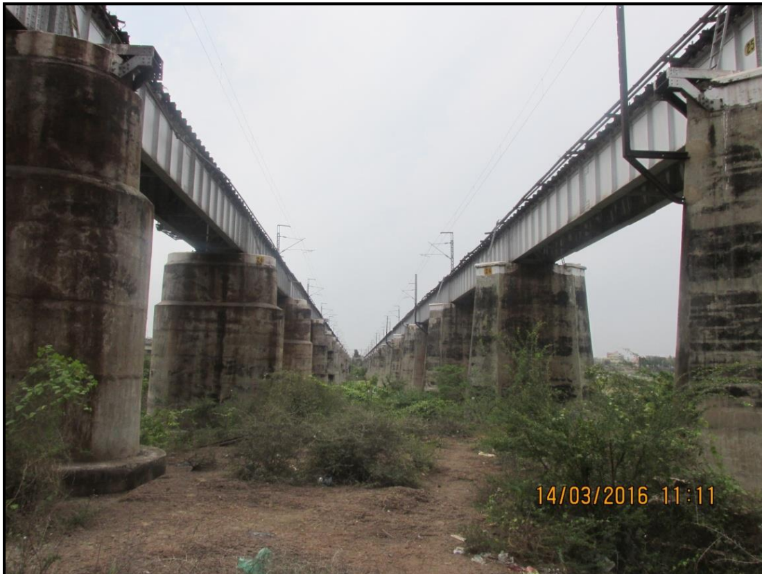
10: Penna Railway Bridge at chainage 28.23 km
