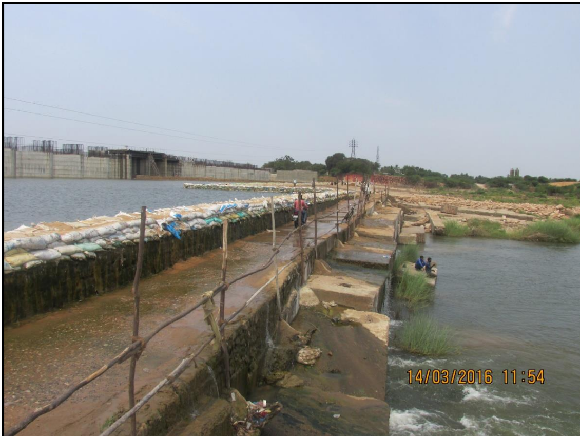
12: Dismantled Nellore Anicut at chainage 28.94 km
