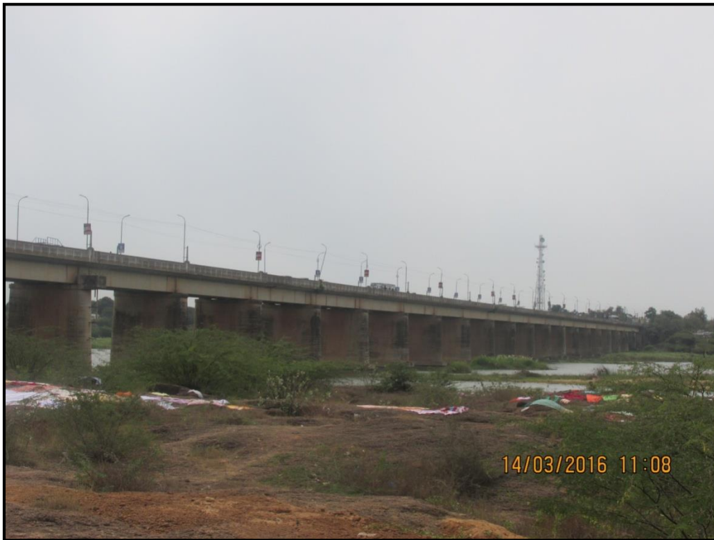
8: Panna Road Bridge 57 (Bellary Nellore Road) at chainage 28.13 km
