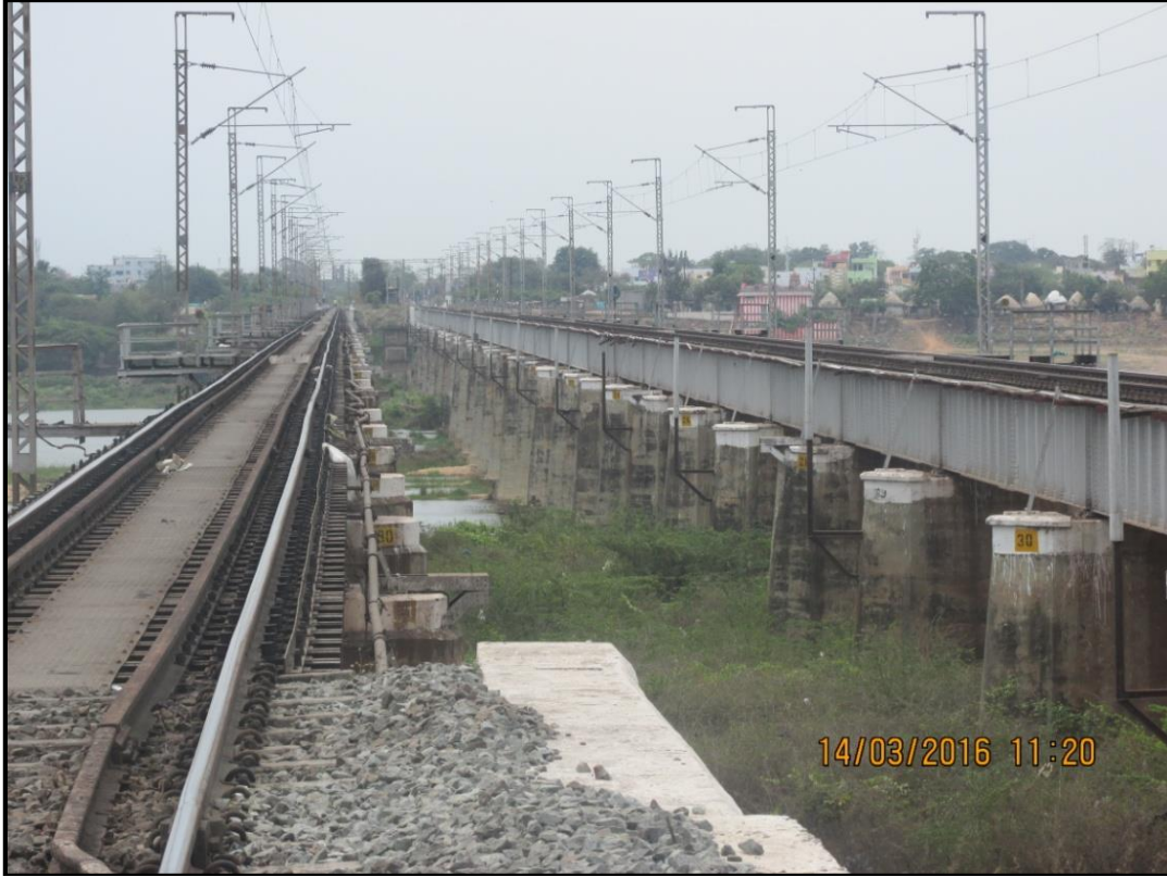
9: Penna Railway Bridge at chainage 28.23 km
