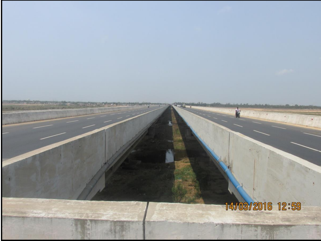
5: Guntur-Chennai National Highway-5 at chainage 25.93 km
