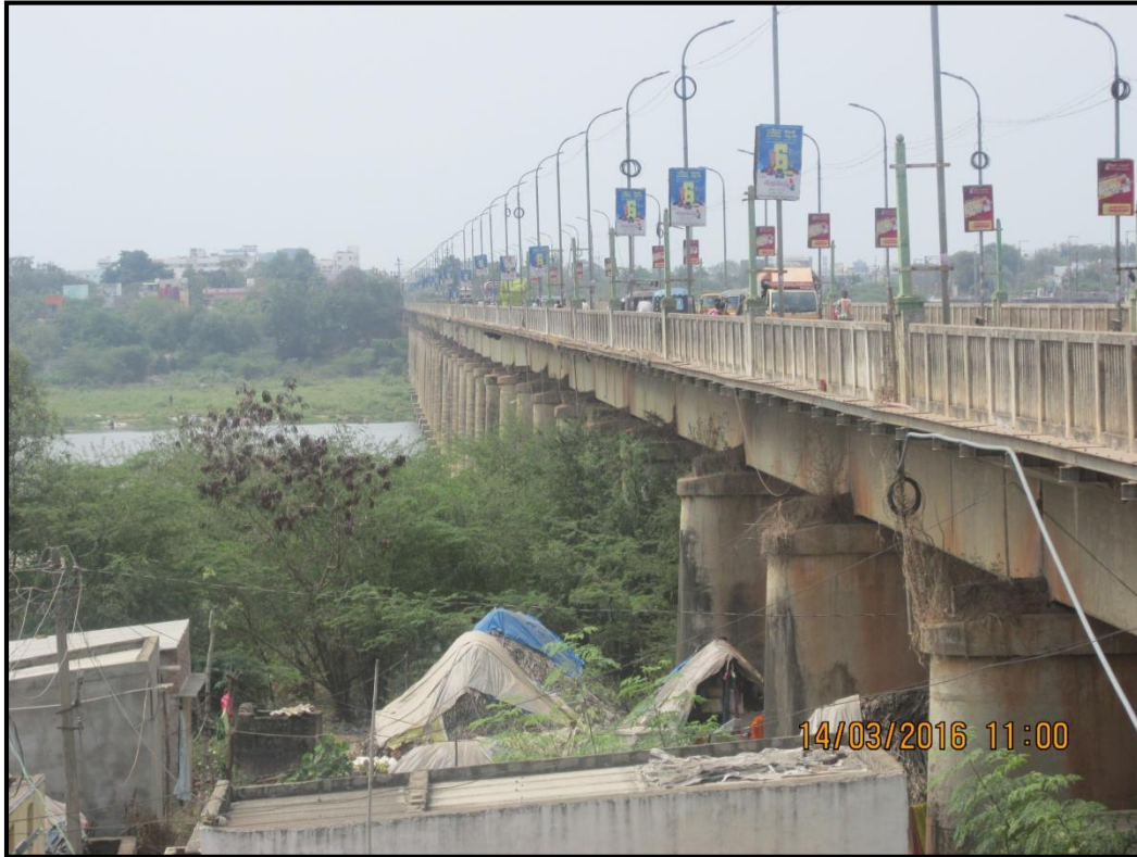
7: Panna Road Bridge 57 (Bellary Nellore Road) at chainage 28.13km
