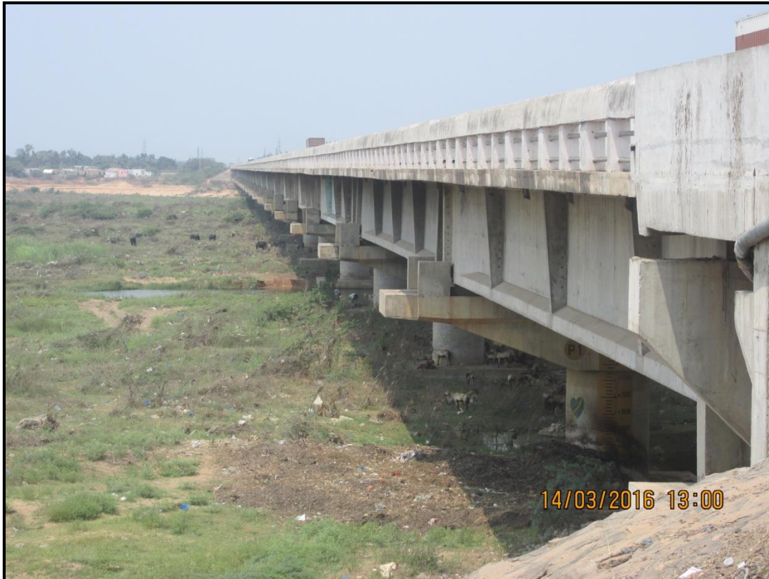
6: Guntur-Chennai National Highway-5 at chainage 25.93
