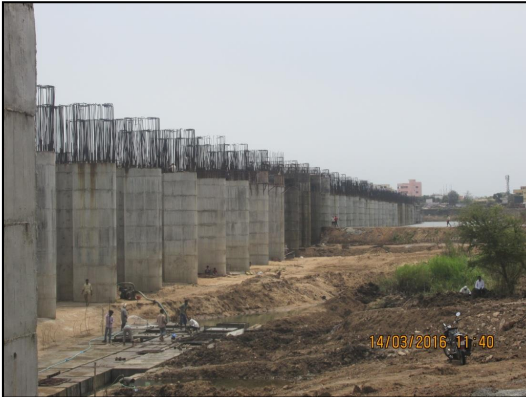
13: Pennar Barrage under Construction at chainage 29 km
