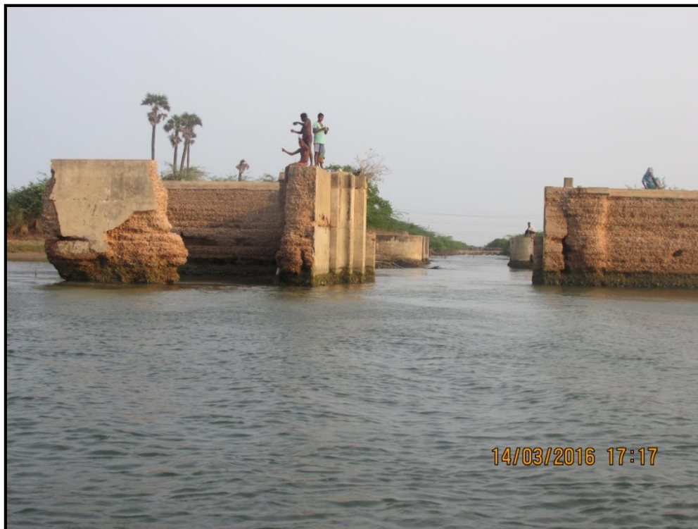
2: Buckingham Canal offtaking from Pennar River at chainage 2.1 km
