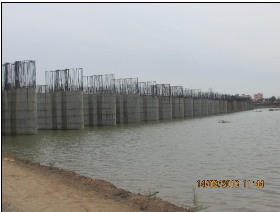
14: Pennar Barrage under Construction at chainage 29 km
