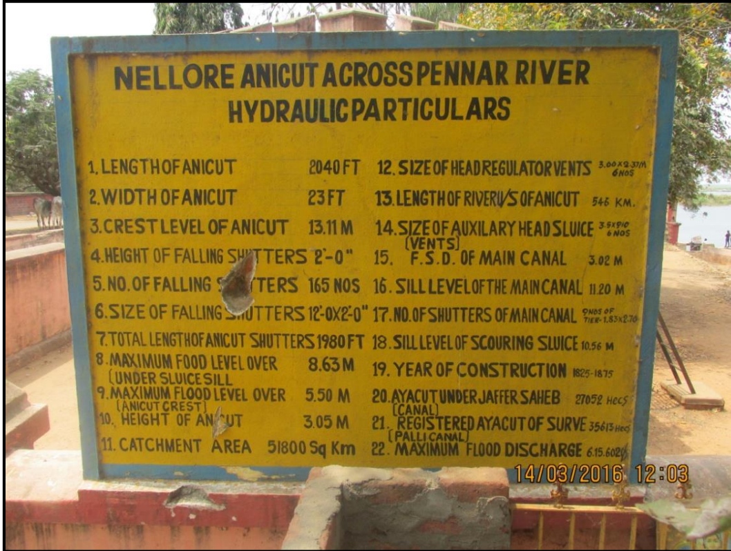
11: Dismantled Nellore Anicut at chainage 28.94 km
