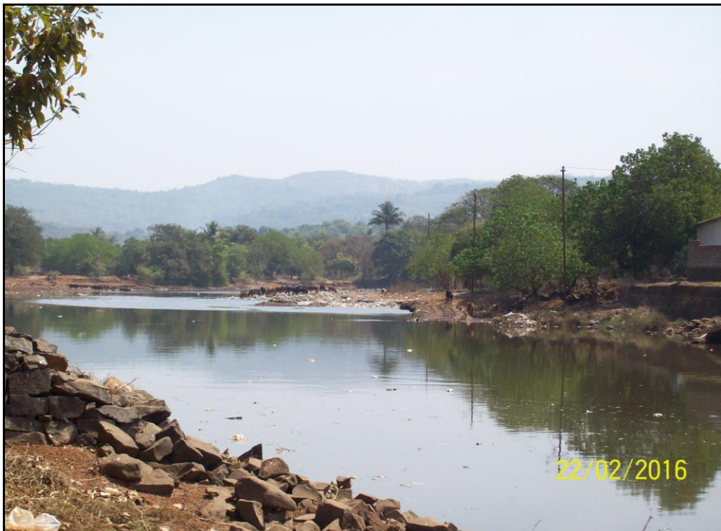
Photo 18: Landward side of the River at Ch 30.78km (18°08'16.7"N, 73°06'35.5"E)
