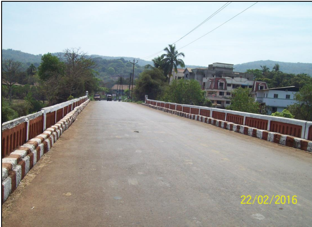
Photo 19: Bridge connecting Mhasala village to Khargaon at Ch 31.31km (18°08'11.7"N, 73°06'52.7"E)
