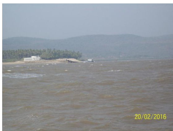
Figure 2.3: Agardanda Jetty at Chainage 6.515km
