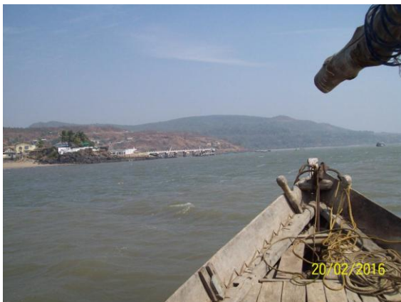
Figure 2.1: Rajpuri Jetty at Chainage 3.521 Km
