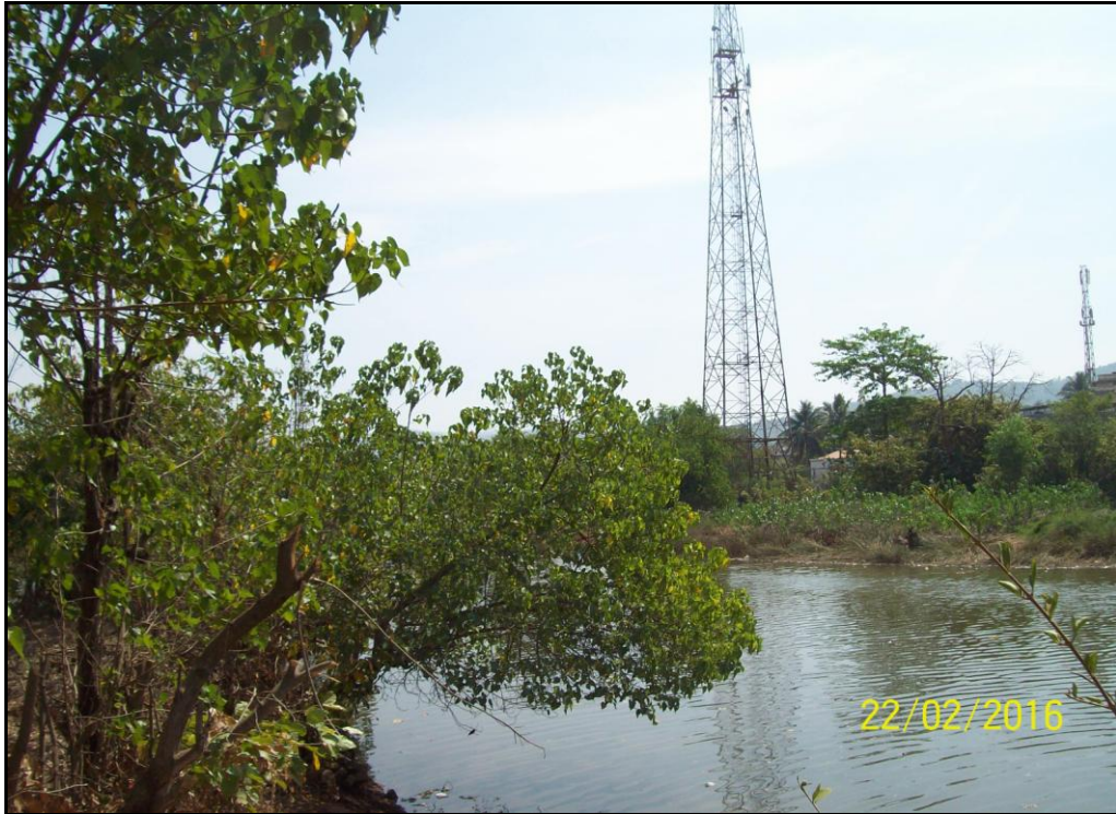
Photo 17: Telephone Tower at Ch 30.51km (18°08'13.2"N, 73°06'27.1"E)
