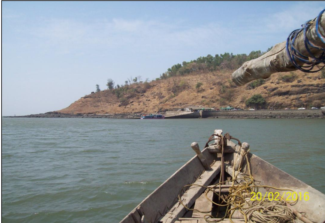
Photo 1: Murud Jetty at about 2.17km prior to Ch 0.0km (18°18'40.1"N, 72°57'45.5"E)
