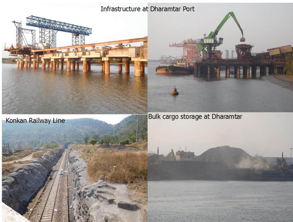
Source: Source: Consultant's Site Visit
