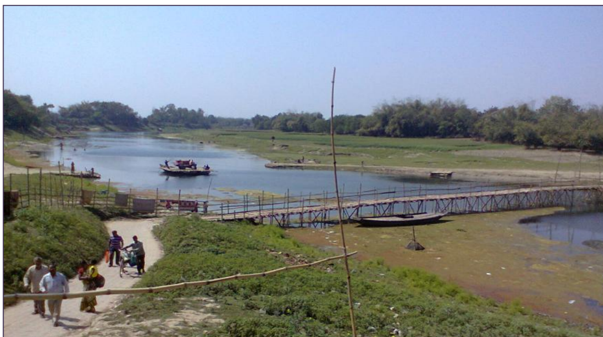
Figure 29- Tehatta ferry ghat and Foot Bridge (Chainage-113.40 km and 113.402 km)
