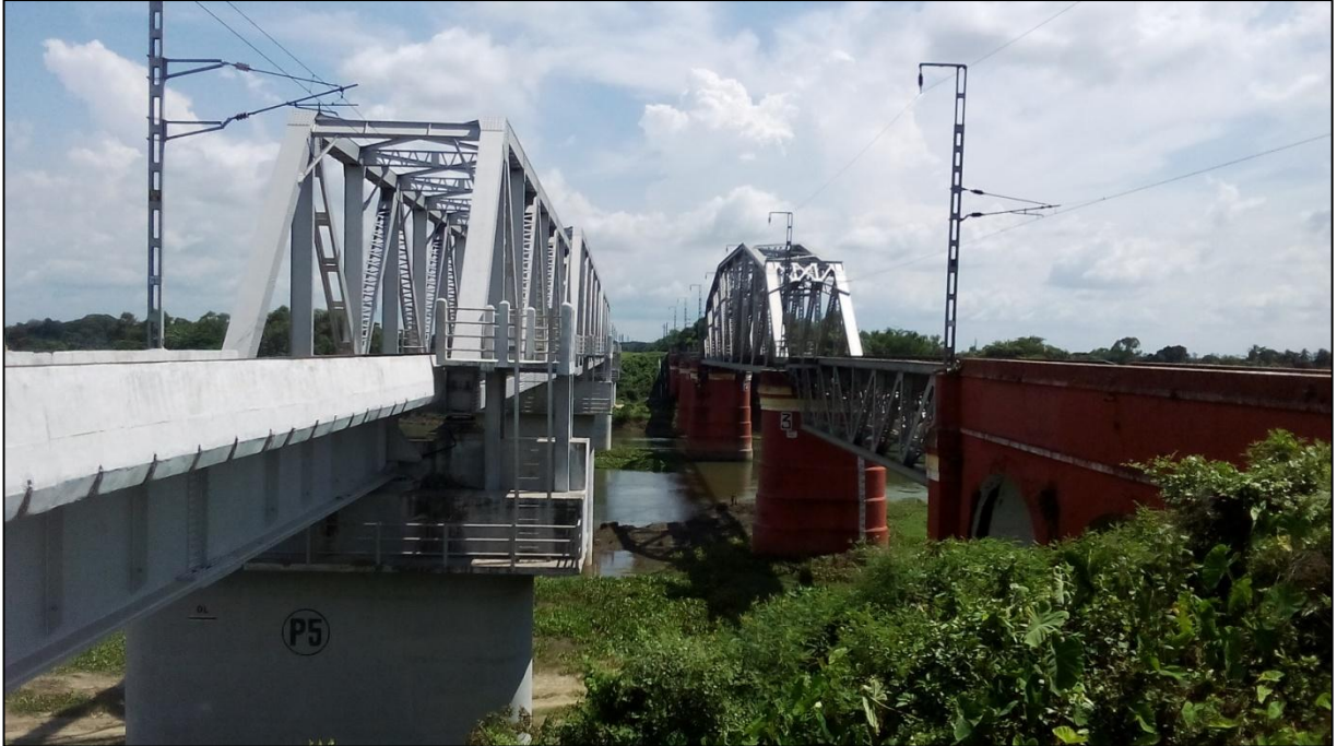
Figure 9- Rail Bridges (Krishnanagar - Bahadurpur) - 15.401 km and 15.421 km
