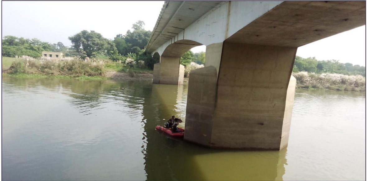
Figure 31- RCC Bridge (Chainage- 130.591 km)
