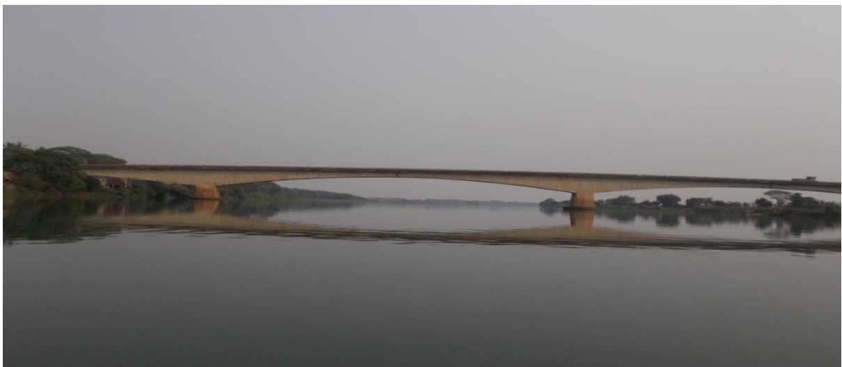
Figure 36: Patrapur Bridge (Ch. 26.0km)
