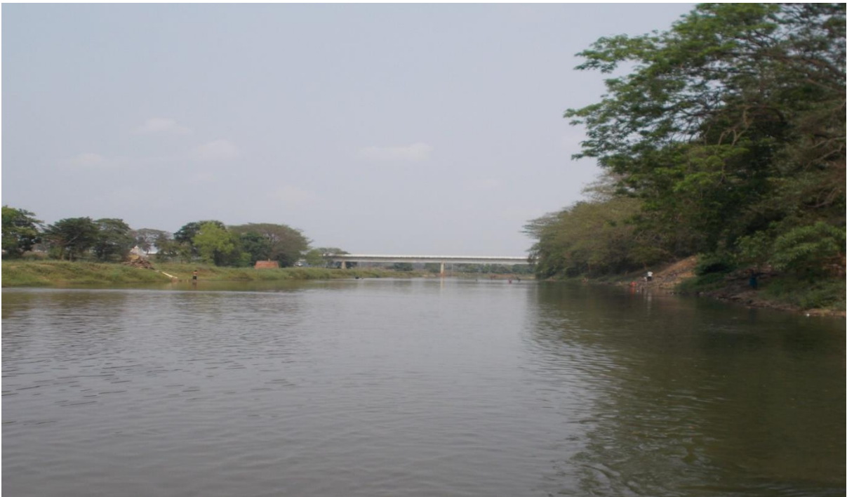
Figure 23 Gajendrapur Bridge (Ch. 53.0 km)
