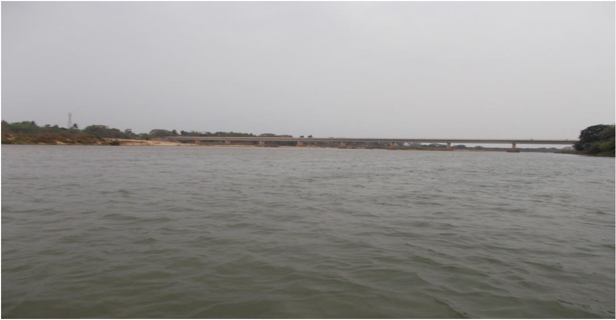
Figure 24 Kampagada Bridge (Ch. 57.6 km)
