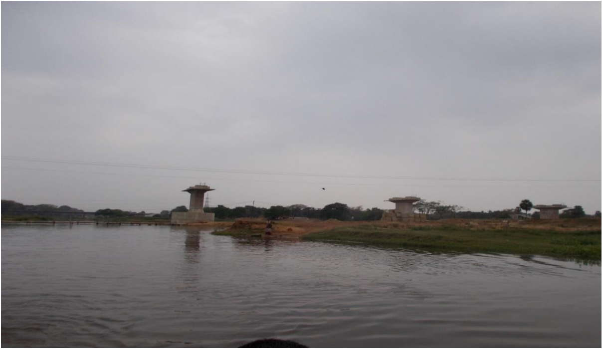
Figure 22: Nanapur Railway bridge (Ch. 45.0 km)
