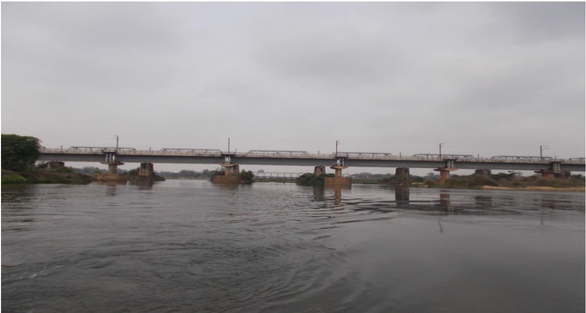
Figure 15: Manguli Railway bridge (Ch. 0.9 km)
