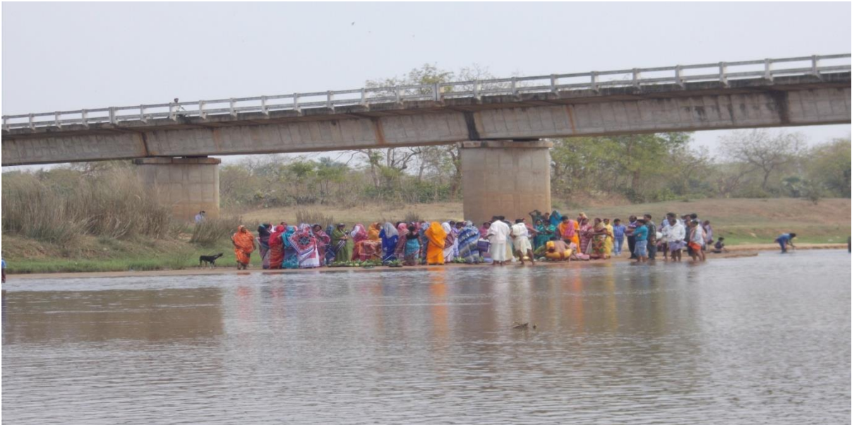
Figure 19: Triveniswar Bridge (Ch. 32.0 km)
