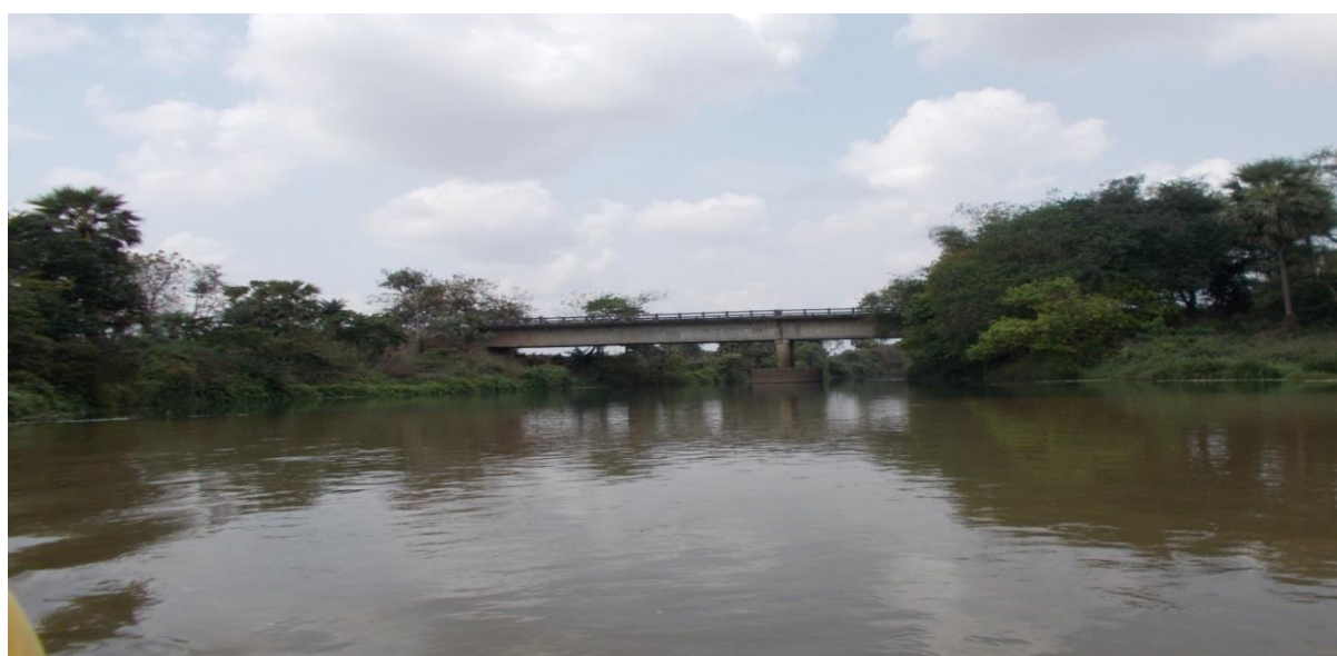
Figure 27: Baishimauja Bridge (Ch 10.85 km)
