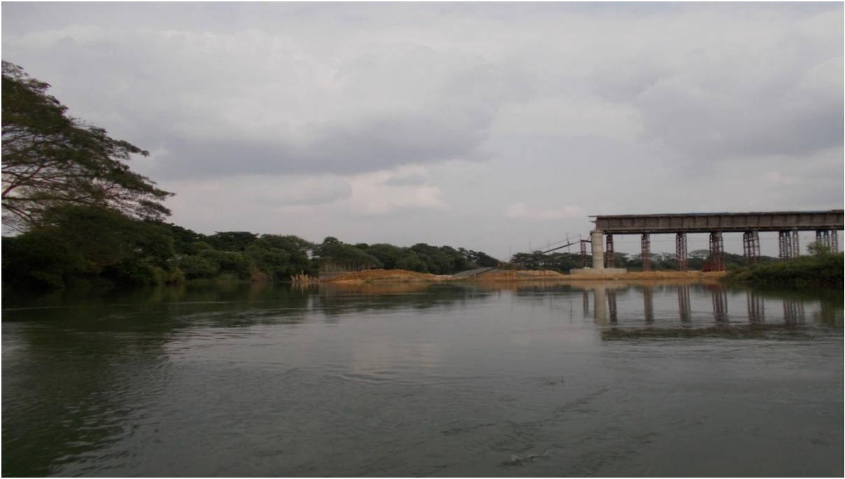
Figure 30: Under construction Badanachhipur Bridge (Ch. 21.0km)
