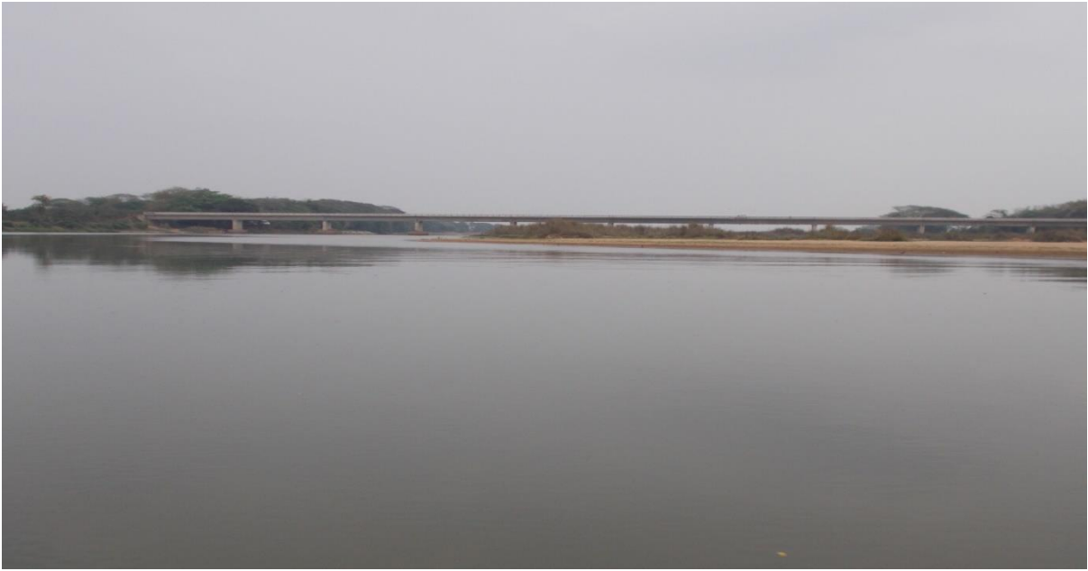
Figure 18: Dashrajpur Bridge (Ch. 26.1km)
