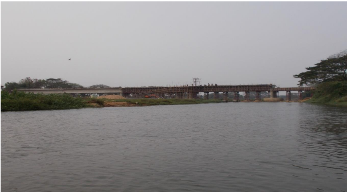
Figure 21: Kusupur Bridge (Ch. 43.5 km)
