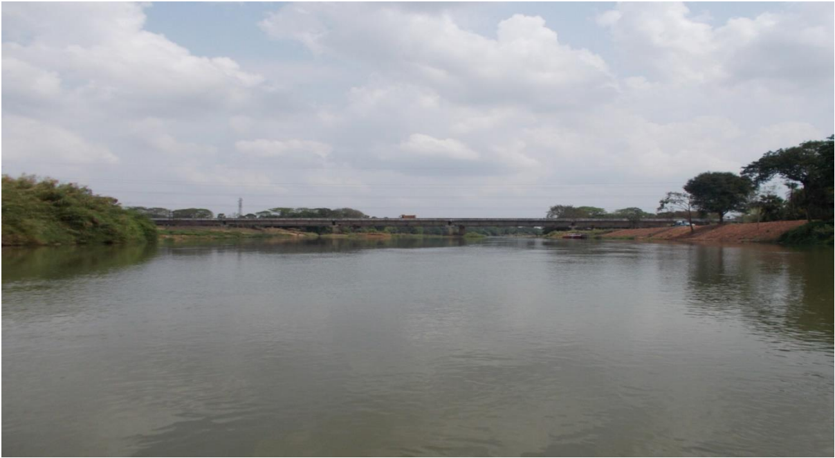
Figure 28: Benapur NH 5A Bridge (Ch. 14.8km)
