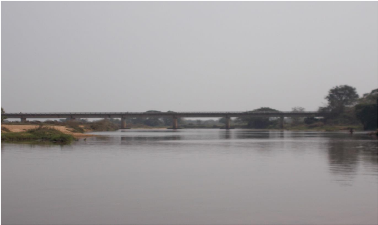
Figure 20: Kuanpal Bridge (Ch. 38.0 km)
