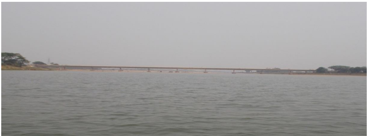
Figure 35: Dandisahi Bridge (Ch. 10.9km)
