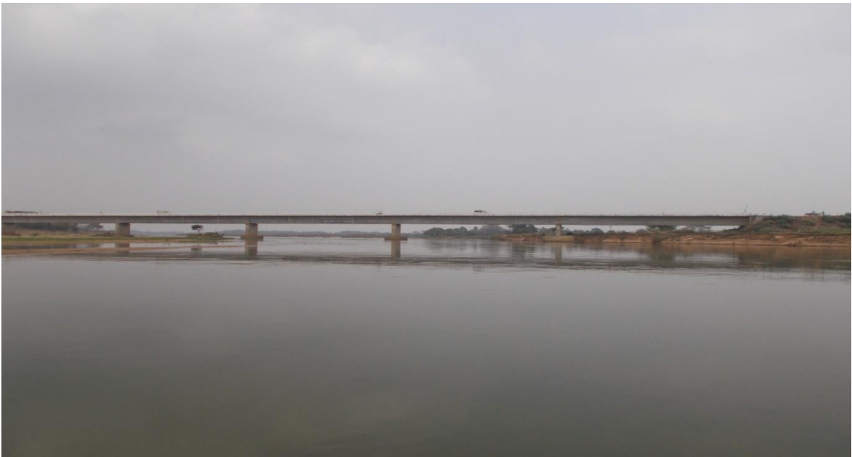
Figure 17: Bhatamunda Bridge (Ch. 12.5 km)
