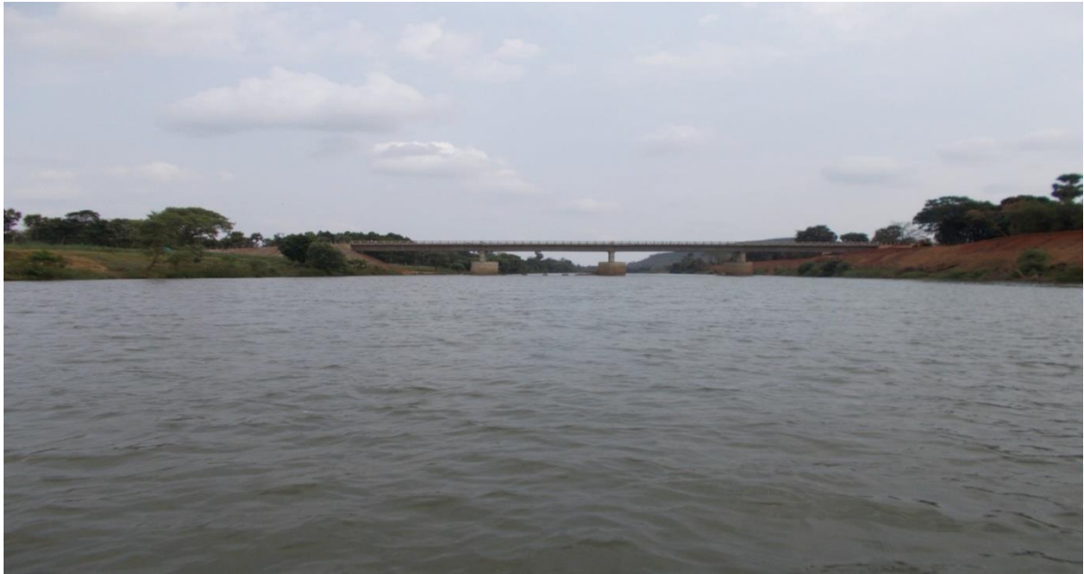
Figure 32: Banamalipur Bridge across Badi Genguti (Ch. 29.5km)
