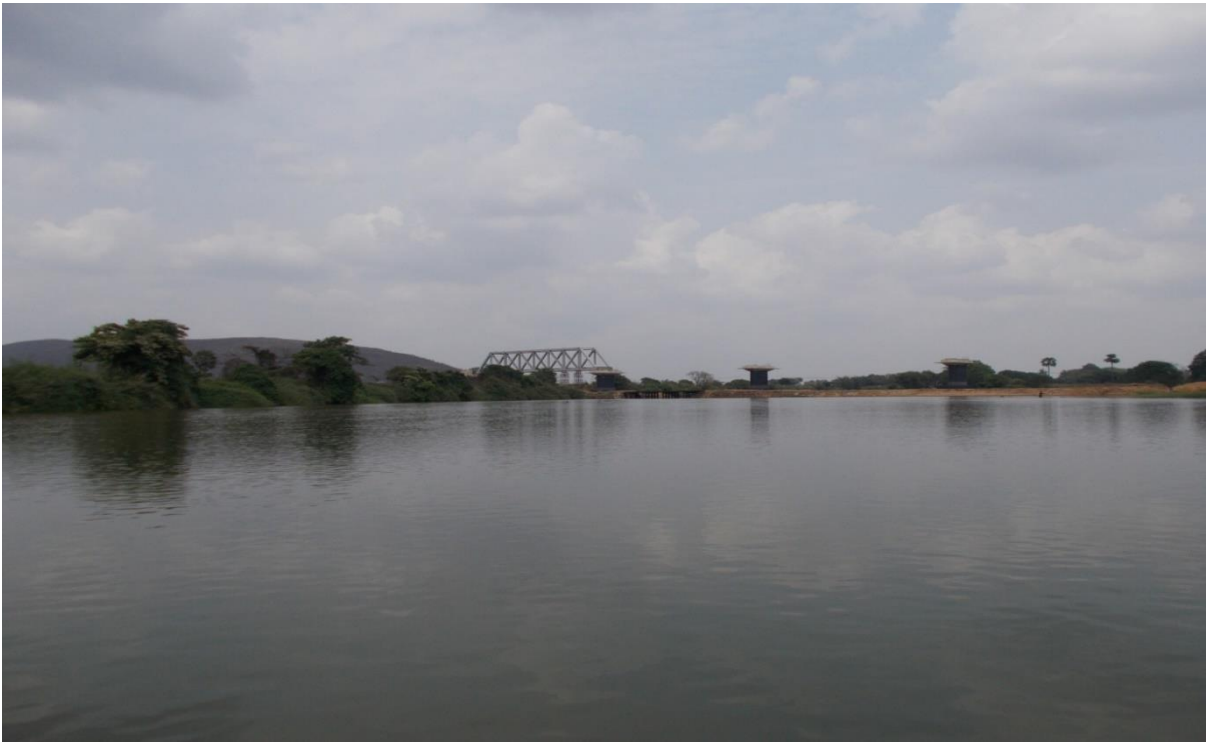
Figure 29: Khadianga Railway Bridge (Ch. 16.7 km)
