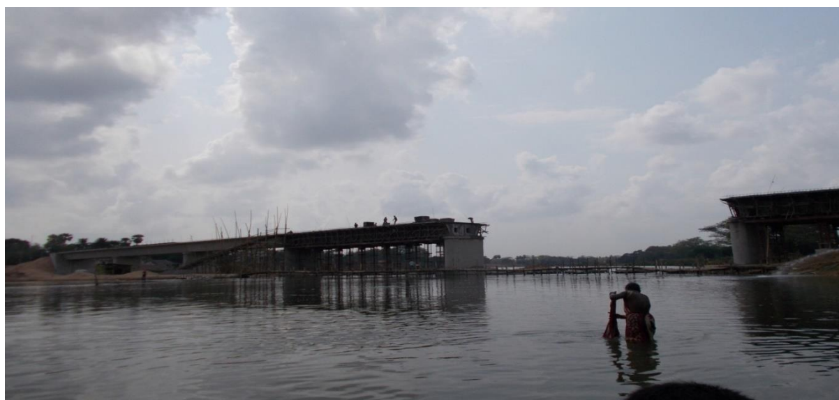
Figure 26: Gopalpur Bridge (Ch 6.3 km)
