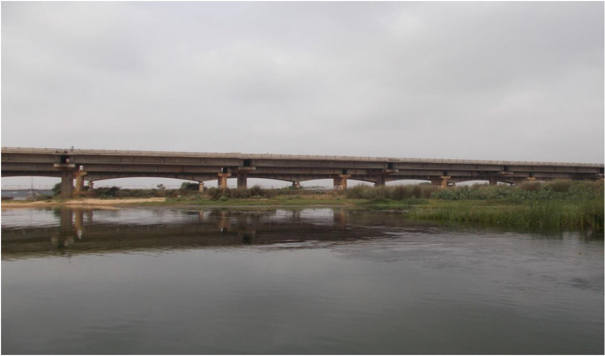
Figure 16: Manguli NH5 bridge (Ch. 1.0 km)
