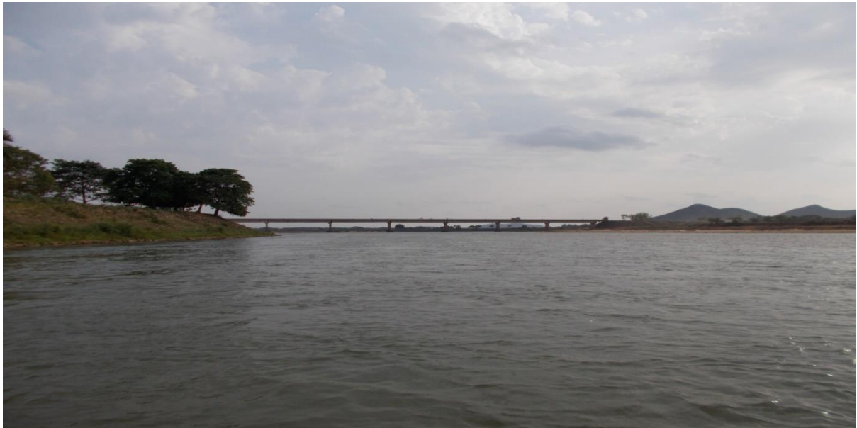
Figure 33: Balikuda Bridge across Badi Genguti (Ch. 33.5km)
