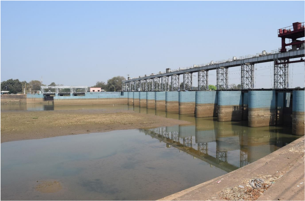
Figure 14: Birupa Barrage (Ch. 0.0 km)
