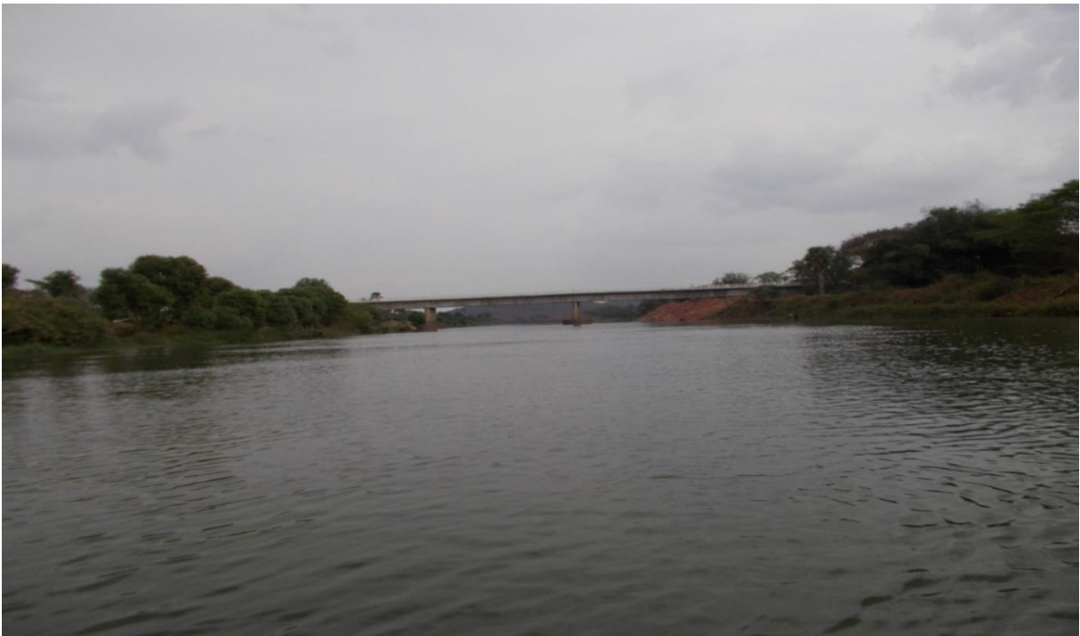
Figure 31: Arikana Bridge (Ch. 24.7km)
