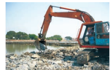
Construction of Rubble-dyke in progress at Sittwe
