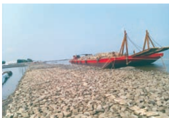
Construction material being brought to Sittwe by IWT barge.
