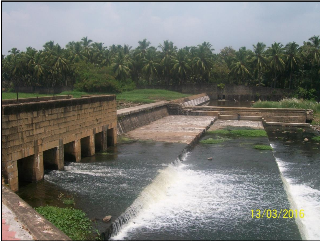
12: Kumari Dam side view at Chainage 14.10km
