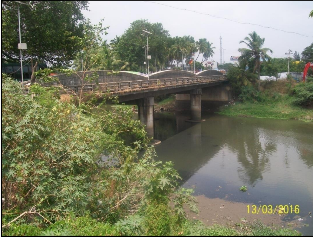
15: Olugunasery Bridge (NH-478) at Chainage 15.6km
