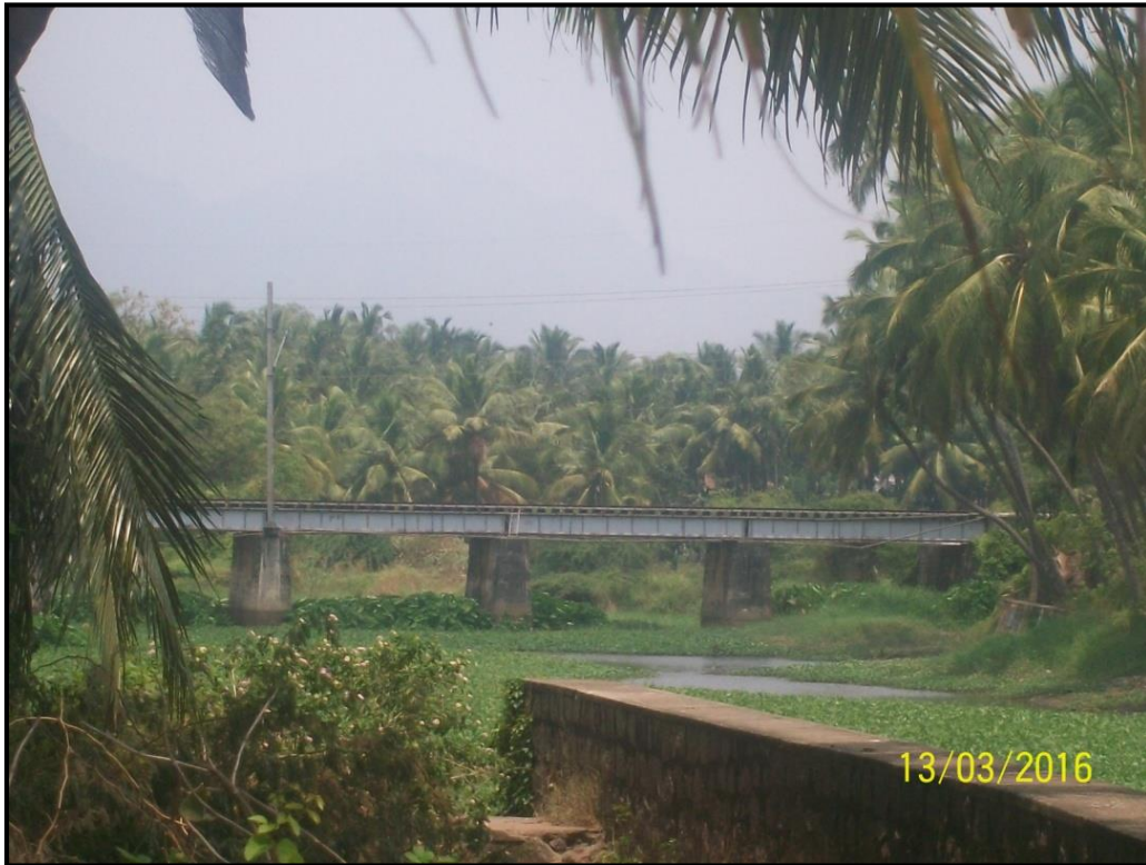
14: Railway Bridge at Chainage 14.6km
