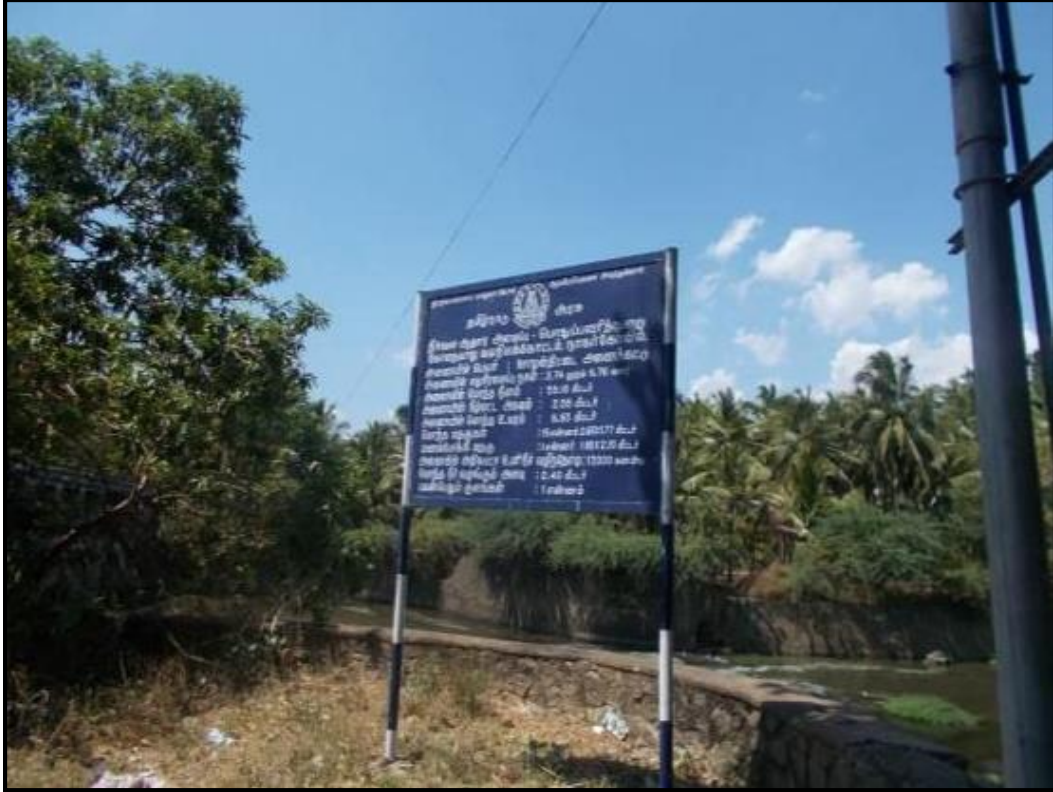
11: Solan Thittai Dam at Chainage 9.87km
