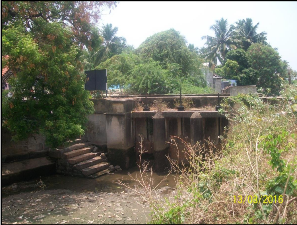
13: Kumari Dam at Chainage 14.10km
