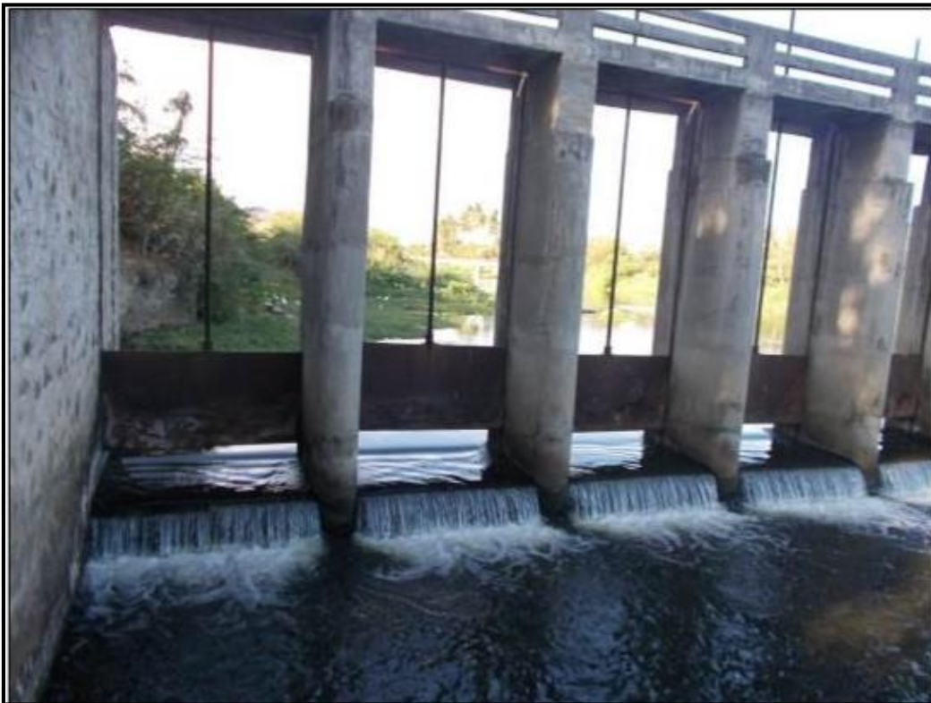
4: Karkurumbathai Shutter Dam
