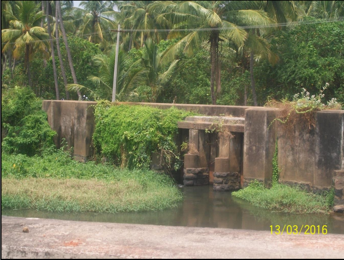
19: Diversion Works and pipeline bridge at Chainage 20km
