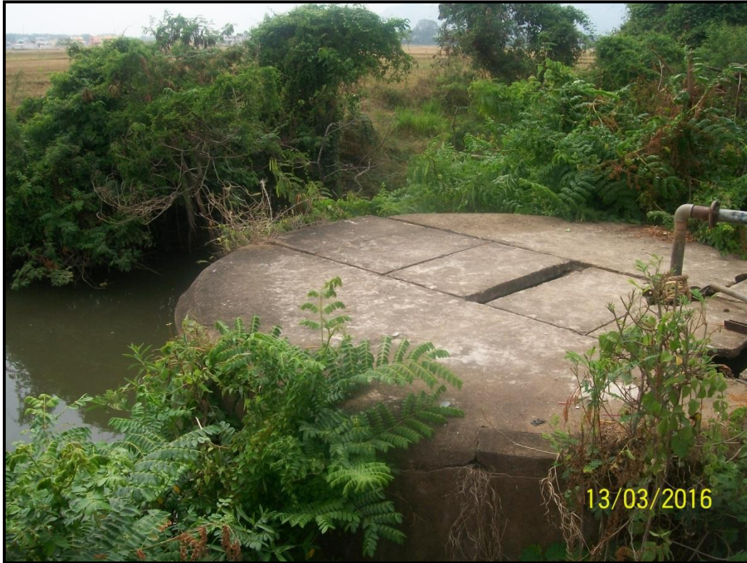
17: Water intake at Chainage 17.8km
