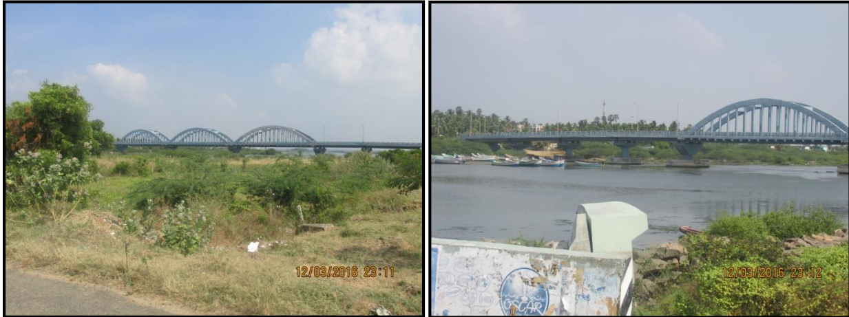
5: Keela Munakudy to Mela Mankudy Bridge at Chainage 4.9km
