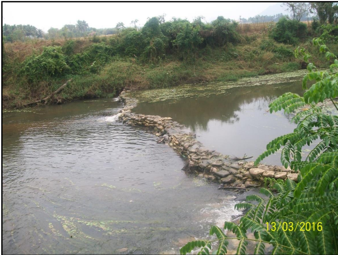
16: Local Bund at Chainage 17.8km
