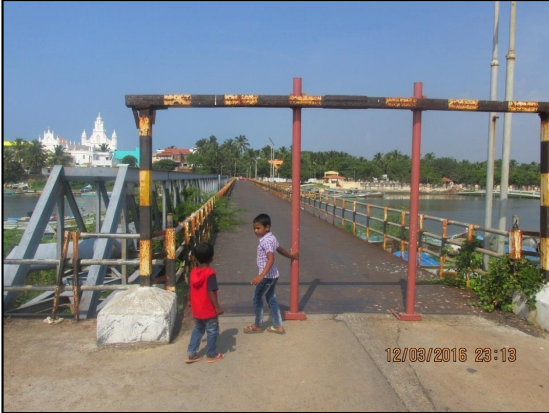
3: Old Steel Road Bridge (SH-179) along with Pipeline at Chainage 4.6km
