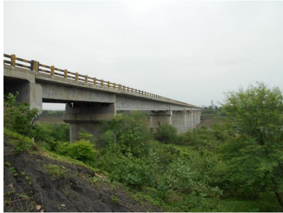
Figure 27 - Relegaon- Dewada Road Bridge (130.944 km Chainage)
