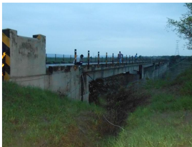
Figure 12 - Thogaon-Wirur Road Bridge (57.235 km chainage)
