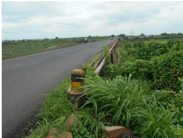
Figure 21 - Manoli Road Bridge (92.039km chainage)
