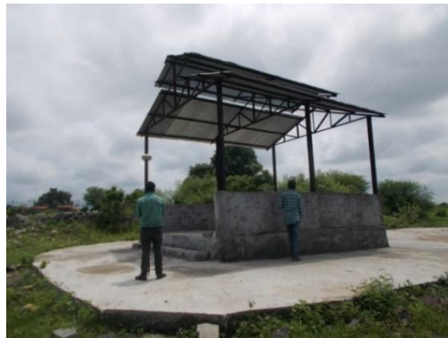
Figure 43 - Shamshan (248.708 km chainage)
