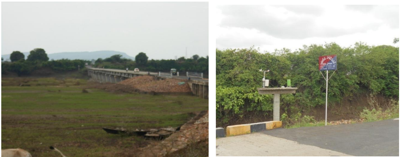
Figure 11 - Venkatraopet Road Bridge and Anemometer Station at Polsa (31.619 km chainage)
