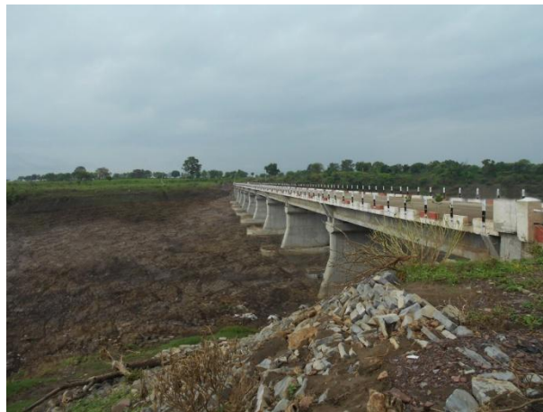
Figure 34 - Kura Road Bridge (187.823 km chainage)
