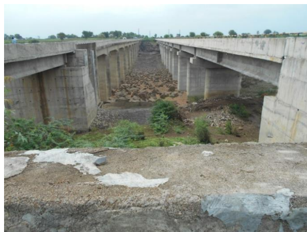
Figure 35 - Dollara Road Bridges (198.910 km chainage)
