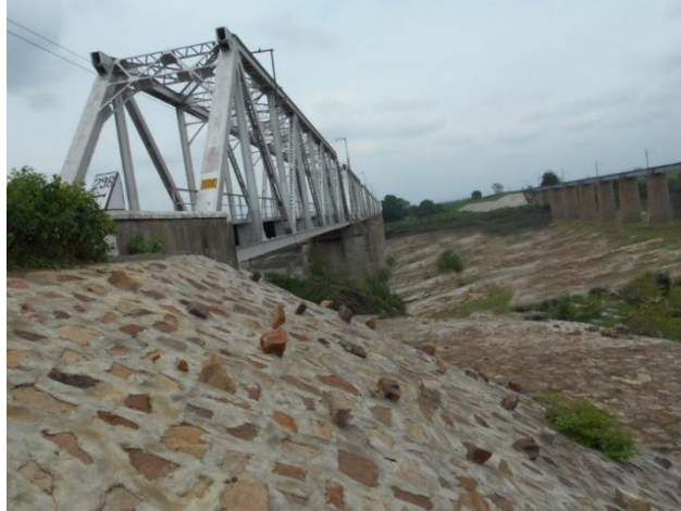
Figure 17 - New and Old Railway line (87.6 km chainage)
