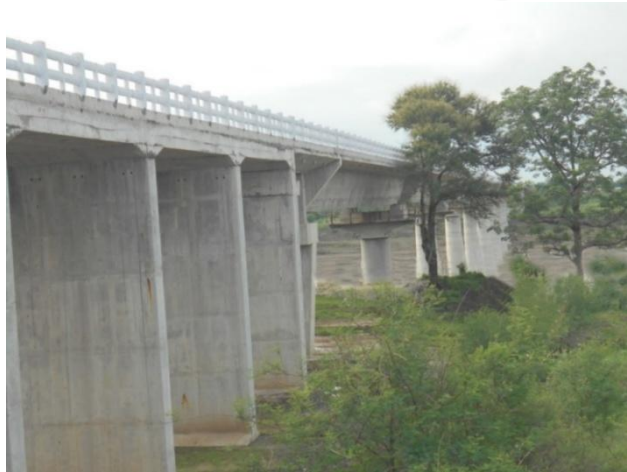
Figure 22 - Wardha Hadasti Road Bridge-MDR -41(100.763 km chainage)
