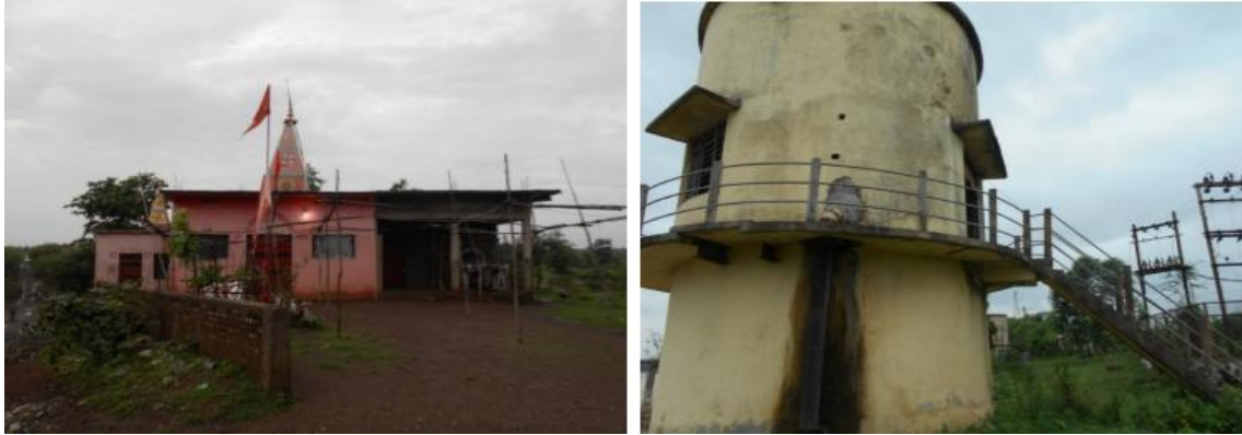
Figure 29 – Temple (138.252 k m chainage) and Pump House (139.458 km chainage)
