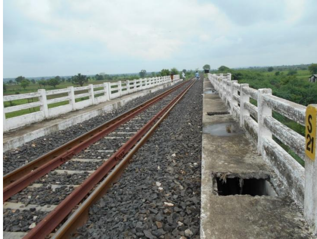
Figure 36 - Kodari Railway line Bridge (201.841 km chainage)
