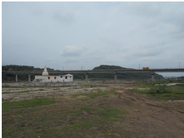
Figure 16 - Mancherial- Nagpur Road Bridge (87.054 km chainage)
