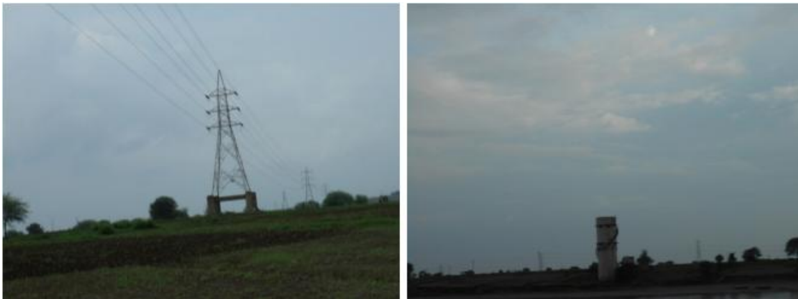
Figure 24 - Features in Stretch 4 (HTL at 114.386 km Chainage and water tank at 98.249 km chainage)
