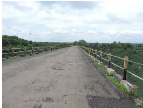
Figure 42 - Unkeswar Road Bridge (248.753 km chainage)
