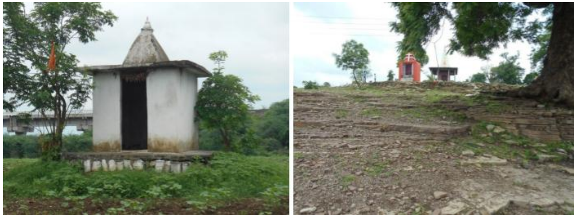
Figure 37 – Temples at 201.365 km and 207.023 km chainage)
