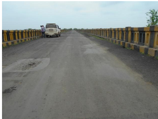
Figure 28 - Bori Road Bridge (139.488 km chainage)
