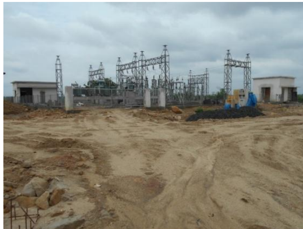
Figure 18 - Irrigation Plant under construction (83.348 km chainage)
