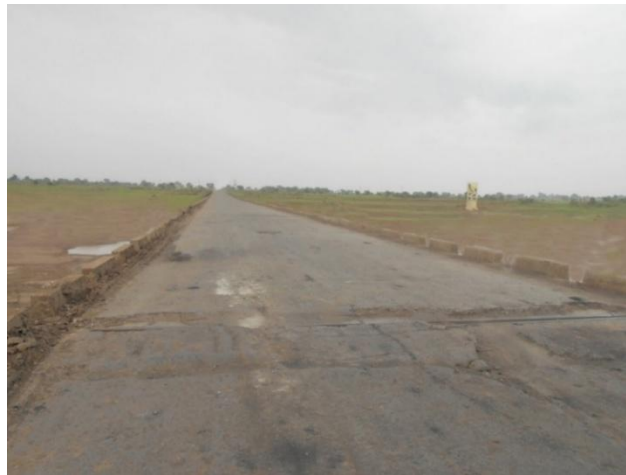
Figure 23 - Penganga Road Bridge (112.899 km chainage)
