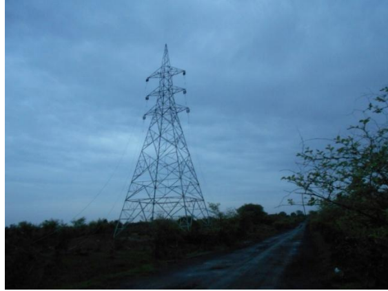
Figure 13 - Power Transmission Line under constructions (57.151 Km chainage)
