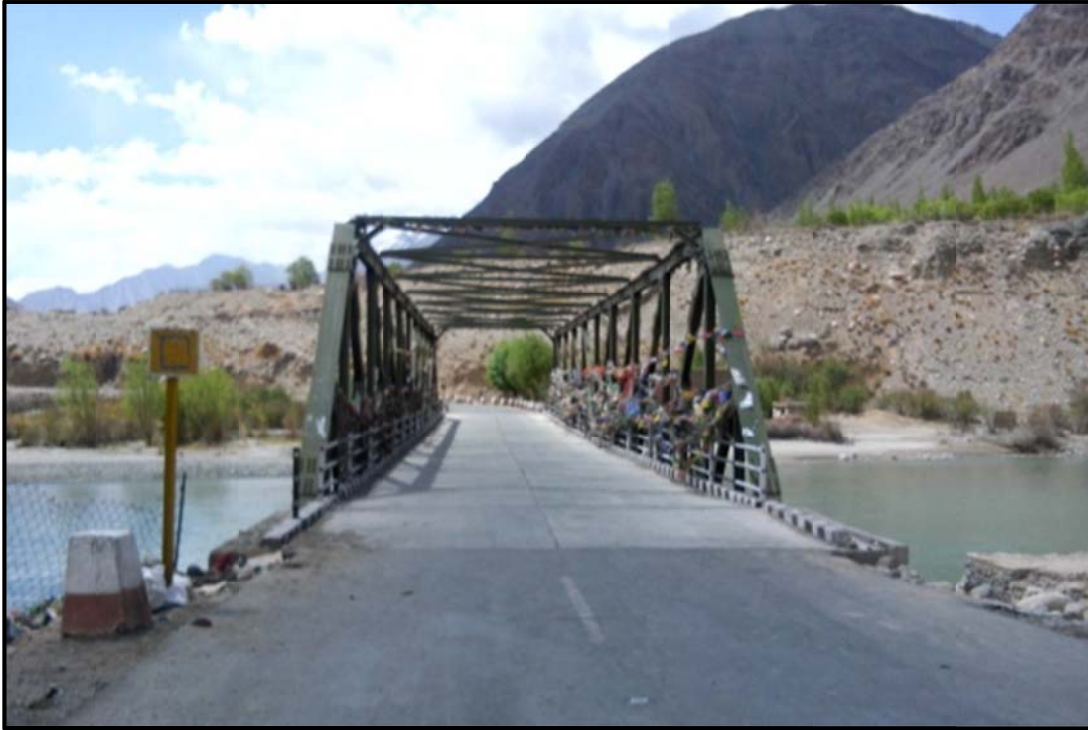
Figure 23 – Ch- 34.672 Km Upshi Bridge
