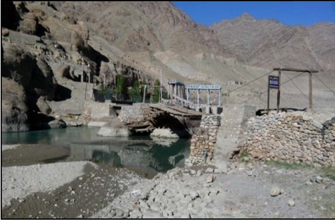
Figure 21 – Ch. – 27.60 Km Water Controlling Gate and Wooden
