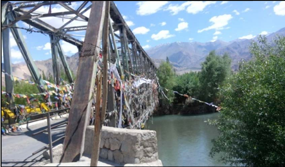
Figure 7 – Ch.0.00 Km Shashe Bridge on Shey Chuchot Road at Shey Village
