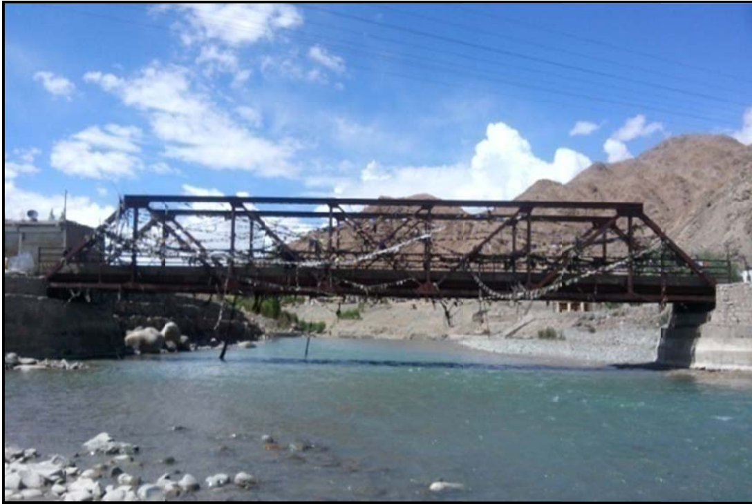
Figure 17 – Ch. 19.83 Km Karu Bridge
