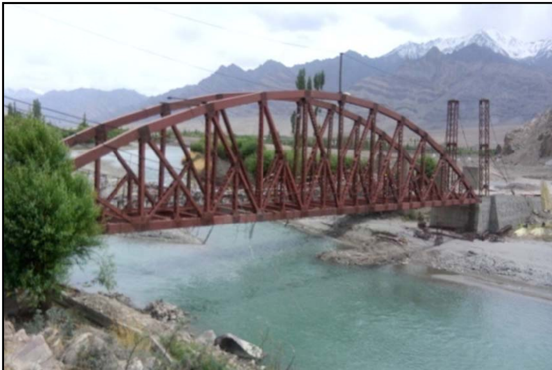
Figure 10 – Ch.8.11 Km Stakna Village Bridge
