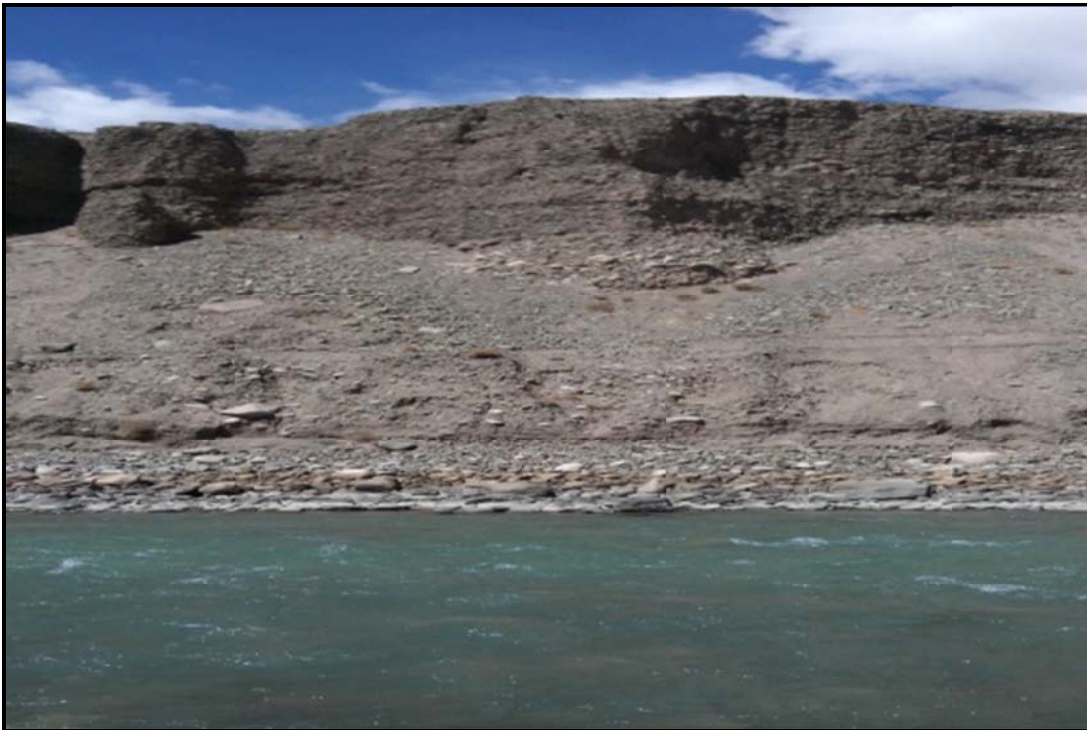
Figure 22 – Ch.- 289.90 Km River Bank
