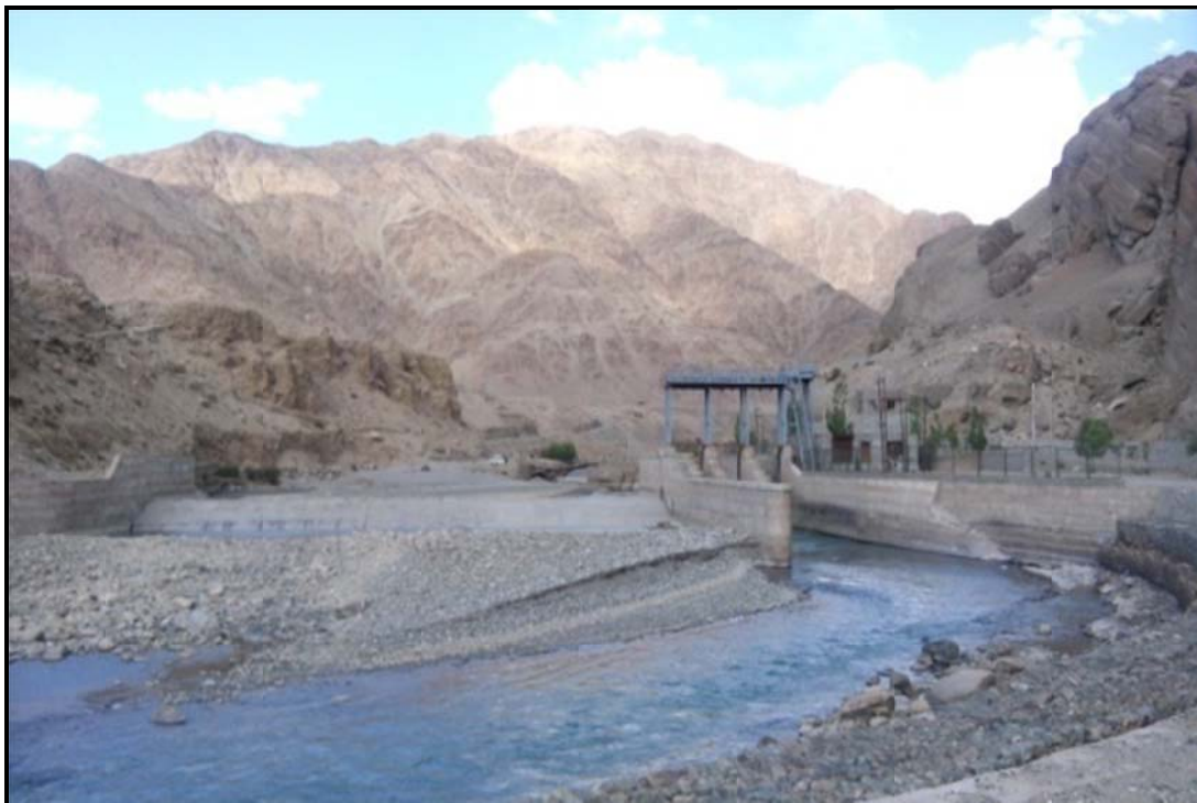
Figure 18 – Ch.- 26.80 Km Water Controlling Gate
