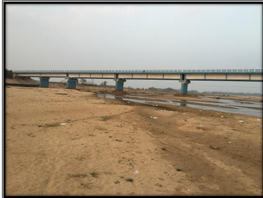
MAJOR ROADWAY BRIDGE CHAINAGE 41.9 KM
