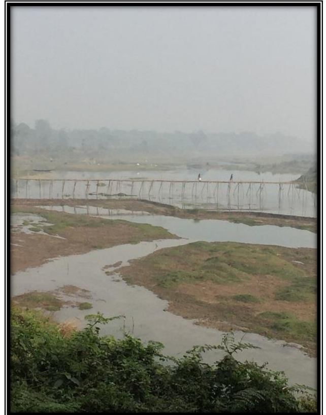
BAMBOO BRIDGE CHAINAGE 93.8 Km
