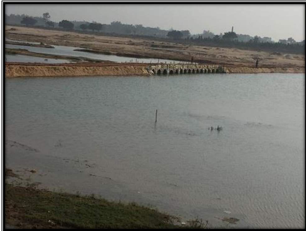
SAND CHECK DAM ALONG WATERWAY
