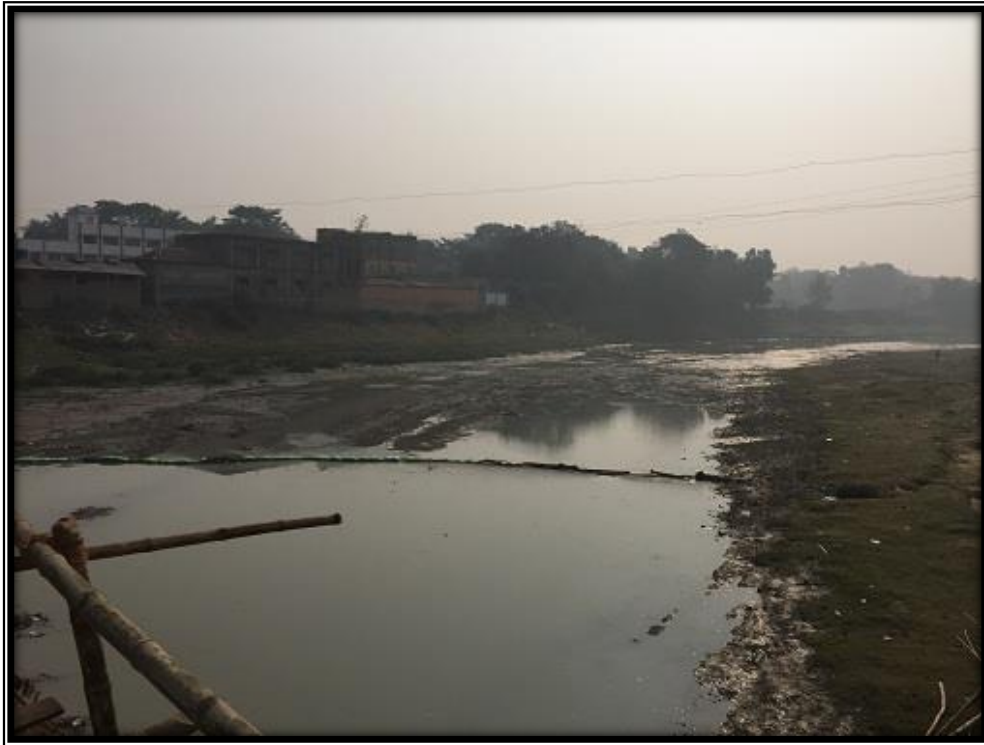
SAND CHECK DAM ALONG WATERWAY
