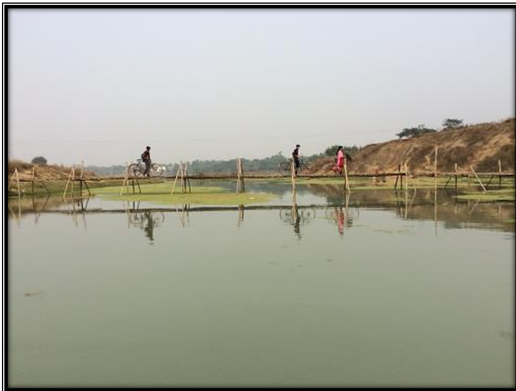
WOODEN BRIDGE CHAINAGE 84.3 Km
