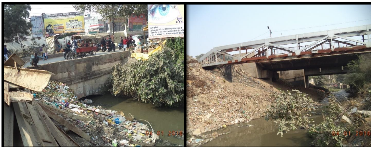
Culvert at Ch. 1.40 km & Ch. 1.60 km
