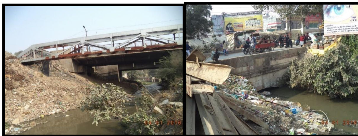
Culvert at Ch. 1.44 km & Ch. 1.62 km
