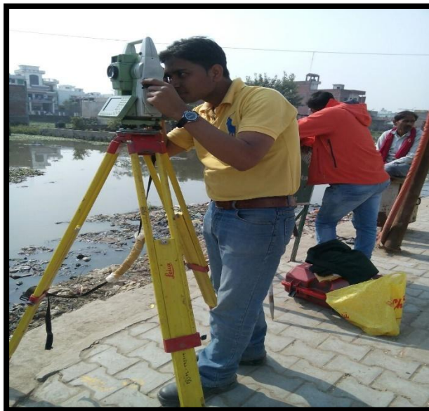
Topographic Spot Levelling by Total Station Leica
