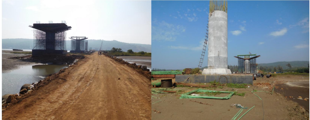
FIGURE 4-8: Upcoming bridge at the mouth of Savitri river
