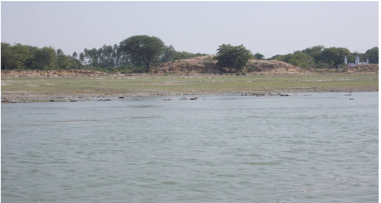
(Image: Prithivipur Collapse Bank)
