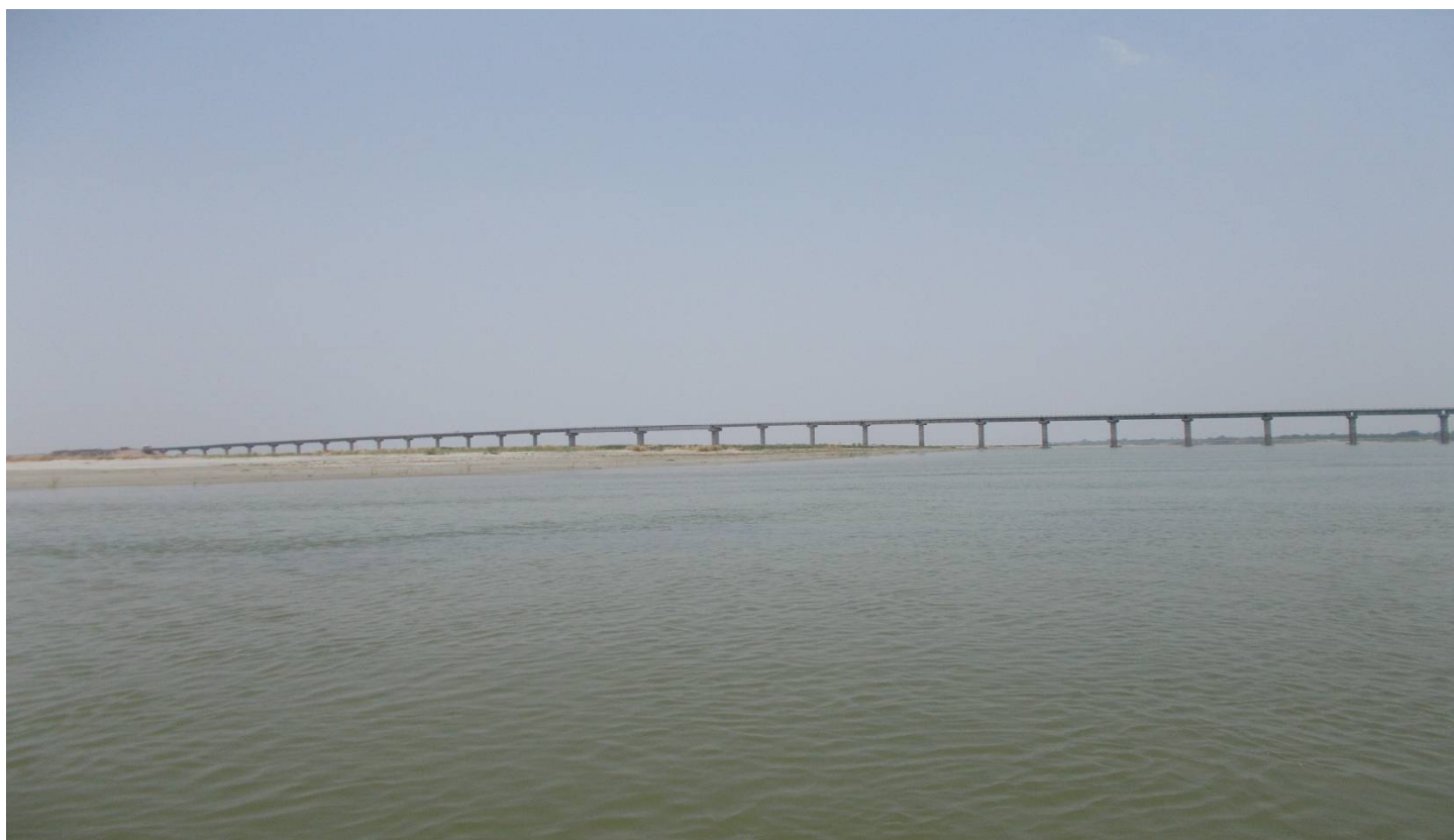
(Image: Bidhar Ghat Road Bridge)
