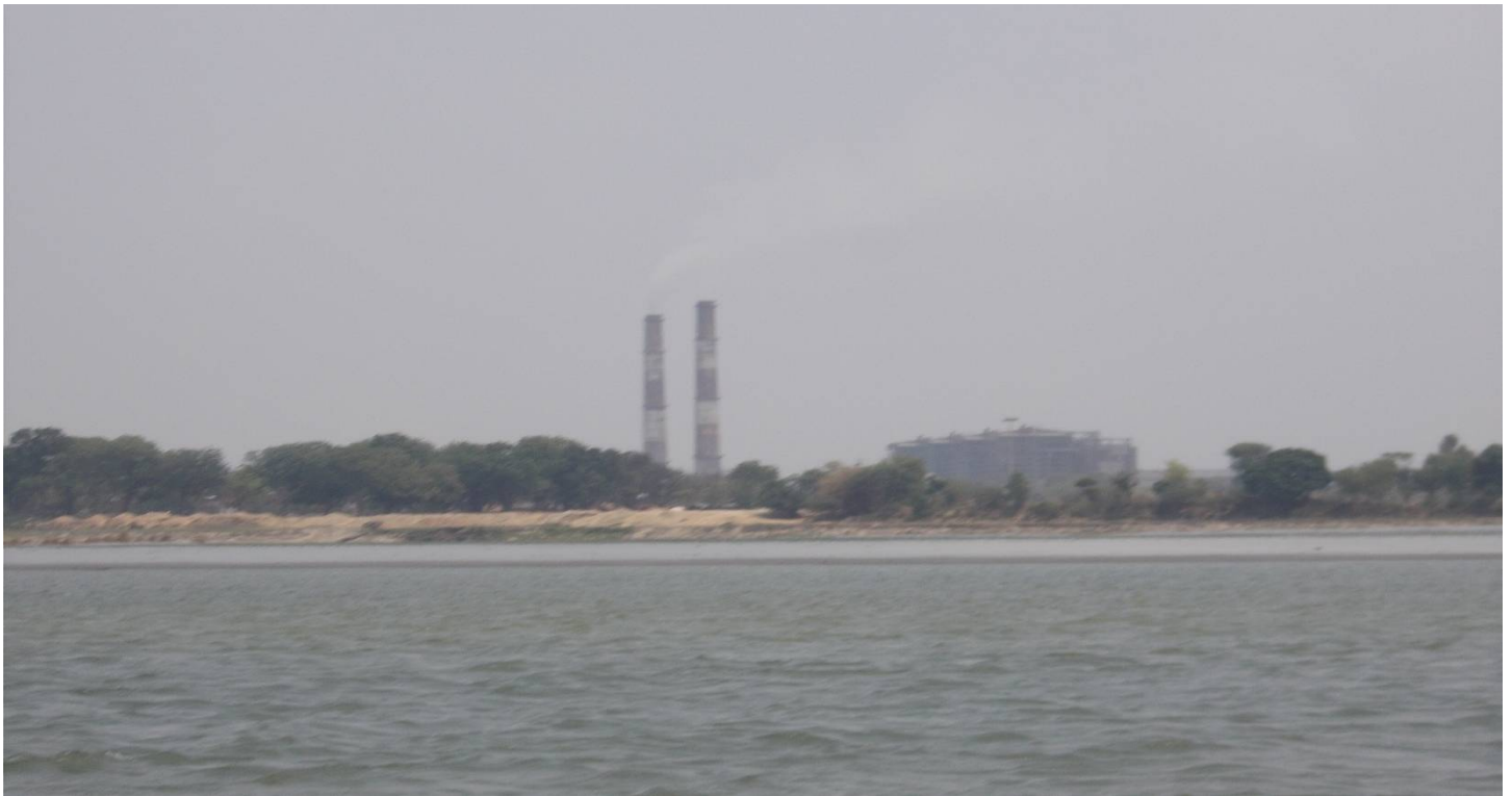
(Image: NTPC Power Plant At Tanda)
