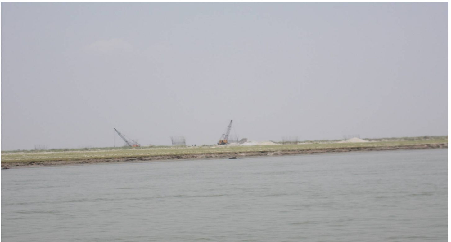
(Image: Kamaria Road Bridge Under Construction)
