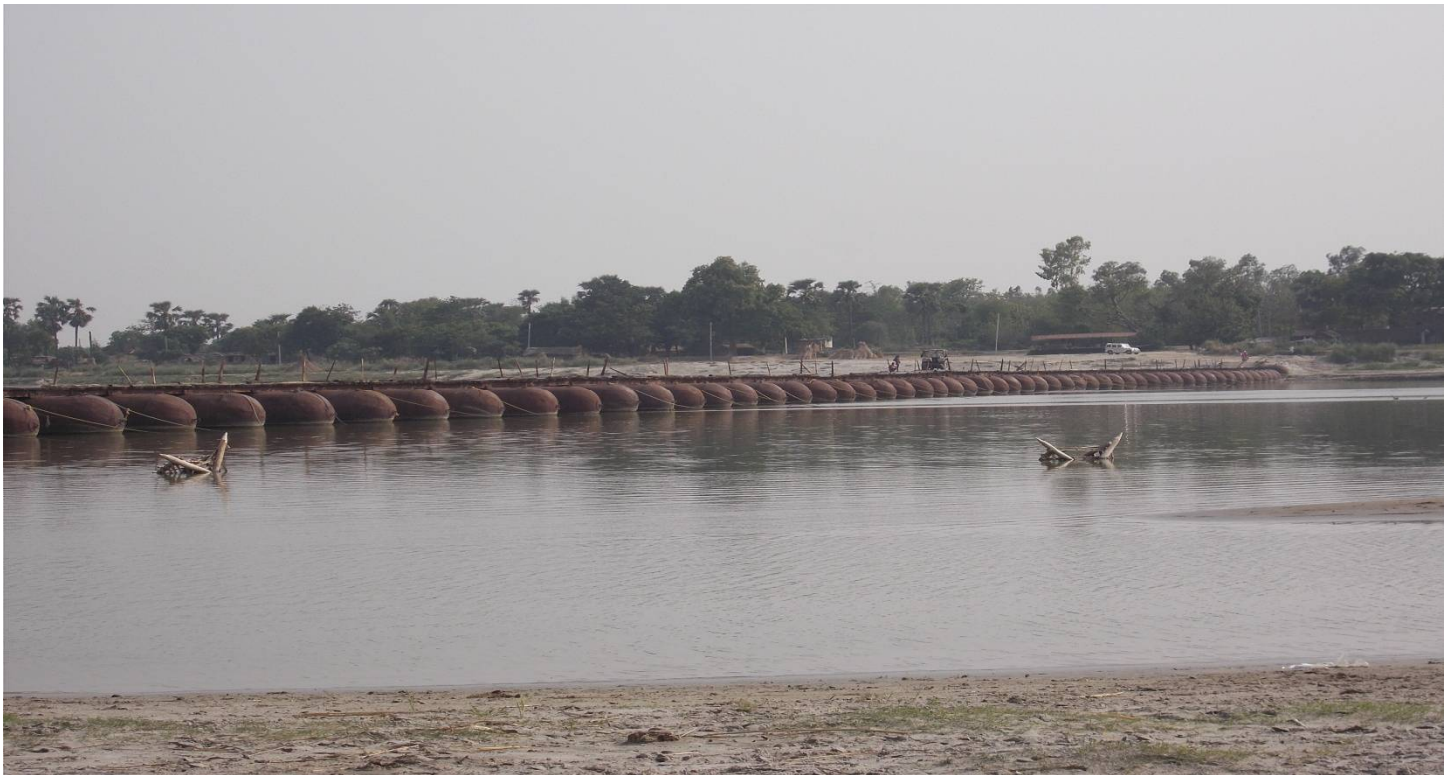
(Image: Kamariya Pipe Bridge)
