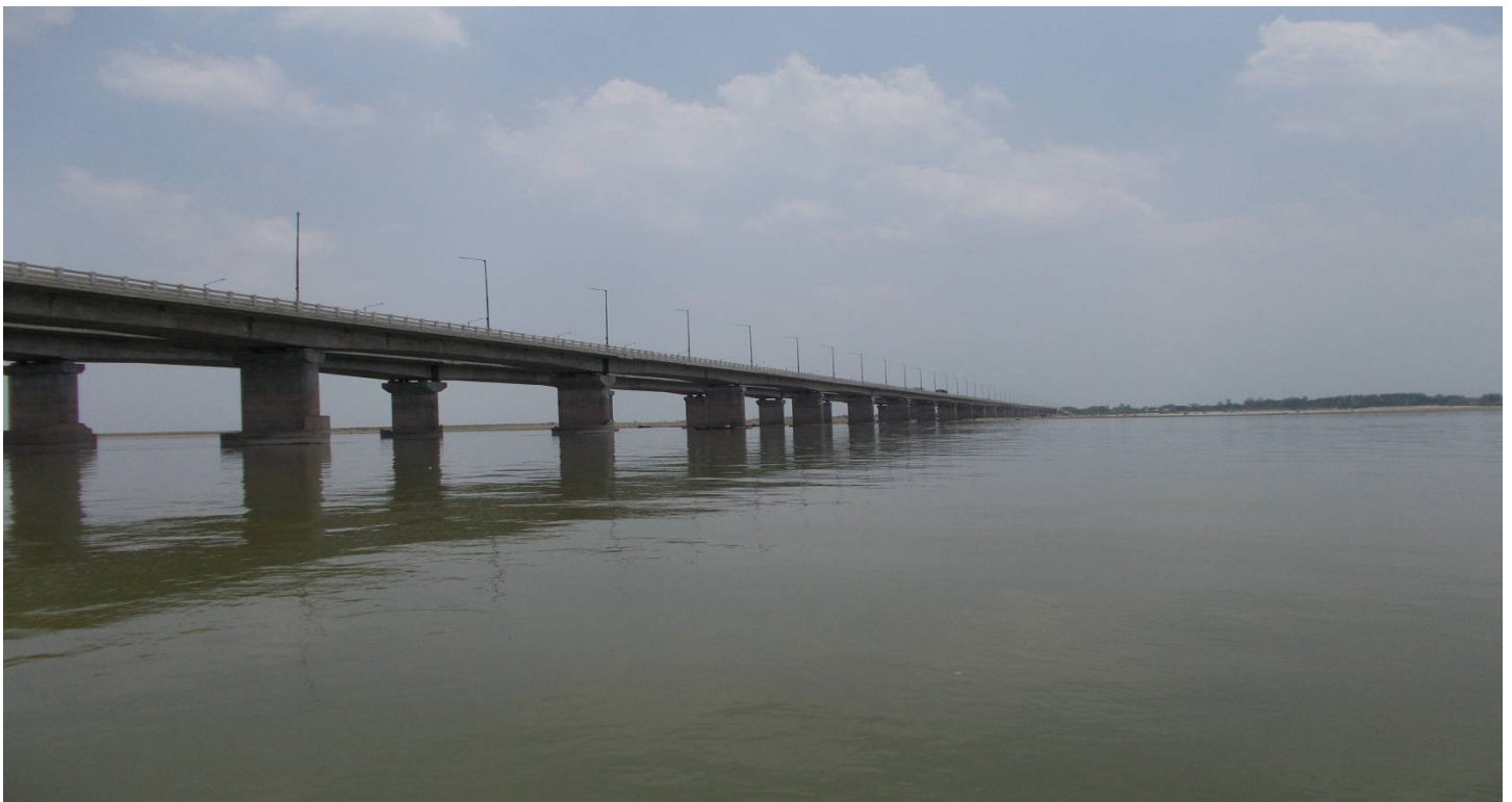
(Image: NH 28 Road Bridge)
