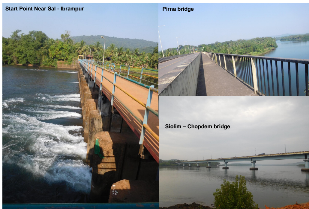
FIGURE 4-9 Existing bridges on river
