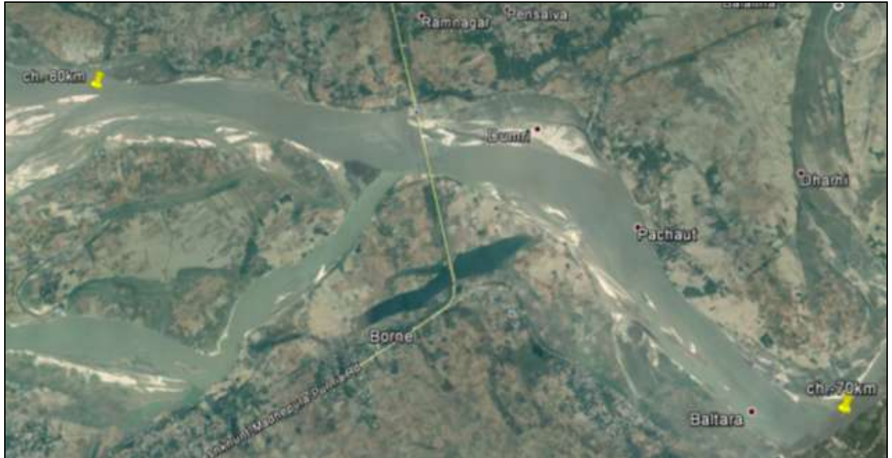
Figure 21- Chainage 70.000 Km. to Chainage 80.000 Km.
