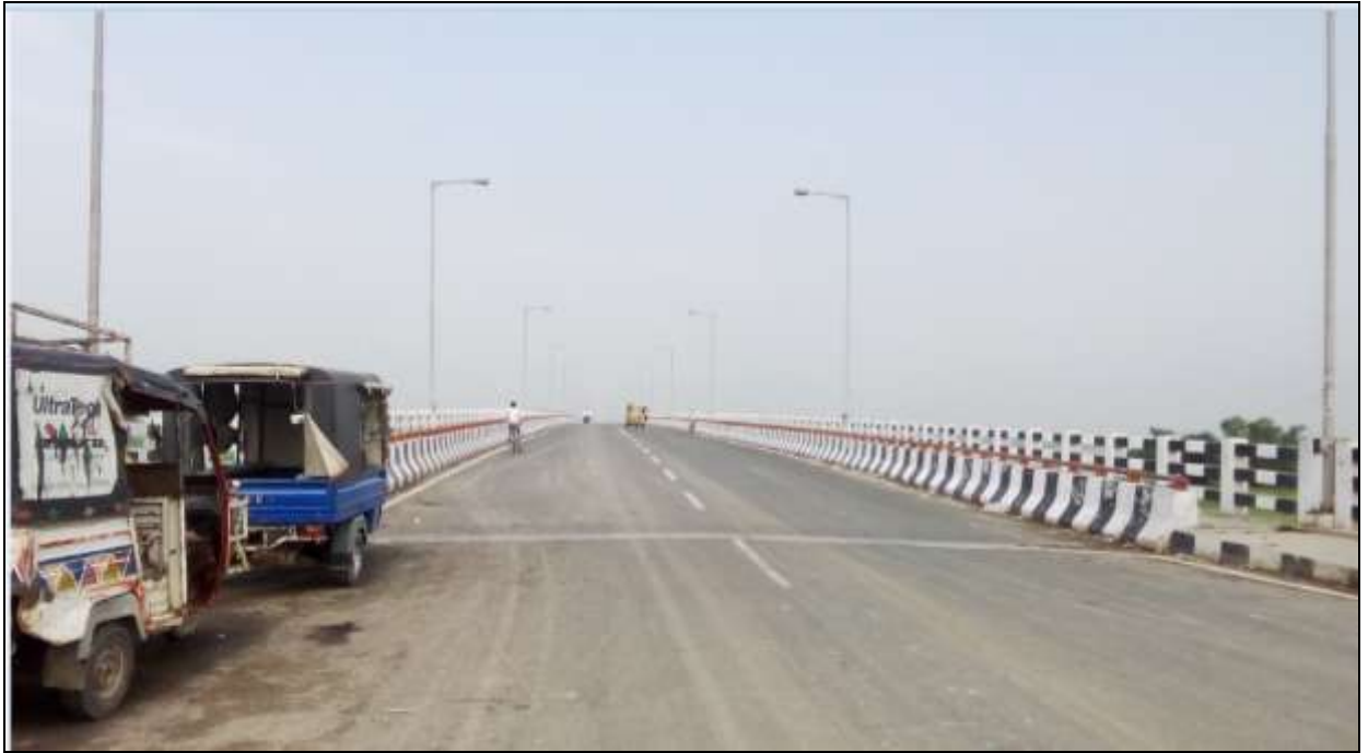
Figure 31- RCC Bridge (Chainage-131.036 km)
