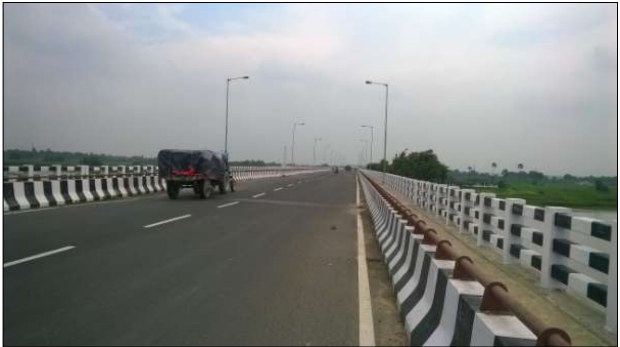
Figure 22- RCC Bridge (Chainage-75.732 km)
