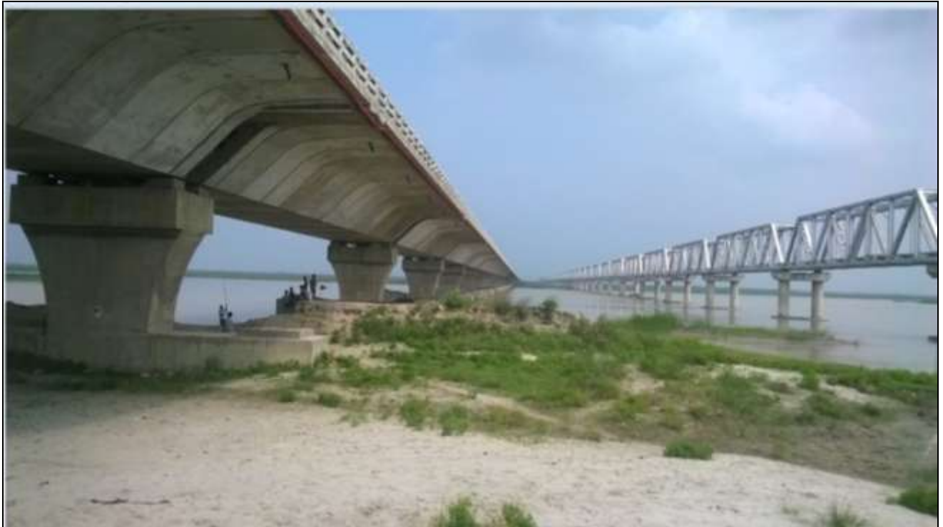
Figure 37- Under Construction Rail Bridge and RCC Bridge (Chainage- 189.100 km and 189.163 km)
