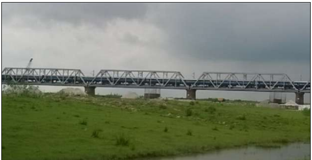
Figure 13- Rail Bridge at Patthar Tala (Chainage- 1.724 km)
