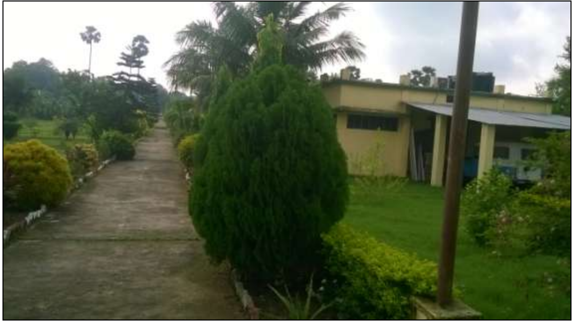
Figure 9- C.W.C office near the Kosi Barrage
