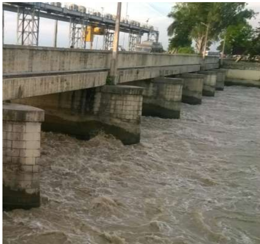
Figure 76- Kosi Barrage view (Chainage-233.040 km)
