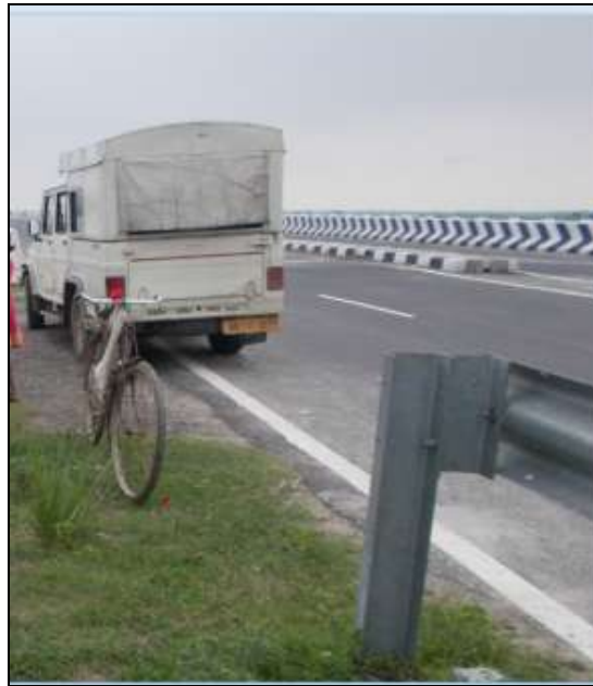
Figure 16- RCC Bridge (Chainage- 27.566 km)
