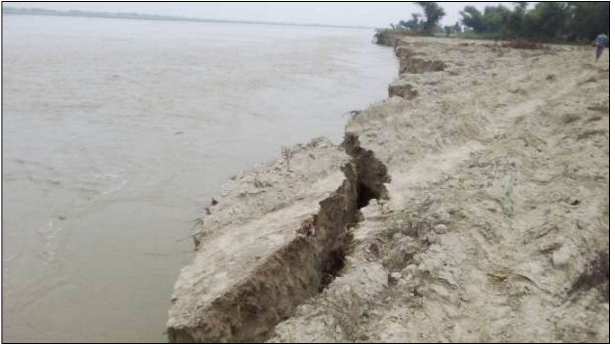
Figure 84- River bank erosion
