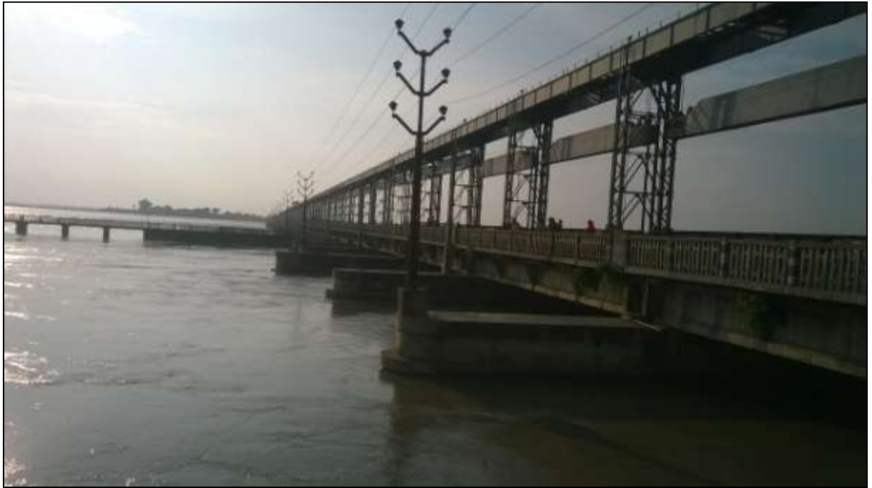
Figure 42- Kosi Barrage (Chainage-233.040 km)
