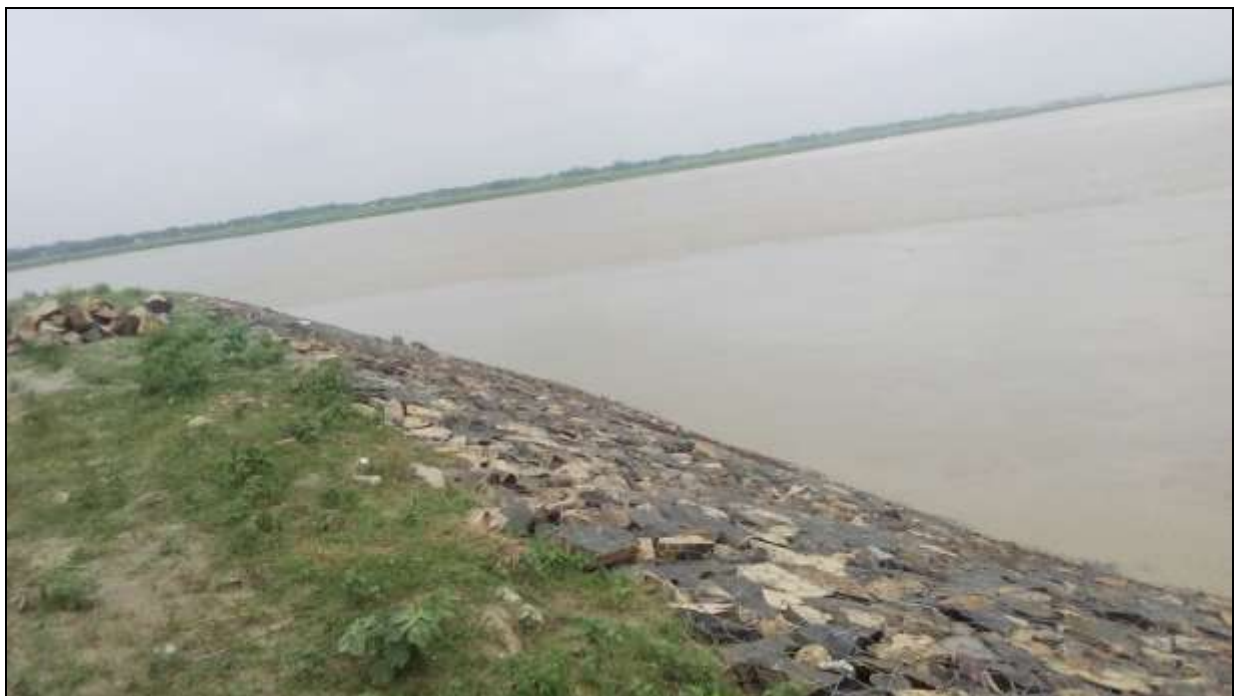
Figure 83- Boulder pitching protect the river side
