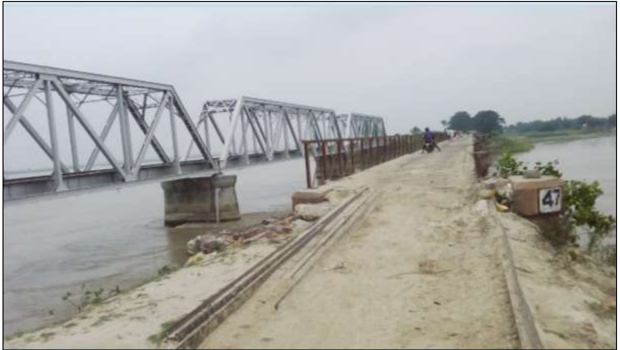
Figure 25- Fungo Rail Bridge and RCC Bridge (Chainage-90.325 km and Chainage 90.294 km)
