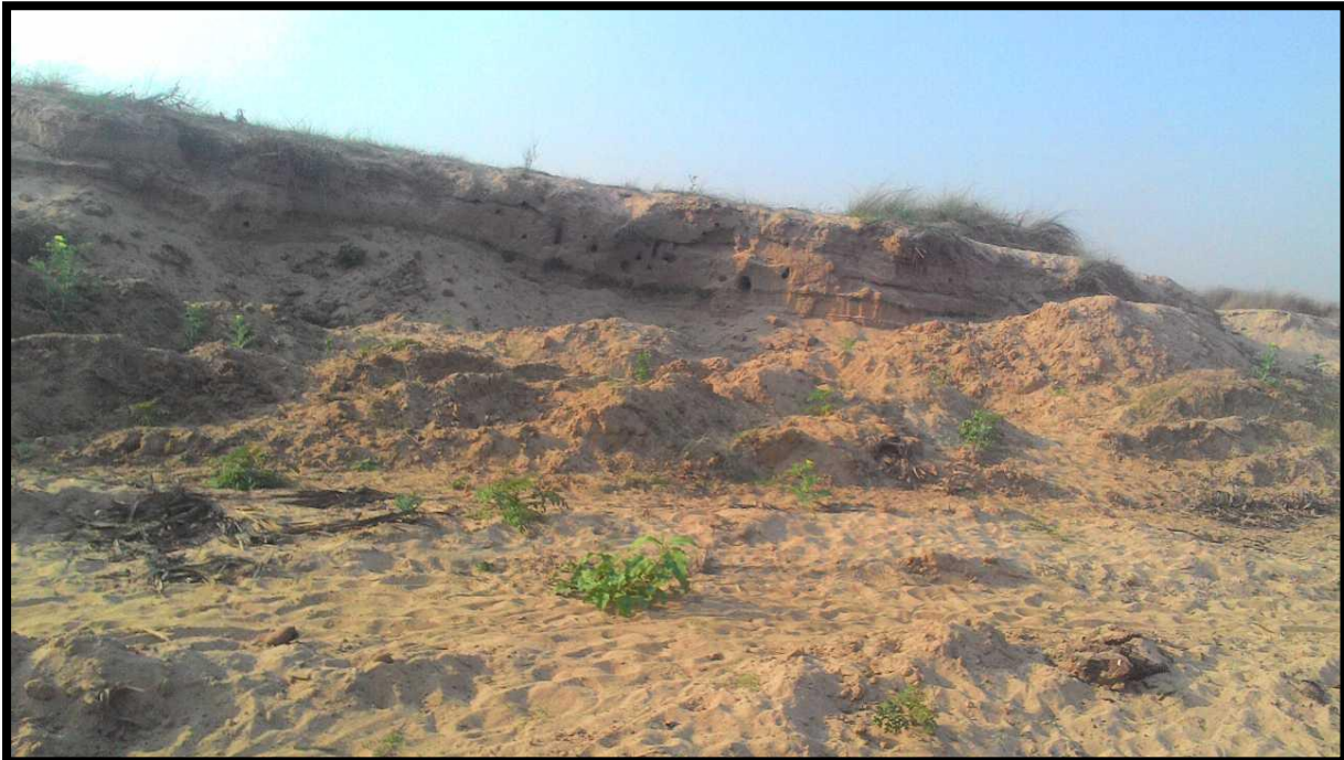
Unprotected Bank at Chainage 11.0
