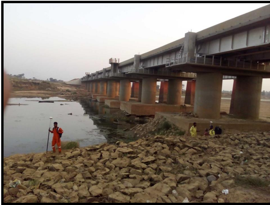
Bridge Under Construction at Chainage 6.5
