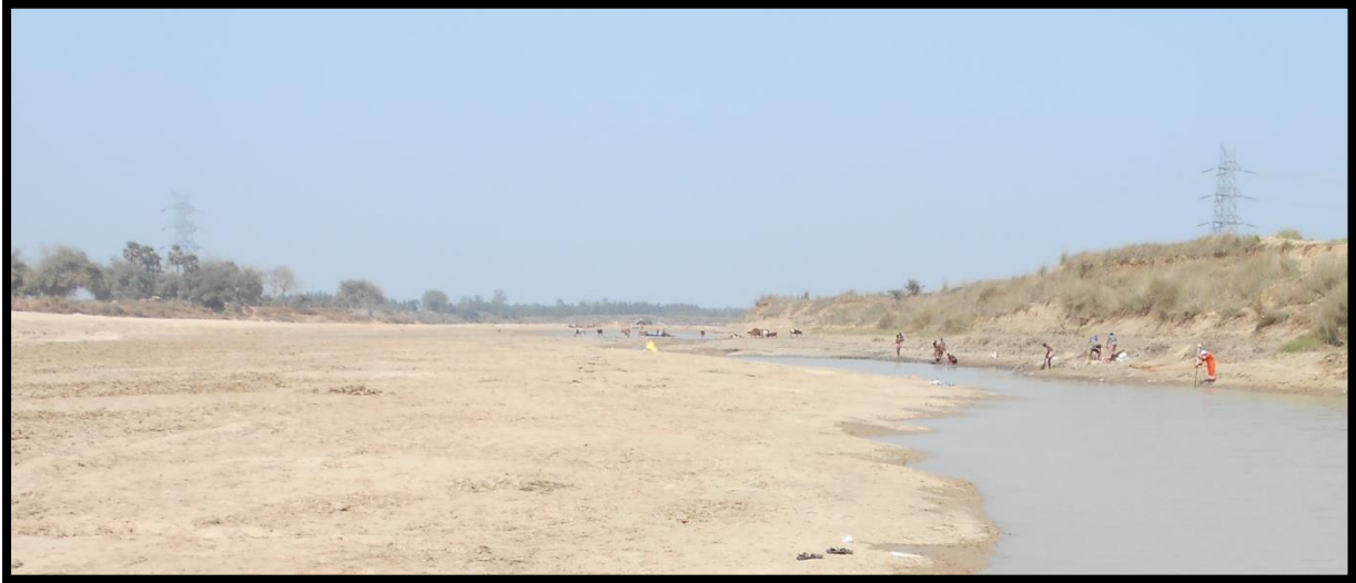
High tension Crossing at Chainage 13.9
