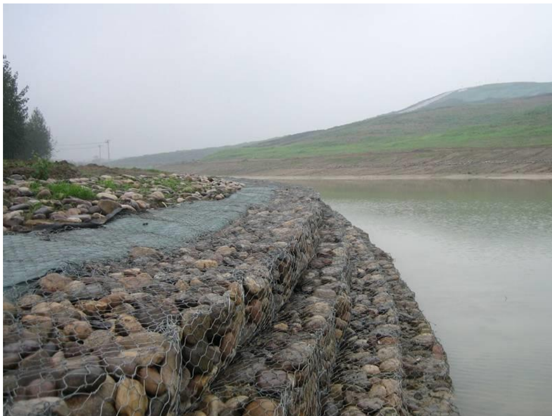
Figure 15: Photograph showing arrangement of Gabion Wall along River Bank
