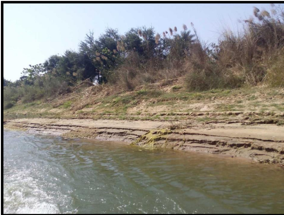
River Bank Chainage 2.3
