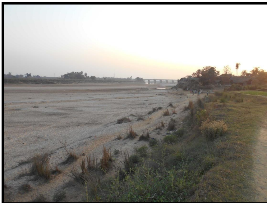
Dry area of Ajoy River at Chainage 6.0 and Road Bridge at 6.5
