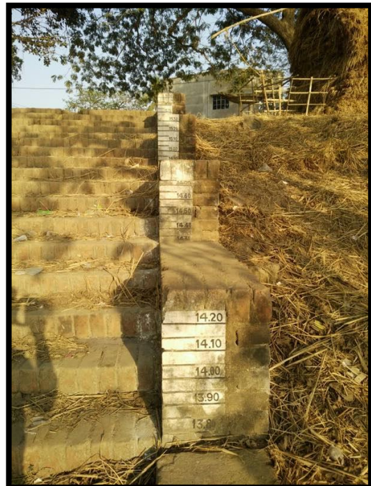
Irrigation Tide Gauge at Katwa
