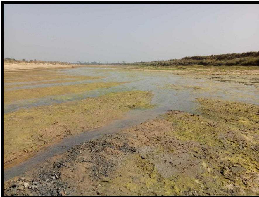
River Condition at Chainage 7.0
