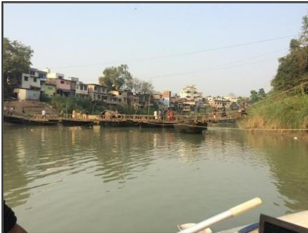
WODDEN BRIDGE GHATAL CHAINAGE-6.50 KM
