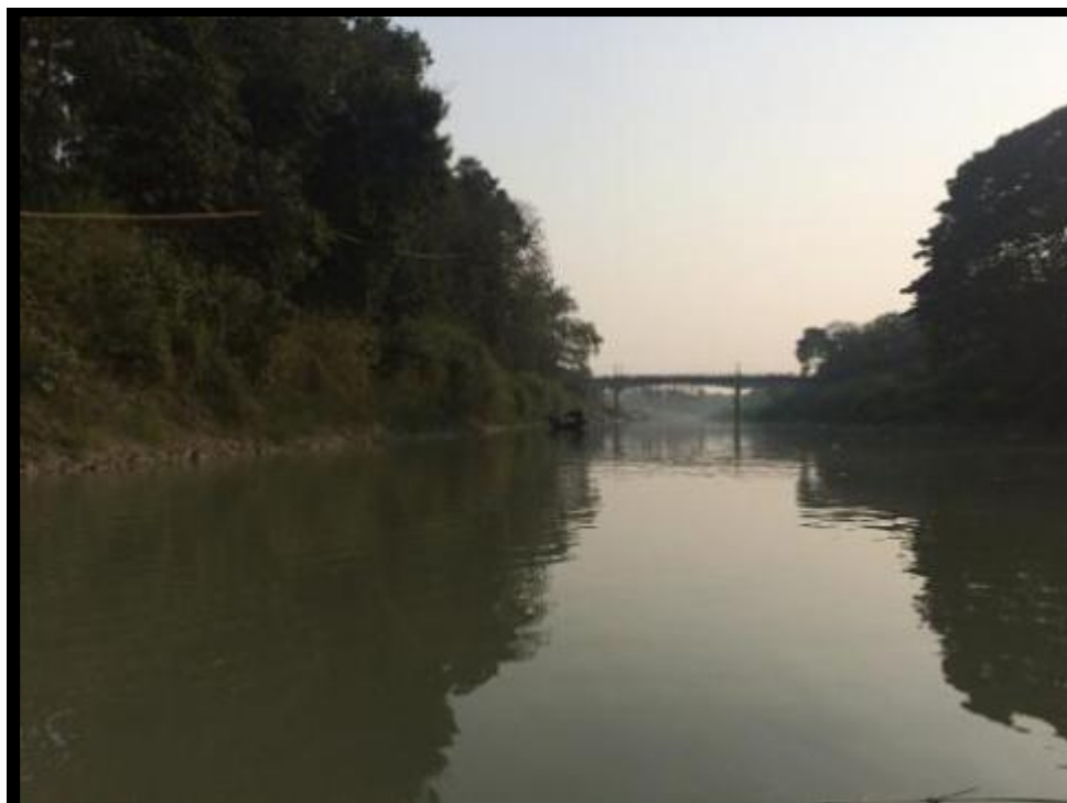
GHATAL BRIDGE CHAINAGE-6.2 KM
