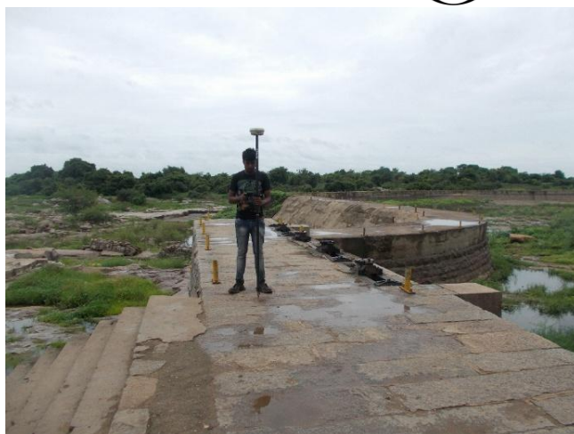
Figure 28 - Edupayala Check dam (147.25km Chainage of Manjira River)
