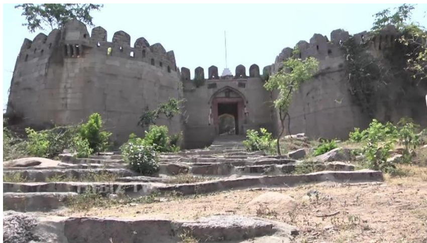
Figure 41 - View of Medak Fort (139.0 km chainage)
