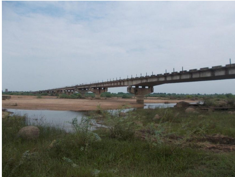
Figure 7 - View of Kandakurthi Bridge (-0.51 km chainage)
