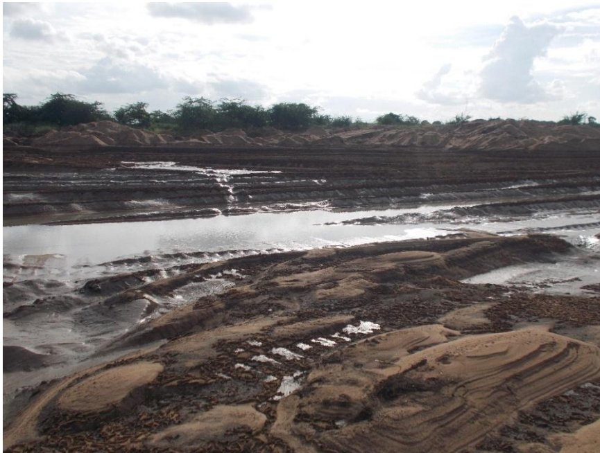
Figure 11 - Sand mining area (17km to 23km chainage area)
