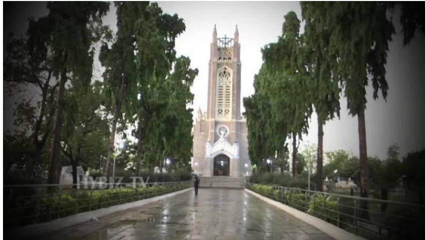
Figure 42 - View of Medak Church (138 km chainage)
