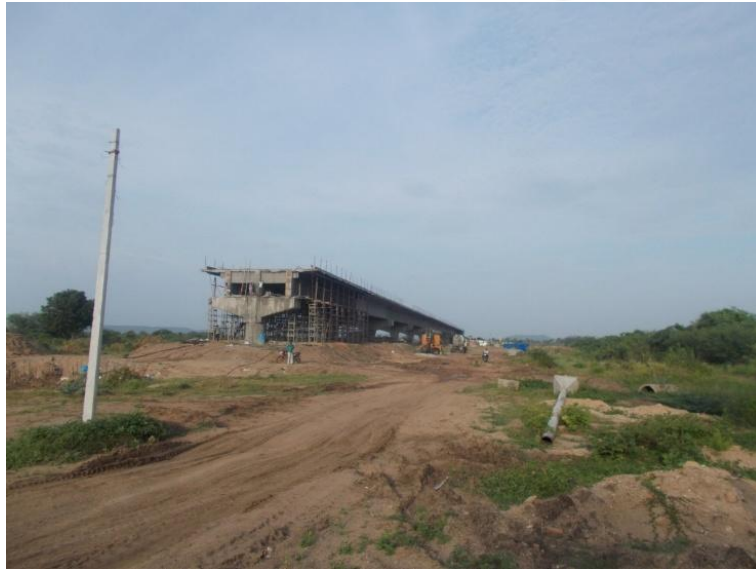
Figure 14 - Bridge under construction near Khatagaon (49.77km Chainage)
