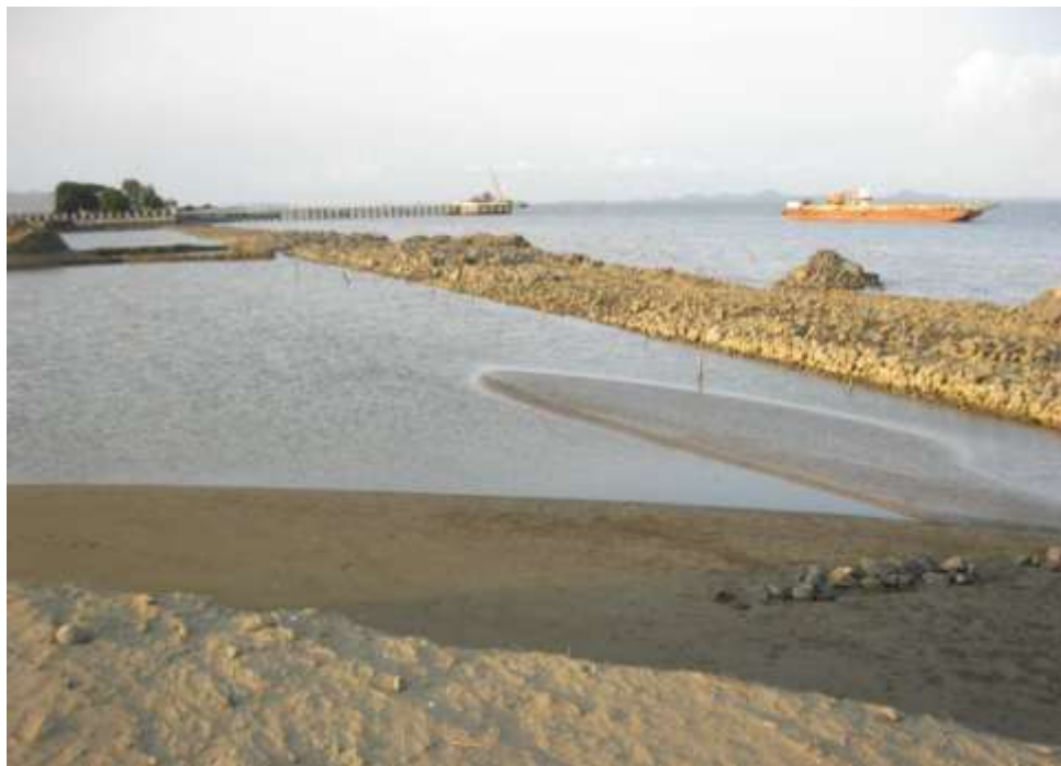
Construction of Dyke & reclamation work in progress at Sittwe
