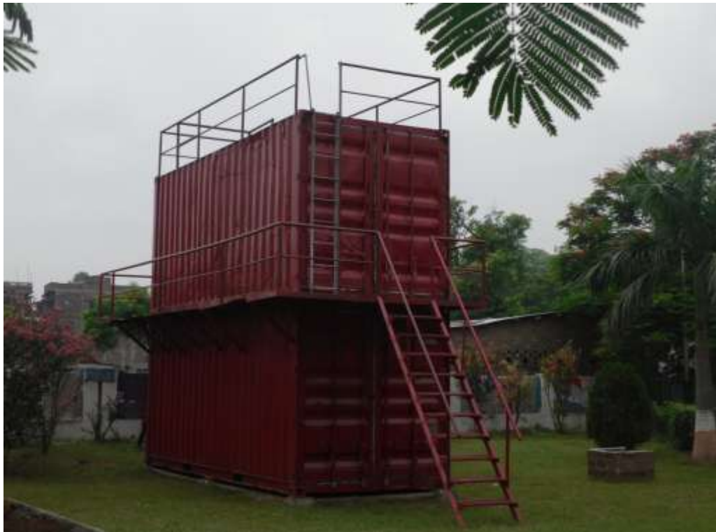
Fire Mock Up for conducting FPF Course
