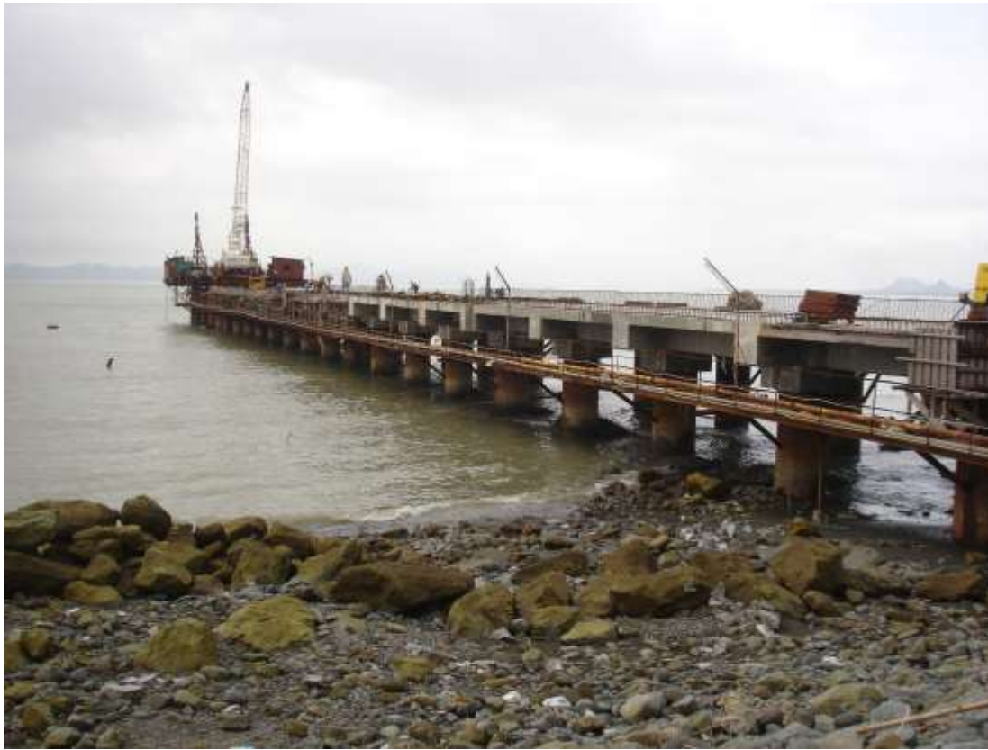
Construction of approach trestle to the Jetty in progress
