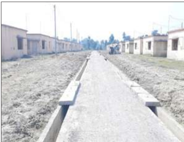
Construction of Road in Resettlement colony, Sahibganj
