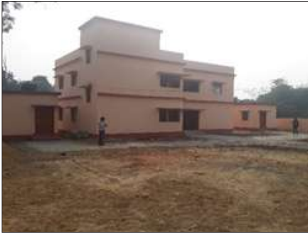
Construction of Primary School in Resettlement Site at Sahibganj
