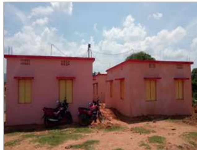
Construction of Houses in Relocation Site at Sahibganj
