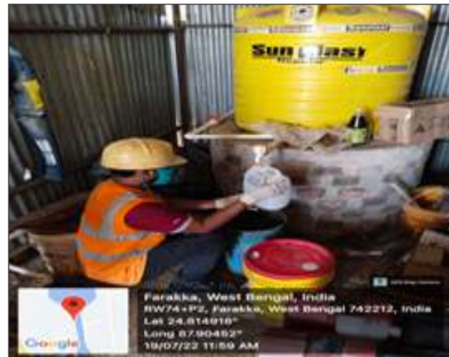
Drinking Water Monitoring at project site (New Navigational Lock Farakka)
