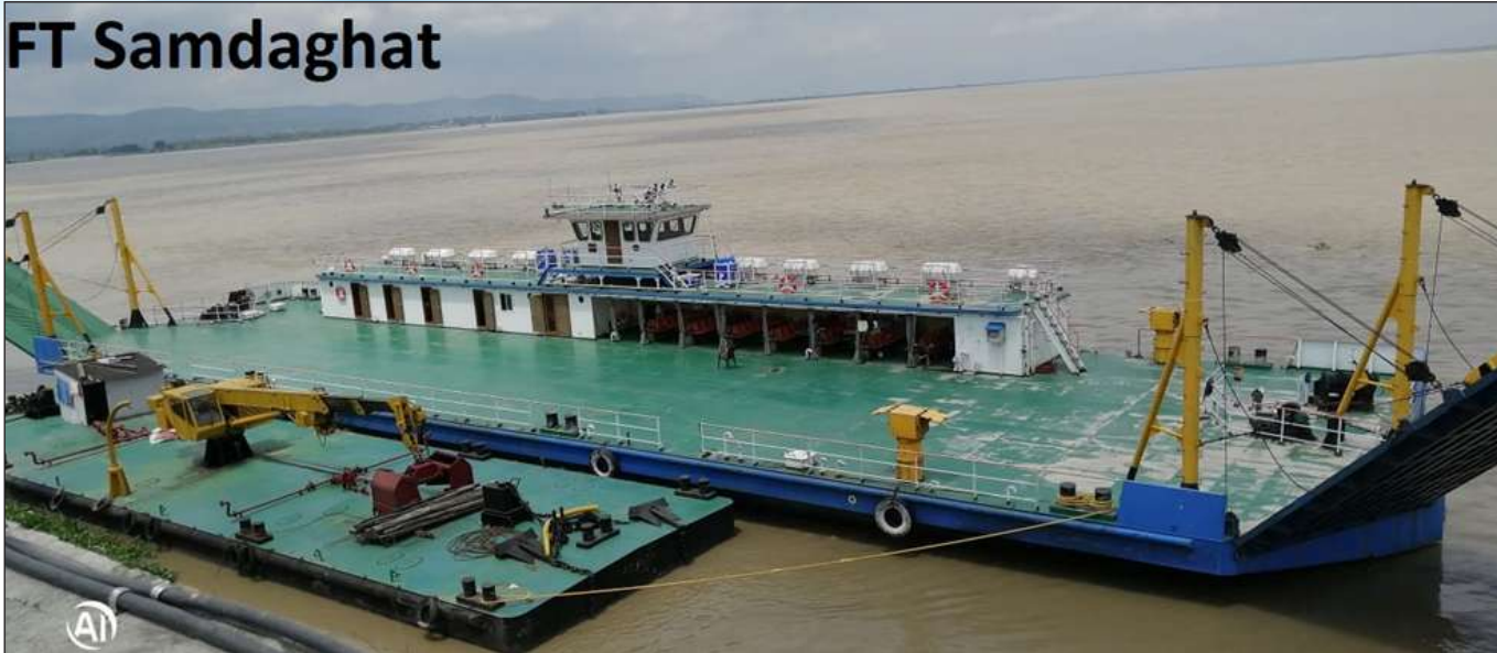
Floating terminal on NW-1
