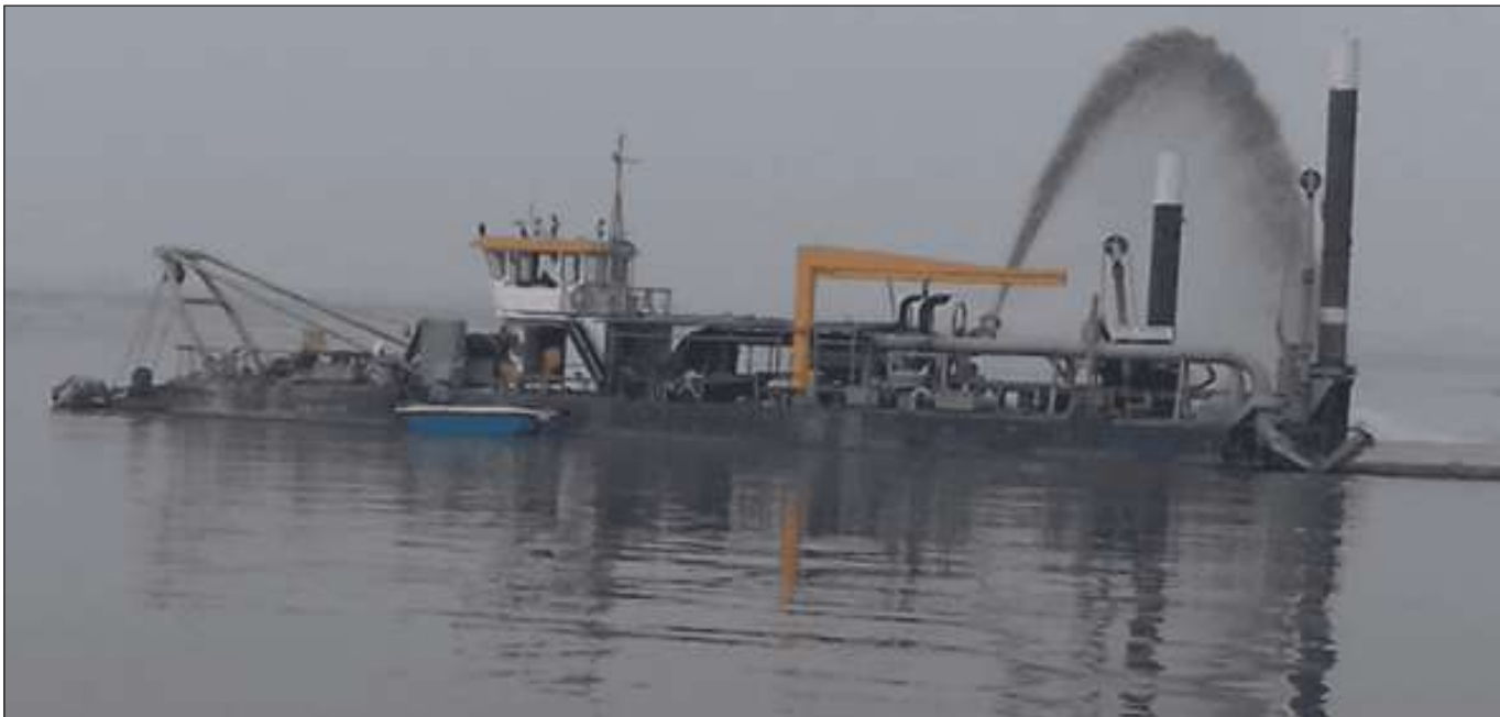
Dredging in progress on NW-1
