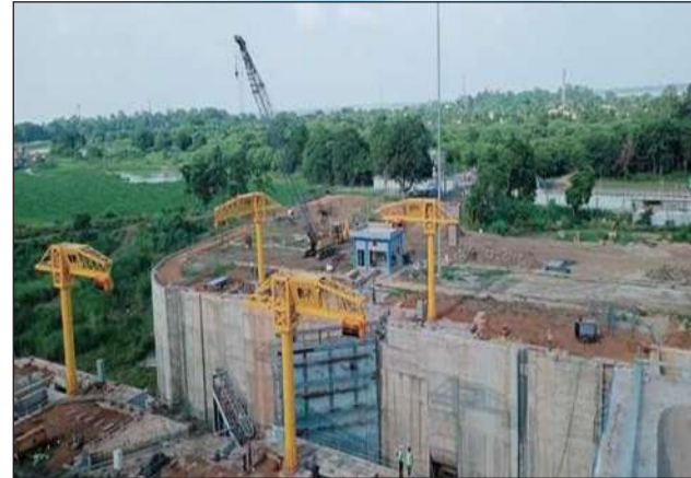
Navigational Lock Farakka under construction
