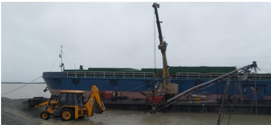
Figure 27- NW-2: Loading operations at Dhubri jetty
