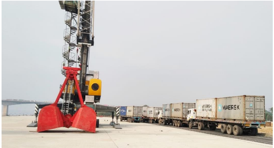
Figure 3- NW-1: Multimodal Terminal at Varanasi
