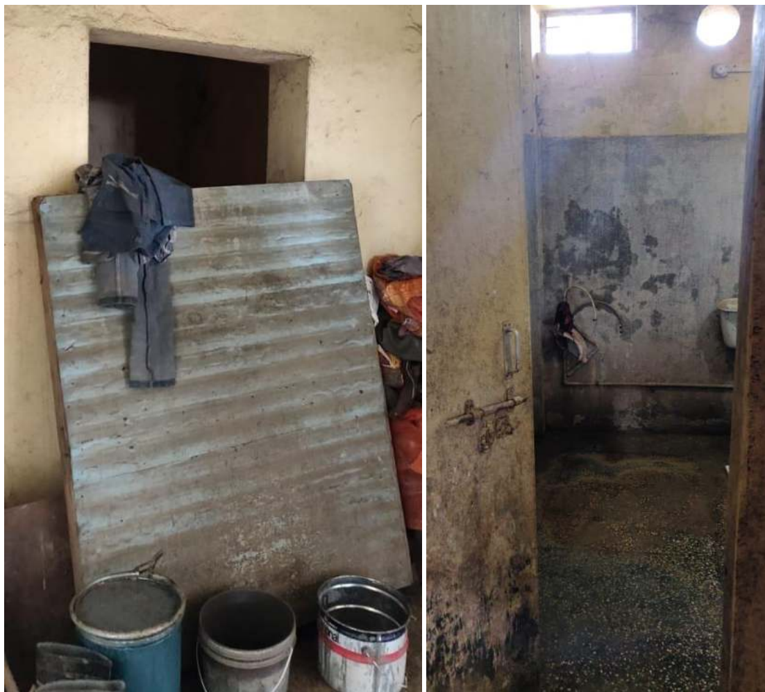
Figure 64: Present Condition of interiors of Control room building
