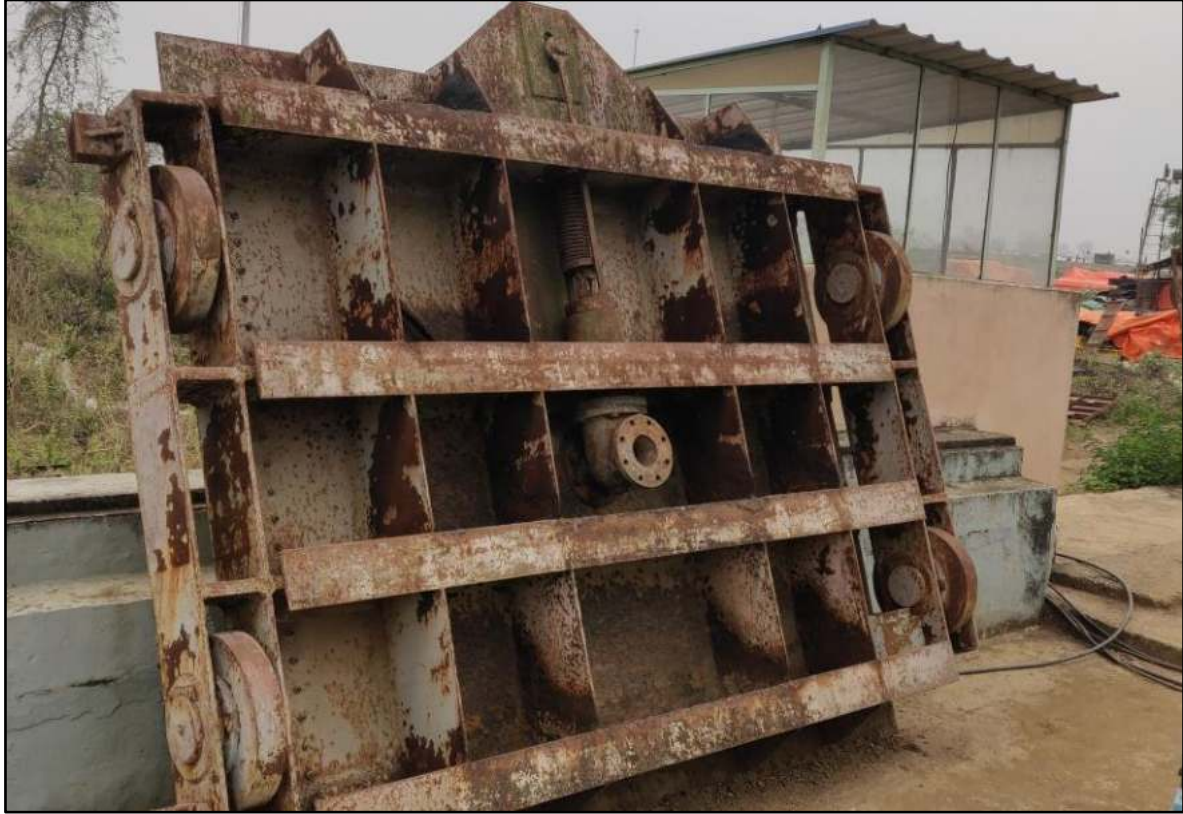
Figure 54: Bulkhead Gates for Radial Gate Maintenance
