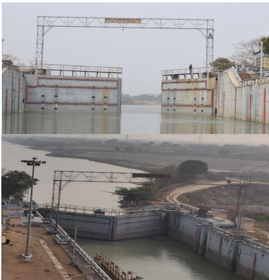
Figure 65: Steel lattice type cable bridges
