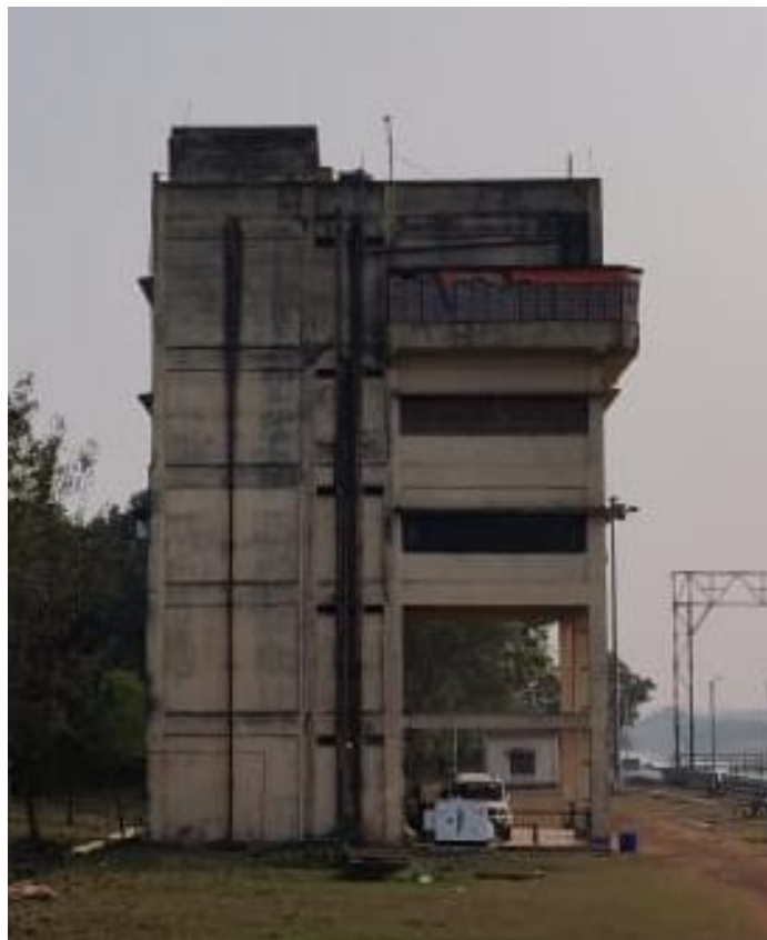
Figure 62: Control room building
