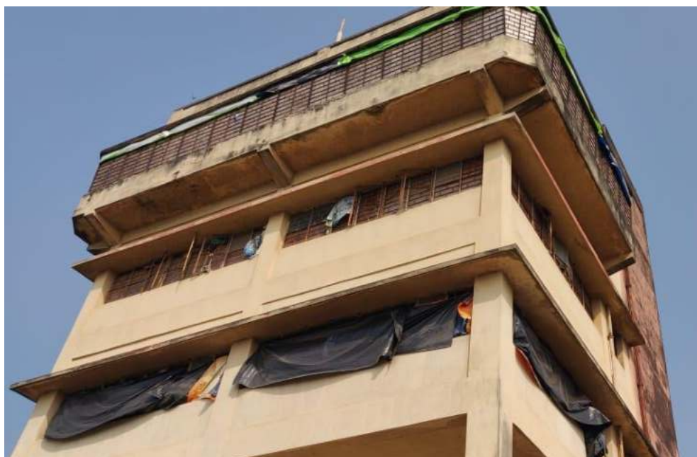
Figure 63: Control room building (Close-up view)
