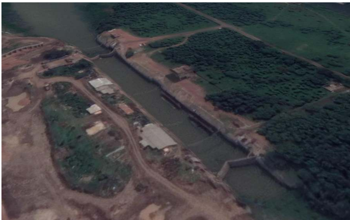
Figure 1: Image of the Farakka Navigational Lock
