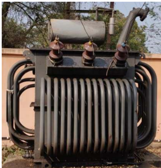
Figure 70: 11 kV to 415 V Transformer
