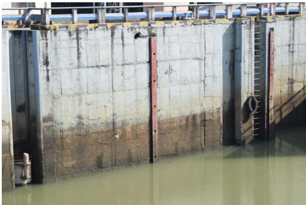
Figure 75: Wooden and rubber tyre fender arrangement
