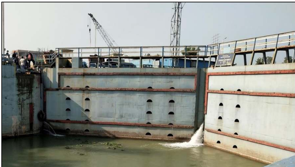
Figure 47: Mitre Gates of Farakka Lock
