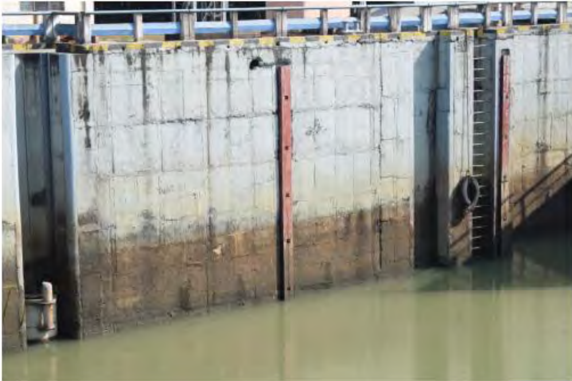
Figure 5.11 Existing wooden fender of the lock chamber
