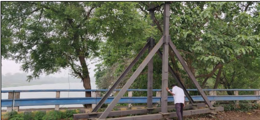
Figure 7.10 Lifting Assembly of Bulkhead Gates
