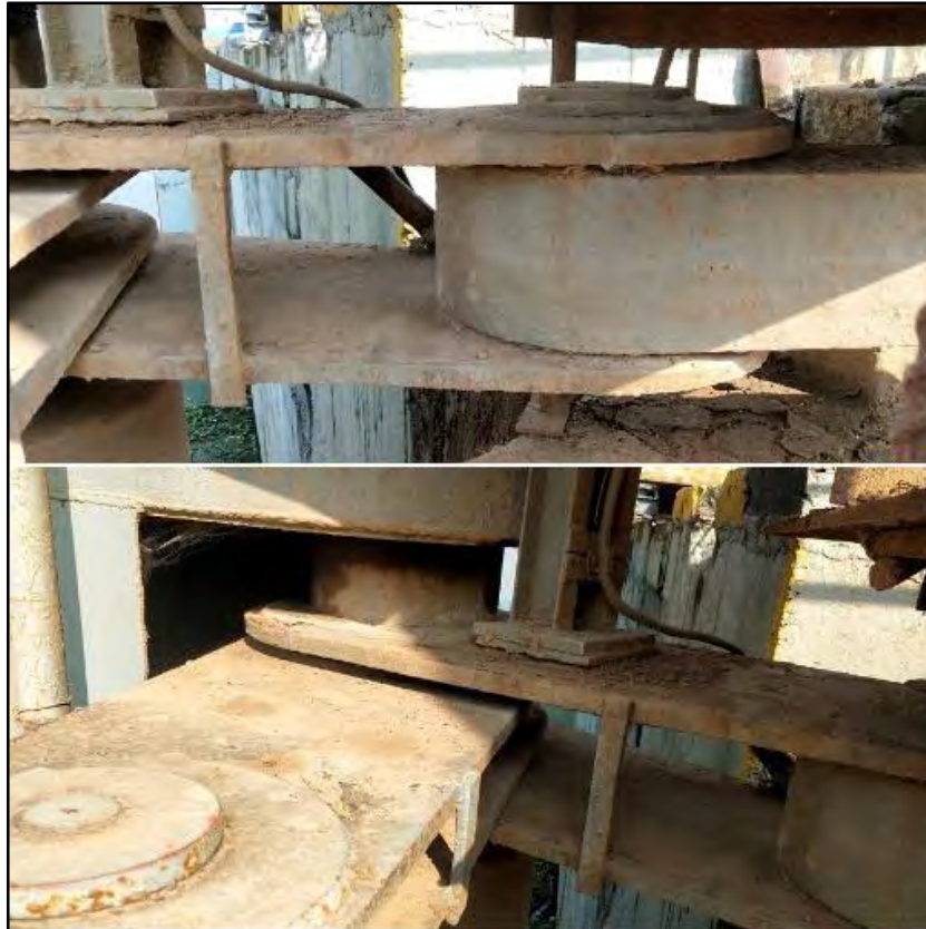
Figure 7.3 Top Bearing of Mitre Gates of Farakka Lock
