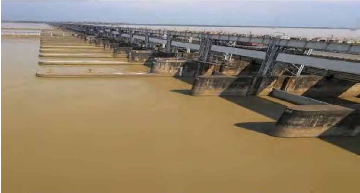
Figure 4.2 Photographs of Farakka Barrage
