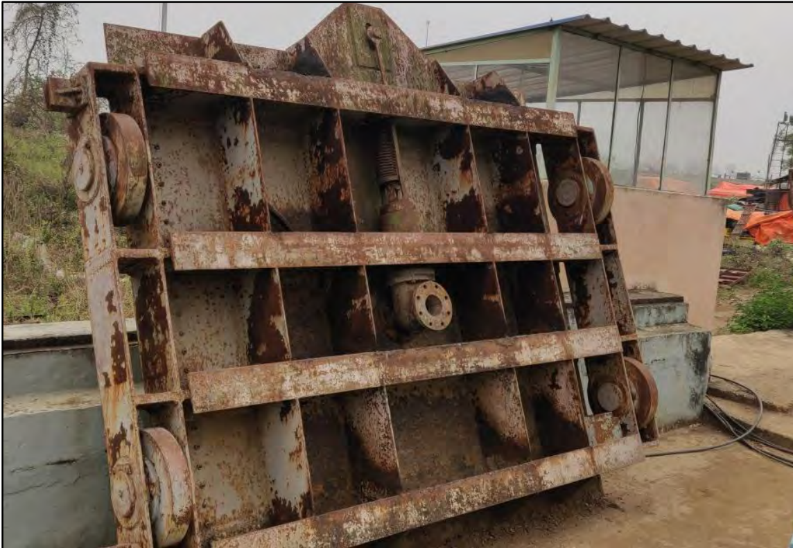
Figure 7.7 Bulkhead Gates for Radial Gate Maintenance
