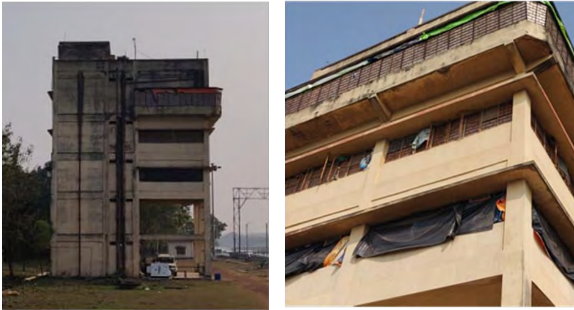
Figure 5.12 Present condition of the control room buildings
