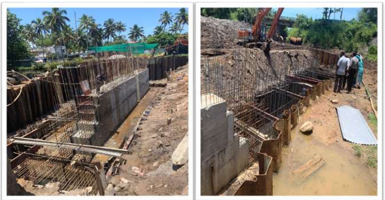
Lock wall construction under progress
